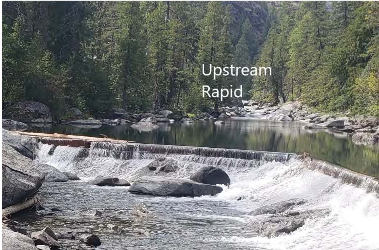
Figure 7. Photo looking upstream at the backwater pool and steep, natural rapid upstream (background) that extends approximately 1,000 ft from current diversion structure. Note the large boulders in the rapid upstream and along the banks. Photograph taken August 2019.
