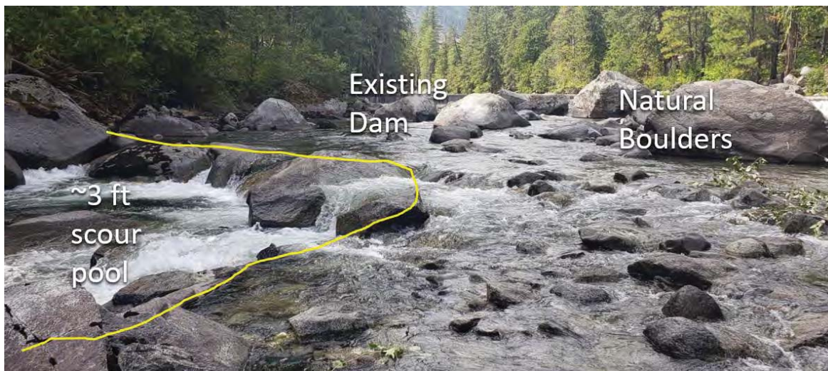
Figure 8. Downstream of the existing diversion structure a natural boulder drop of 2 to 3 ft exists (photo looking upstream) with a deep scour hole immediately downstream. Additional large boulders are present in this photo that range in diameter from 5 to 15 ft. Photograph taken August 2019.
