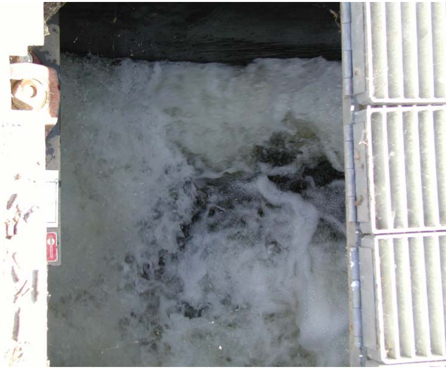
Figure 4-4. View looking inside the fish ladder pool after removal of the bar grating shows a high velocity jet shooting out of the orifice, making fish passage difficult (Reclamation photograph by P. McGowan, 2007).
