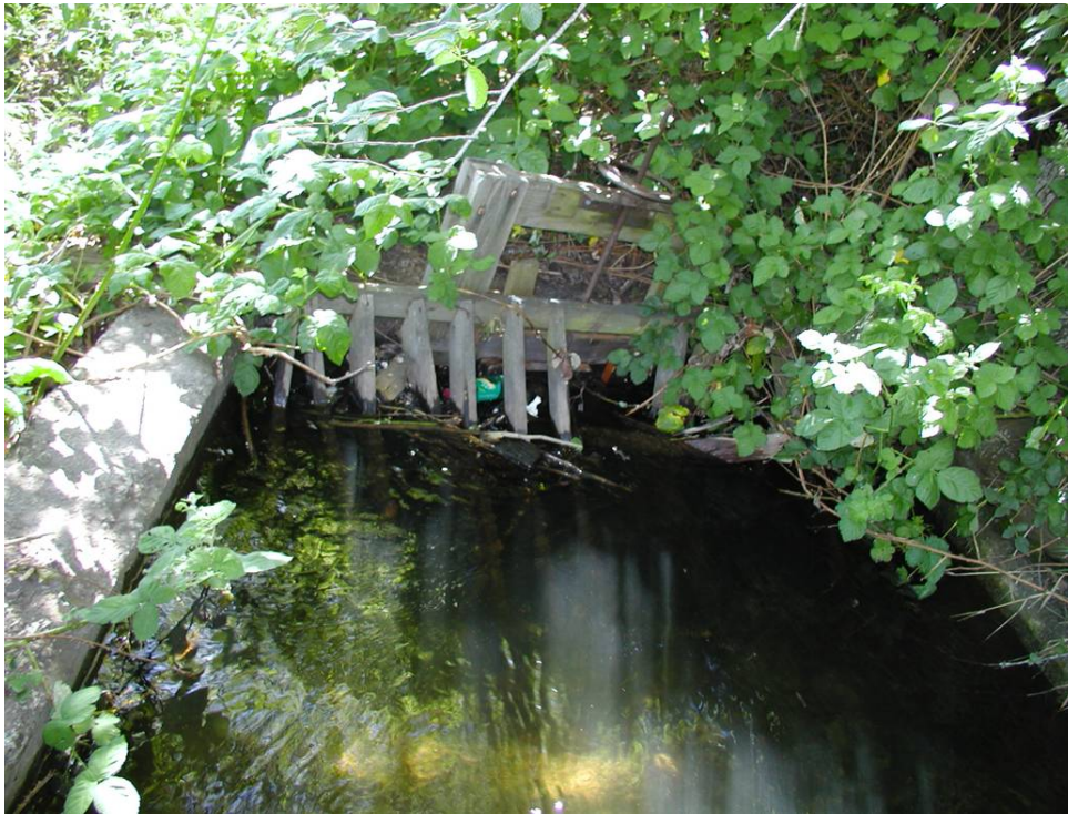
Figure 4-6. Existing headgate structure for Ashland Creek Diversion (Reclamation photograph by P. McGowan, 2008).
