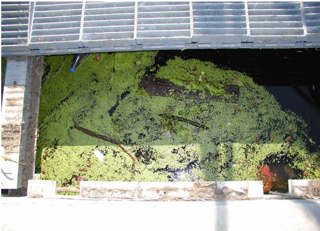
Figure 4-3. The fish passage orifice in the uppermost pool plugged by sediment and woody debris (Reclamation photograph by P. McGowan, 2007).
