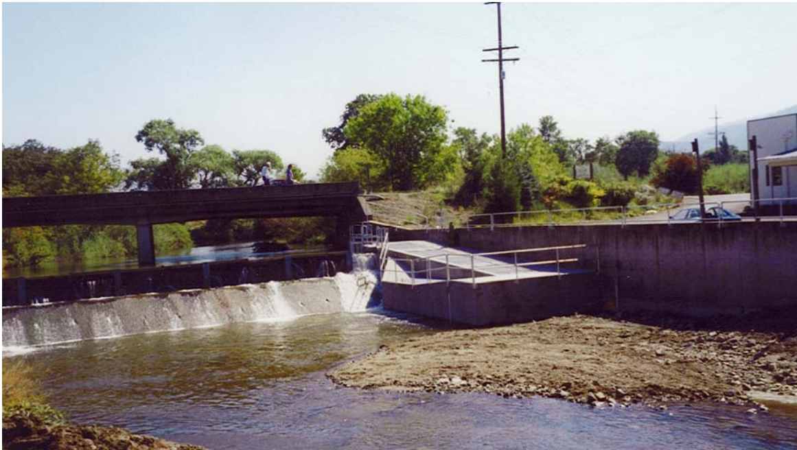
Figure 4-2. Oak Street Diversion fish ladder downstream of Oak Street Bridge also showing gravel parking area on the left side of Bear Creek (Reclamation photograph by P. McGowan, 1998).
