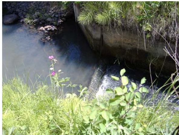
Measurement weir below pipe outlet on Webb Canal
