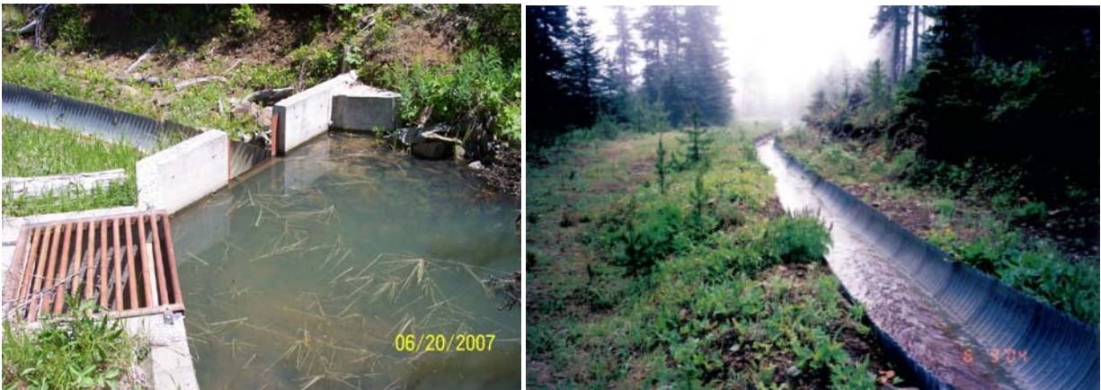
The Captain John diversion structure and a portion of the Captain John Canal
