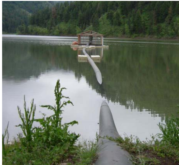
Lake Waha Pump and part of the outlet pipeline
