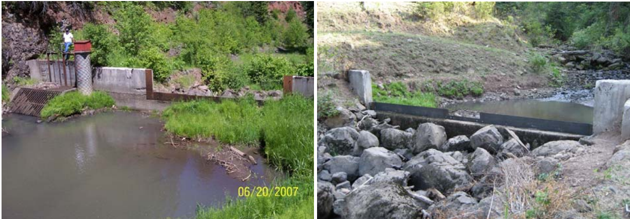
The Webb Creek diversion structure. Photo at right shows compound measurement weir on the dam crest.
