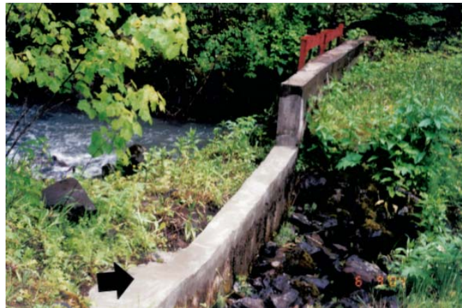
West Fork Diversion Dam
