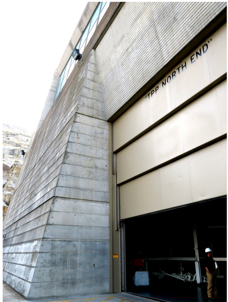
Figure 8, Above: Detail of concrete work at north service door. The form lines on the header and the new return wall will duplicate the existing appearance.
