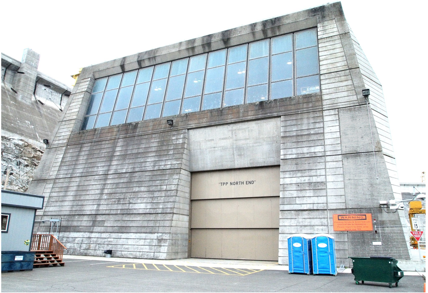
Figure 6, Above: The TPP's North end service door. Character defining features on this end are the large clerestory window and the concrete details. Figure 7, Below: Diagram summary showing work to be performed for planned expansion of the service door. Detailing and color of new concrete will match existing.
