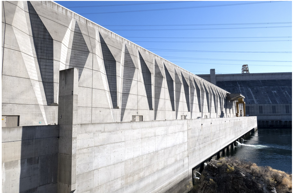
Figure 3: View of the TPP looking north showing relation to dam and important architectural character defining features, most notably Breuer's structural folded façade.
