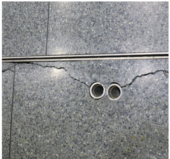
Figure 9, Below: Terrazzo floors on powerplant interior will be repaired and will match existing floors.
