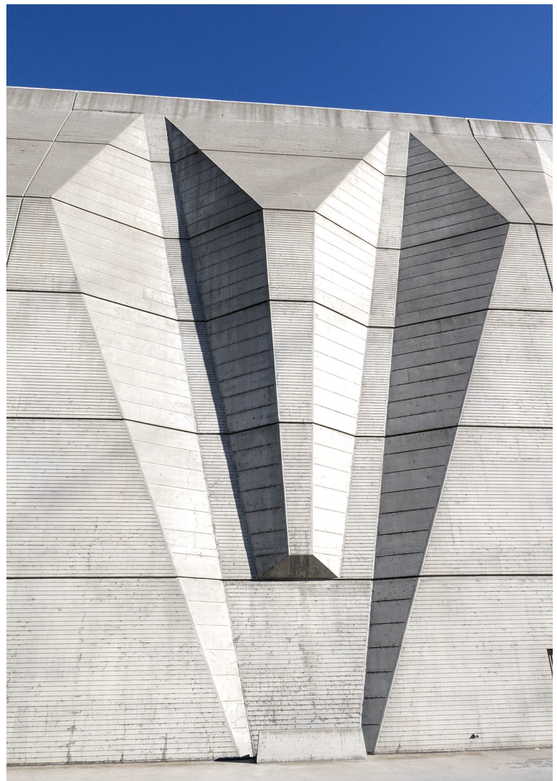
Figure 4: Detail view of TPP west façade demonstrating the play of light across Breuer's pleated panels as well as character defining concrete detailing.
