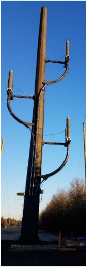
Figure A-3. Typical underground transition structure and duct bank
