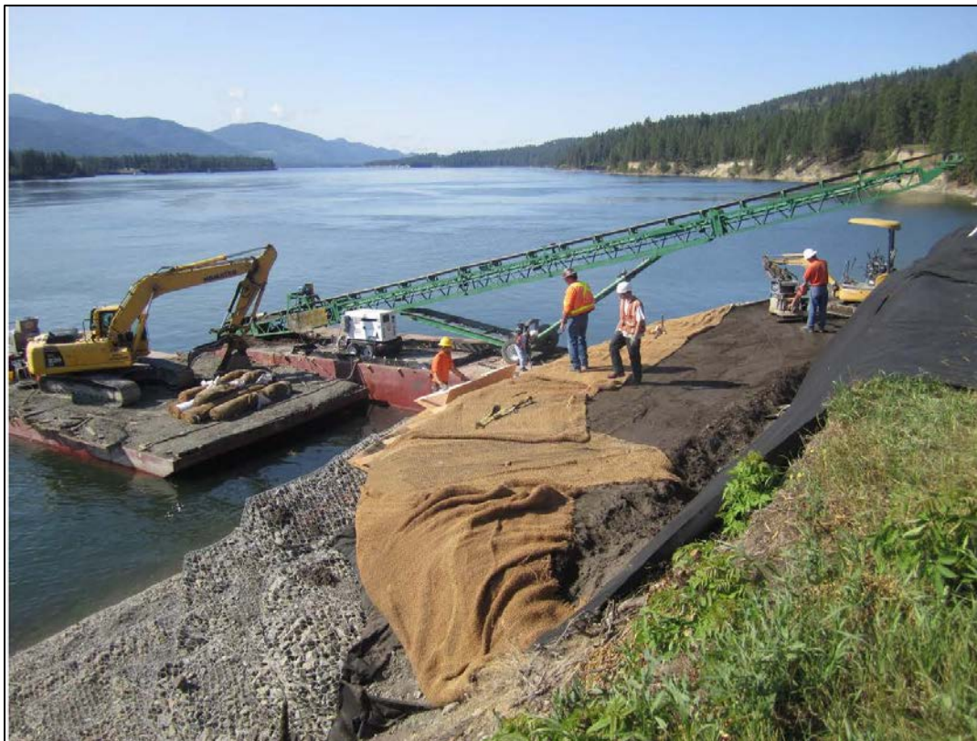
Photograph 2-1. Example of barge-based construction work
