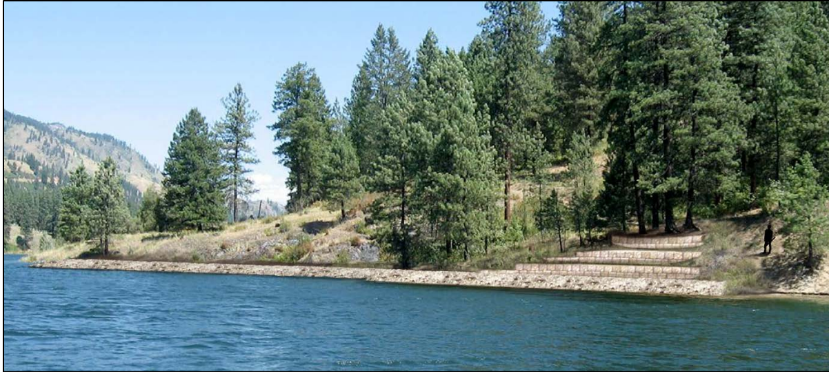
Figure 3-3. Conceptual diagram of the stabilization site with tiered retaining wall and surface-treated riprap
