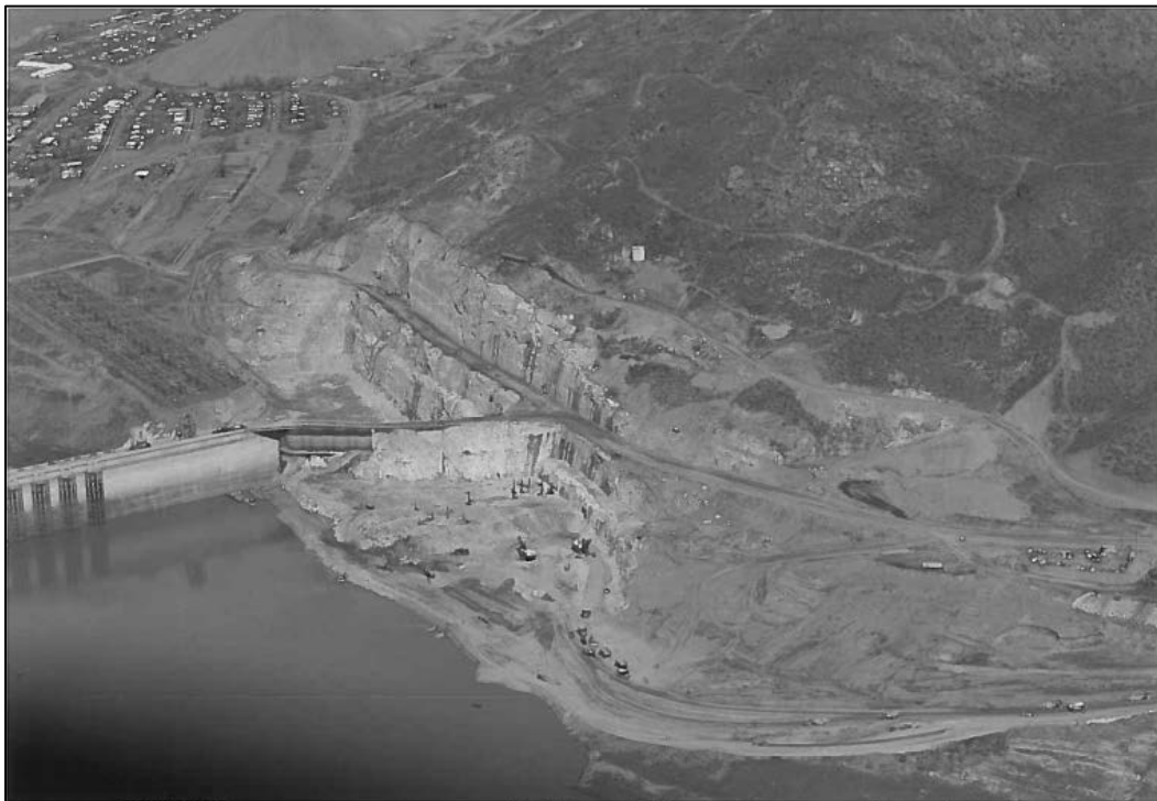
Photograph 3-1. Aerial view of the TPP excavation and haul road, taken April 7, 1969. The reservoir elevation in the photograph was 1166.9 feet.
