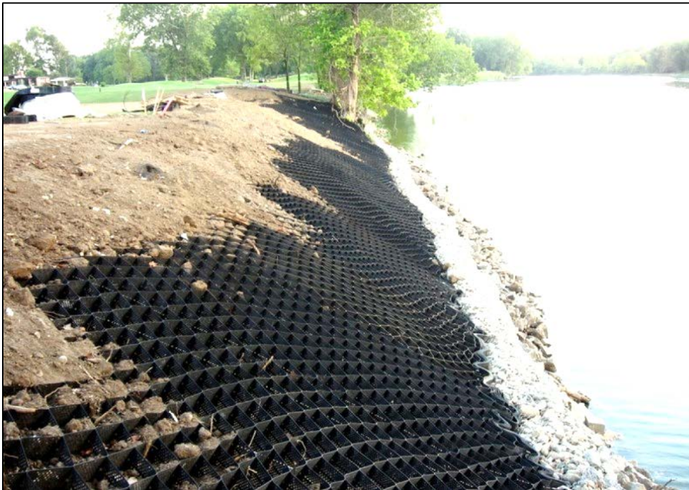
Figure 4. Slope stabilization application of Geoweb (partially constructed example)
