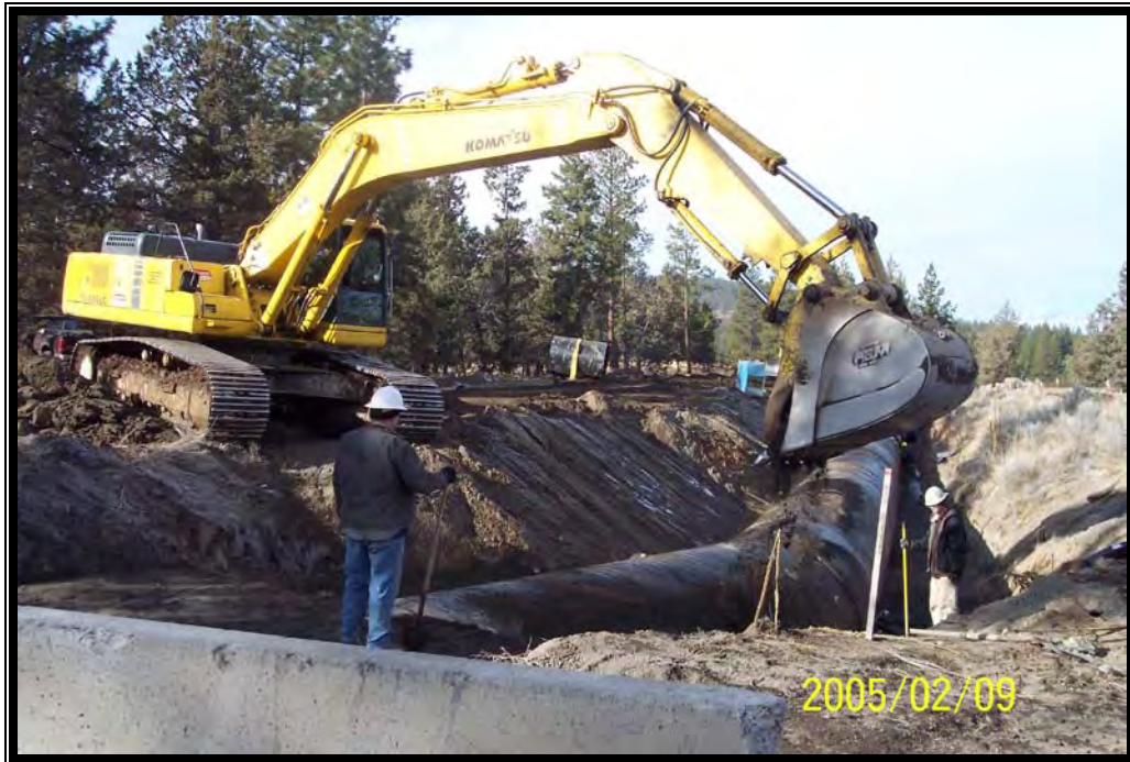
Typical pipe installation in irrigation canal – from Bend Feed Canal piping project
