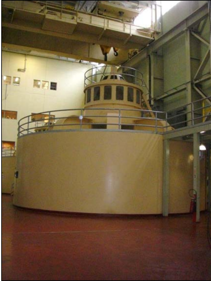
Photograph A- 1. One of four generators in the Hungry Horse Powerplant. Note the bridge cranes across the top of the photograph.
