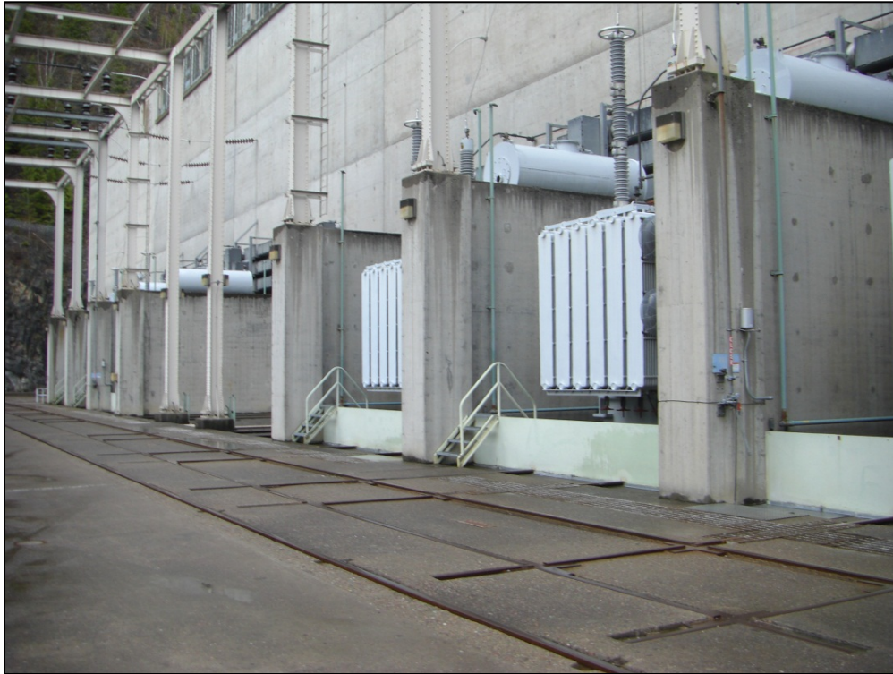
Photograph A- 4. View of the transformer deck and the transformer stalls. Note the tanks and fire-suppression sprinklers.
