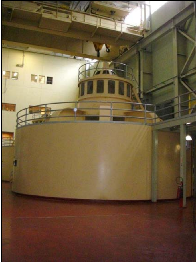
Photograph 1-1. One of four generators in the Hungry Horse Powerplant. Note the bridge cranes across the top of the photograph.
