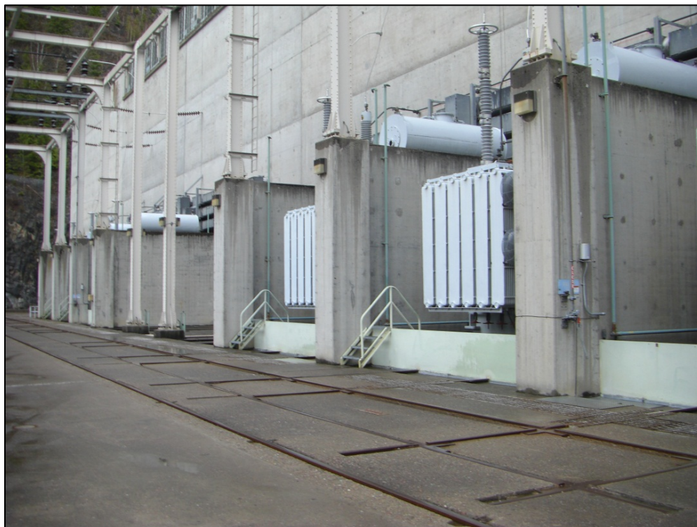
Photograph 1-4. View of the transformer deck and the transformer stalls. Note the tanks and fire-suppression sprinklers.
