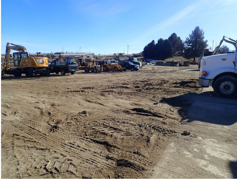
Figure 4. Major staging area near the west entrance to the BPBOC yard
