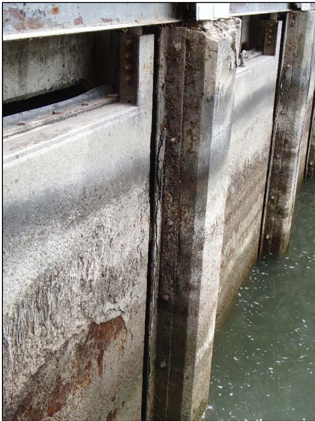
Photograph 2. View of the deterioration downstream side of the Unit 7 roller gates. Concrete spalling and lamellar corrosion (corrosion that proceeds laterally from sites of initiation along planes parallel to the surface, generally at grain boundaries) are visible on concrete and steel.
