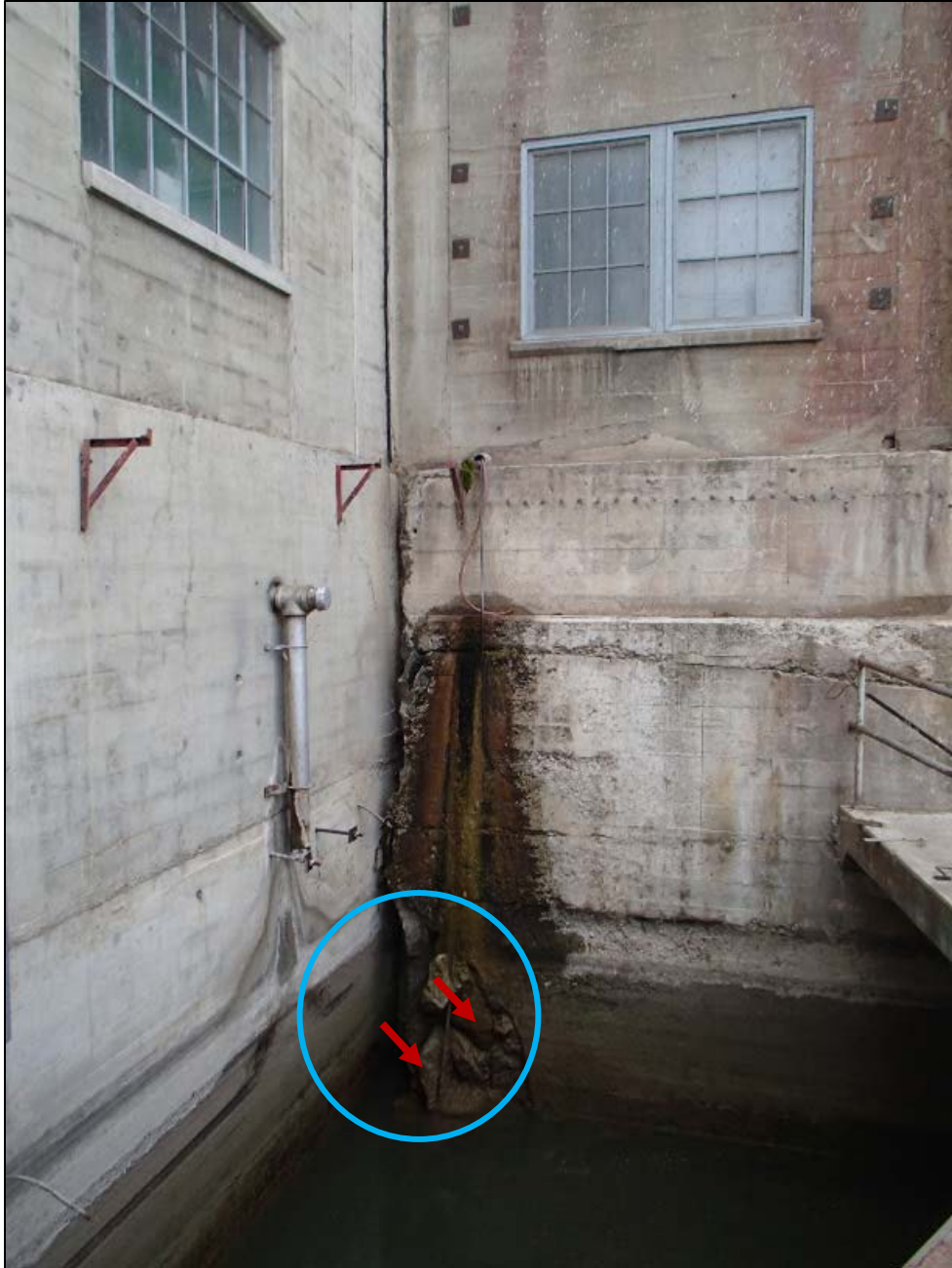
Figure 2. General view of a growing gap between the original powerhouse and the Unit 7 structure caused by ongoing deterioration of structural concrete. Sections of missing concrete and exposed rebar are highlighted by blue circle and arrow, respectively.
