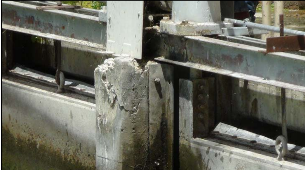
Photograph 1. This photograph, taken from the downstream side of the Unit 7 bulkhead gate structure, shows an example of the deterioration of supporting concrete present on the original pier nose.
