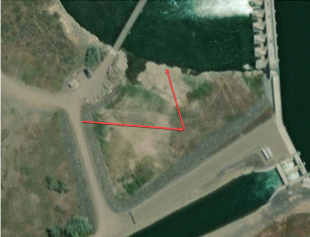
Figure 9. Aerial imagery from June 2021, with red arrows showing the approximate location of the terrestrial portion of the proposed temporary access road
