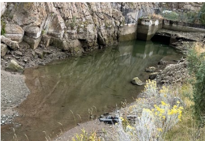
Discharge area after pumping water out.
