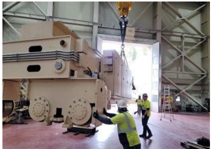
Section of new crane being hoisted into place.
