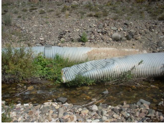
SO 20 – culverts lying in channel, Reach 2, RM 0.4
