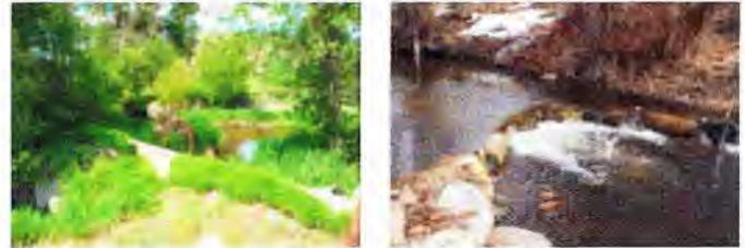
Figures 2 and 3. Before and after photographs of Beaver Creek. Left: Diversion dam in Beaver Creek that impaired or completely blocked fish passage upstream. Right: Diversion dam replaced with instream vortex weir allowing fish passage and maintaining ability to divert water for irrigation.
