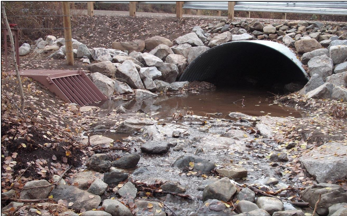
Figure 2. A barrier road culvert on Poorman Creek, as well as an irrigation diversion immediately downstream of the culvert, were replaced in 2009 with a natural-bottom culvert and rock vortex weir that allow passage at all flows. Photo from Reclamation.
