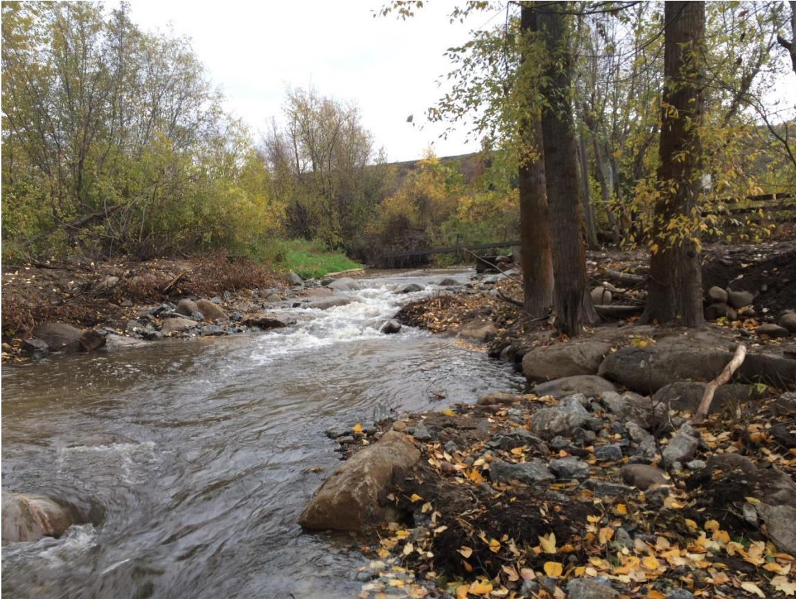
Figure 34. Roughened channel constructed to replace a barrier at one of the Fort Thurlow diversions. Photo provided by Reclamation.
