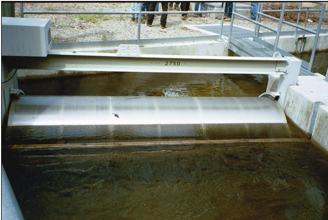
Figure 3. Upgraded diversion with fish screen on the Chewuch River.
