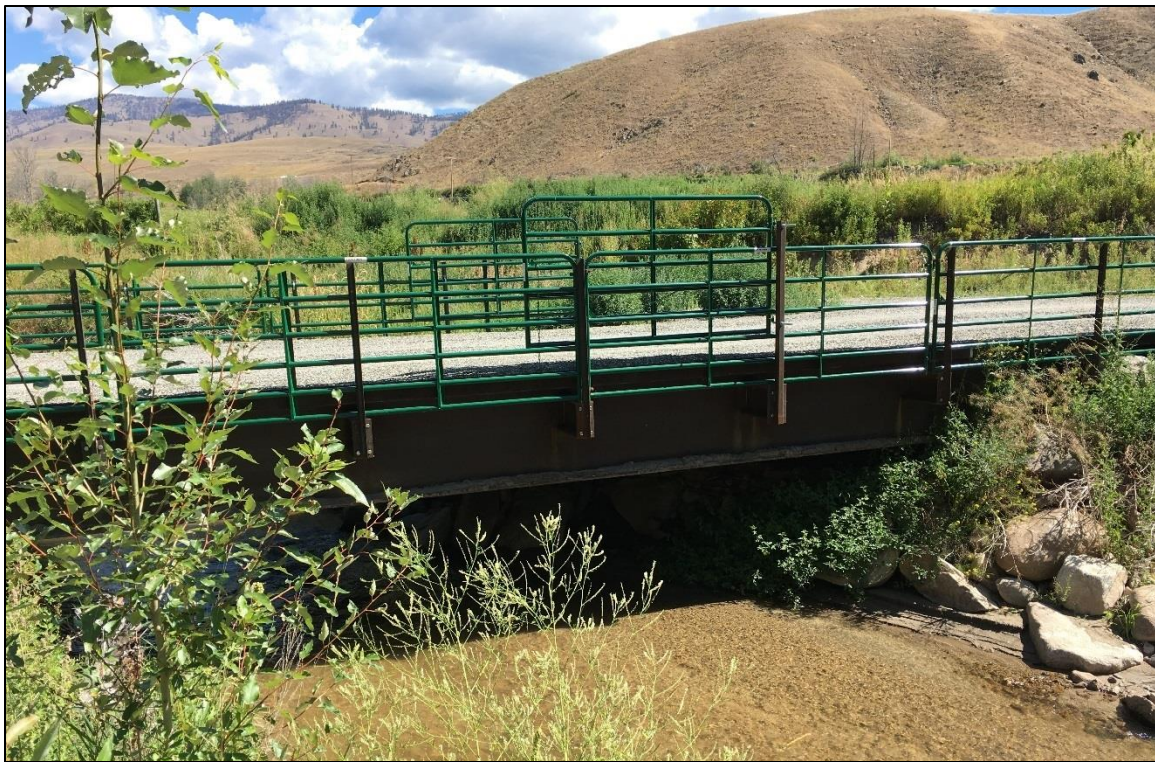
Figure 4. Failing double culverts were replaced with a channel spanning bridge on Beaver Creek to improve fish passage and geomorphic process.
