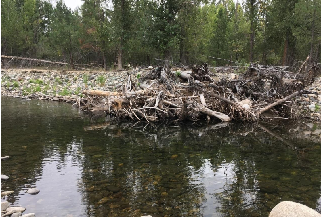
Figure 5. Constructed large wood jam at Whitefish Island, mainstem Methow River (photo by Inter-Fluve 2016).
