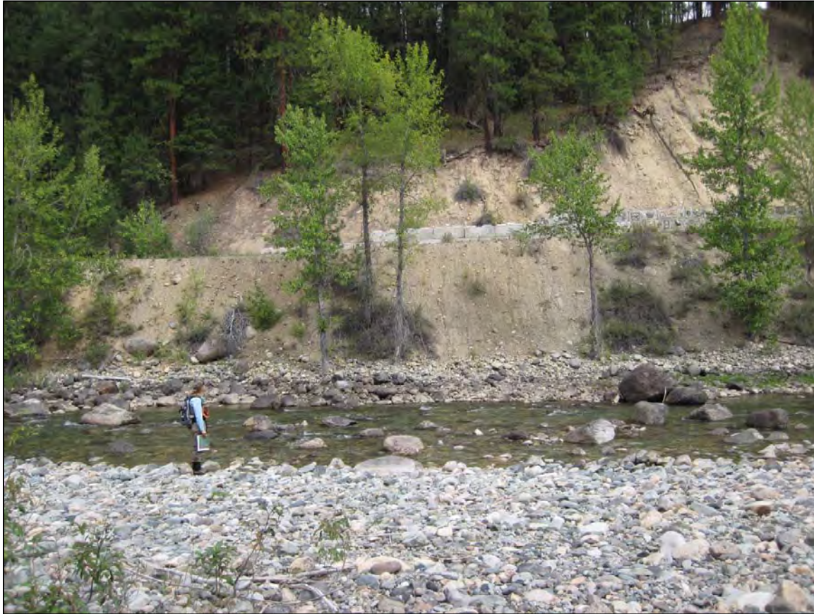
Figure 41. Cut bank of glacial outwash terrace on river-left at RM 64.55. Old road grade cut into the bank with cement retaining wall for preserving community trail access. (9/3/2014)
