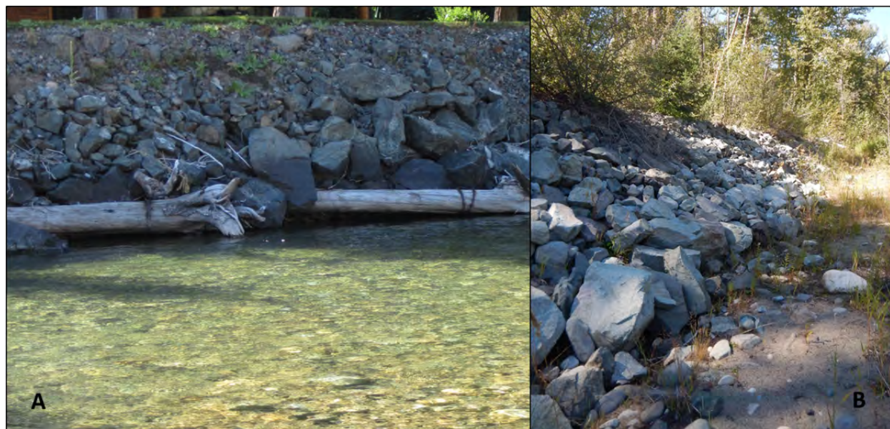
Figure 46. Examples of confining features constructed of large angular riprap in Reach 2, (A) riprapped bank with cabled and anchored logs on river-right at RM 62.7; (B) section of the levee composed of riprap on river-right at RM 63.5. (9/4/2014)
