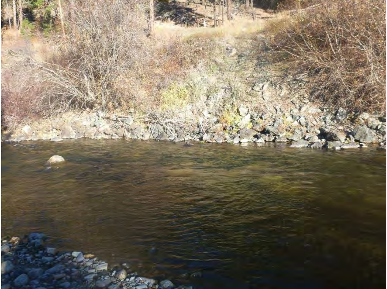
Figure 46. RM 10.27 river left, the road embankment and large angular riprap installed at the bank toe.
