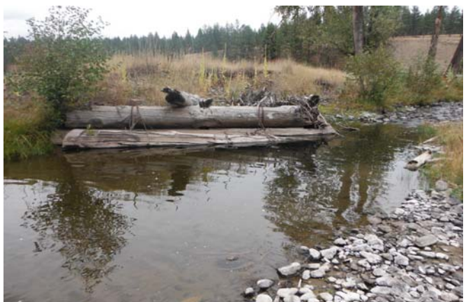
Reach 15 - Unit 702 - Cabled logs form a habitat structure
