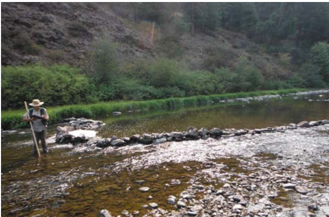
Reach 9 - Unit 537 - Human-built step-over-structure pools water.
