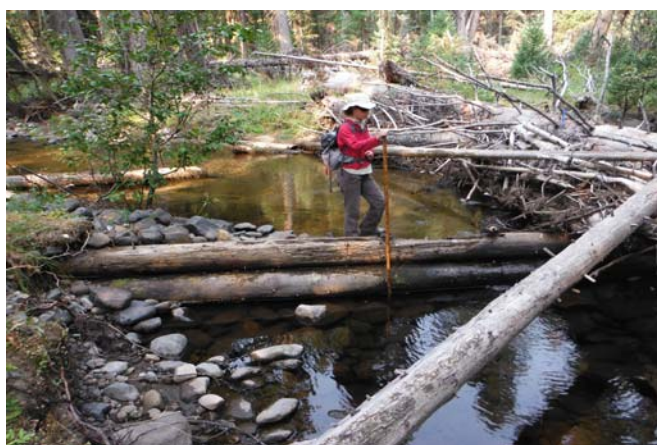
Reach 24 - Unit 1679 - Due to the summer low flows, this habitat structure was poised to be a potential barrier to fish movement. Water flowed through the structure, but not over it.
