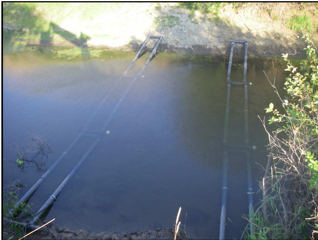
Fig. 1: Antenna configuration of the PIT tag interrogation system installed at the Johnson site.
