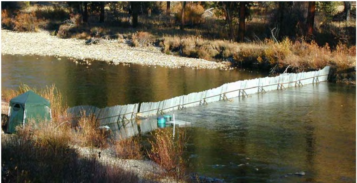
Photograph No. 3. Temporary weir installed on North Fork of the Boise River, Idaho.
