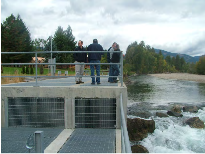
Photograph No. 1. Site visit at Foghorn Dam.
