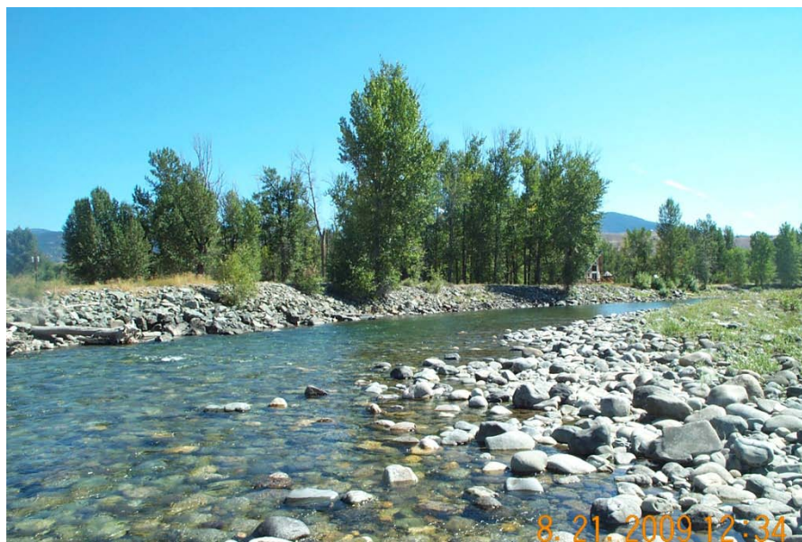
Photograph No. 30. View to the east looking downstream at riprap placed along river left. W2 Assessment – Methow Subbasin, Washington – Bureau of Reclamation Photograph by E. Lyon, August 21, 2009.
