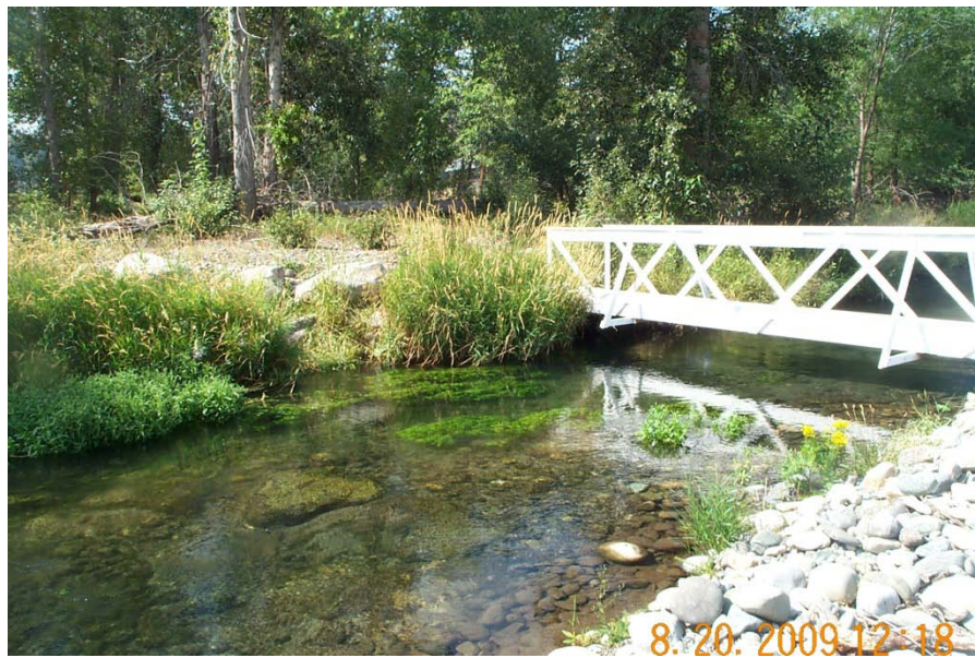
Photograph No. 8. View to the west looking upstream at foot-bridge along the Winthrop Hatchery side channel. Note riprap along river right and grade-control structure in stream. W2 Assessment – Methow Subbasin, Washington – Bureau of Reclamation Photograph by E. Lyon, August 20, 2009.
