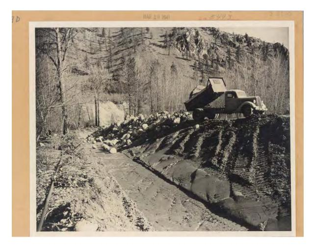
Figure 3. Entiat National Fish Hatchery Complexity. Photo of the levee construction in March 1941. The levee appears to have been constructed of native floodplain material and armored with coarse rock.
