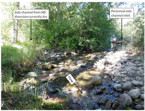
Figure 21. Hanan-Detwiler Diversion. Confluence of the dry fish return channel and a perennial side channel of the Entiat River. The dry channel is over 1,500 feet long and is dependent on the Hanan-Detwiler diversion for water.
