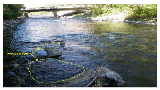
Figure 40. Fire Station Weirs. Photo of upper Fire Station weir taken September 2011 at low flow (about 400 cfs), illustrating where two header rocks were moved out of the weir. Several header and footer rocks were moved from this weir by high flows.
