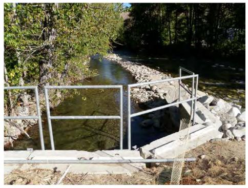
Figure 12. Knapp-Wham Diversion. Photo looking upstream at the new Knapp-Wham headworks and wing-dam (September 2011).
