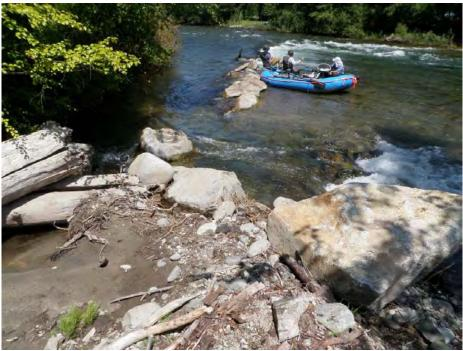
Figure 20. Hanan-Detwiler Diversion. Photo taken July 2011 looking upstream where boulders were relocated from the structure in order to plug the diversion at the site of the diversion headworks.
