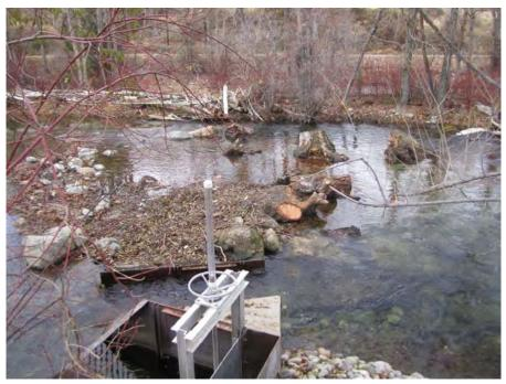
Figure 63. Below the Bridge. Photo taken in November 2011 from the right bank at the point of diversion showing the diversion structure after the excess woody debris had been cleared and the incorporated root wads were trimmed. Most of the wood in the photo is loose debris that was removed from the structure and will be mobilized in the next high-flow event.
