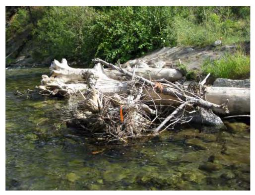
Figure 51. Milne. Photo of double root wad log structure showing the pool maintained at apex of root wads. Photo was taken at low flow in September 2010.
