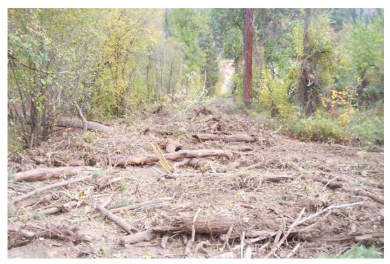
Figure 5. Entiat National Fish Hatchery Complexity. Photo of slash scattered across the footprint of the levee following removal. Photo taken in September 2011.
