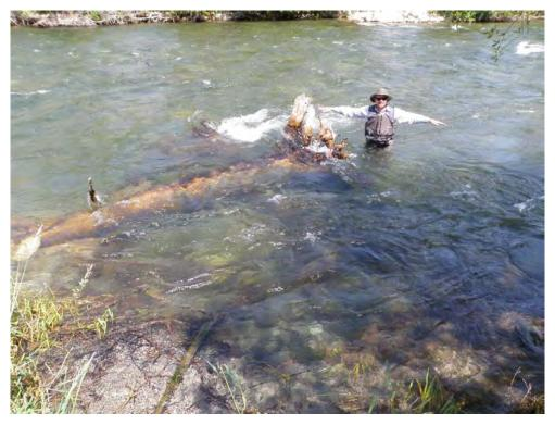
Figure 50. Milne. Single 2-log rootwad structure along the right bank (photo taken September 2011 at about 1,000 cfs).
