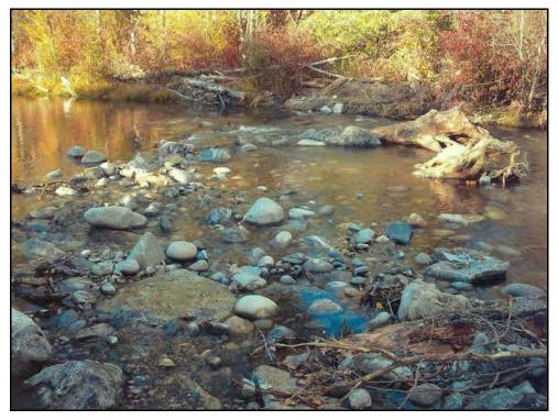
Figure 57. Below the Bridge. Photo of the rock and log diversion structure taken immediately after construction in 2010. Flow is from left to right, and the point of diversion and sediment sluice are located out of the photo below the frame. Note three of the incorporated root wads, two in the background and part of one visible in the foreground.
