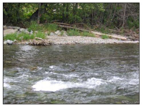
Figure 42. Fire Station Weirs. Photo taken at low water in 2006 illustrating gravel deposition on the left bank in the lee of the lower weir partially burying the LWM structure in this location. The top of the root wad can be seen on the left side of the photo.
