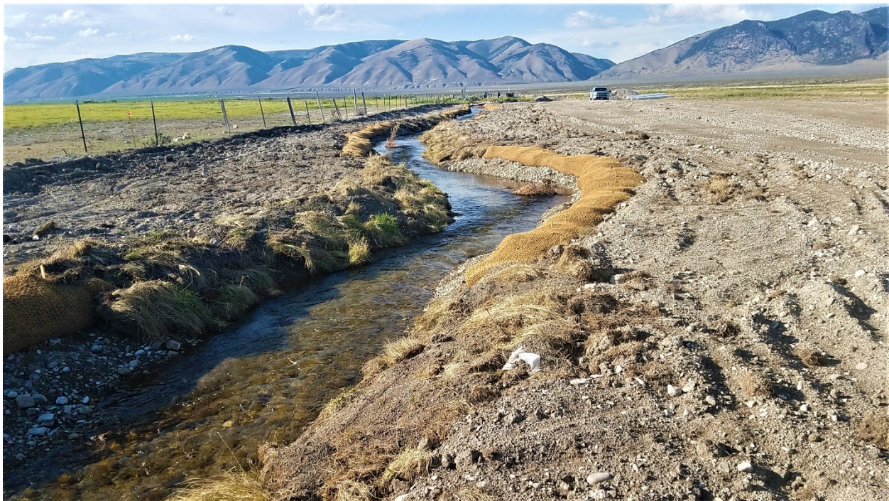
Photograph 4: The newly constructed Eighteenmile Creek channel, which will provide a more efficient stream function. (Middle Eighteenmile Creek Habitat Improvement Project) (Reclamation/Brian Hamilton)
