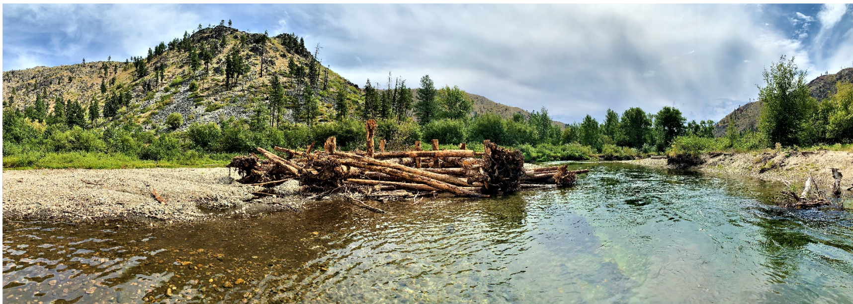
Photograph 33: The large wood structures were constructed in key locations to encourage flows onto the floodplain and side channels. When a river accesses the floodplain, key rearing habitat for juvenile salmonids is available. (Middle Entiat, Gray E) (Reclamation/Steve Kolk)
