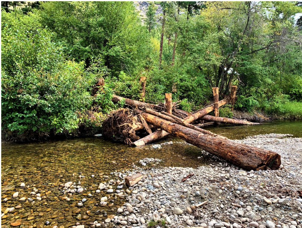
Photograph 31: Large woody material was engineered in key locations to encourage flows into side channels, which improves stream processes and habitat. (Middle Entiat, Gray E) (Reclamation/Steve Kolk)
