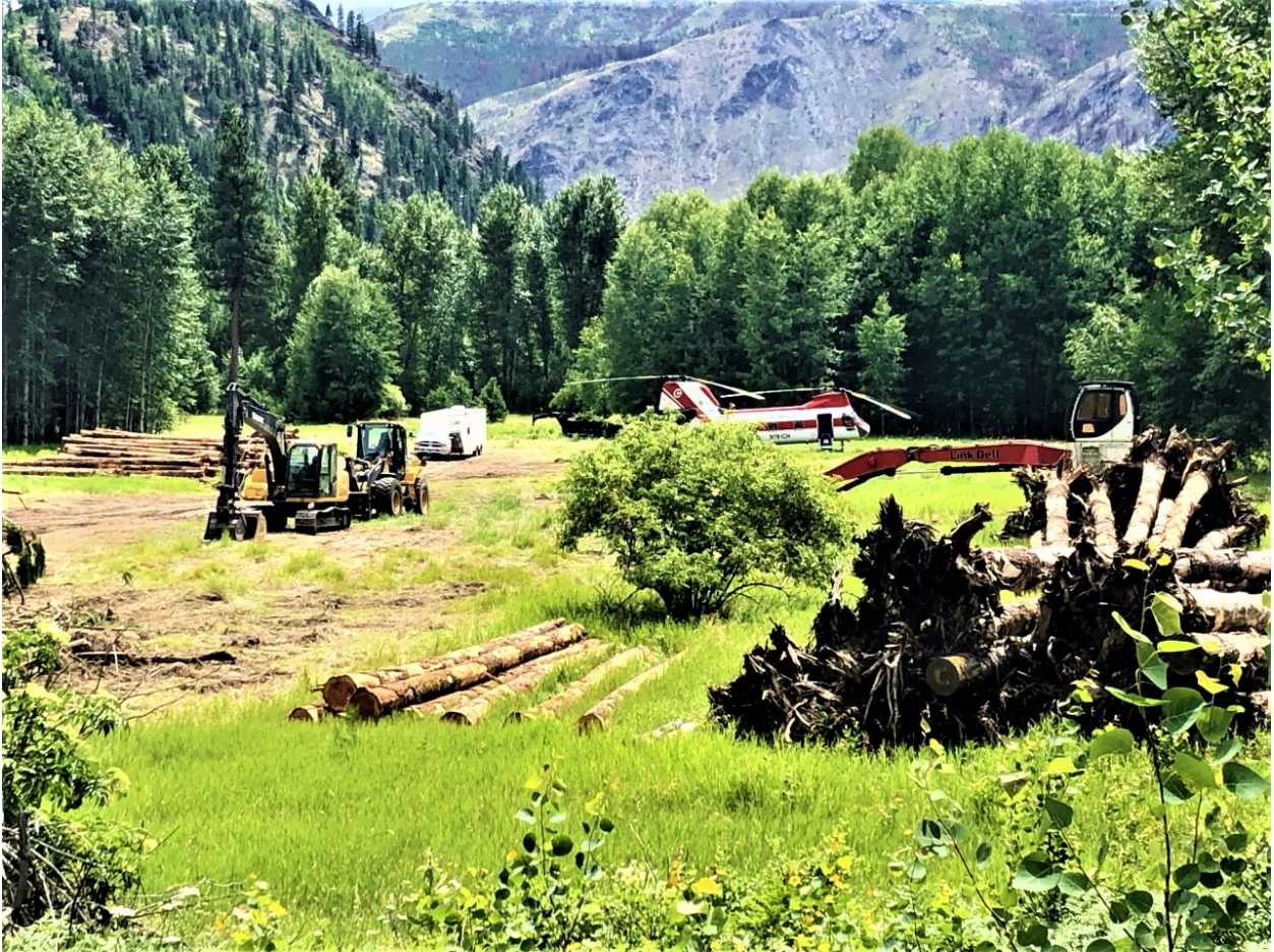
Photograph 27: Large wood was staged and transported to the individual structure sites via helicopter. (Middle Entiat, Stormy B) (Reclamation/Steve Kolk)
