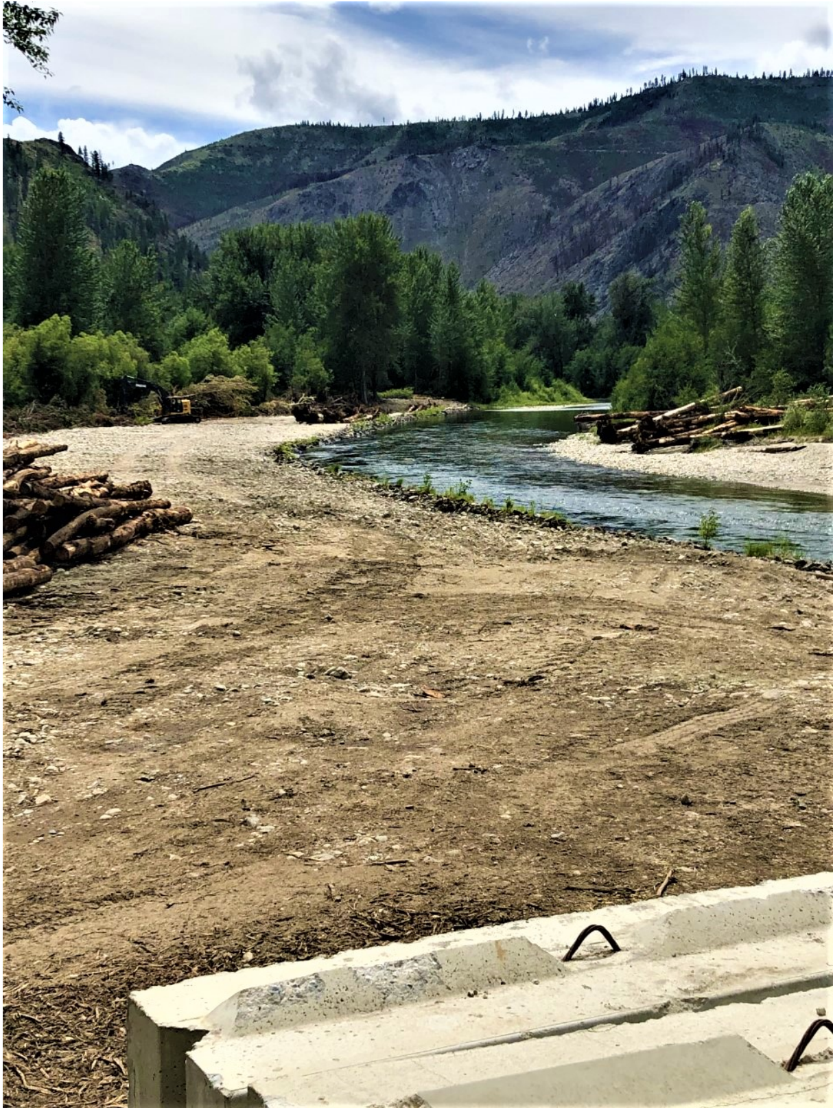
Photograph 28: Throughout the project, levees were removed down to the level of the natural floodplain. This allows the river greater access to improve habitat on the floodplains. (Middle Entiat, Stormy B) (Reclamation/Steve Kolk)
