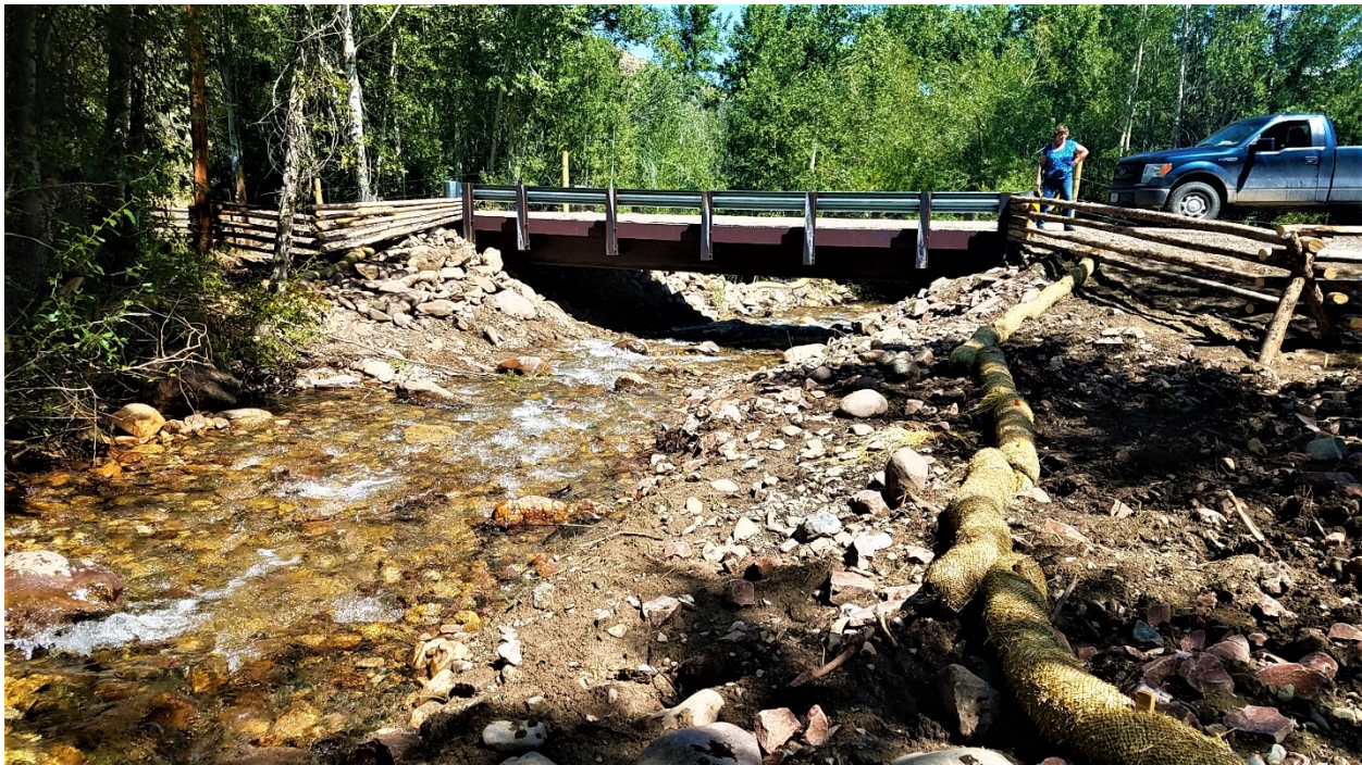
Photograph 8: This post-project view looking downstream shows the newly constructed bridge. The project now provides passage for adult and juvenile salmonids all year. (Garden Creek - Chipmunk Hill Culvert Removal) (Reclamation/Brian Hamilton)
