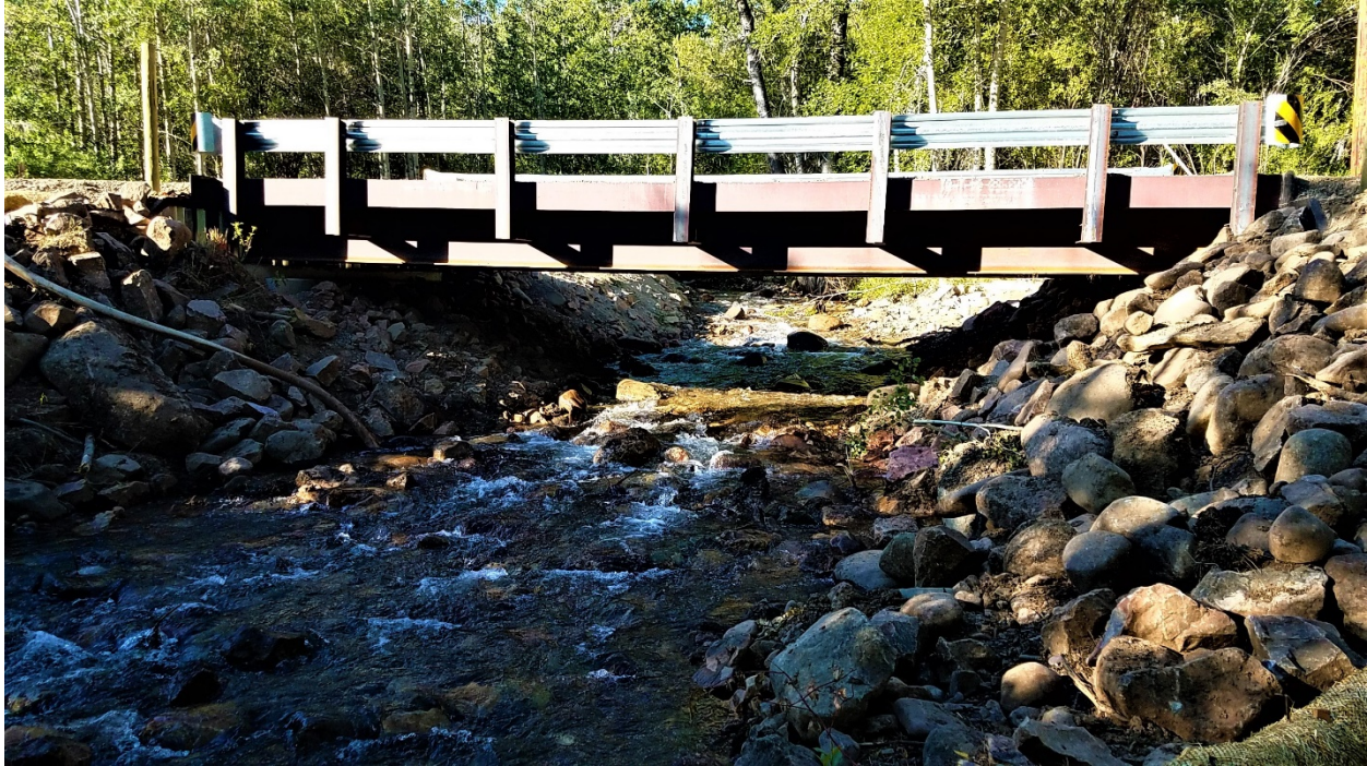
Photograph 7: This post-project view shows the newly constructed bridge, which now allows fish passage into the upper reaches of Garden Creek. (Garden Creek - Chipmunk Hill Culvert Removal) (Reclamation/Brian Hamilton)
