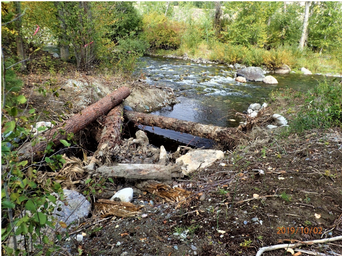
Photograph 35: This view shows the completed entry to the side channel. The side channel activates during low and high flows, providing valuable rearing habitat. (Twisp River Floodplain Phase II) (Reclamation/Steve Kolk)
