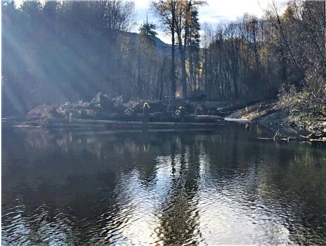
Photograph 23: This large wood structure ensures flow into the newly constructed side channel on the river right. (Middle Entiat, Stormy A) (Reclamation/Steve Kolk)
