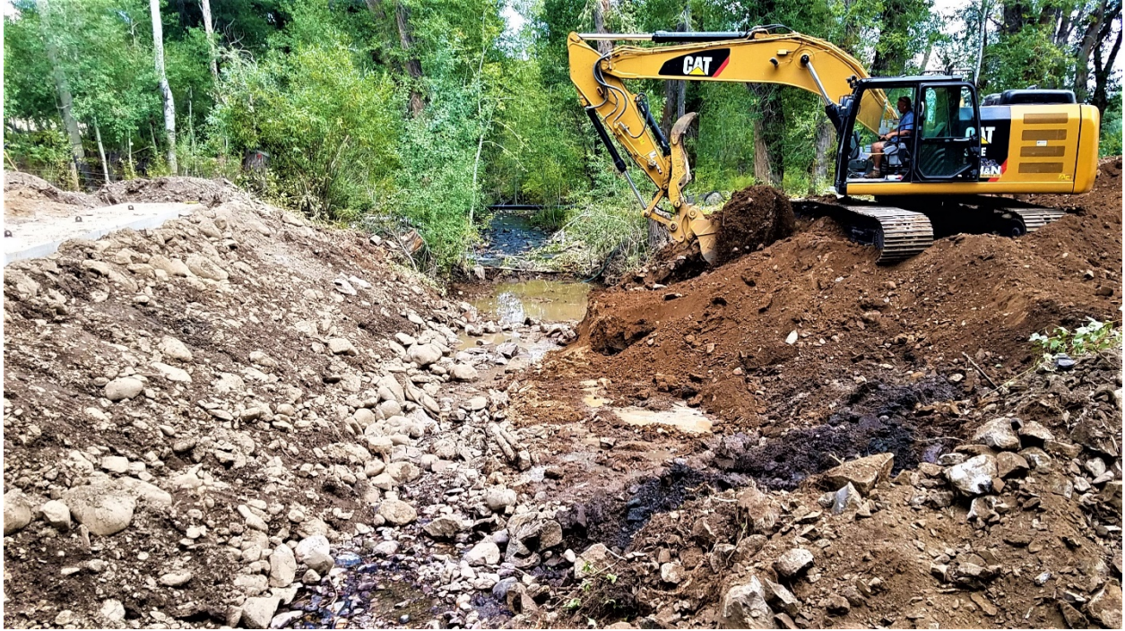
Photograph 11: Excavation on the new channel where the old culvert was removed. (Garden Creek - County Road Culvert Removal) (Reclamation/Brian Hamilton)
