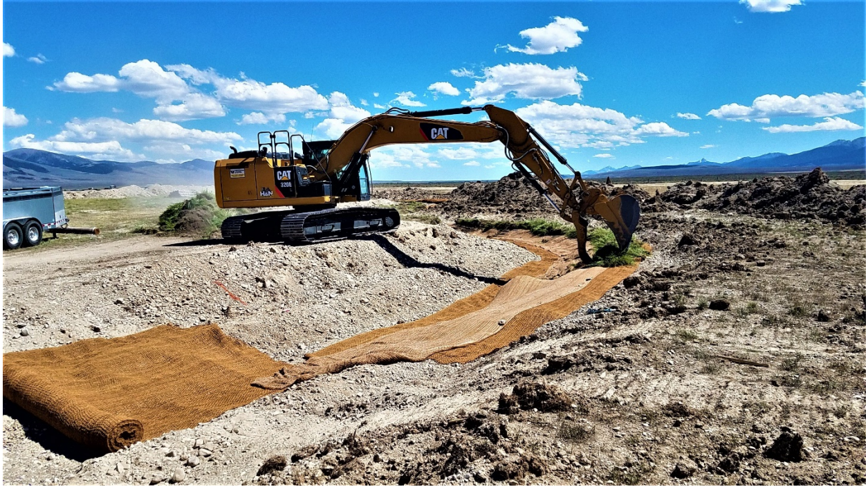
Photograph 1: Excavator placing sod mats on the fabric that forms the outside bends of the newly excavated channel. (Middle Eighteenmile Creek Habitat Improvement Project) (Reclamation/Brian Hamilton)
