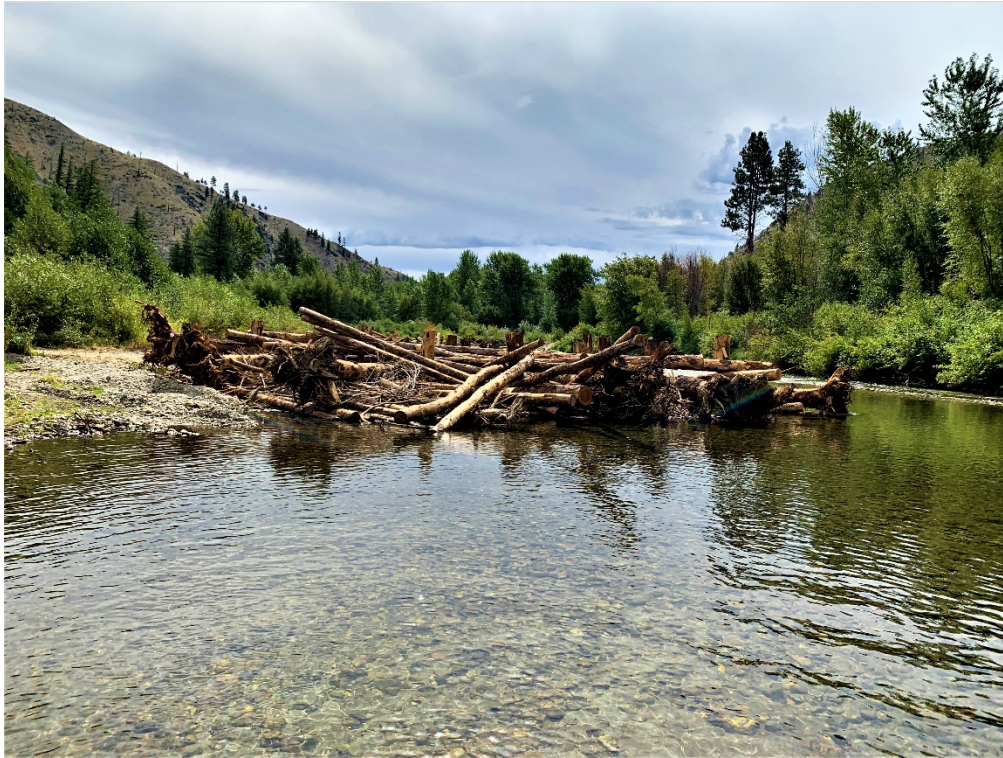
Photograph 30: Large woody material was placed in-stream to improve stream dynamics, provide habitat, and narrow the channel to allow the river to access the floodplain. (Middle Entiat, Gray E) (Reclamation/Steve Kolk)
