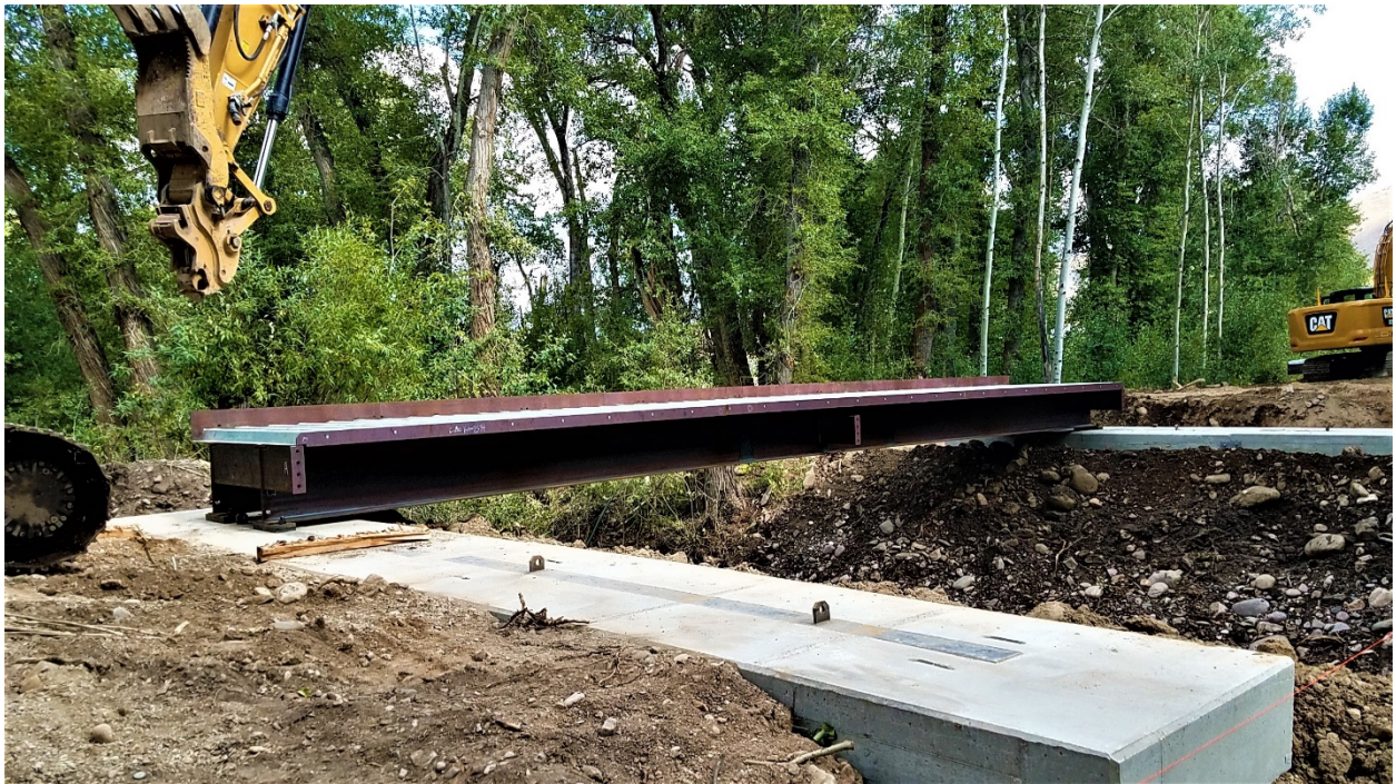
Photograph 12: The first section of the new bridge resting on the concrete footers. There were four sections of the bridge, which were bolted together after placement. (Garden Creek - County Road Culvert Removal) (Reclamation/Brian Hamilton)
