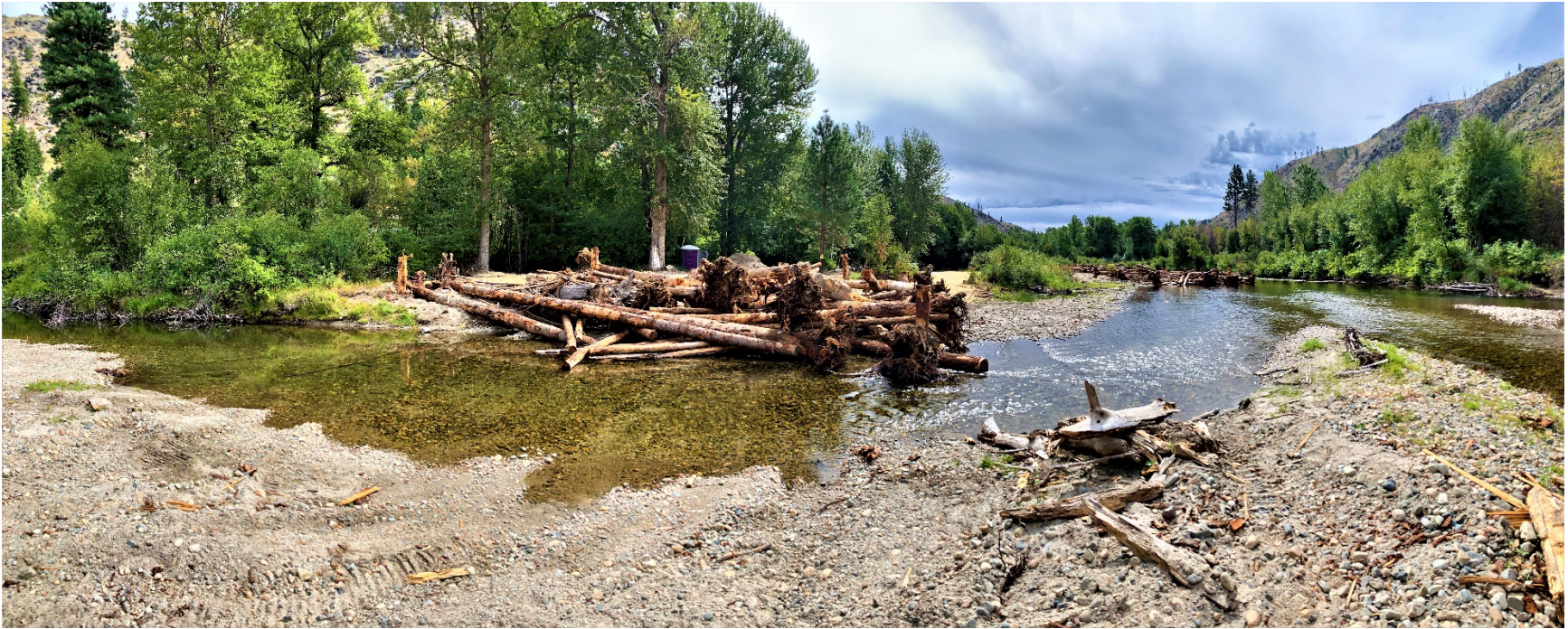
Photograph 32: Construction of the large wood structures involves driving vertical timbers to help stabilize the more horizontal portions of the structure. Root wads have proven to be crucial to the function of the large wood structures. (Middle Entiat, Gray E) (Reclamation/Steve Kolk)
