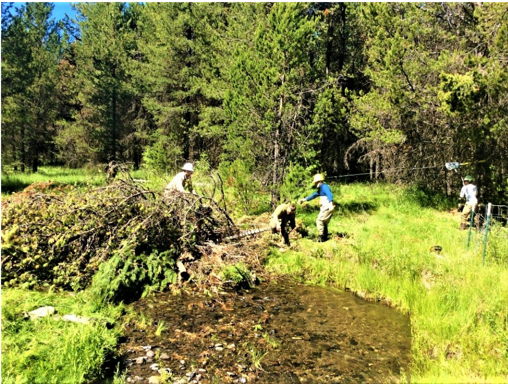
Photograph 20: This view shows a hand crew using grip hoists to drag large trees into the stream. The large woody material will provide cover and refuge for salmonids and improve stream function. (Sheep Creek Habitat Enhancement Phase I) (Reclamation/AI Simpson)
