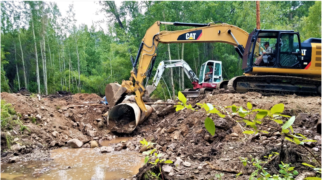
Photograph 6: This view shows the removal of the Chipmunk Hill culvert. (Garden Creek - Chipmunk Hill Culvert Removal) (Reclamation/Brian Hamilton)
