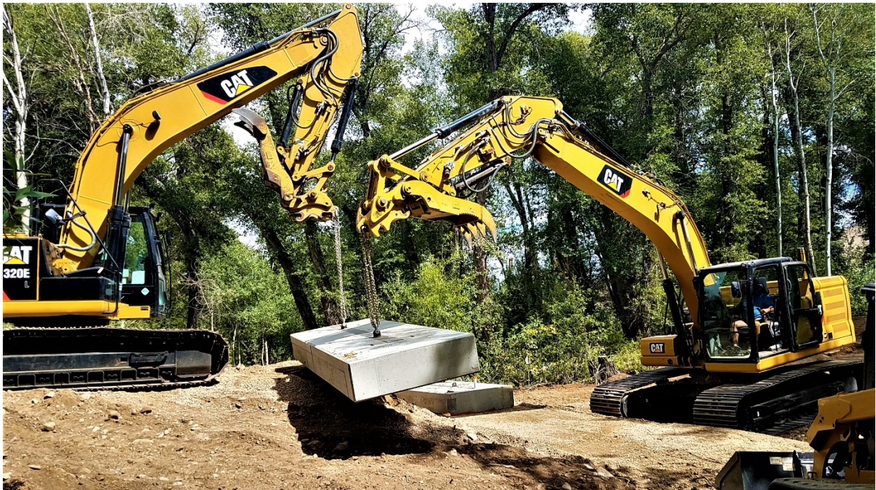
Photograph 10: Placement of the pre-cast concrete footers for the new bridge. (Garden Creek - County Road Culvert Removal) (Reclamation/Brian Hamilton)
