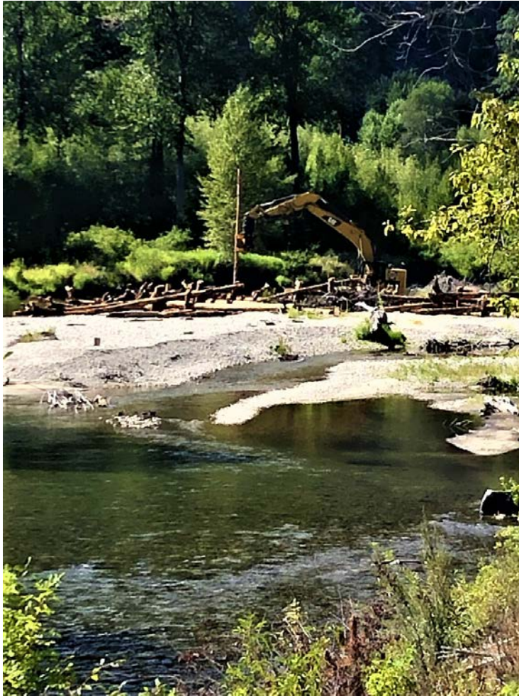
Photograph 24: This view shows the typical construction of the engineered log jams in the project area. (Middle Entiat, Stormy A) (Reclamation/Steve Kolk)
