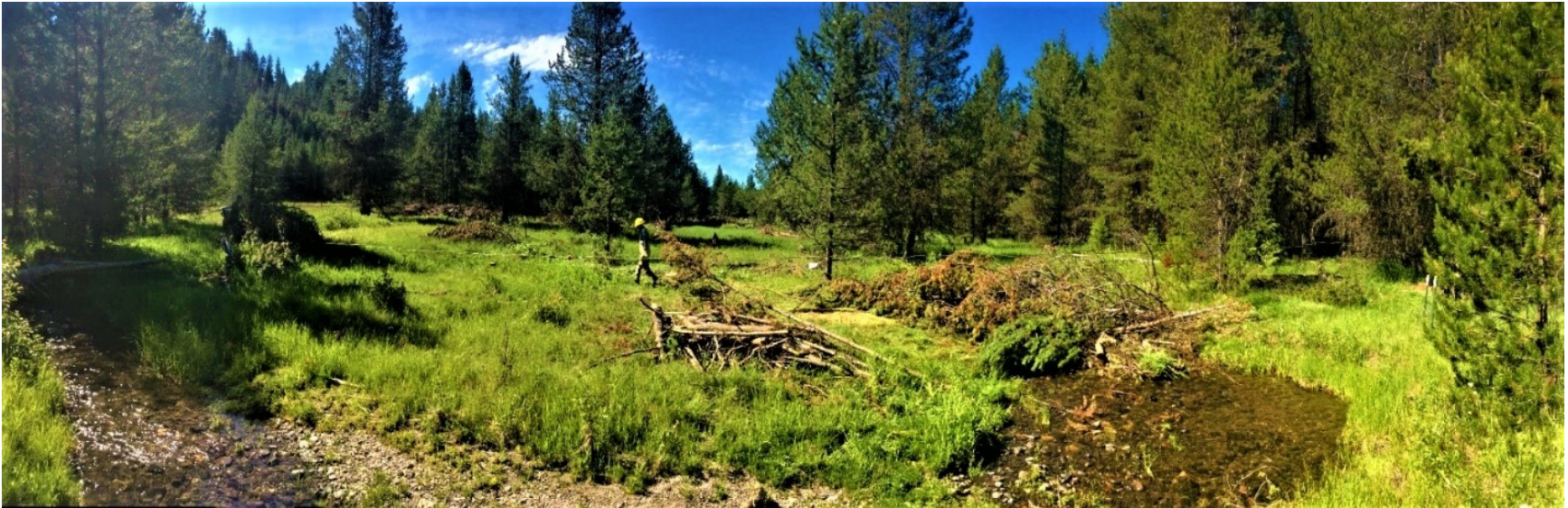
Photograph 22: Completed large woody debris structure constructed by a hand crew. (Sheep Creek Habitat Enhancement Phase I) (Reclamation/Al Simpson)
