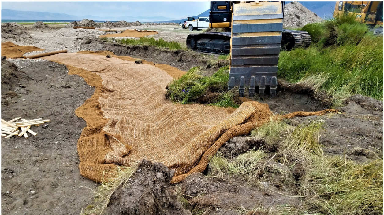
Photograph 2: Fine and coarse layers of fabric were wrapped around sod mats excavated from the banks of the old channel. The sod mats contained sedges, grass, and small willows to help form the riparian zone of the newly constructed channel. (Middle Eighteenmile Creek Habitat Improvement Project) (Reclamation/Brian Hamilton)
