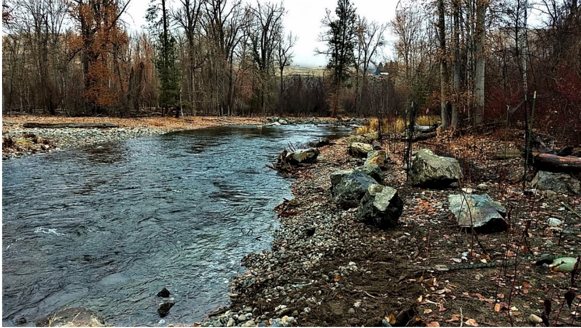
Photograph 34: The right bank levee was removed in this area, which will allow access to the floodplain. This view shows the riparian plantings and roughness added to the right bank. (Twisp River Floodplain Phase II) (Reclamation/Steve Kolk)
