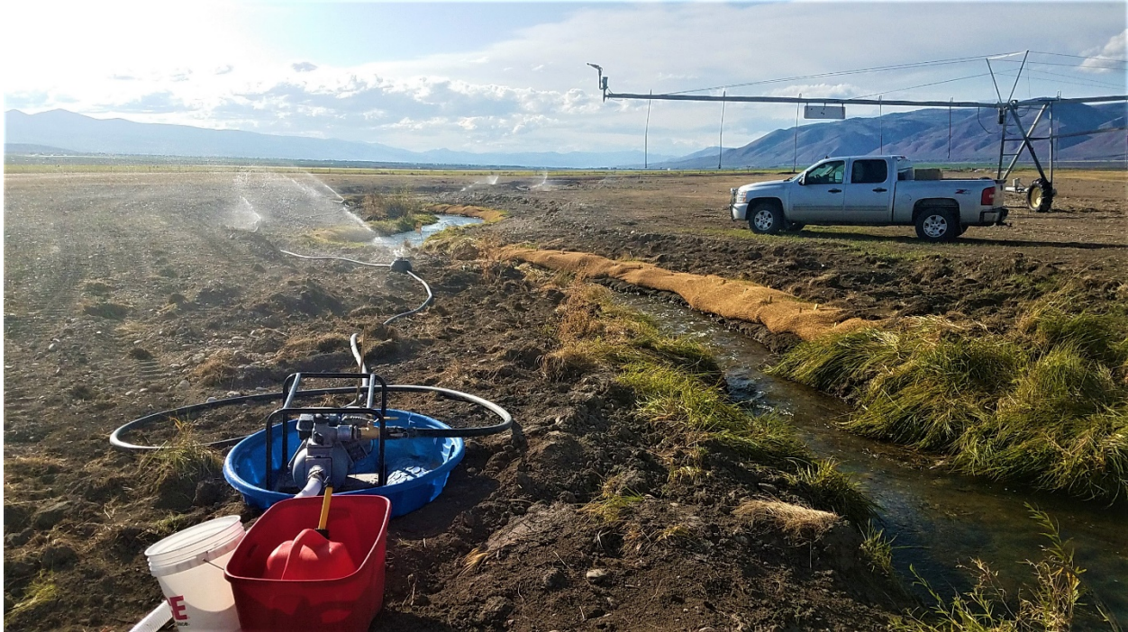
Photograph 3: Sprinkler pods were used to irrigate the riparian zone of the channel alignment. (Middle Eighteenmile Creek Habitat Improvement Project) (Reclamation/Brian Hamilton)
