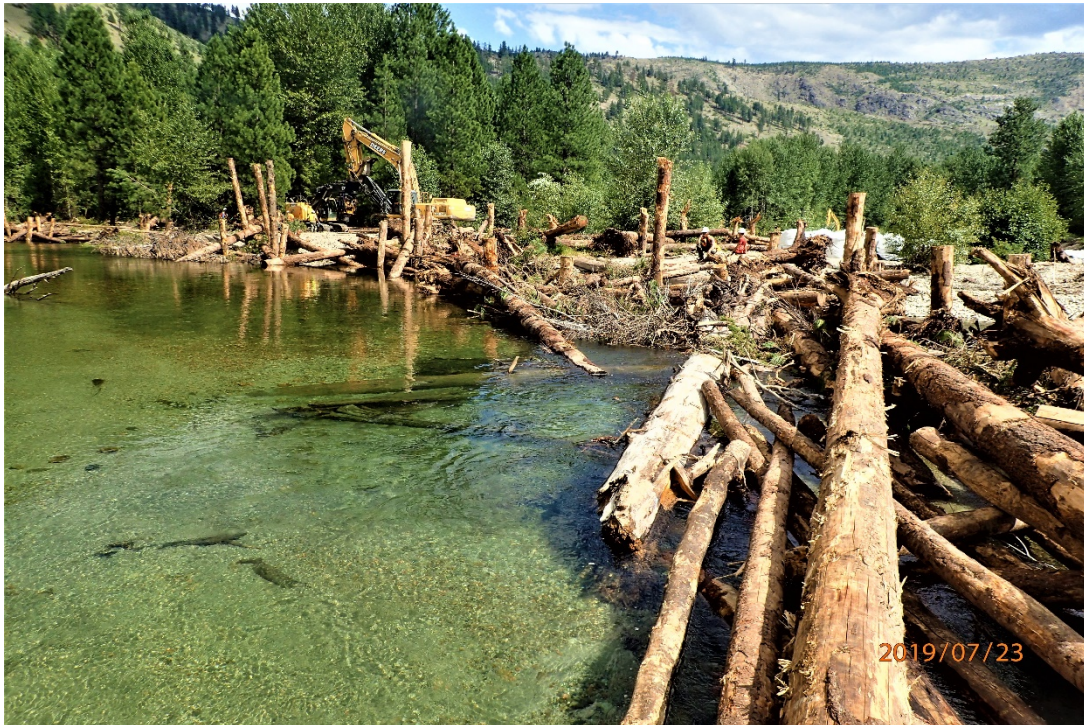
Photograph 26: Large wood is stabilized with vertical piles that are driven into the streambed. The large wood disrupts streamflow, which allows natural river processes to resume. (Middle Entiat, Stormy B) (Reclamation/Steve Kolk)
