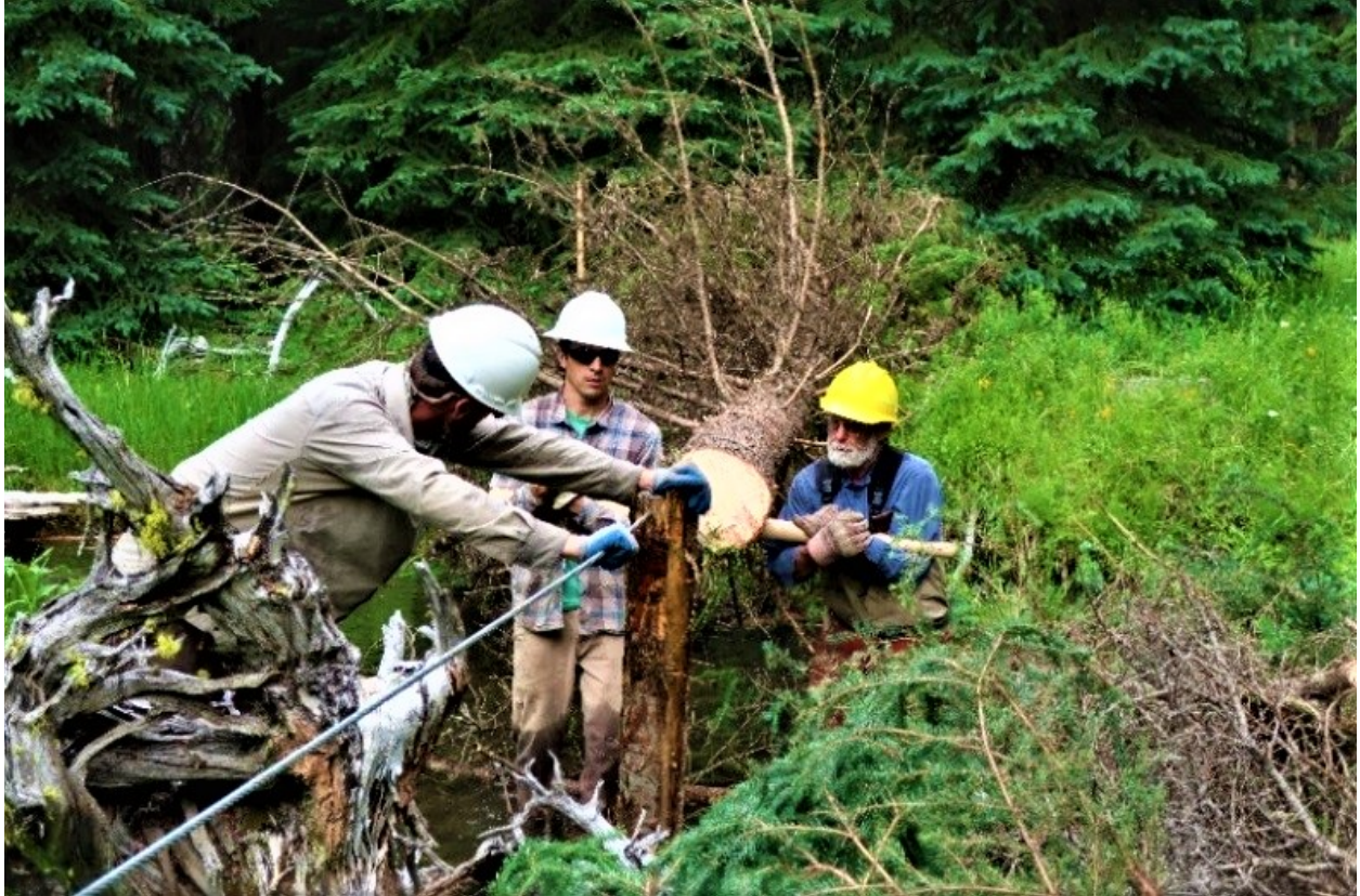
Photograph 21: Hand crew using grip hoist and two-person log carrier to drag large trees into the stream. (Sheep Creek Habitat Enhancement Phase I) (Reclamation/Al Simpson)
