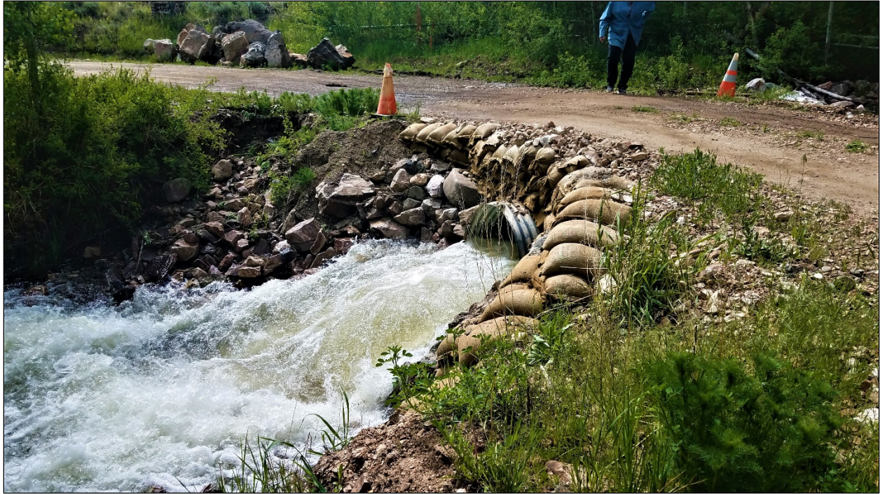
Photograph 5: This pre-project view of the Chipmunk Hill culvert shows the flow barrier to fish movement into the upper Garden Creek drainage. (Garden Creek - Chipmunk Hill Culvert Removal) (Reclamation/Brian Hamilton)
