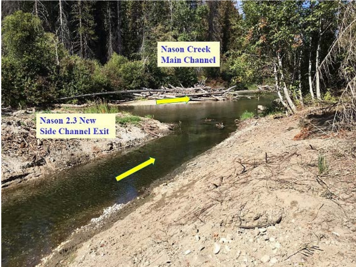
Figure 12: Post-project view shows the side channel flowing back into the main channel of Nason Creek.
