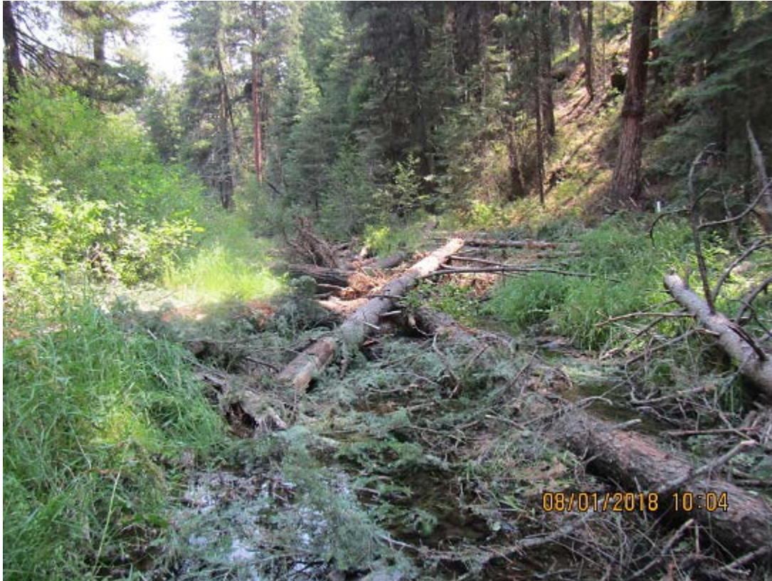
Photograph 18: Post-project view showing the large wood that was added to the stream to create cover and habitat for juvenile steelhead and salmon.
