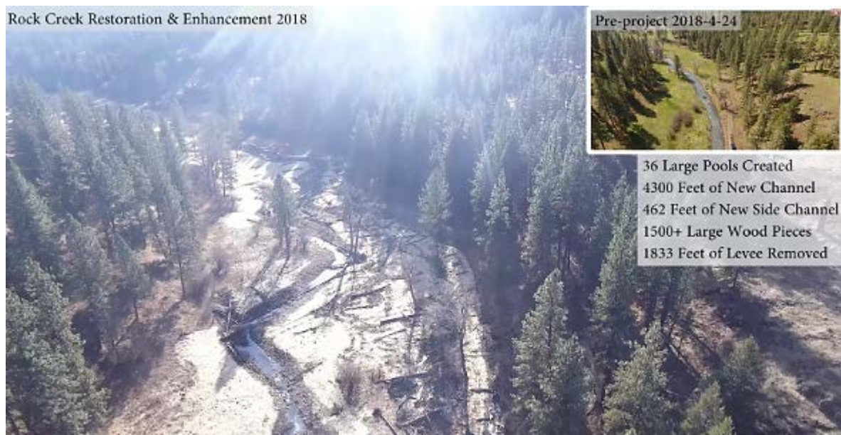
Photograph 9: Post-project view shows the complex channel and side channel with the addition of pools, riffles, and wood.
