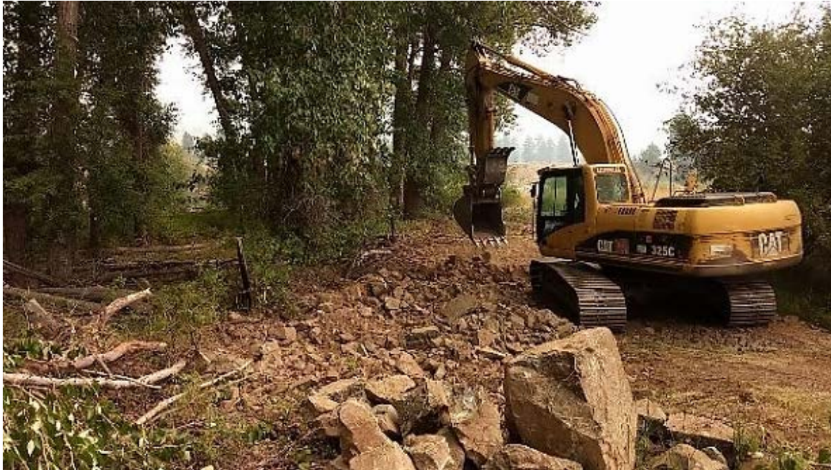
Photograph 26. View of the construction process to remove the cross levee.
