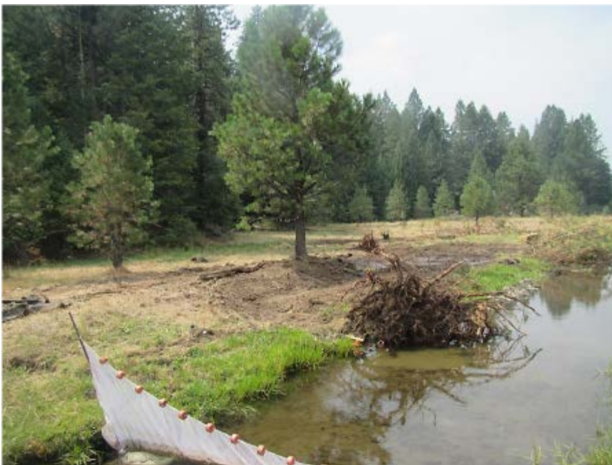
Photograph 15: Post-project view of the inlet to Side Channel No. 2.
