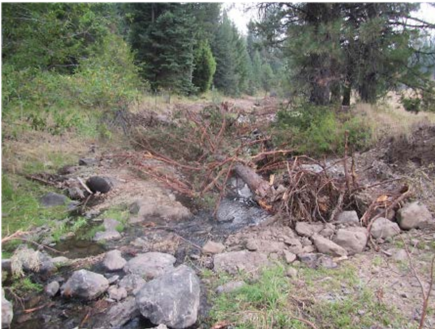
Photograph 11: Post-project view of the complexity added to the same channel.
