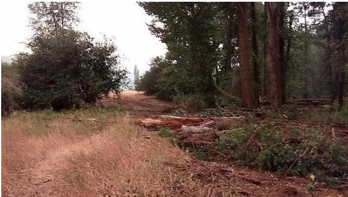
Photograph 27. Post-project view looking east along the new floodplain where the cross levee was removed.
