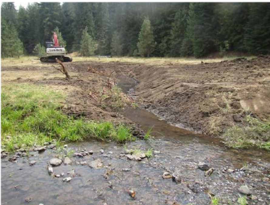
Photograph 17: Post-project view of the outlet location of Side Channel No. 3.
