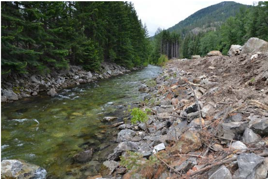
Photograph 33: Pre-project photograph shows the typical condition of the river prior to construction.
