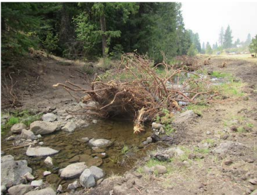
Photograph 13: Post-project view of the completed channel in the Pool No. 9 section.
