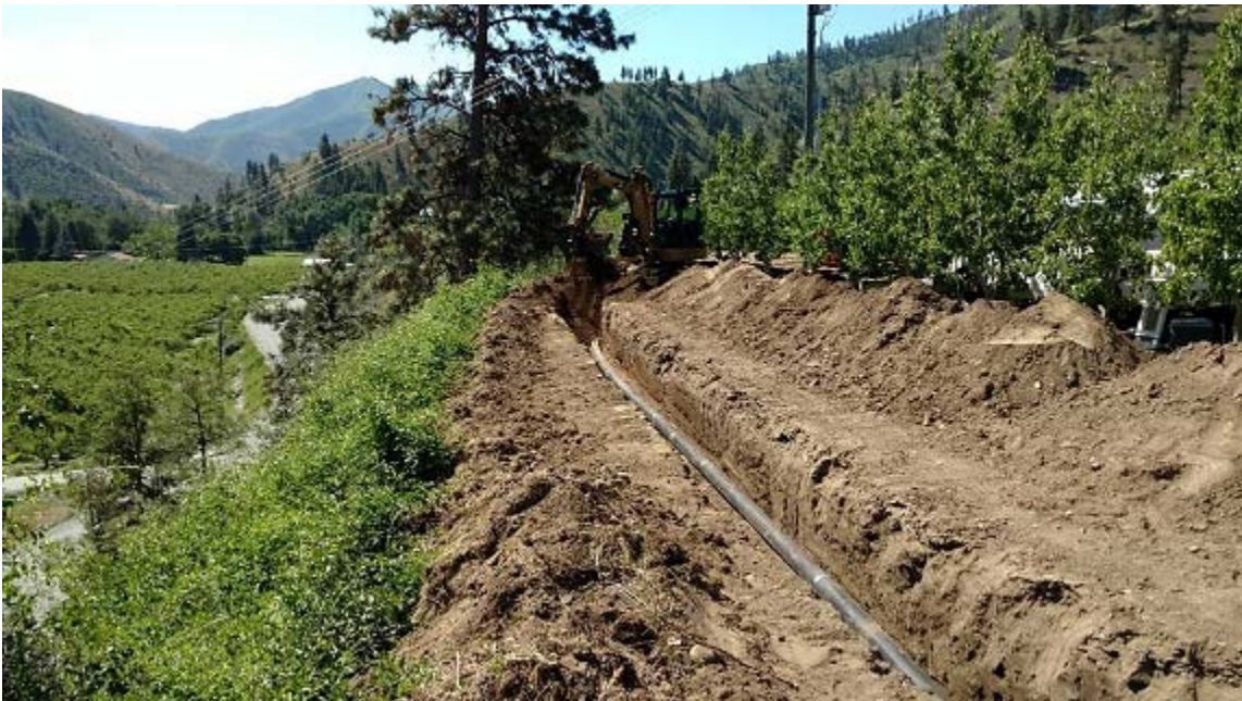
Photograph 29: Construction photograph shows the new efficient water delivery system being installed.
