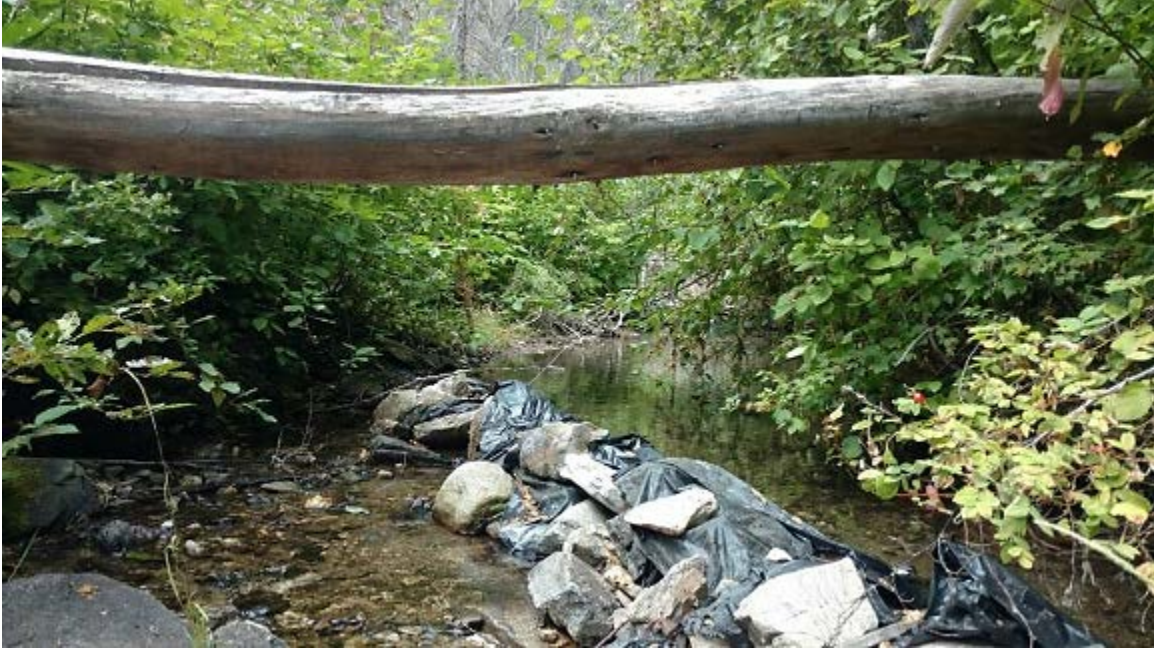
Photograph 28: Pre-project photograph of Roaring Creek Diversion looking upstream. The diversion completely blocks the channel.
