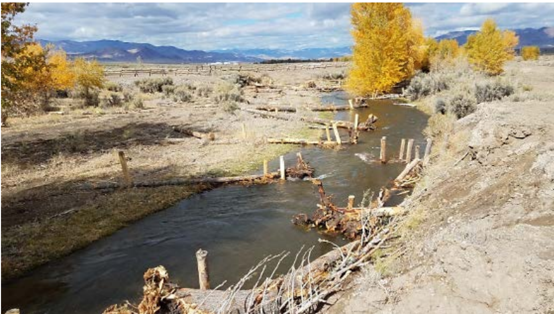
Photograph 4: Post-project view displays a sample of the 430 large rootwad trees and more than 6,000 potted plants and willow stakes in 1.10 miles of the stream channel and riparian zone.
