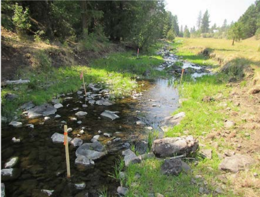
Photograph 12: Pre-project view showing bank layback and new Pool No. 9 location.
