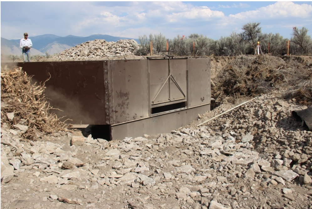
Photograph 34: A new steel head gate structure was installed. Diverted flows will be much less than before due to the improvements in the irrigation system downstream.
