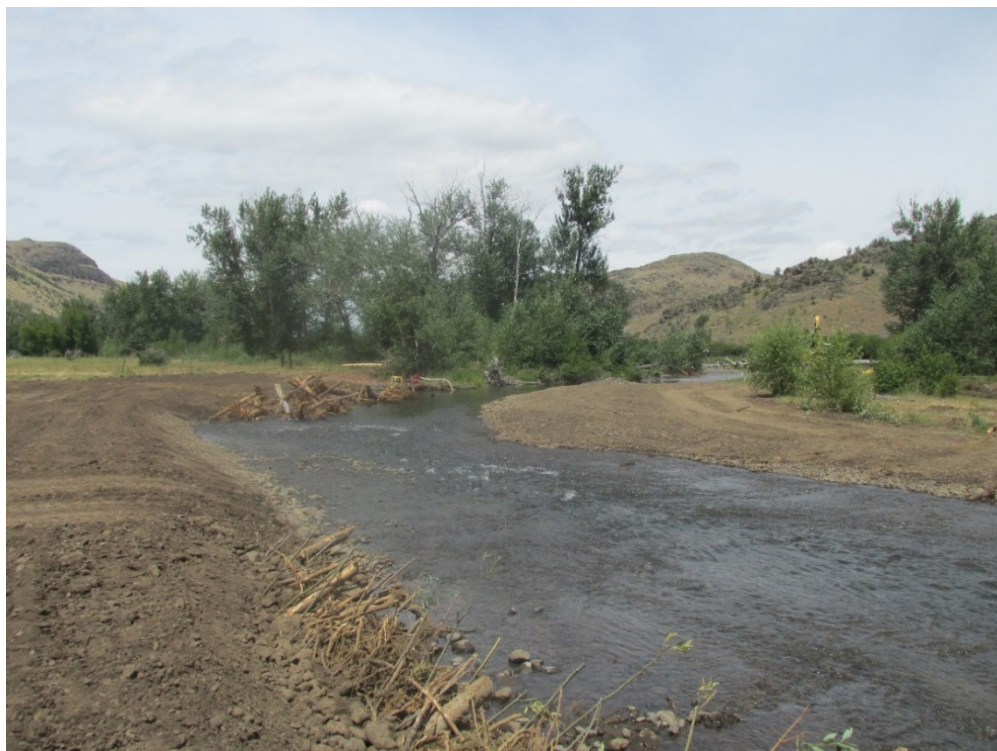
Photograph 45: Showing large wood debris (LWD), bank zone planting and floodplain grading after channel activation.
