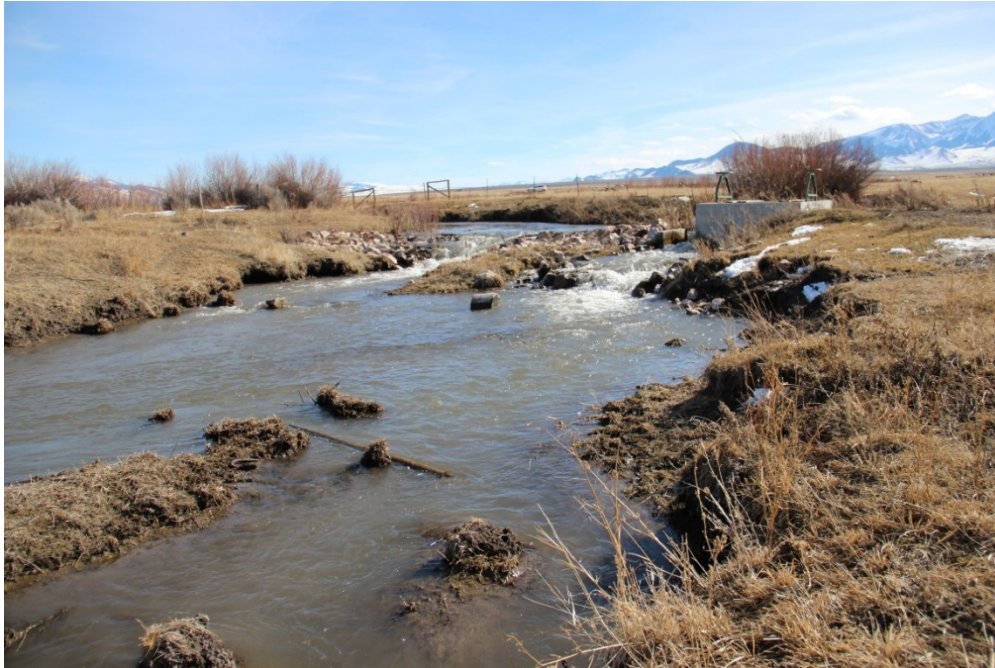
Photograph 29: The P-13 diversion structure and head gate was removed. Sulphur Creek was narrowed up and lengthened in this area to accommodate the drop over the old diversion structure.
