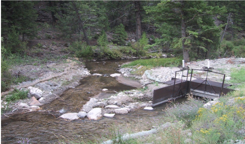
Photograph 16: New LHaC-03 point of diversion and head gate.
