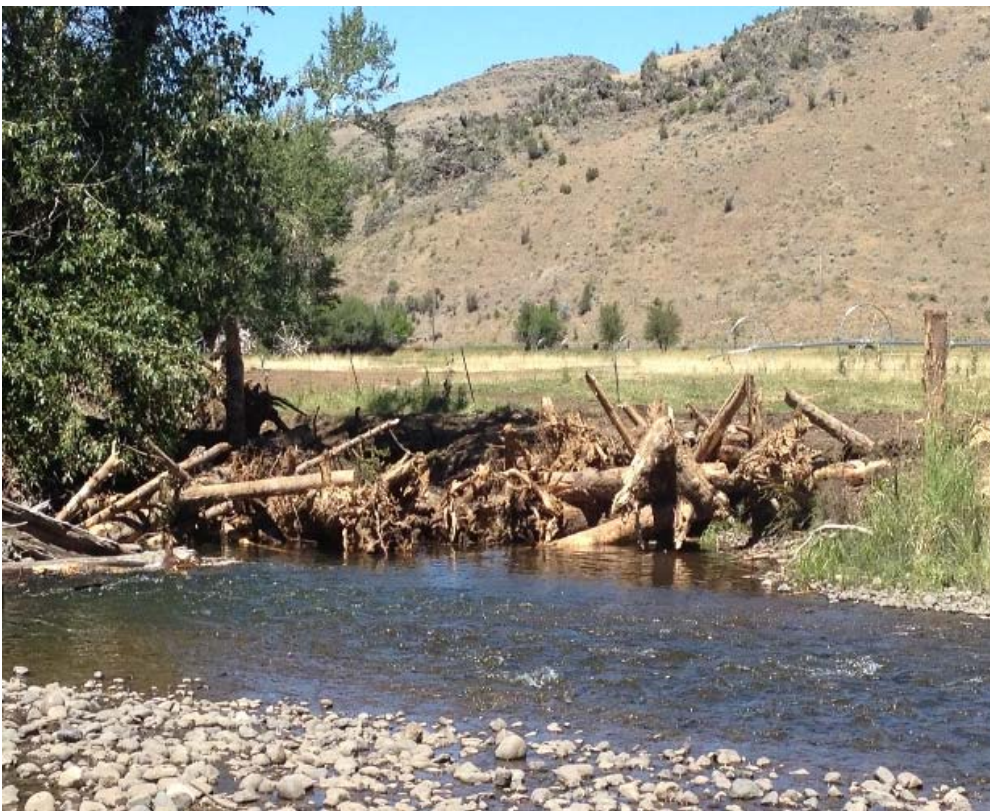
Photograph 47: Constructed LWD structure at the inlet to side channel 3 (same location as Photograph 3).
