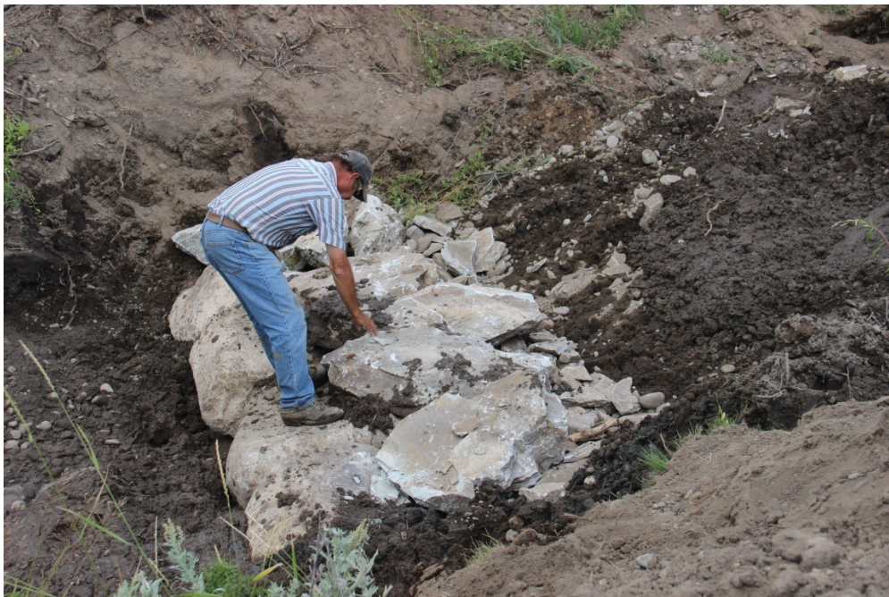
Photograph 32: Large rock was used to make the low head rock weir that will allow water to be diverted into the new ditch without blocking fish movement in the river.
