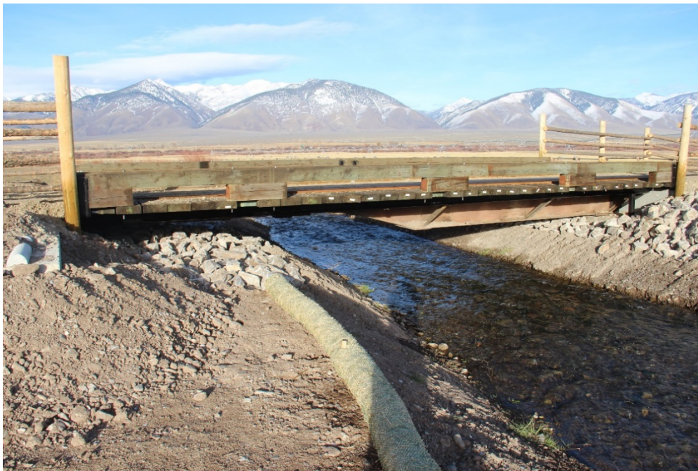
Photograph 37: Looking downstream at the new railcar bridge.
