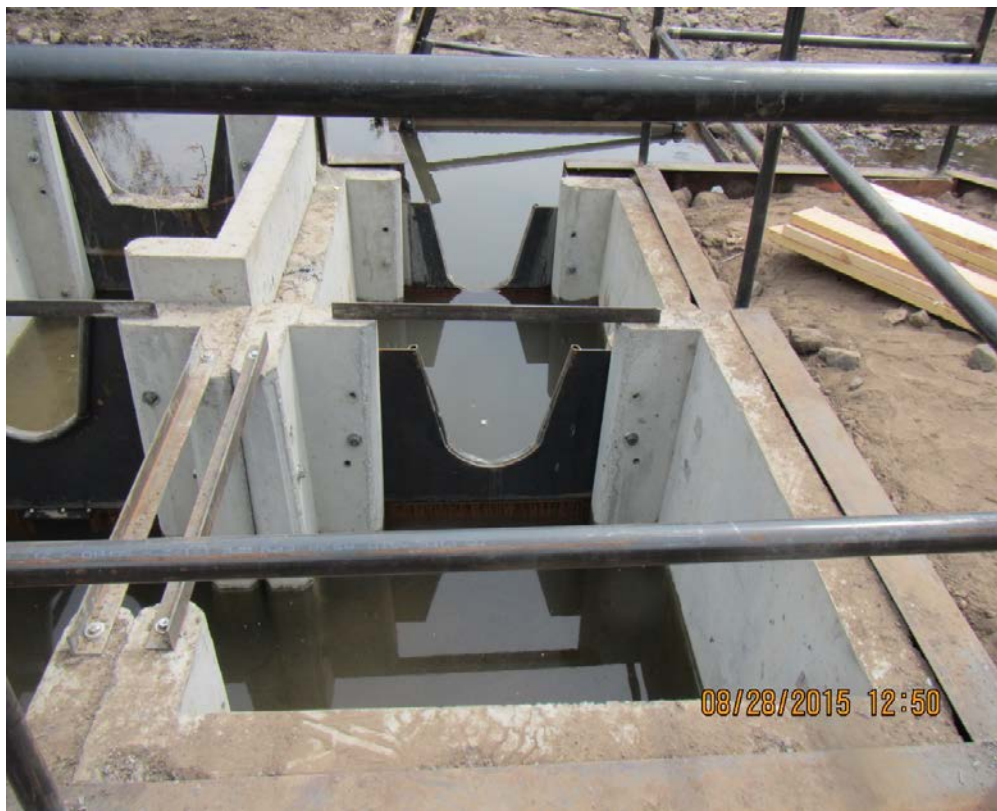
Photograph 62: Pool and weir fish.
