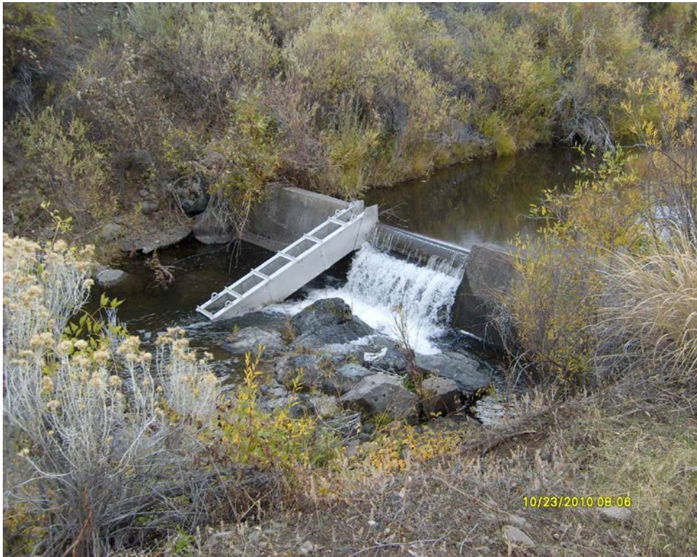
Photograph 65: Concrete diversion with flash board in.
