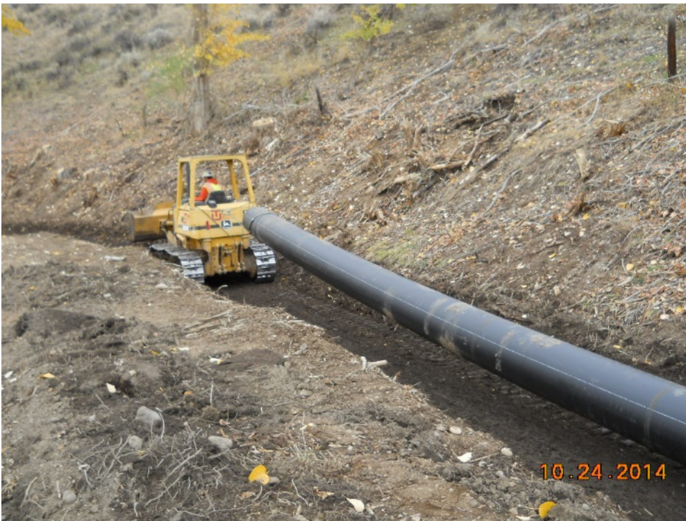
Photograph 76: Laying pipe.
