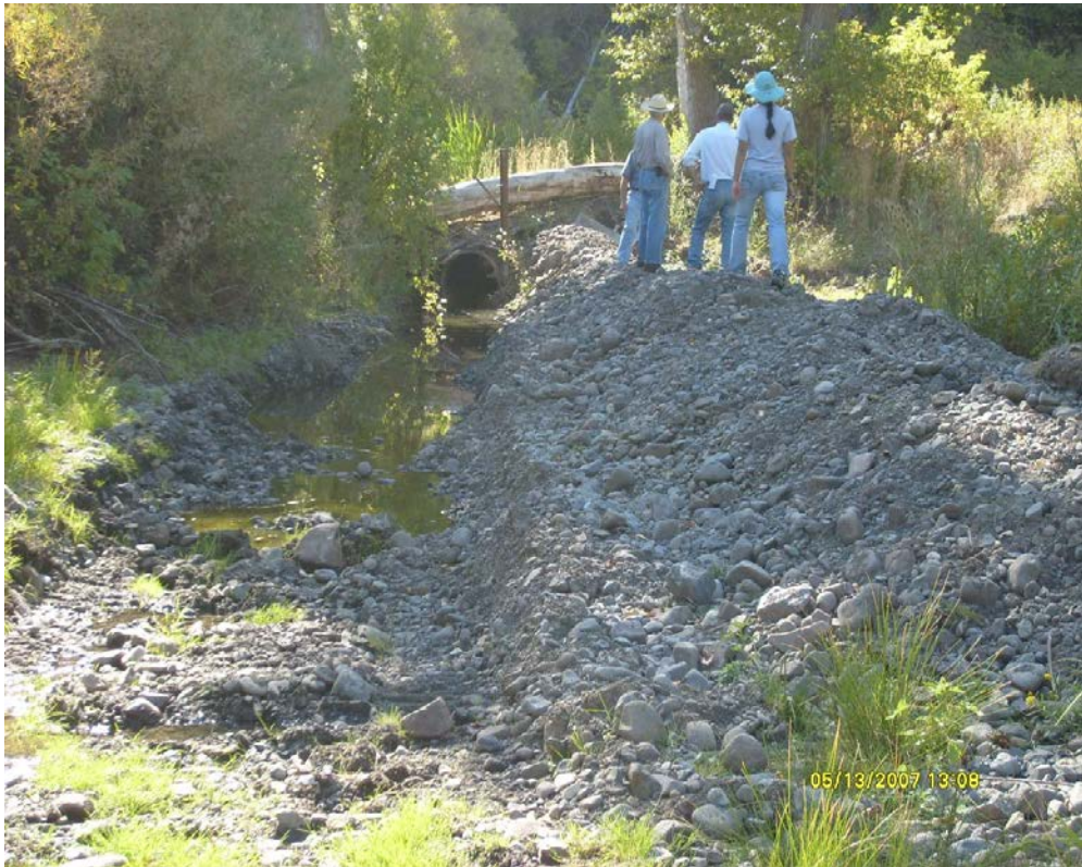
Photograph 59: Gravel wing dam leading to Diversion #1.
