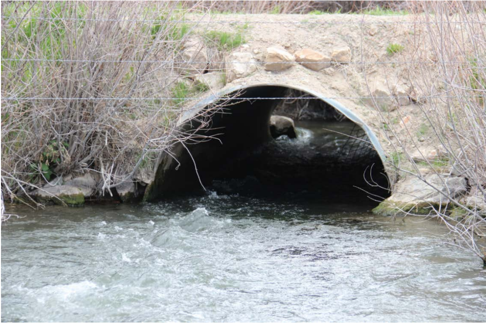
Photograph 25: Photo taken looking upstream at the undersized culvert that was removed and replaced with a steel beam bridge.
