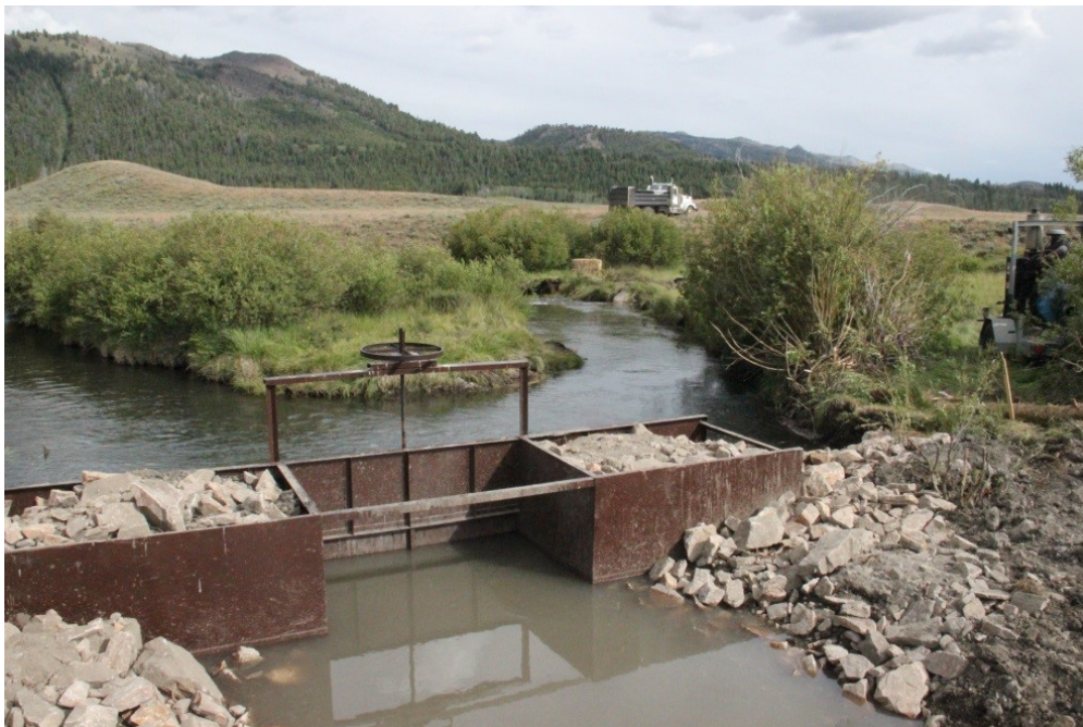
Photograph 39: The new head gate installed. Pole Creek is on the far side of the head gate, the new irrigation ditch is on the near side.
