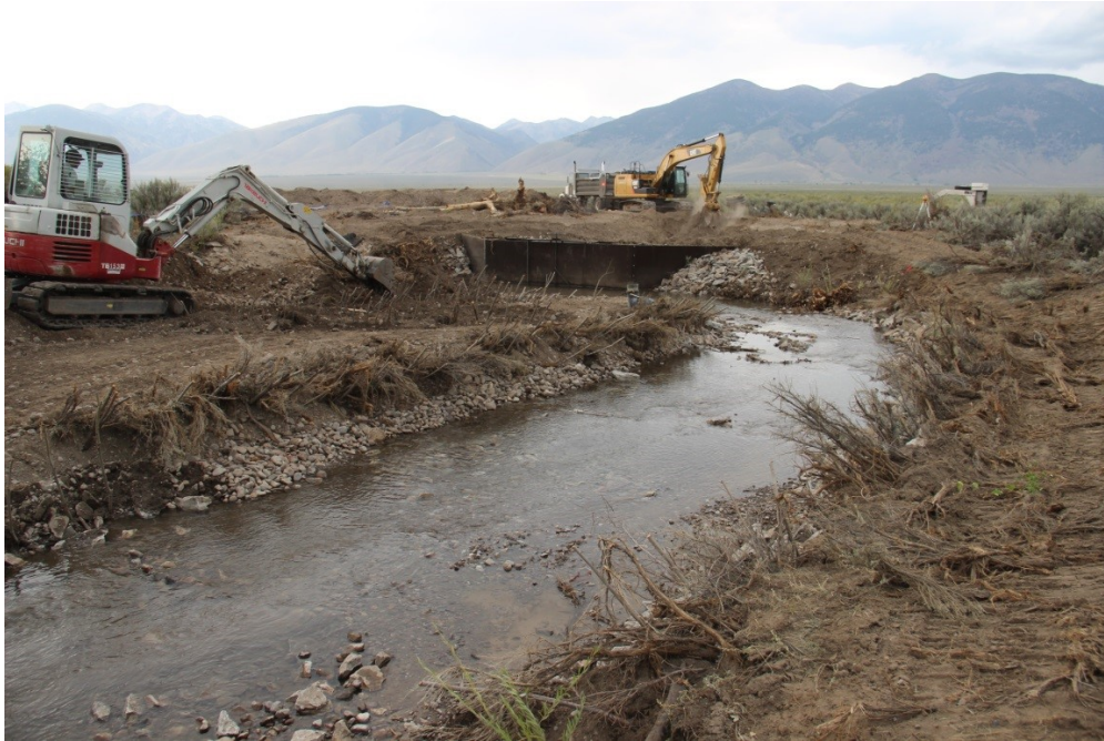
Photograph 35: The Pahsimeroi River was moved slightly upstream of the new head gate structure. Willows were planted along both banks and dead brush installed to roughen the banks until the willows begin growing.
