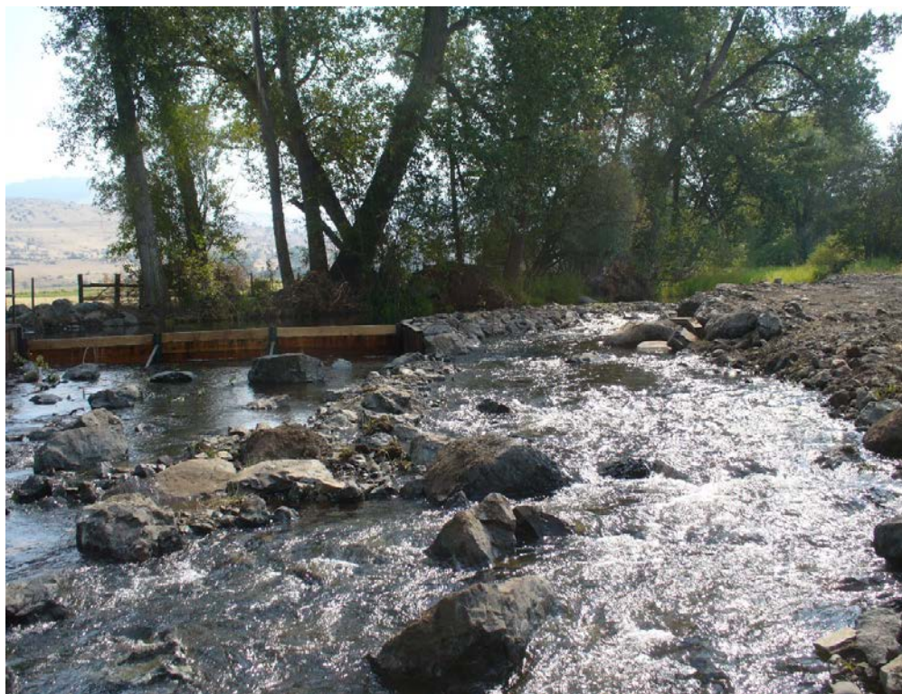
Photograph 56: Main channel stanchion dam and alluvial passage on far right, looking upstream.
