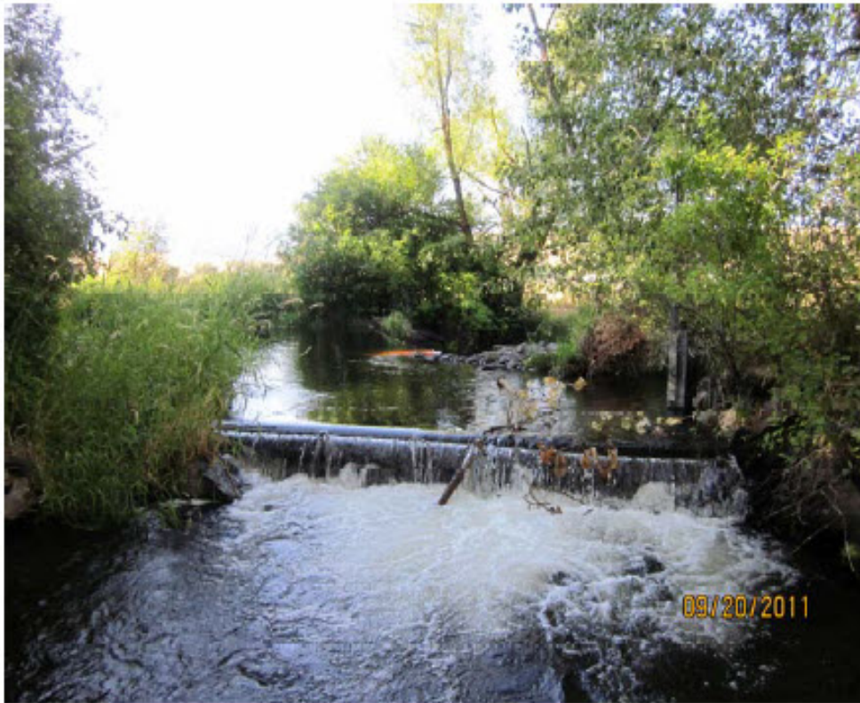
Photograph 57: Log sill on side channel.
