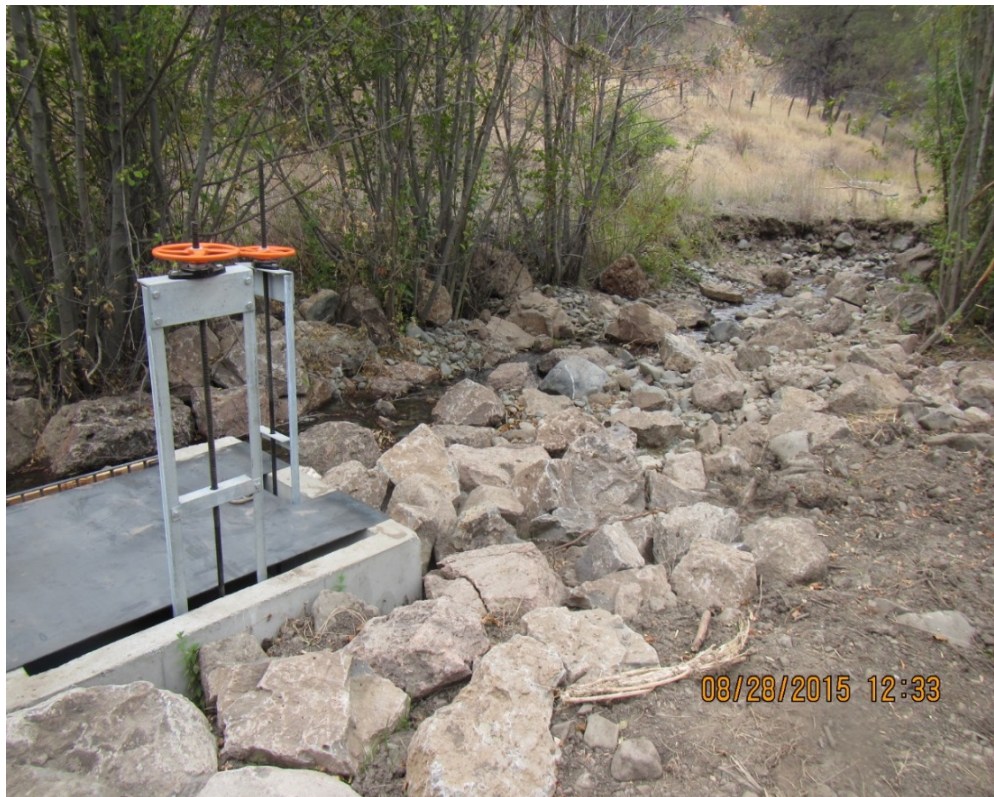
Photograph 73: New diversion and constructed riffle looking downstream.
