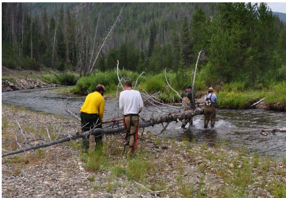
Photograph 41: Large wood being placed by U.S. Forest Service staff.
