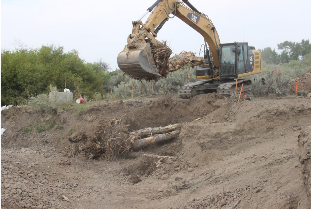
Photograph 33: Rootwad trees were installed upstream and downstream of the new head gate structure to provide fish habitat.
