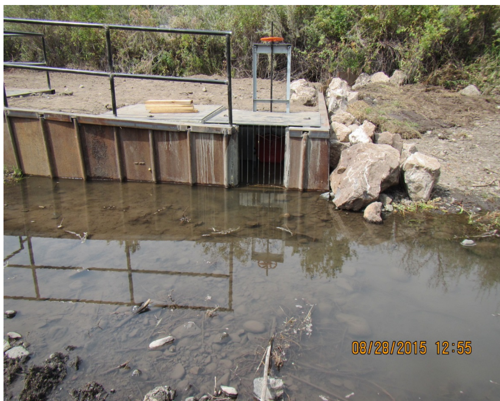
Photograph 63: Irrigation headgate.
