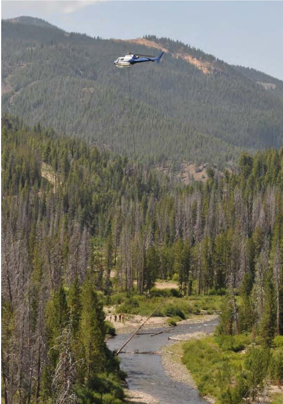
Photograph 42: Large wood was added to the channel using a helicopter.
