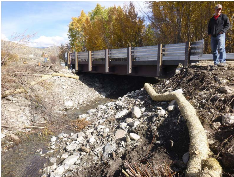
Photograph 13: Completed bridge installation and stream re-watered.
