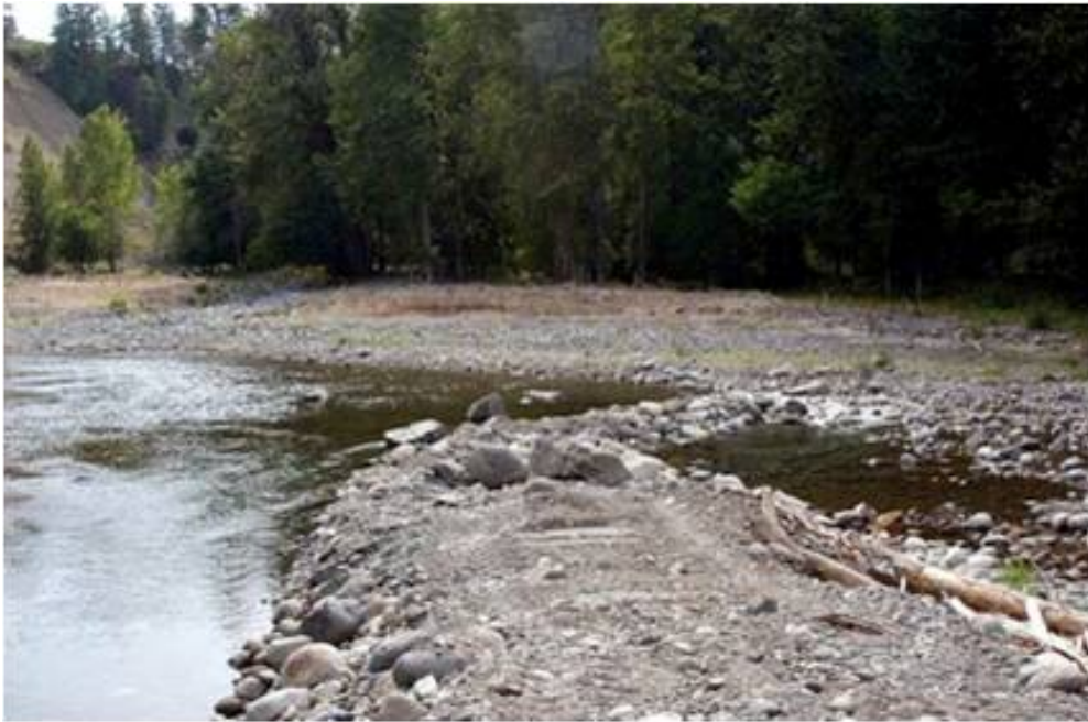
Photograph 75: MVID push-up dam on the Twisp River, blocking mainstem and diverting most of the flow into the headgate.
