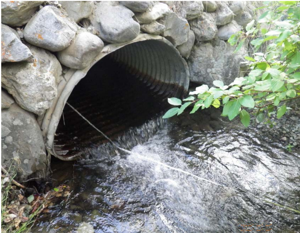
Photograph 12: Perched outlet of Pratt Creek Culvert.
