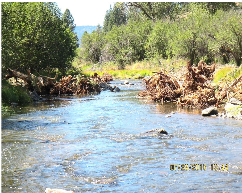
Photograph 52: Log jams placed on alternating sides of the river.
