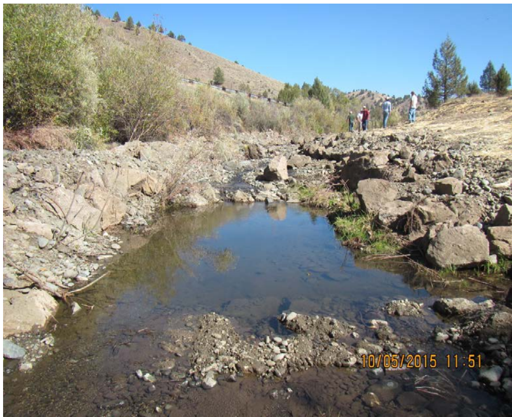
Photograph 68: Pool at bottom of riffle to dissipate energy.
