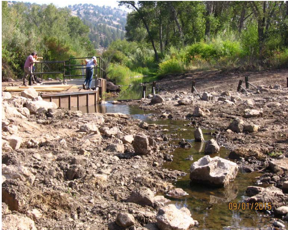
Photograph 61: Completed diversion with low flow channel below structure.
