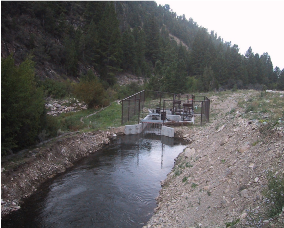
Photograph 17: Completed LHaC-03 fish screen.
