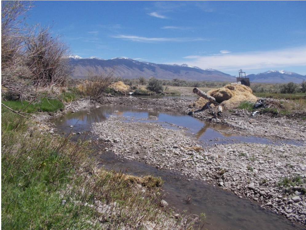
Photograph 31: The old diversion was a gravel push-up dam that dried up the Pahsimeroi River in the summer.
