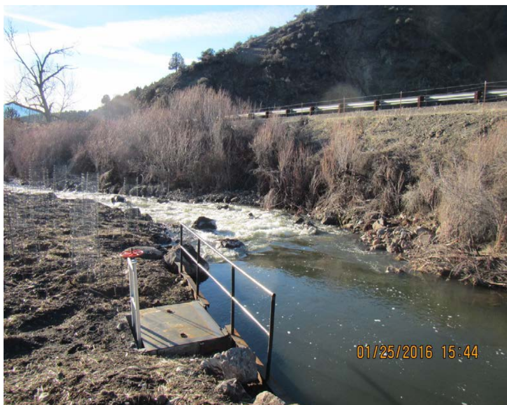
Photograph 69: New riffle with head gate structure, winter.
