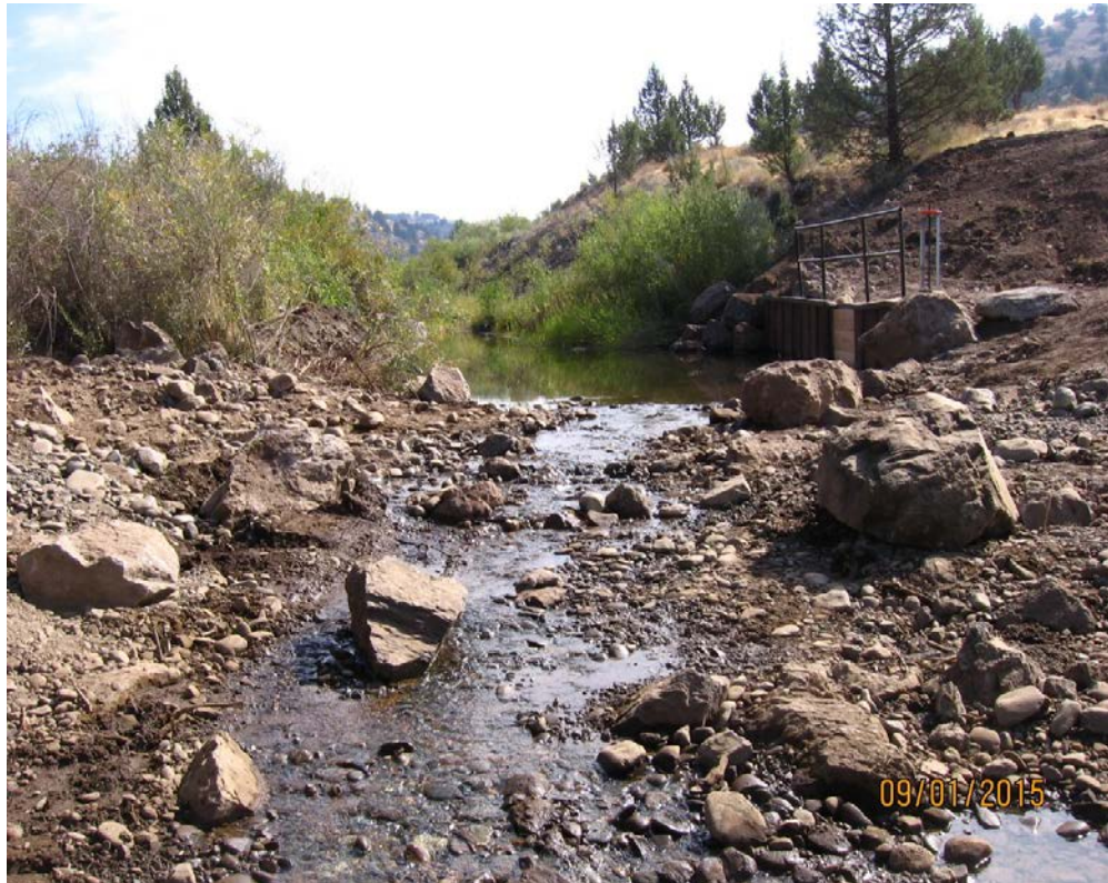
Photograph 67: Top section of completed riffle and head gate structure at low summer flows and diversion shut.
