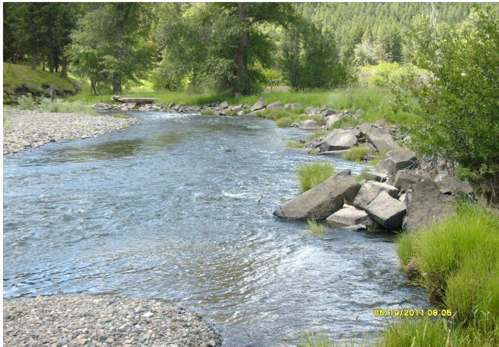
Photograph 51: Rock barbs and rip rap to be removed.
