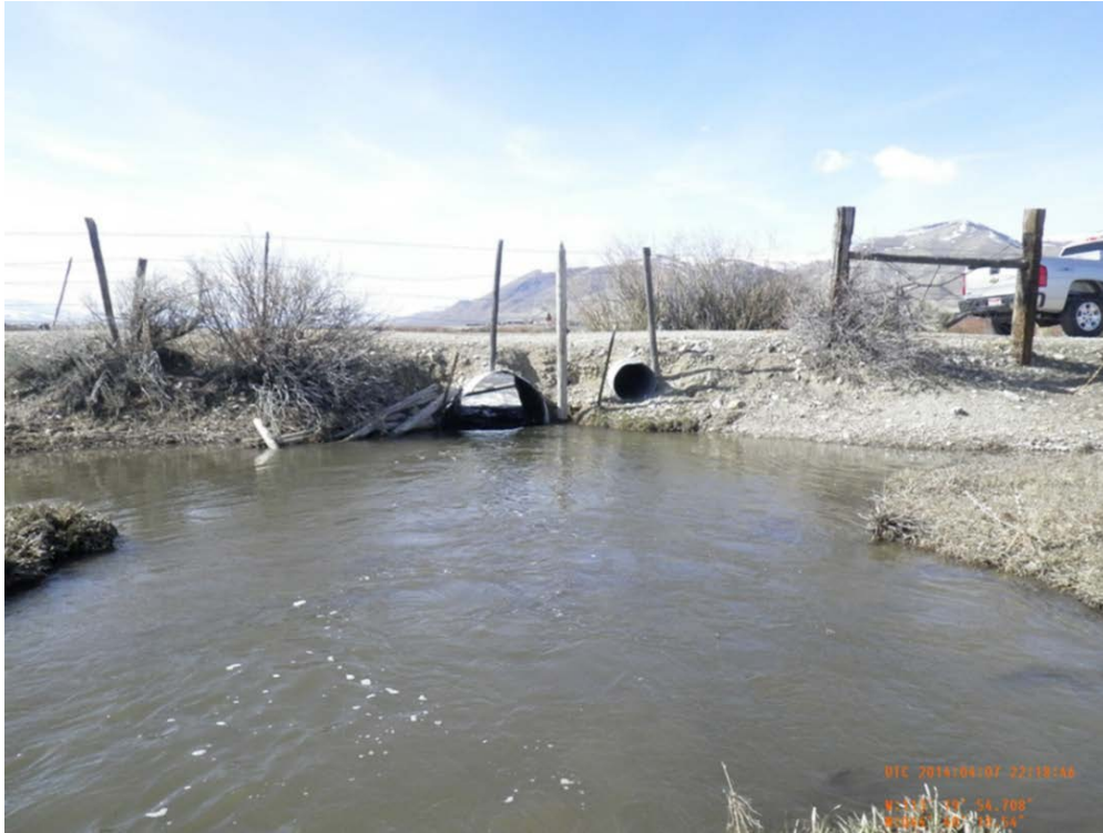
Photograph 5: Eighteenmile Creek Culverts before replacement.
