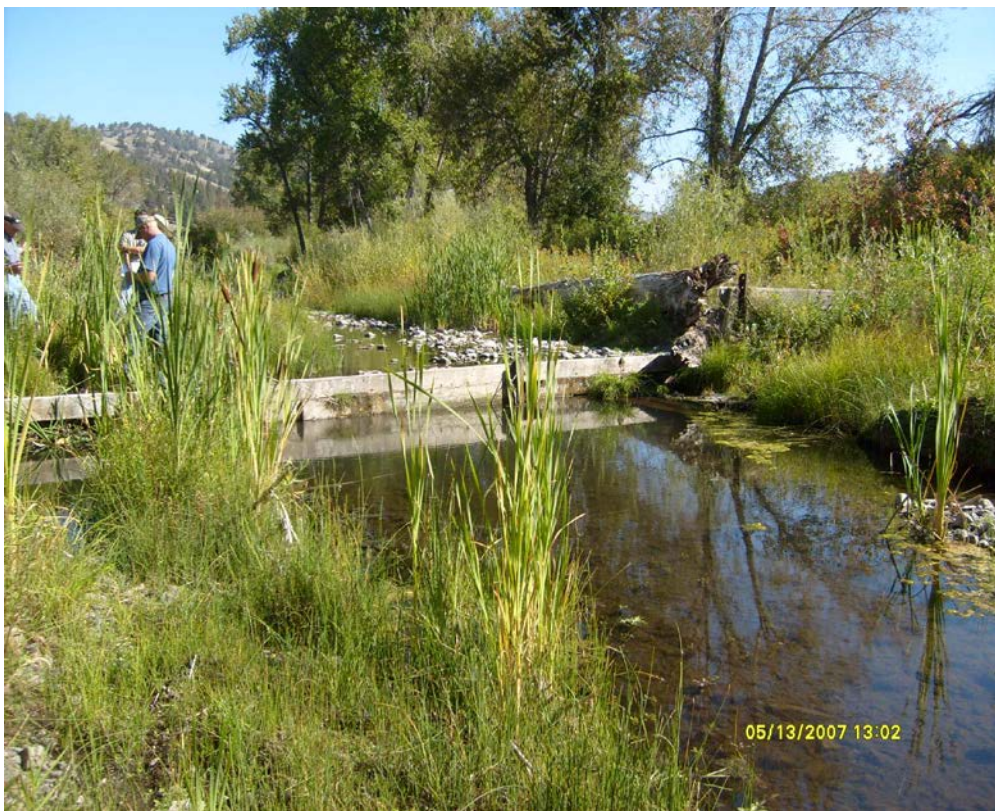
Photograph 60: Steel post and timber semi-permanent grade control check for Diversion #2.
