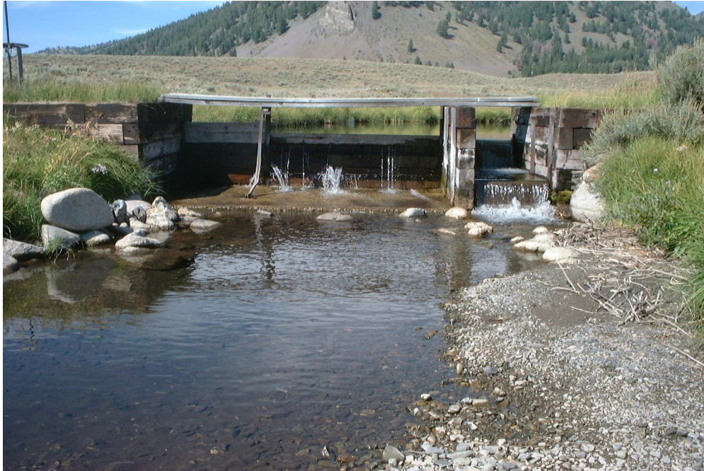
Photograph 38: The old diversion structure was a barrier to fish passage. IDWR Agreements kept a minimum of 5 cfs. in the stream channel below the diversion.
