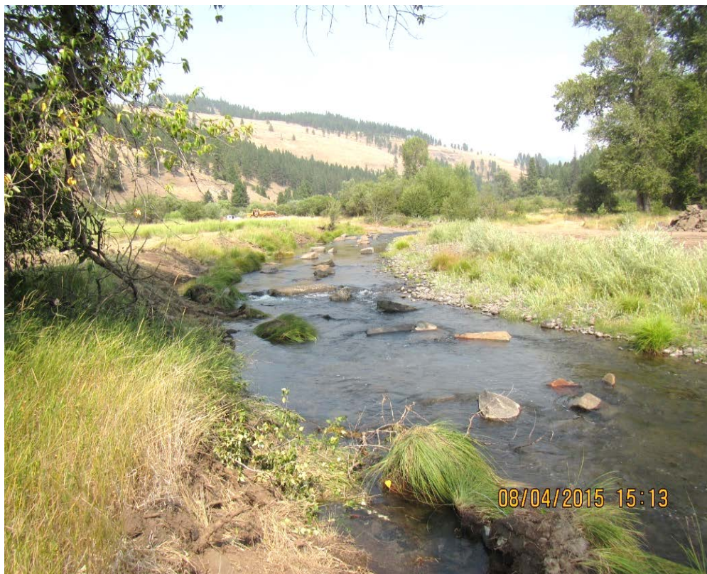
Photograph 54: Large boulders placed instream and rip rap removed from river.
