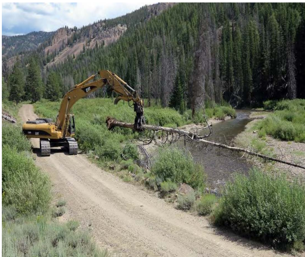
Photograph 43: Placement of large wood in the main channel of the Yankee Fork.
