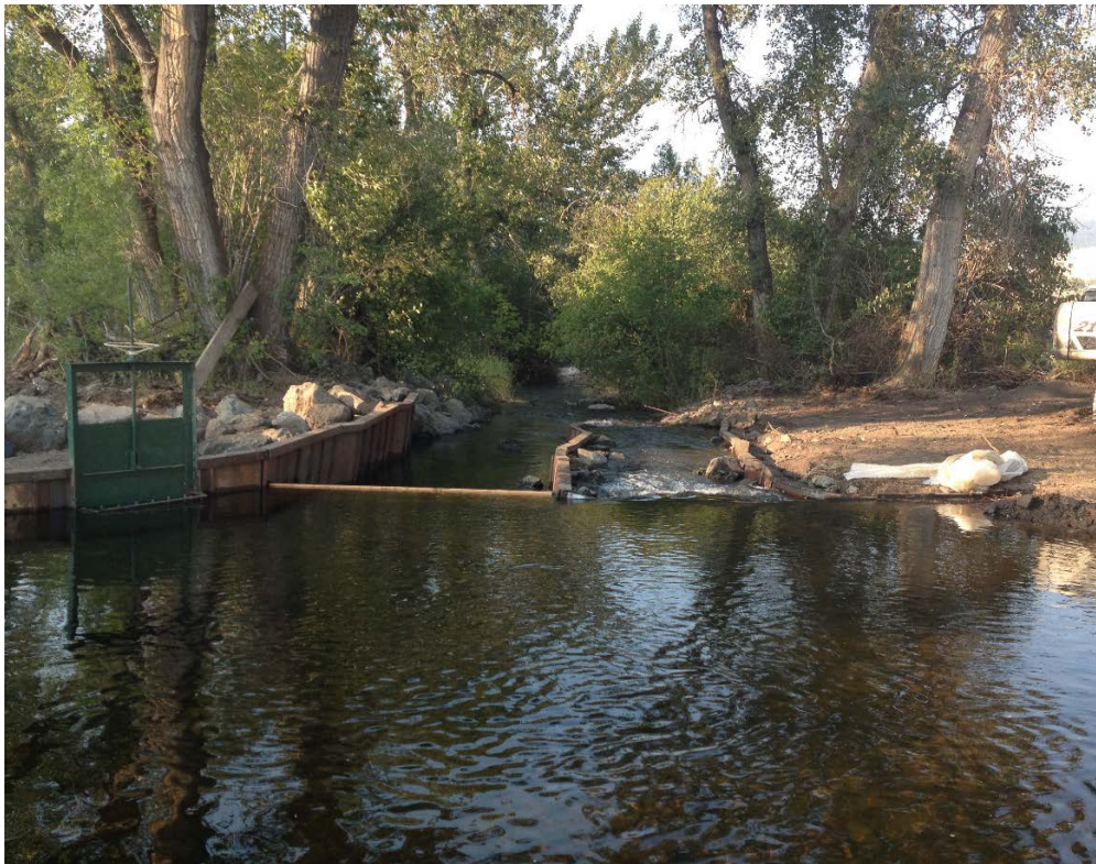
Photograph 58: Side channel stanchion and alluvial passage, looking downstream.
