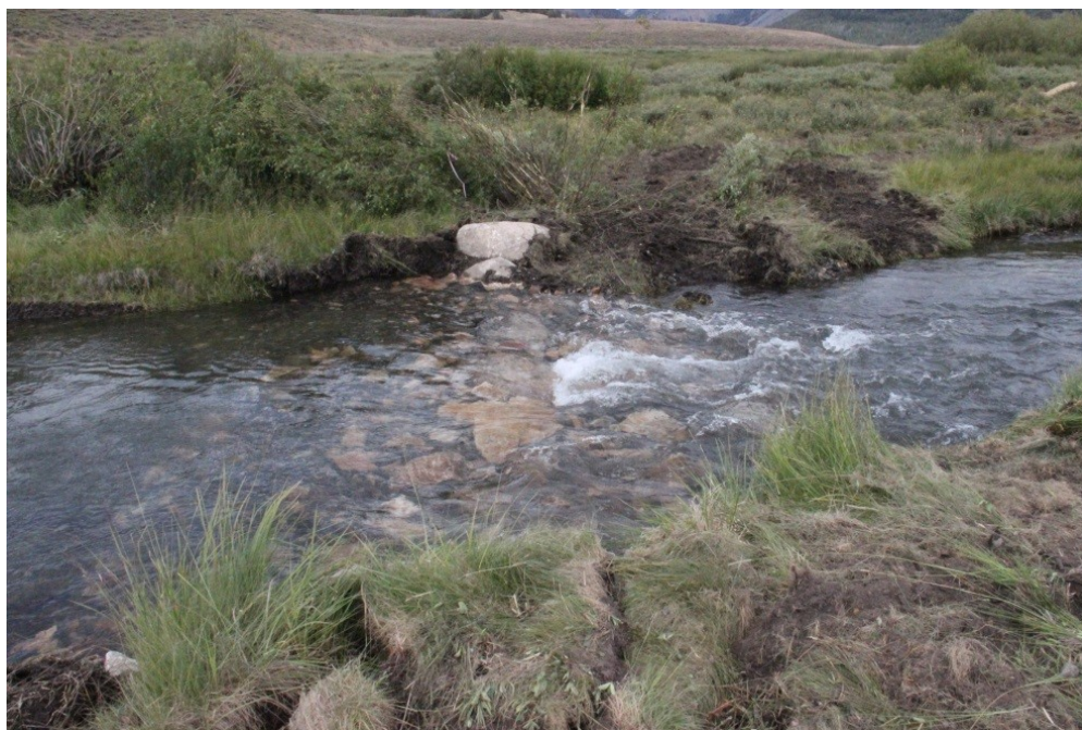
Photograph 40: The new diversion structure is a low head rock weir that spans the channel and provides a water surface elevation high enough to fill the new ditch without inhibiting fish movement.
