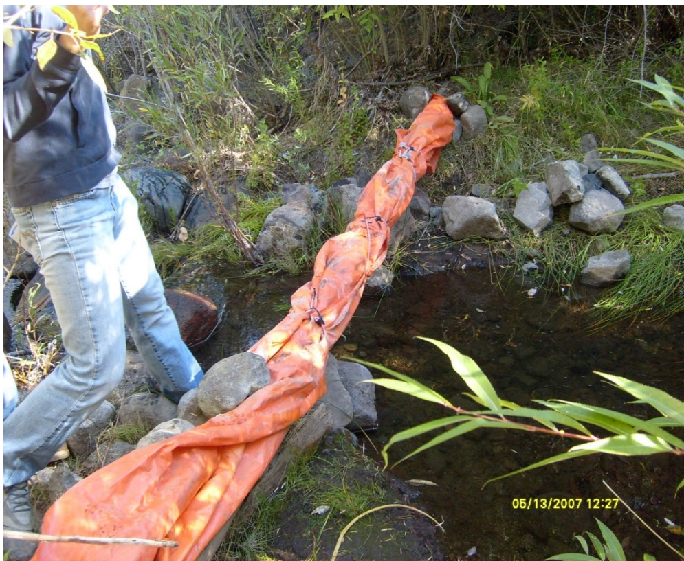
Photograph 72: Tarp used to block the stream and direct it into the ditch.
