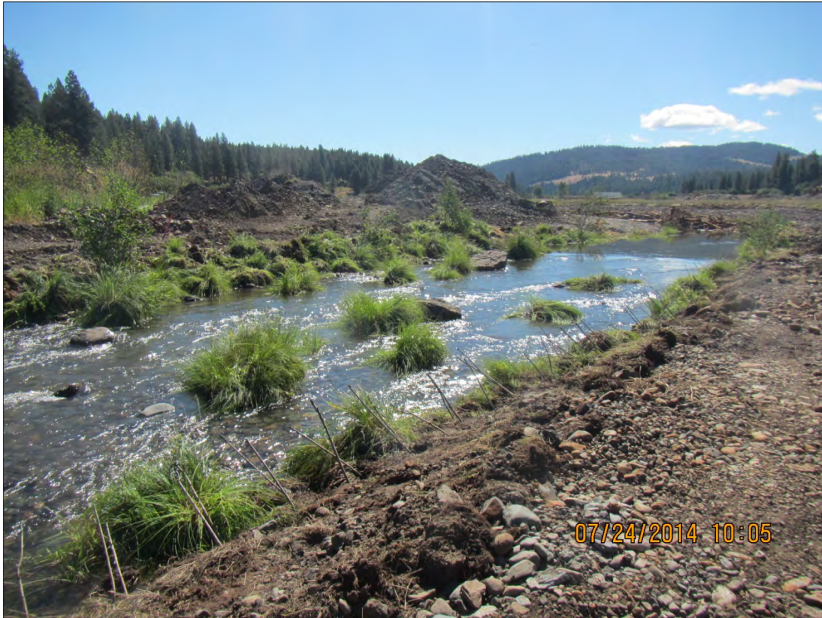
Photograph 45. Completed riffle in the new channel, showing willow cuttings and torrent sedge transplants
