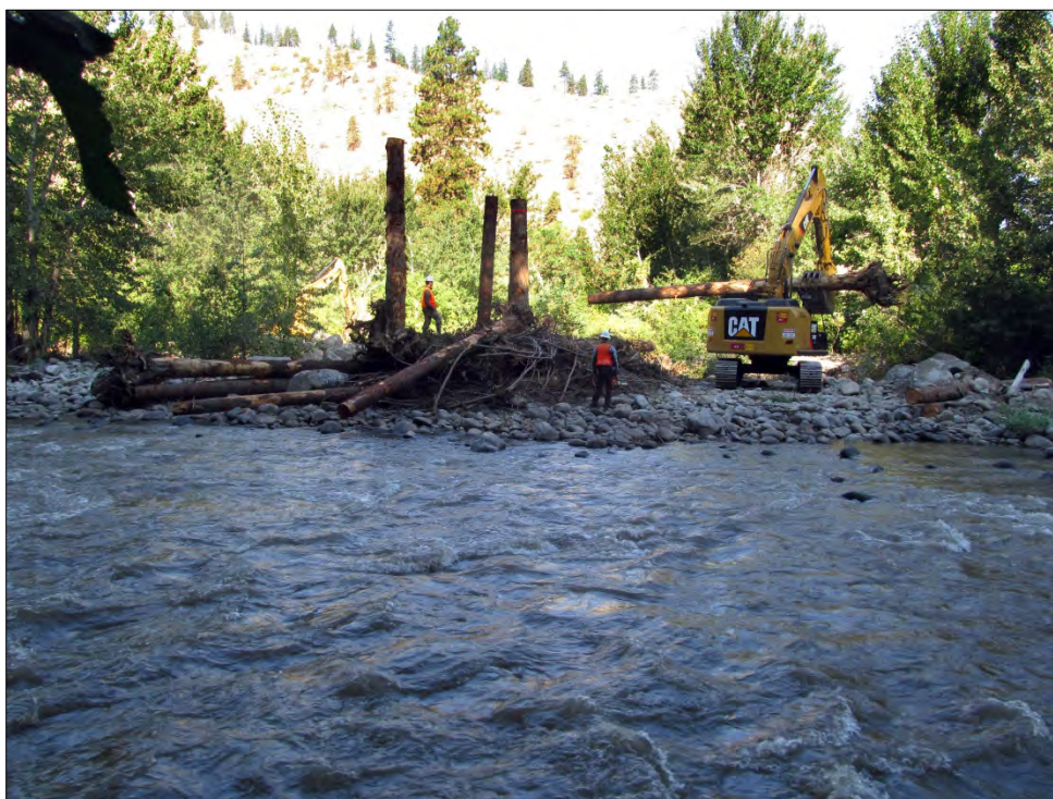
Photograph 50. ELJ during construction at the head of the island, with a boulder cluster to the right of the backhoe at RM 6.8
