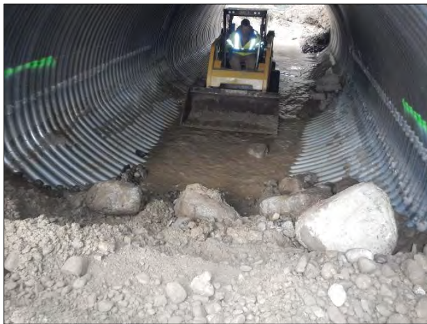
Photographs 83 and 84. The large culvert was placed low enough to allow the contractor to install engineered streambed material to create a more natural passage channel through the large culvert.
