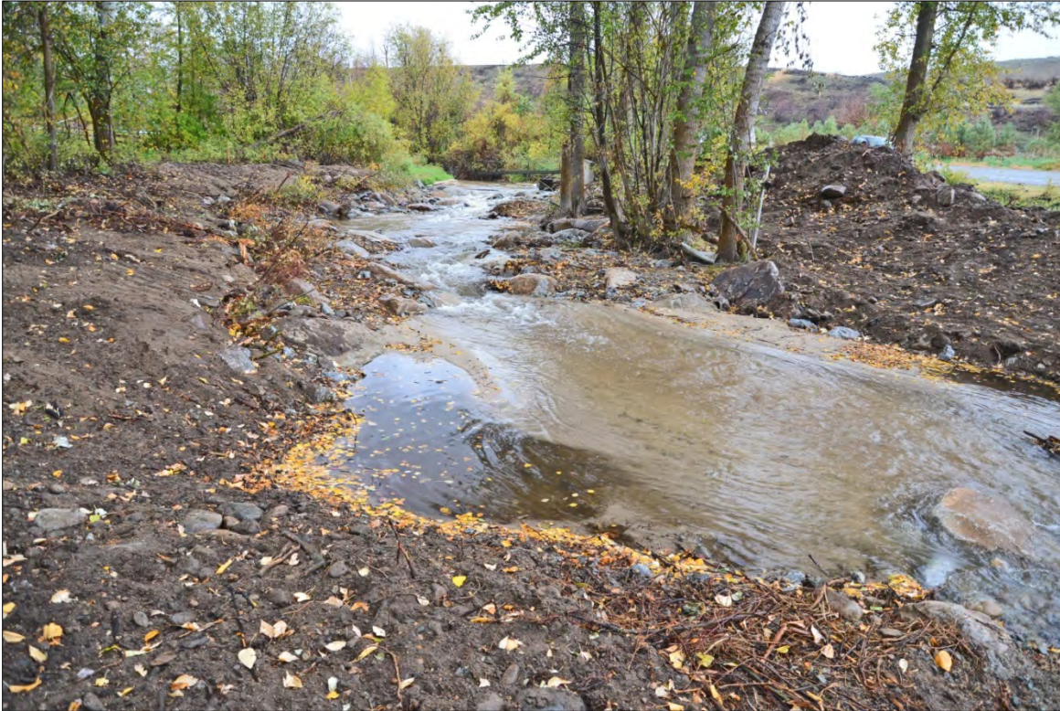
Photograph 71. The Fort Thurlow diversion as the Beaver Creek flows were introduced to the chute-pool roughened channel after construction was completed. The design looks natural and provides fish passage for all life stages.
