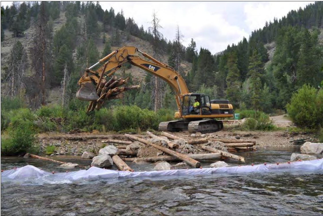
Photograph 28. Habitat was enhanced with construction of a simulated debris flow in the treated reach.
