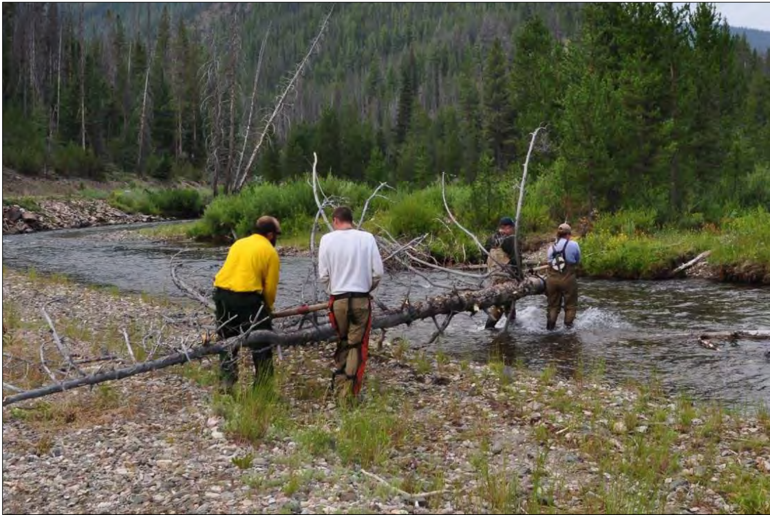
Photograph 26. Placement of trees by hand in the treated reach of the Yankee Fork
