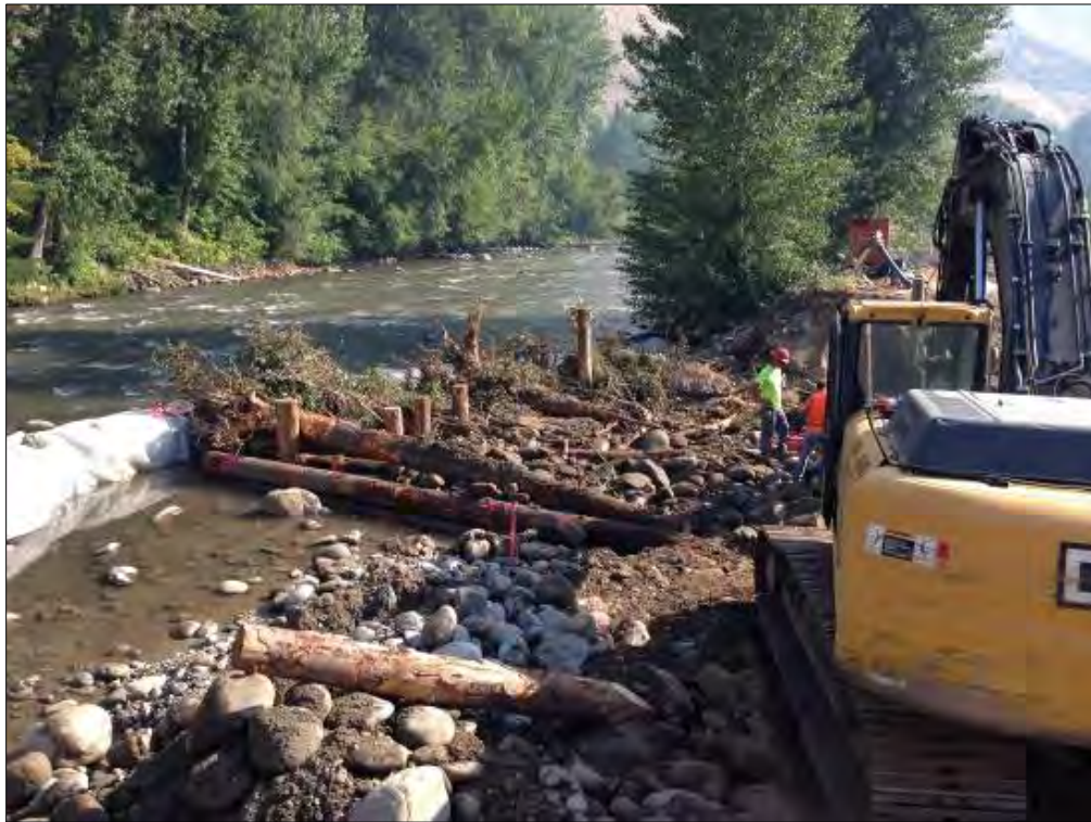
Photograph 58. A view from upstream of one of five right-bank ELJs under construction in the main Entiat channel
