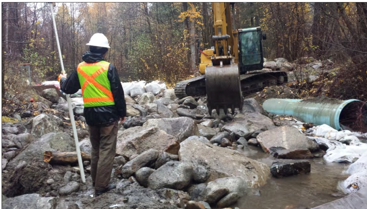
Photograph 66. The Marrachi diversion during construction of the roughened channel
