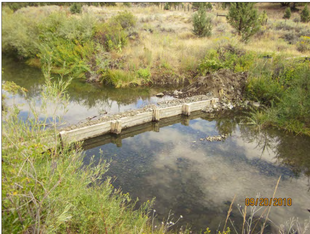
Photograph 46. Pre-project Meredith Beech Creek Diversion #5 shown with a passage barrier
