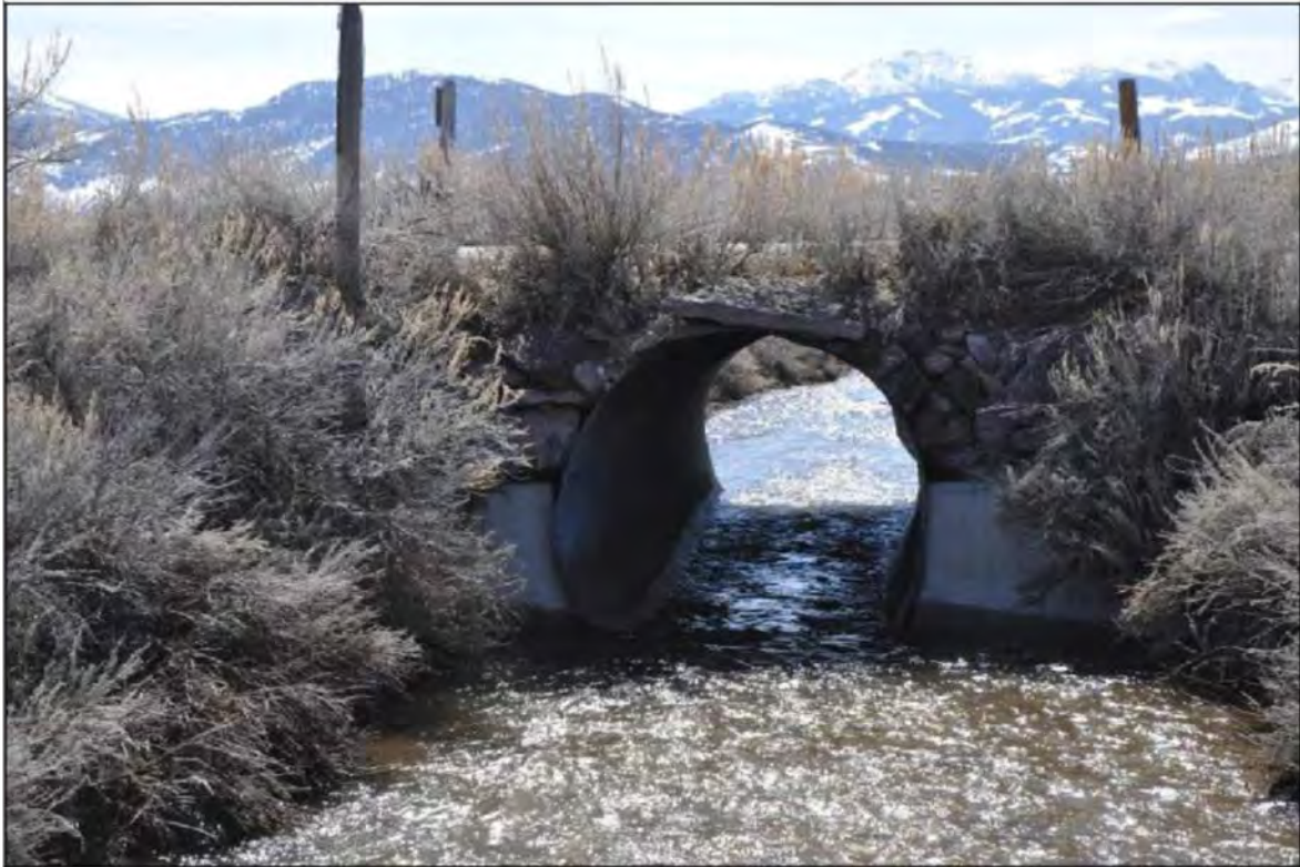
Photograph 1. This culvert under the county road on Hawley Creek restricted fish passage during various flow conditions and was removed as part of the project.
