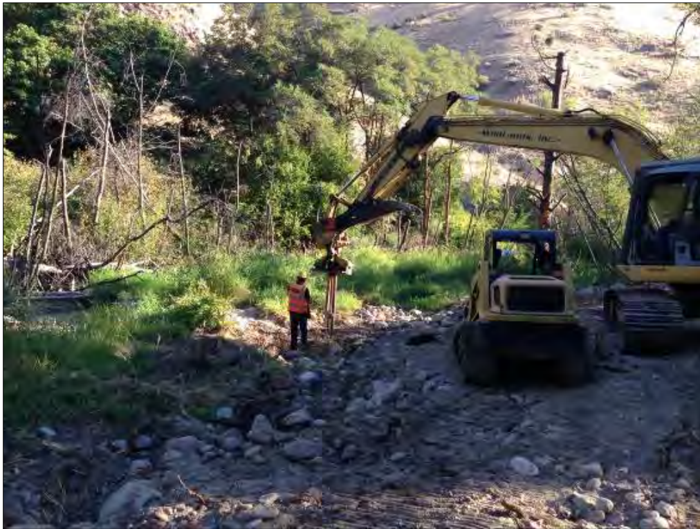
Photograph 56. An expandable stinger mounted on a track hoe for planting the eliminated levee area near inlet
