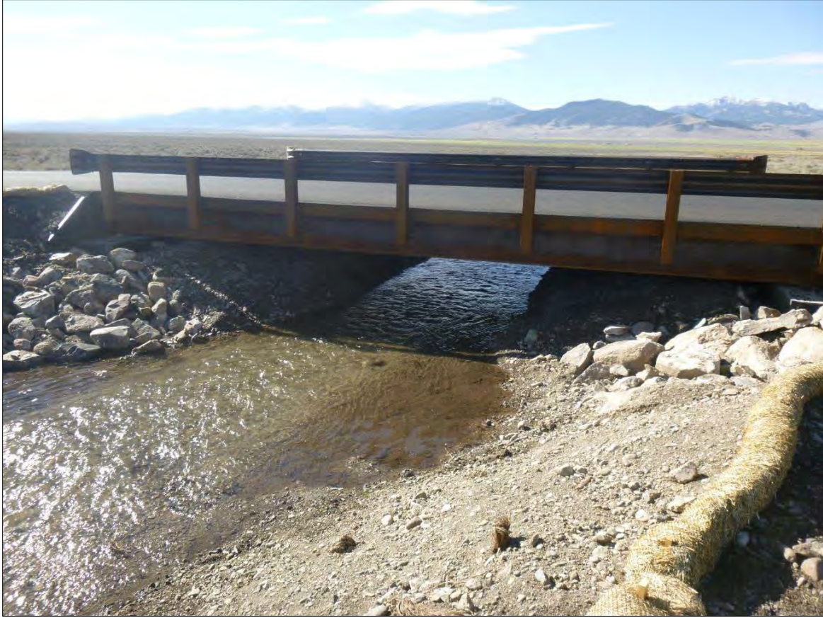
Photograph 2. Hawley Creek Bridge after construction; fish passage is greatly enhanced during all flows.
