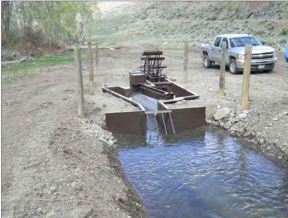
Photograph 19. A new fish screen was installed at the consolidated diversion to ensure that fish remain in the stream.
