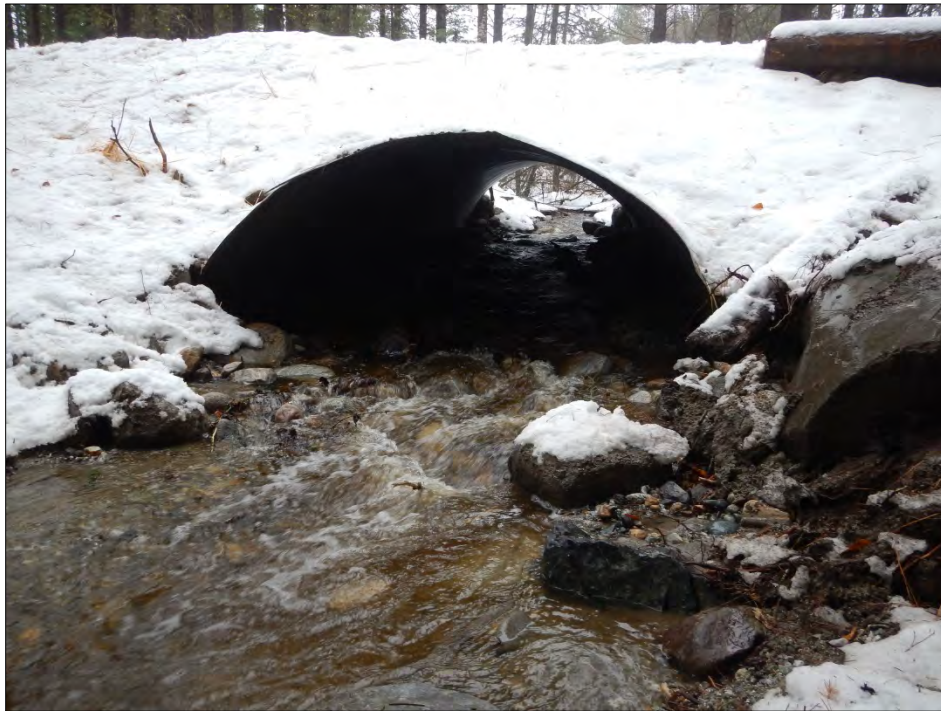
Photograph 85. The completed project allows for fish passage at all flows and all life stages.
