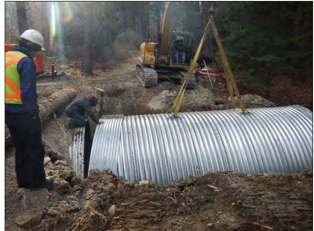
Photographs 81 and 82. The contractor and field engineer discussing progress and installation of second half of the arch pipe
