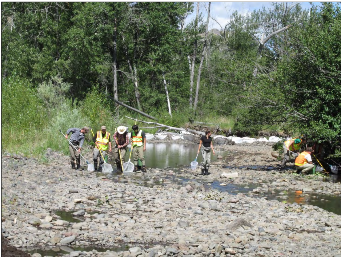
Photograph 38. Employees from ODFW, CTUIR, and Reclamation complete fish salvage on the roughed channel area before construction. In order to avoid and minimize impacts on ESA-listed fish species and other aquatic species, non-lethal methods are used to remove fish and relocate them downstream.
