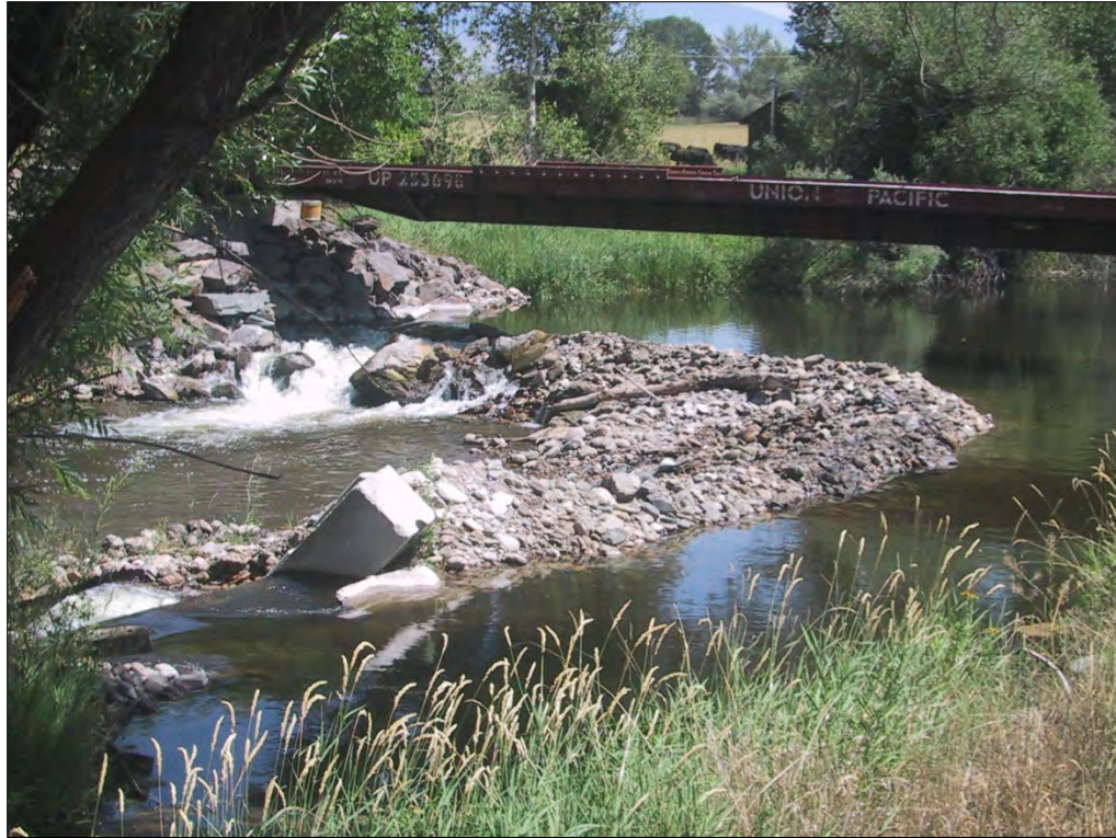
Photograph 3. Lemhi River at L-1 Diversion before the project, with the push-up dam in place
