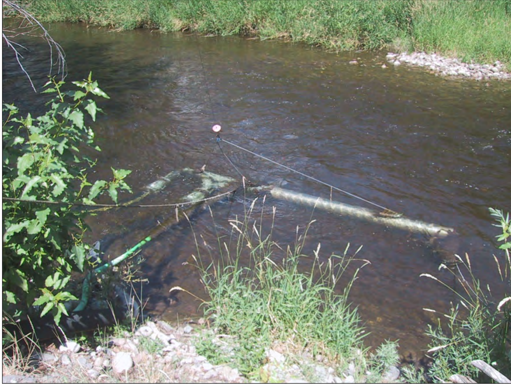
Photograph 7. New L-1 fish screen and pump intake
