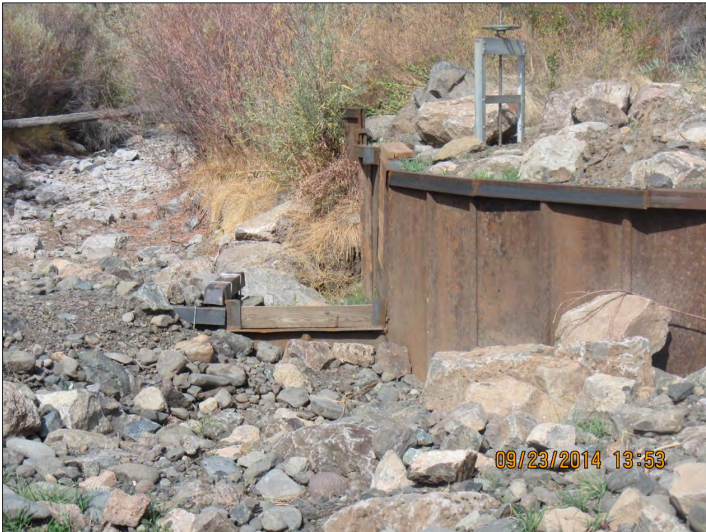
Photograph 47. Photo of completed diversion project showing low flow notch with flashboard in place
