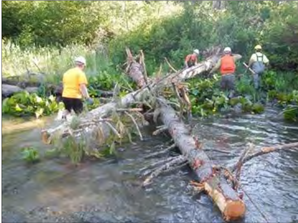
Photograph 87. Logs placed by helicopter lessened the construction impacts of the project while increasing the work efficiency.
