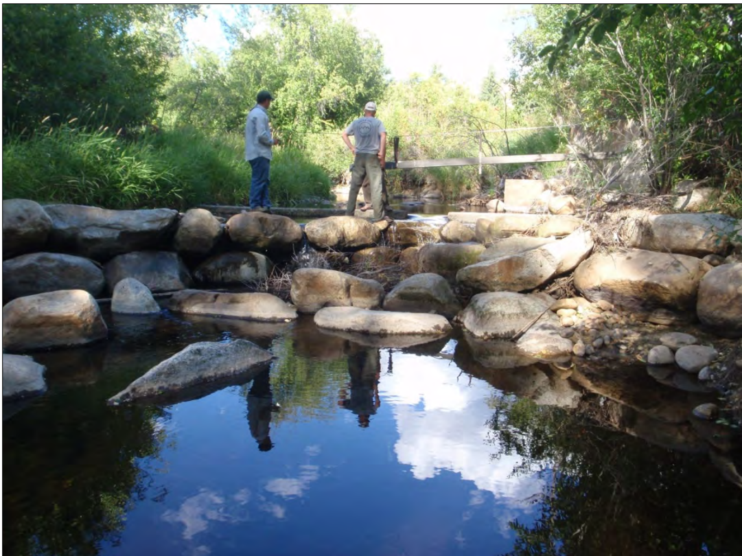
Photograph 68. The Fort Thurlow diversion before construction, showing portions of the diversion weir that were damaged by the 500-year flood event
