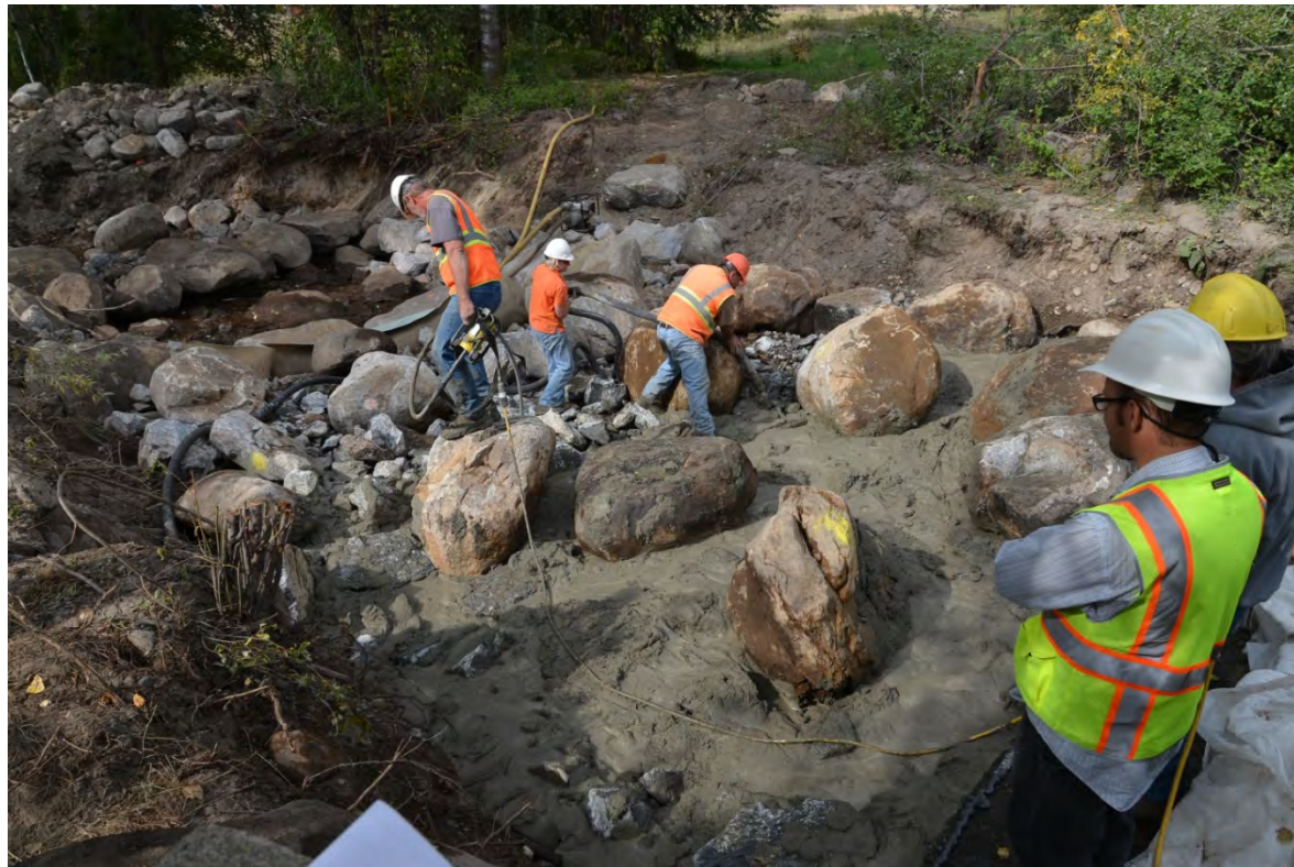
Photograph 70. The chute-pool roughened channel design called for grouting a portion of the engineered materials to create the desired fish passage channel.
