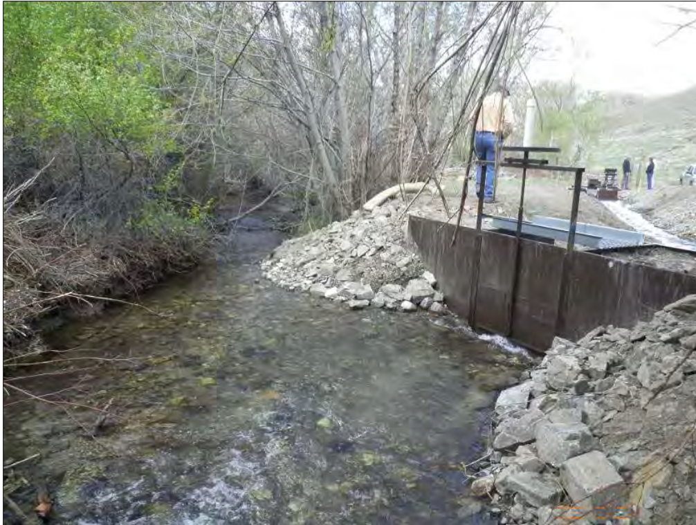
Photograph 18. The new consolidated diversion along with the efficiency improvements ensures that 9.2 cfs are available for fish passage and habitat.
