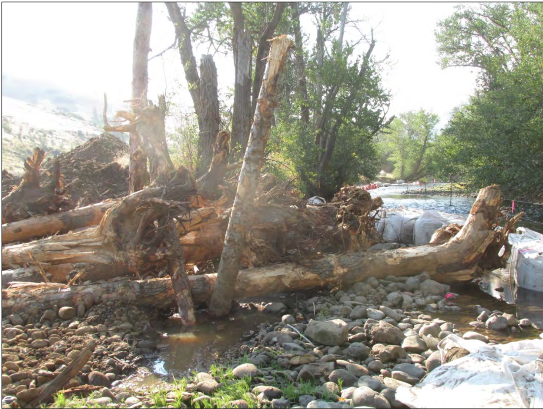
Photograph 40. This LWM structure is intended to provide habitat during all flows and rack material during high flows. It will also promote bed scour and gravel recruitment.
