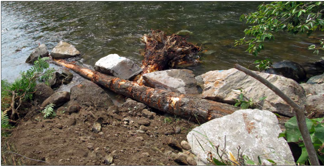
Photograph 61. Habitat log structure and boulders at RM 1.6
