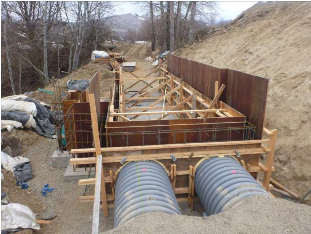
Photograph 72. The Dempsey drop control structure in the Chewuch Canal is the start of the project. The water is screened for trash and flows a short distance in twin HDPE pipes.
