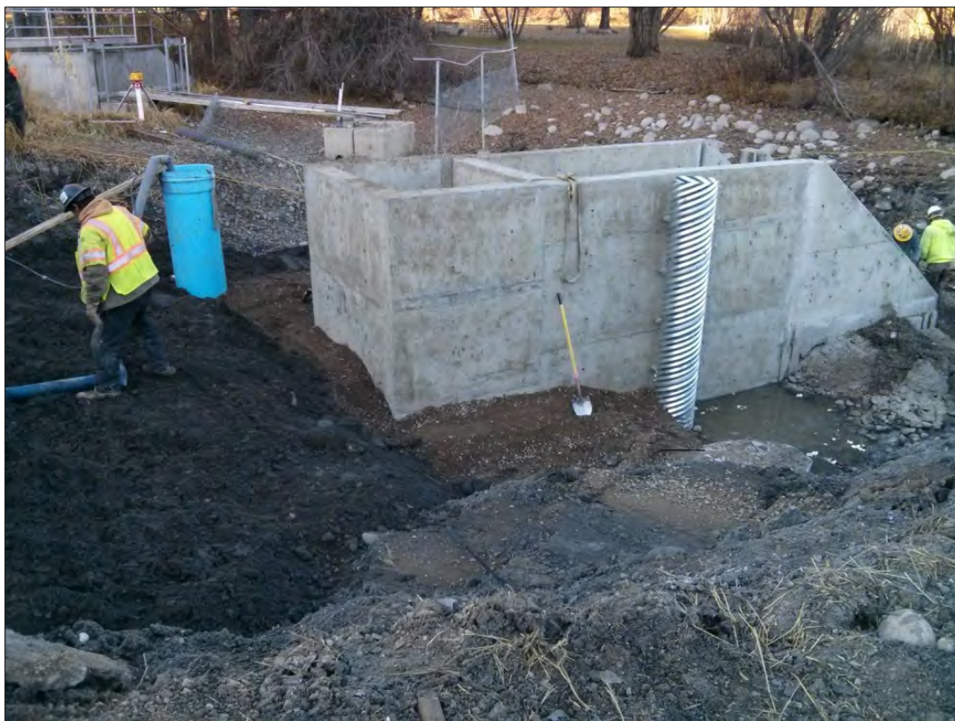
Photograph 74. Outlet works/ inflow Structure at Pearrygin Lake is designed to fill or withdraw water from reservoir and allows a greater efficiency of the reduced diverted flows.
