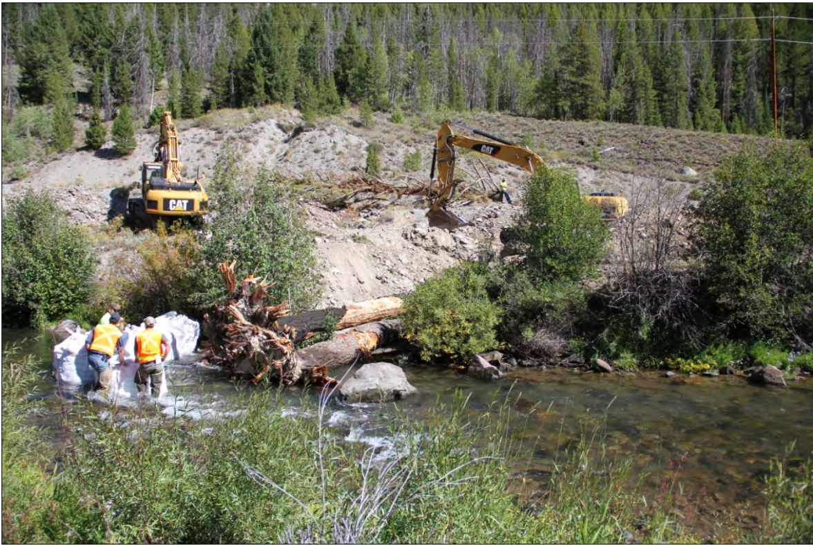
Photograph 34. Installation of one of 13 log and rock structures added to the Preachers Cove reach as part of the project
