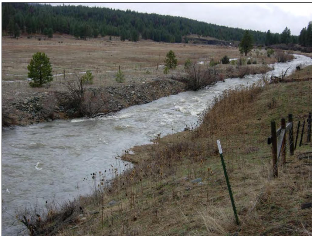
Photograph 42. Before Phase 3, the Middle Fork John Day River flowed through a confined and straightened dredge channel in the project area.
