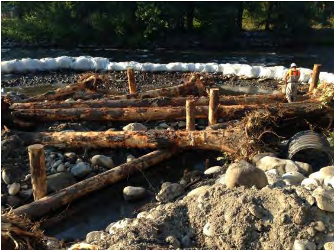
Photograph 54. A Type 4 structure under construction at the side channel inlet
