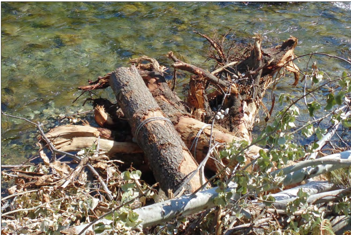
Photograph 64. Margin wood added to the Entiat River provides rearing habitat and refuge for juvenile fish.
