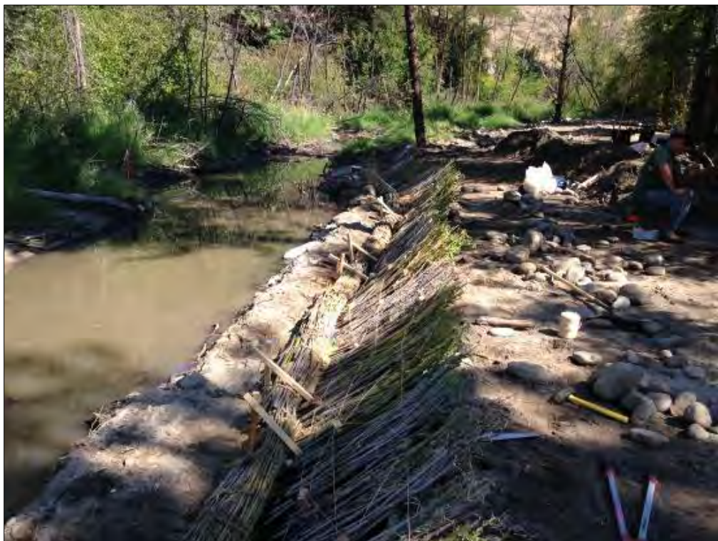
Photograph 57. Brush mattress installation in the Harrison side channel will provide additional fish habitat.
