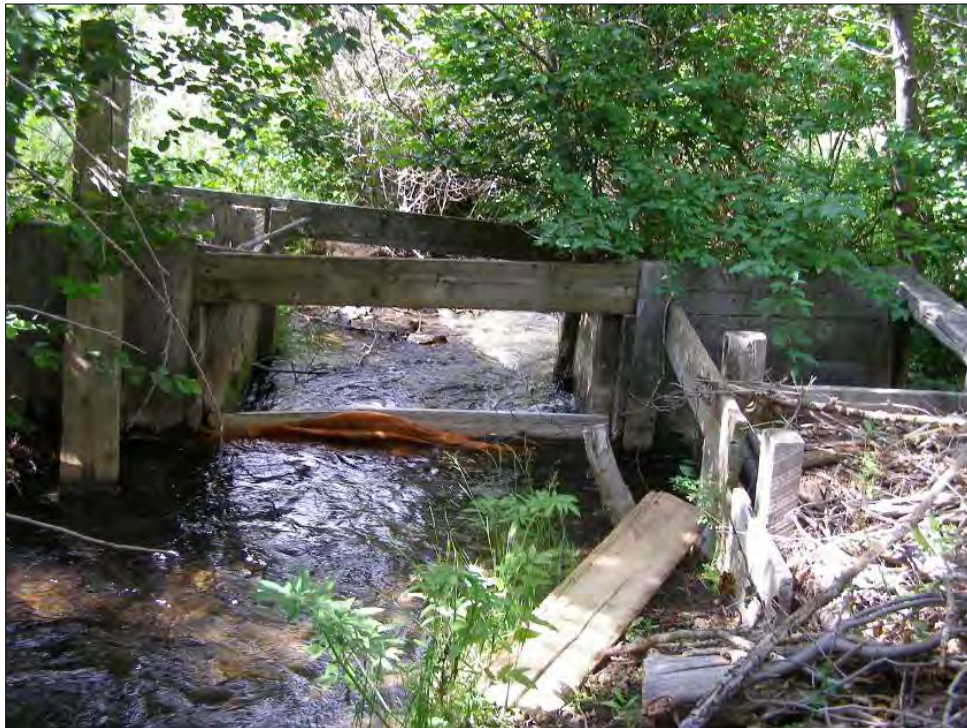
Photograph 17. One of the passage-blocking diversions that was removed by the project
