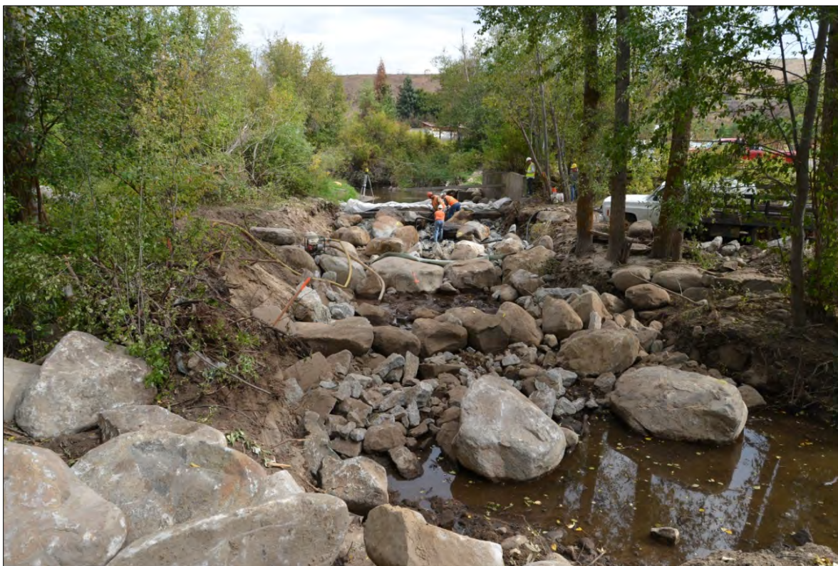
Photograph 69. The Fort Thurlow diversion during construction, with Beaver Creek flows bypassed around the site
