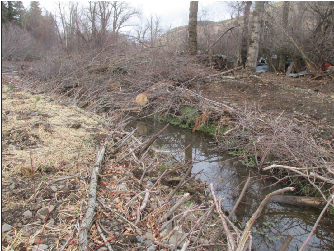
Photograph 36. This photo of the side channel shows a brush mattress structure that was created during the project. The purpose of the brush mattress is to control bank erosion while also providing shade to the stream. This lowers water temperatures and offers protection from predators to improve fish habitat.
