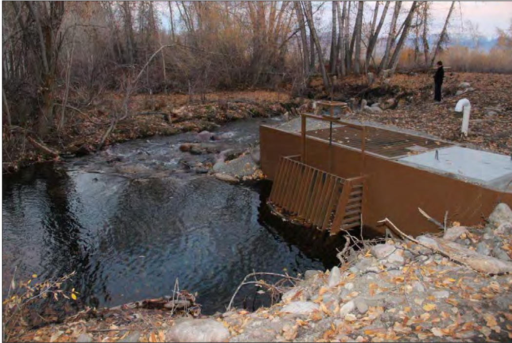
Photograph 14. A new diversion was established approximately 100 yards upstream of the old diversions. This diversion provides passage to fish at all life stages.
