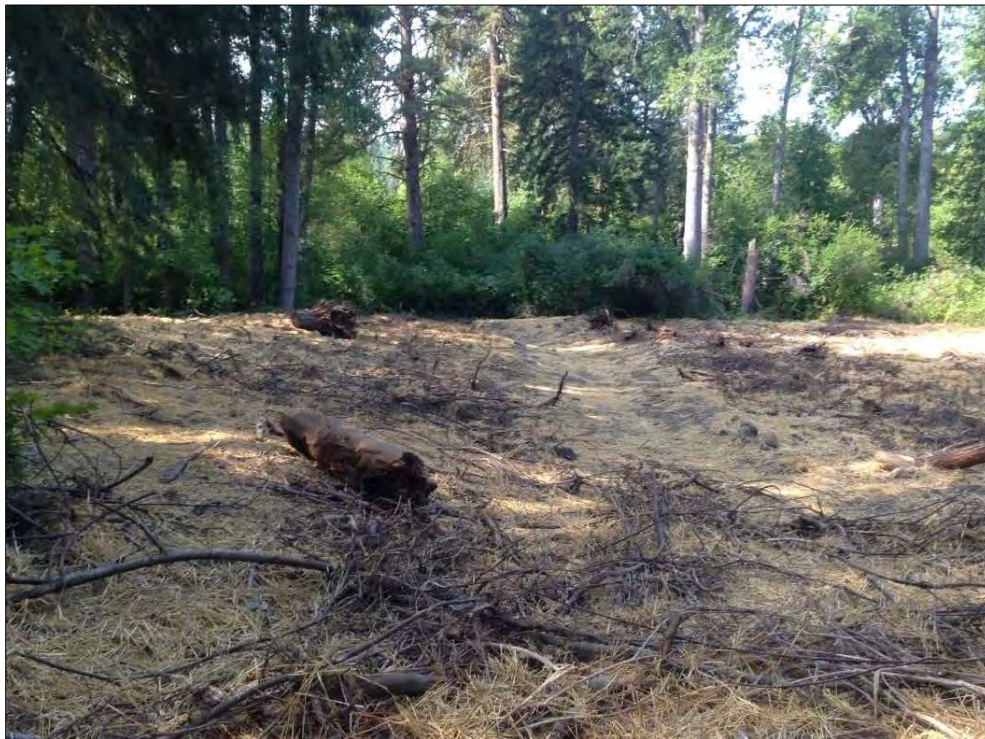
Photograph 88. Anthropogenic fill in the floodplain was removed to allow Nason Creek greater access to the flood plain.
