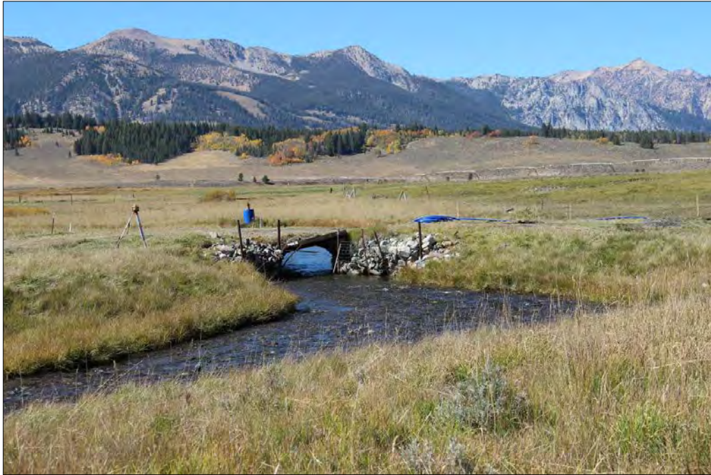
Photograph 22. This culvert providing access across Pole Creek was removed because it did not meet fish-passage criteria.
