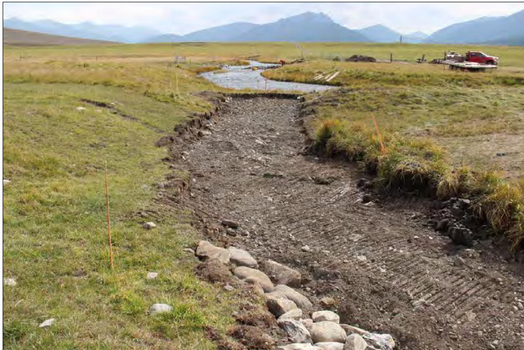
Photograph 23. This portion of the historic channel was cut off when the culvert was installed years ago. The channel was re-constructed as the culvert was removed. The photo was taken just prior to Pole Creek being moved back into it. Wetland sod has been placed along the bank, and willows were added later.
