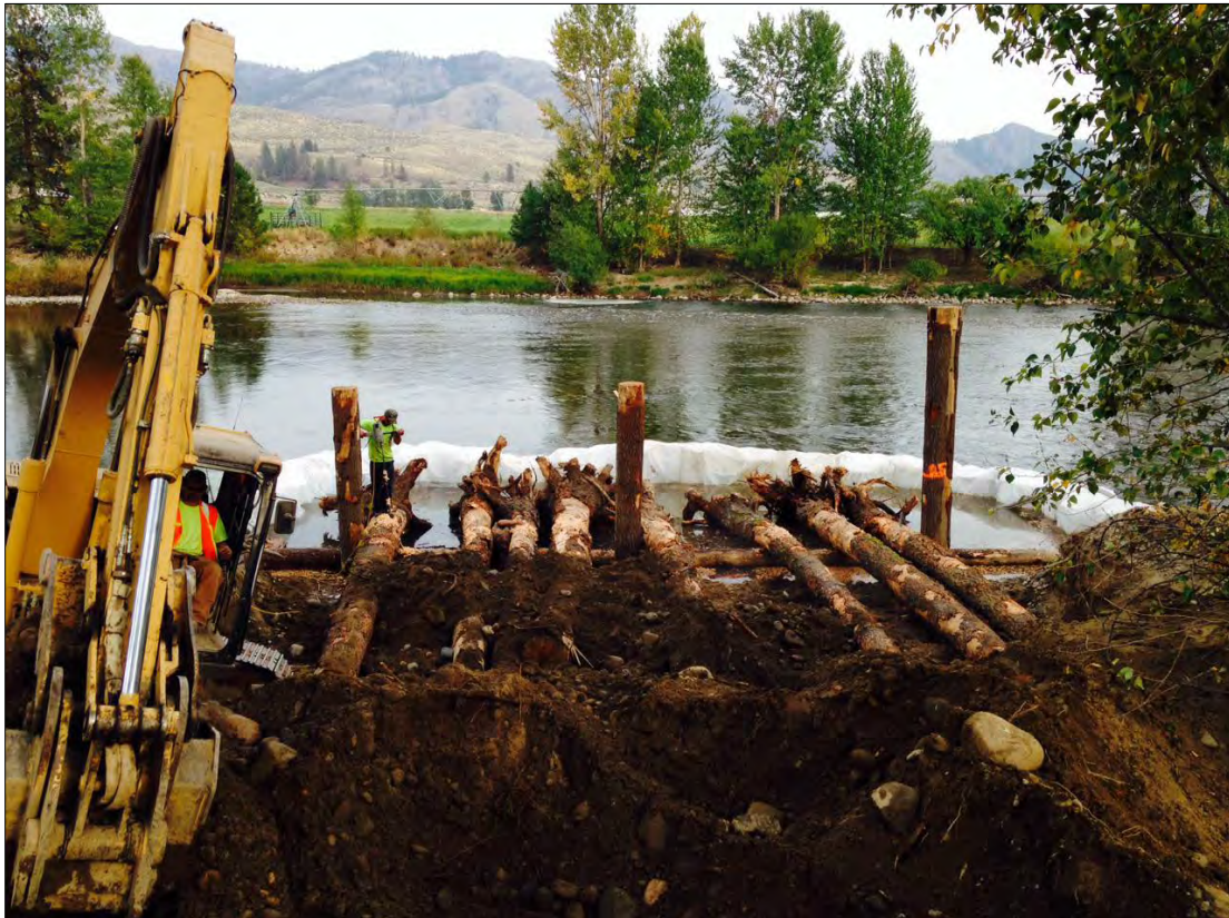
Photograph 75. View shows construction of one of the engineered log jams along the right bank of the Methow River in the project area.
