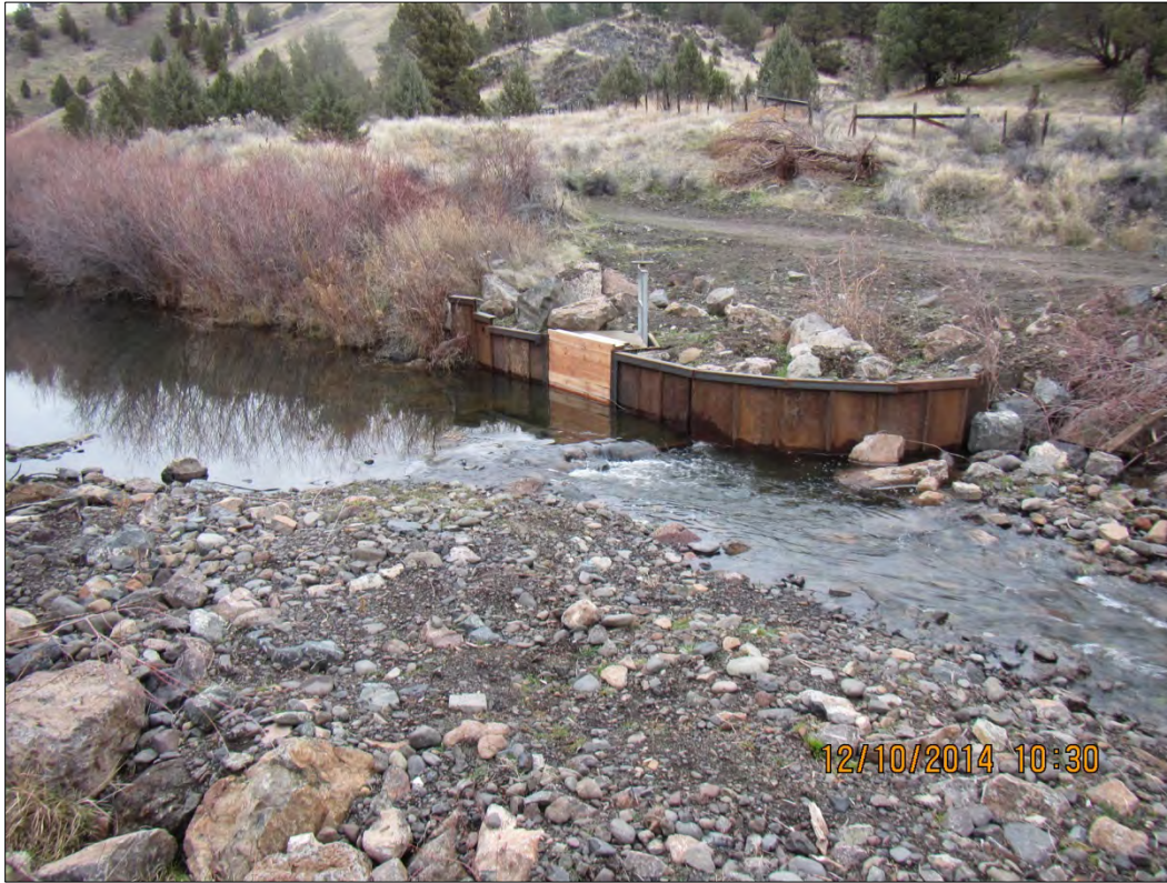
Photograph 49. Completed diversion structure showing submerged concrete head gate box protected by flash boards and the low flow notch
