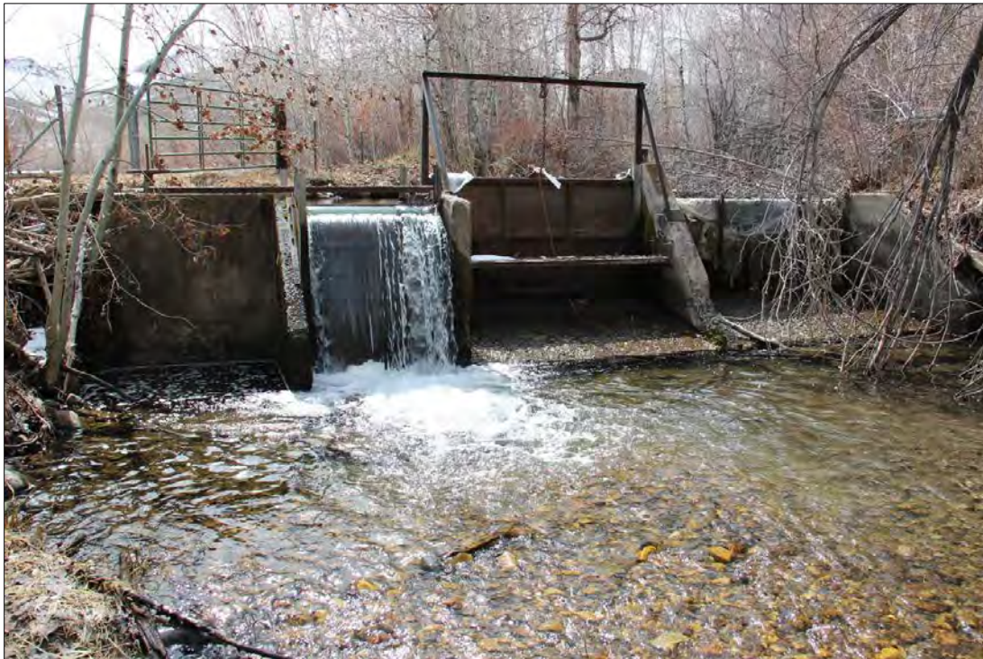
Photograph 12. City of Challis diversion structure on Garden Creek; this structure was a complete barrier to fish movement. It was removed as part of this project.
