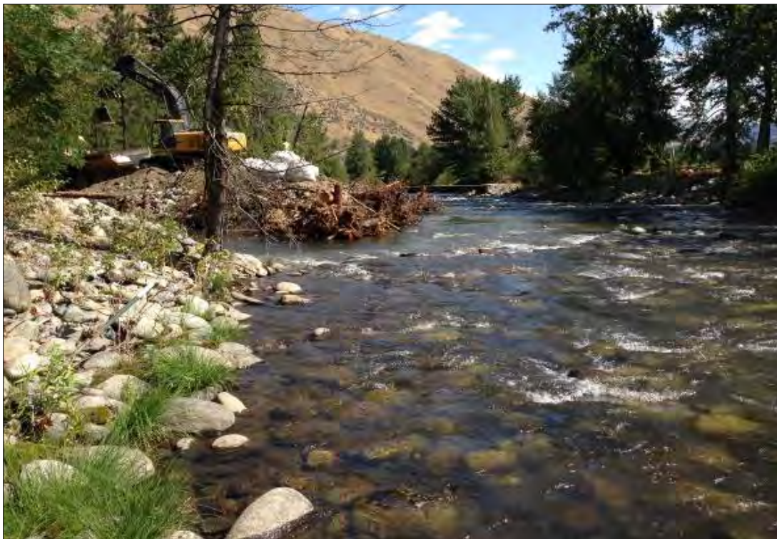
Photograph 55. Side channel inlet from upstream, featuring the new ELJ at the inlet to the side channel
