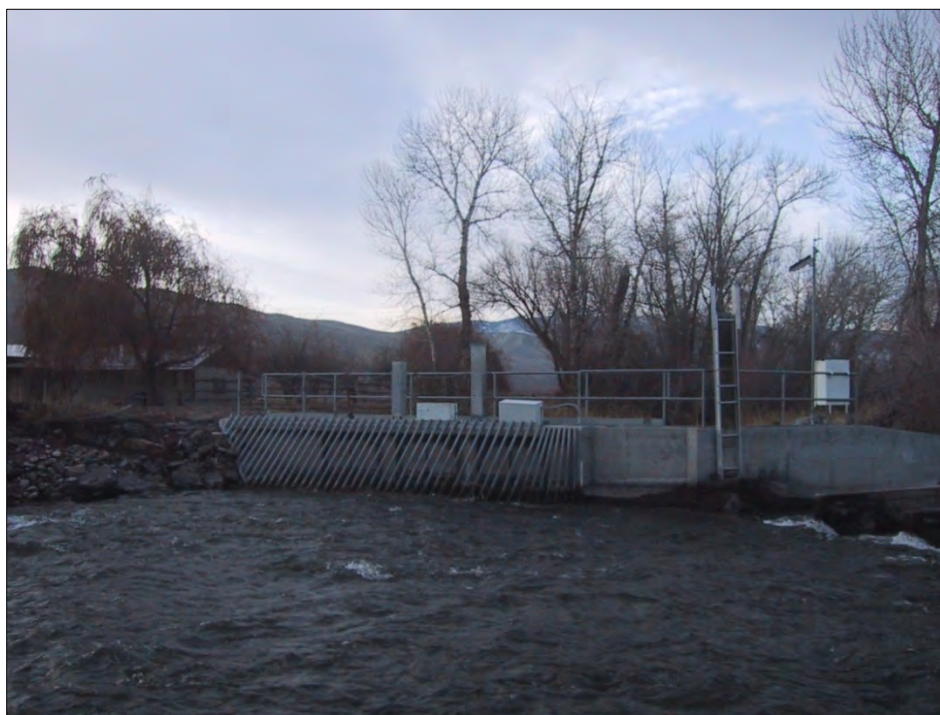
Photograph 9. With the headgate automated, the system will ensure that flows in the river receive first priority and the L-6 diversion flows are second priority.
