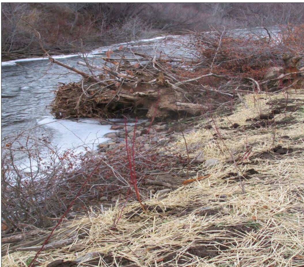
Photograph 37. This view shows a LWM structure on the right bank of Catherine Creek. It is intended to provide habitat during all flows and rack material during high flows. The LWM structure will promote bed scour and gravel recruitment.
