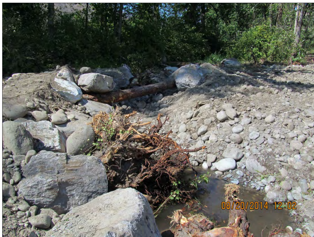
Photograph 60. Side channel outlet at RM 1.6 with wood and rock installed as part of the project.
