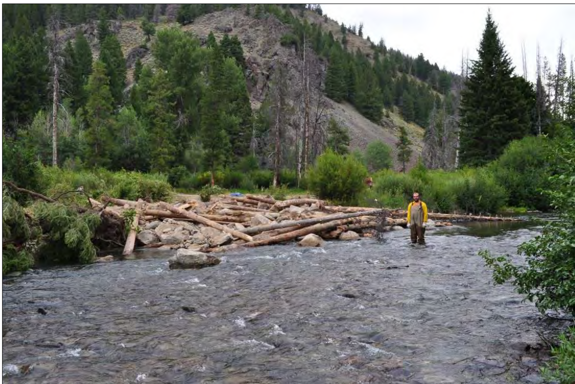
Photograph 29. The completed simulated debris flow will allow holding areas for adult fish and refuge for juvenile rearing.
