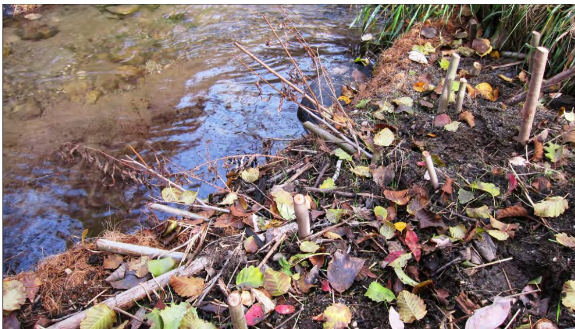
Photograph 79. Riparian enhancement by installing willow plantings
