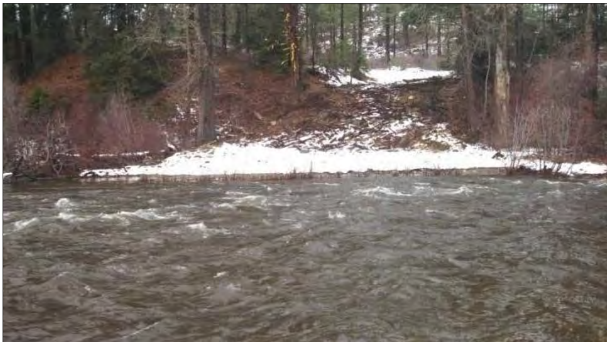
Photograph 90. Removal of the old bridge abutment allowed Nason Creek flows to access the area during a 2-year flow event.
