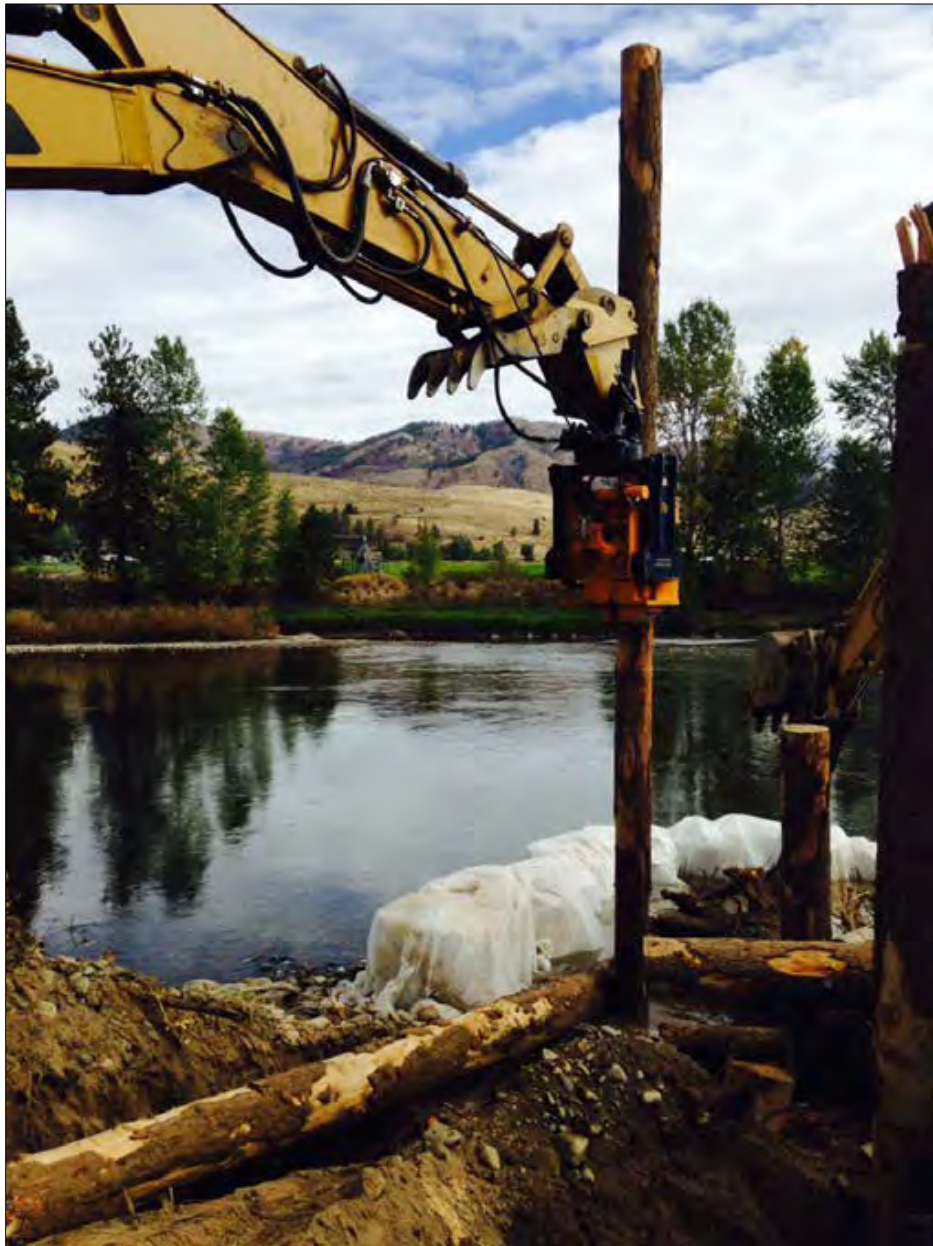
Photograph 76. Vibratory pile driver at work placing vertical piles as part of the ELJs, which were constructed as project features to enhance fish habitat for juvenile salmon and steelhead.
