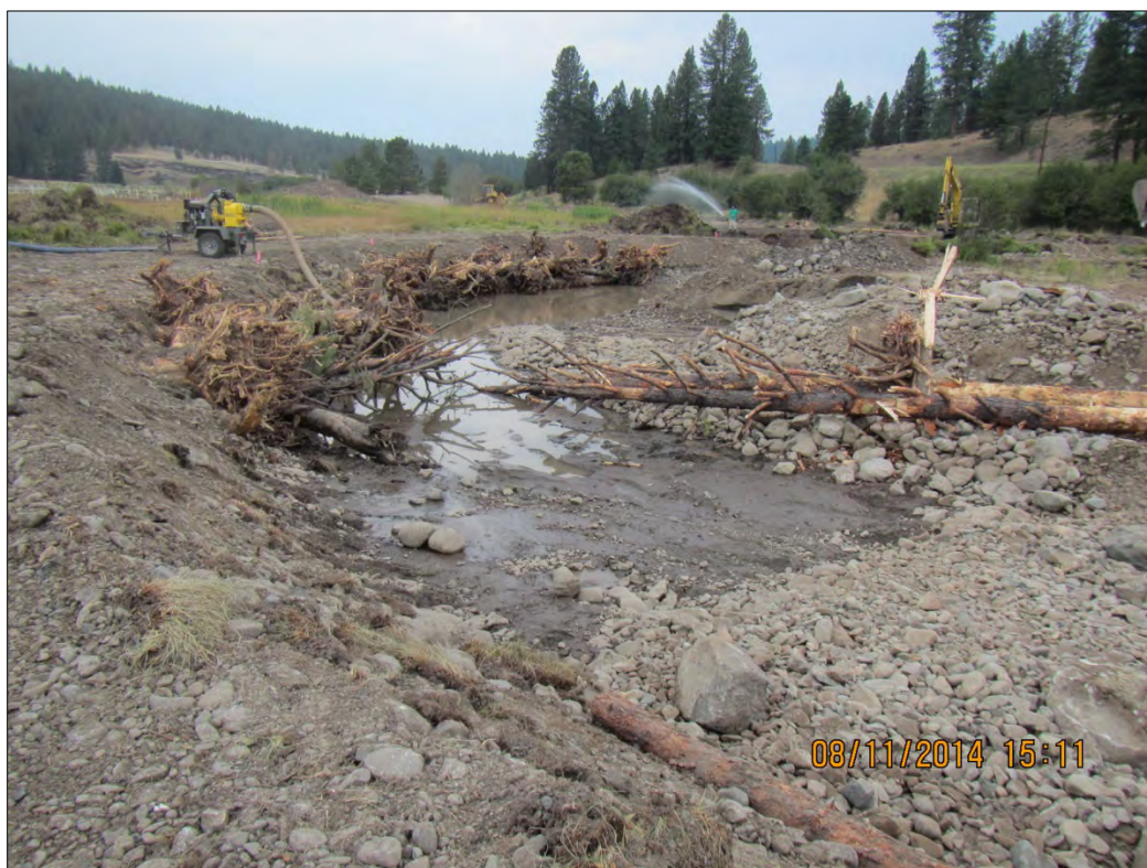
Photograph 43. A new channel section during construction, prior to releasing the Middle Fork flows into it
