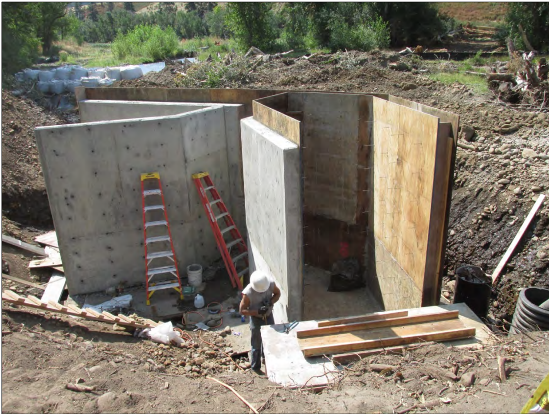
Photograph 41. This picture shows construction of the consolidated diversion and intake structure outside the creek near the roughened channel. The diversion design promotes natural river processes, allows fish passage for all life stages, removes three annual push-up dams, and consolidates three points of diversion into one.
