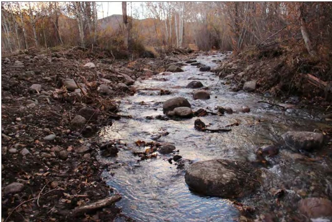
Photograph 15. The Garden Creek channel near the old City of Challis diversion structure. The channel was re-built with additional habitat features along the existing alignment where the old diversion structures were located. Large rock was installed to hold the channel at the new grade and provide fish habitat.
