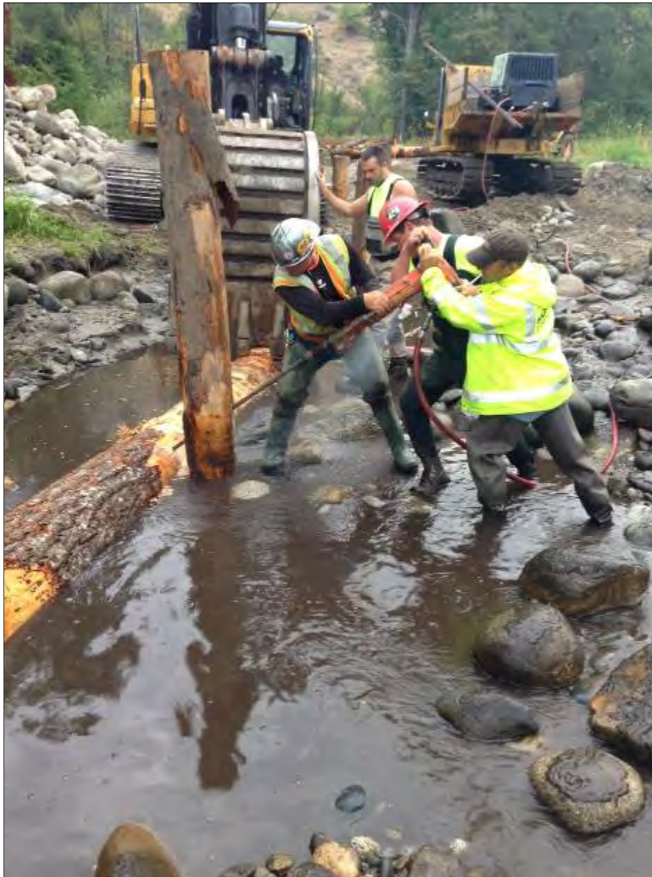
Photograph 53. Workers pin key members of an ELJ, which was established at the entrance to the Harrison side channel to enhance habitat and to encourage flow into the side channel.
