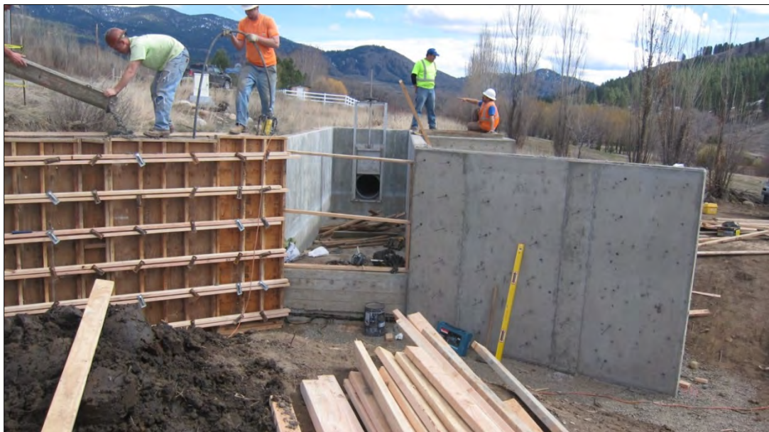
Photograph 73. The Silverline Control Structure screens the water as it enters the CCC pressure pipe system. Water can also be delivered to irrigated land above Perrygin Lake from this structure.
