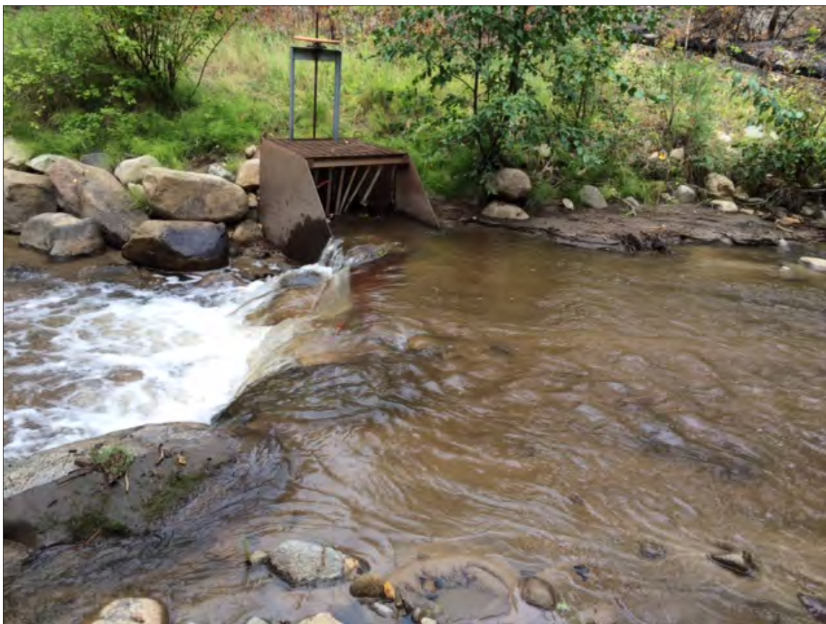
Photograph 65. The Marrachi diversion as damaged by the 500-year flood; the diversion weir provided some fish passage but not at all life stages.
