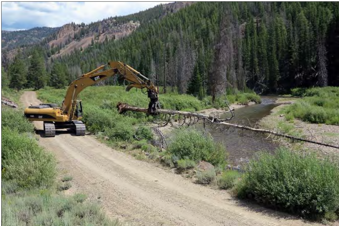
Photograph 27. Placement of trees in the Yankee Fork to enhance fish habitat using an excavator
