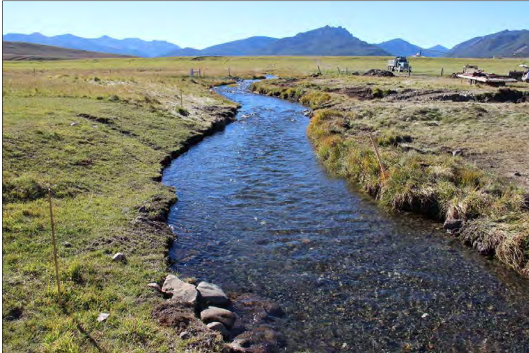
Photograph 24. Looking upstream along the same alignment as the previous photo, after water was returned to the historic channel alignment. Willow cuttings were planted along both sides of the new channel, and fencing installed to keep livestock out of the area.
