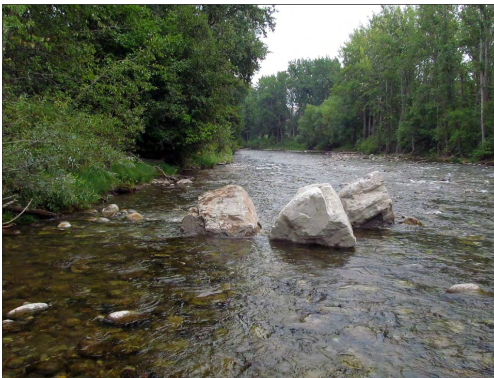
Photograph 59. Boulder cluster at RM 2.2 provides flow disruption and habitat variety.
