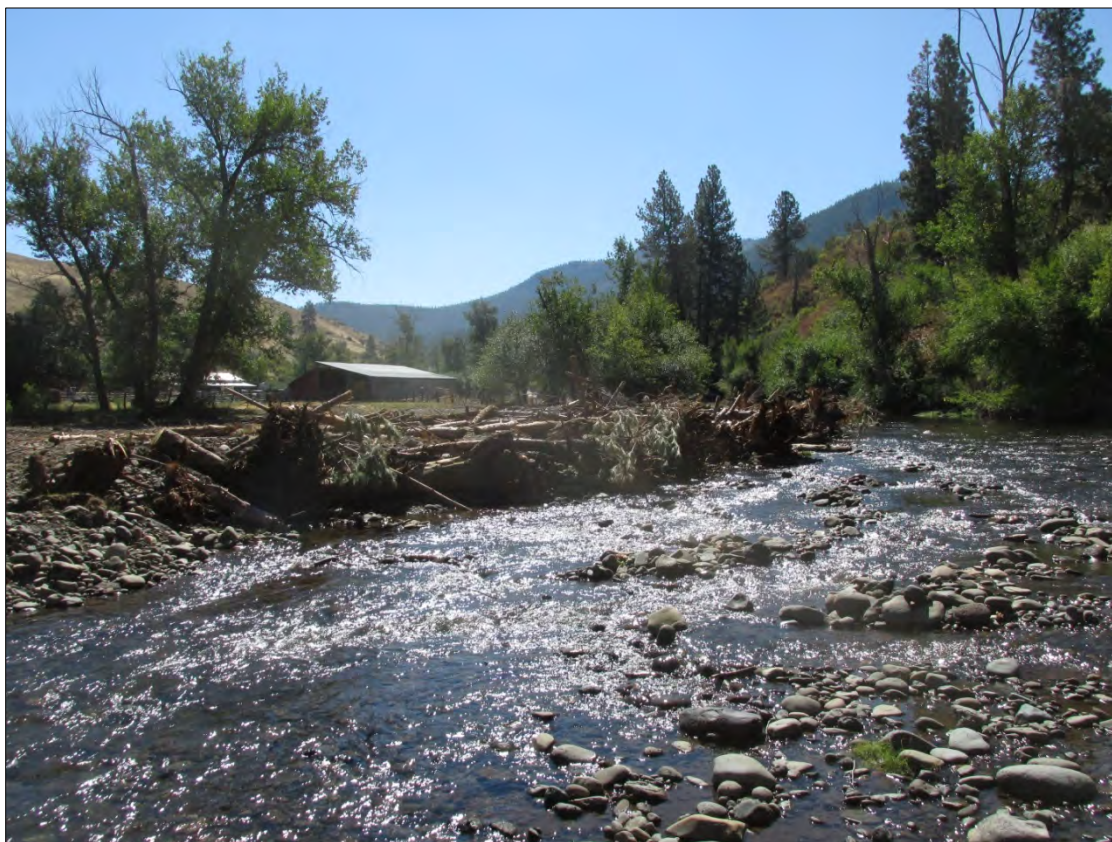
Photograph 39. This picture shows a LWM structure placed in a section of Catherine Creek that has over-widened due to excessive grazing. Removal of vegetation through overgrazing can lead to unstable banks and erosion during high flows. The LWM structure provides fish habitat, serves as a framework for channel narrowing, and is keyed into the existing bank to protect the right floodplain flank of the structure from channel avulsion.
