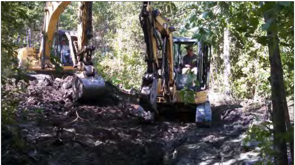
Photograph 62. Contractor excavating the deepened side channel to allow inundation at lower river flows
