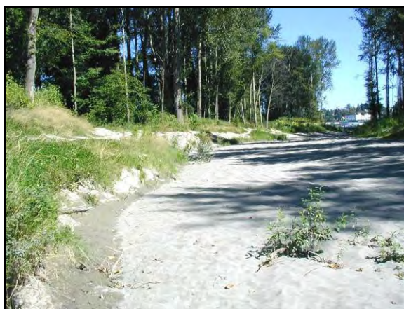
Dry side channel looking upstream in Year 3 (2007). A few of the willow stakes are growing through the sandfill in the lower right foreground.
