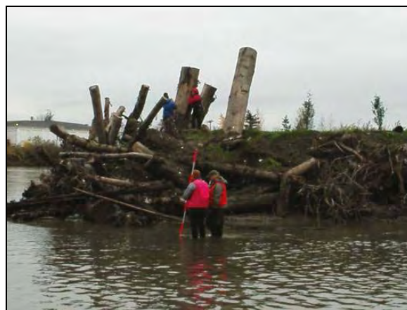
Upstream end of predicted paleo-channel in 2004 (Year 0) LWD placed in constructed channel (2005)
