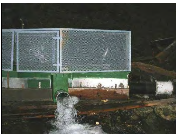
Diversion screen and bypass system at the McDaniel property (upper site) in Year 2 (2008)
