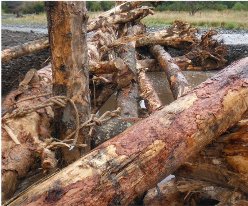
Photograph 9. Rope used as a fastener on a LWM structure.
