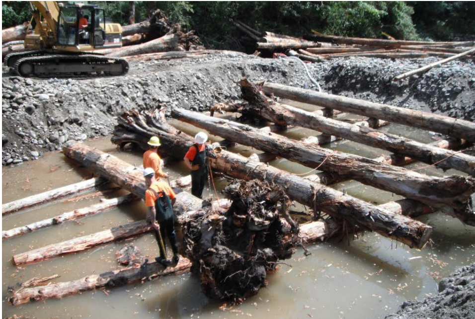
Photograph 5. Gravity foundation being installed on the Salmon River.
