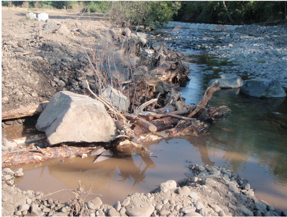
Photograph 3. Boulder ballast material placed on top of a LWM structure.
