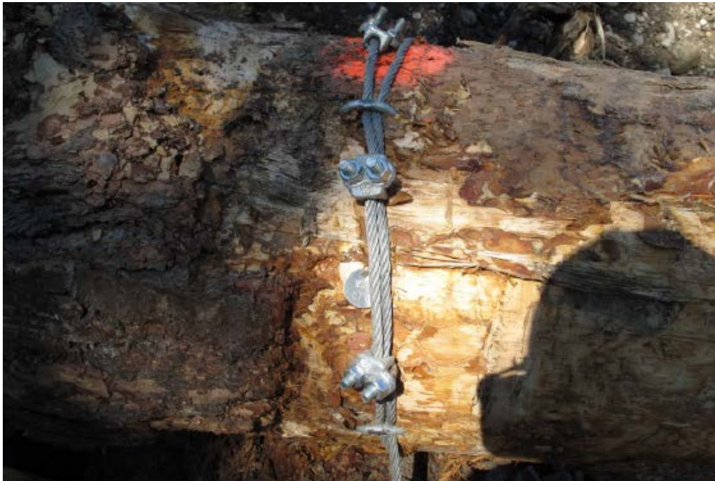
Photograph 18. LWM structure being connected with cable.
