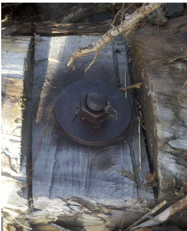
Photograph 13. Close-up view of threaded steel rod with connected with a wide washer and nut after being sprayed with rust inhibiting paint.
