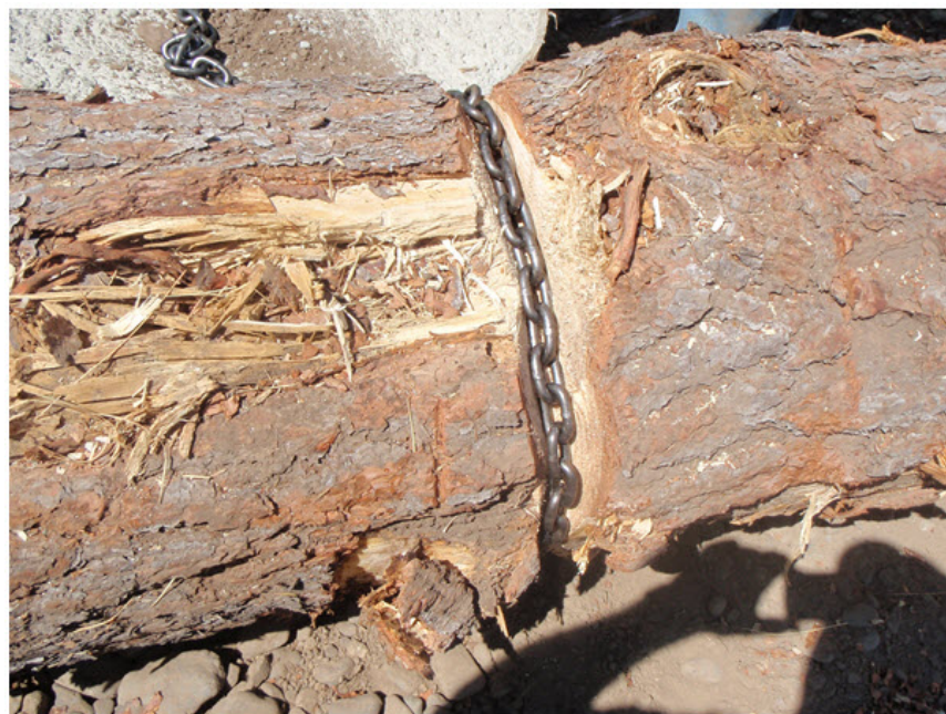
Photograph 15. Large log grooved with chain installed around the bole.
