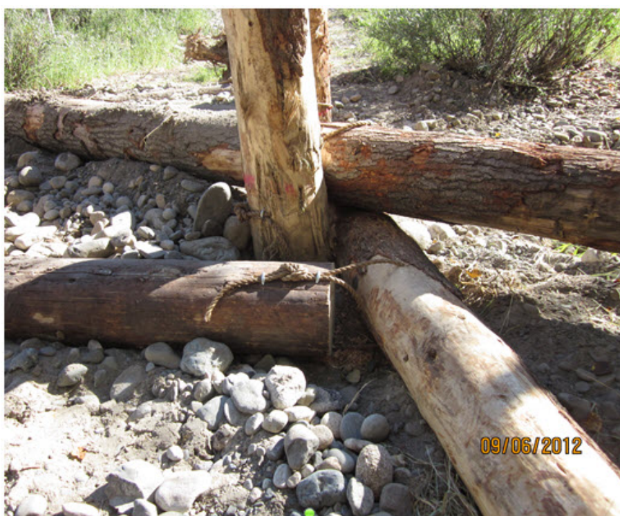
Photograph 8. Rope used as a fastener on a LWM structure.
