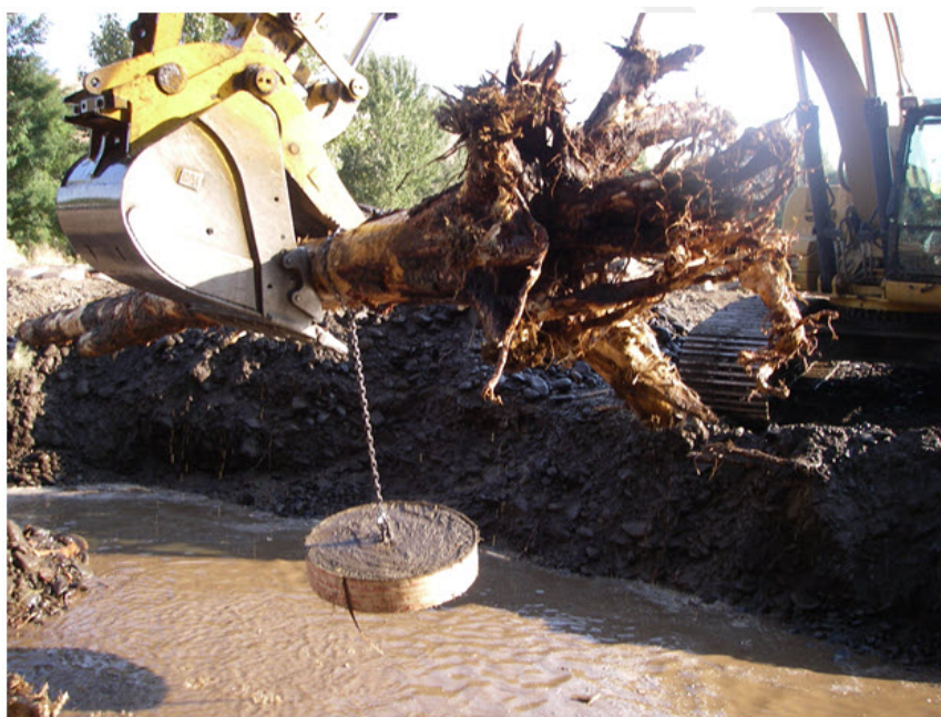
Photograph 7. Custom made concrete deadman anchor attached to chain and a key wood member to resist buoyant forces in a high risk location.
