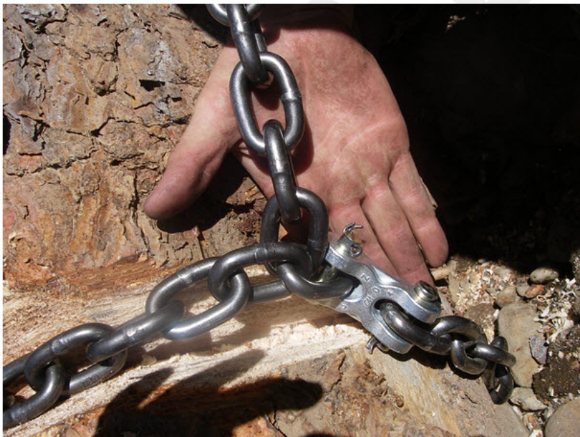
Photograph 16. A pin connection of chain anchor around a large log with chain leading to a deadman anchor.
