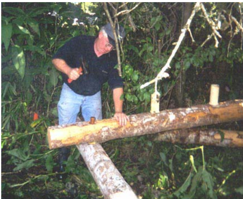
Photograph 10. Wood pins being installed to connect pieces of LWM.
