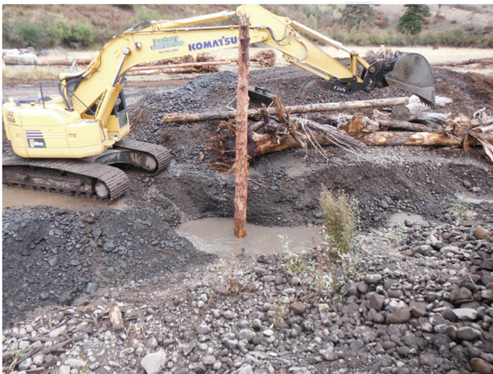
Photograph 4. Excavated pile being backfilled.
