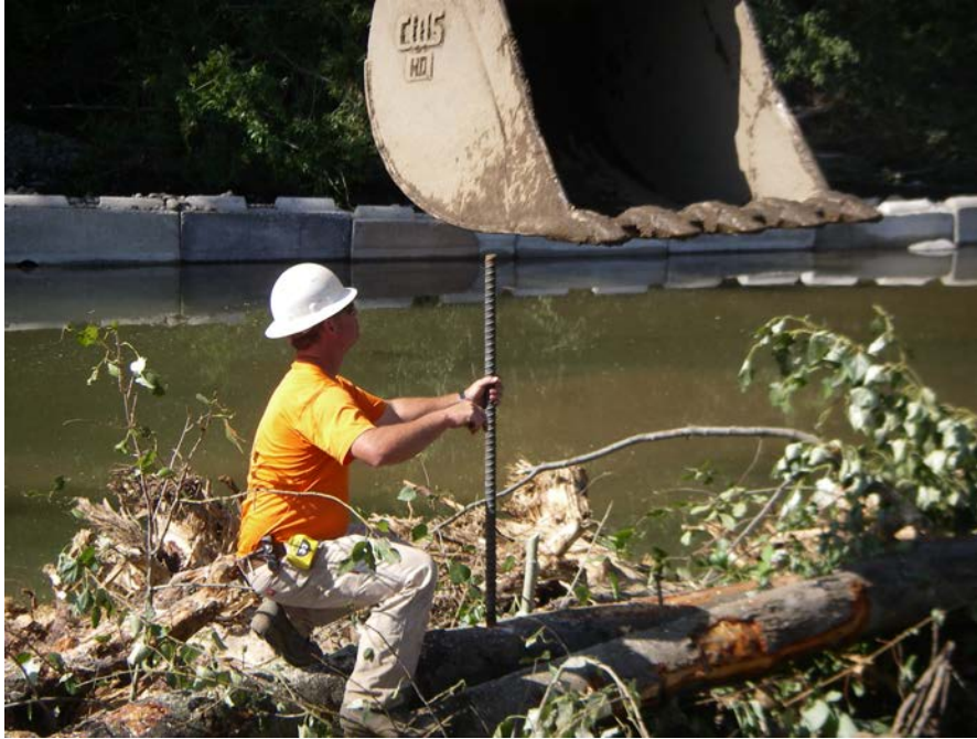
Photograph 11. An excavator pushing in a rebar steel pin into a LWM structure.
