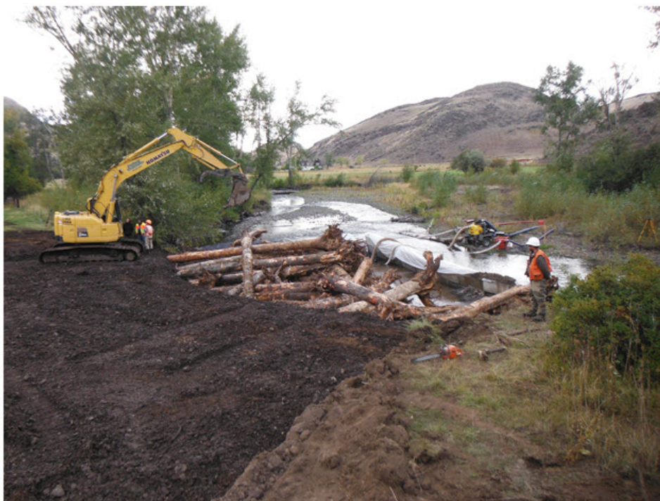
Photograph 2. Backfilling a LWM structure with native gravel material to increase stability.
