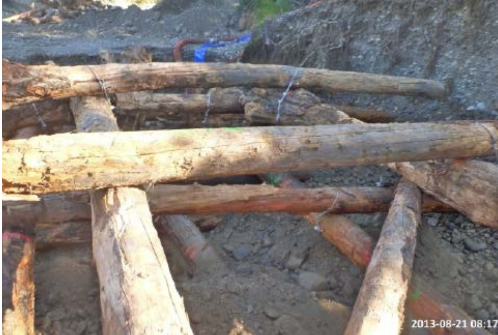
Photograph 17. LWM structure being connected with cable.
