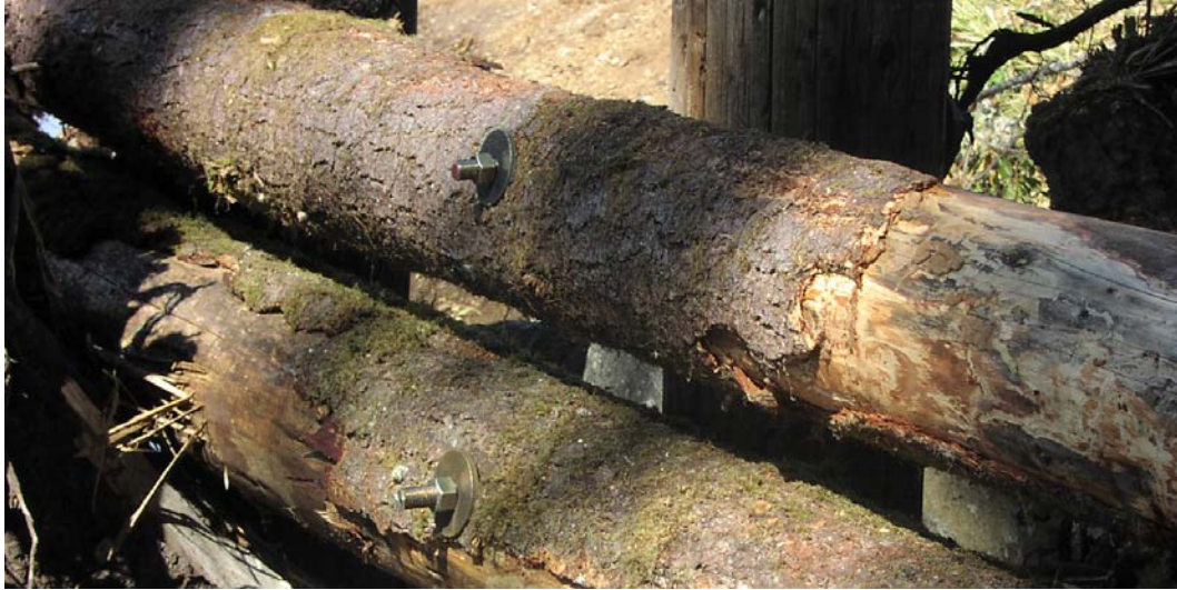
Photograph 14. View of threaded steel rods used to connect logs to a wooden pile for a LWM structure.
