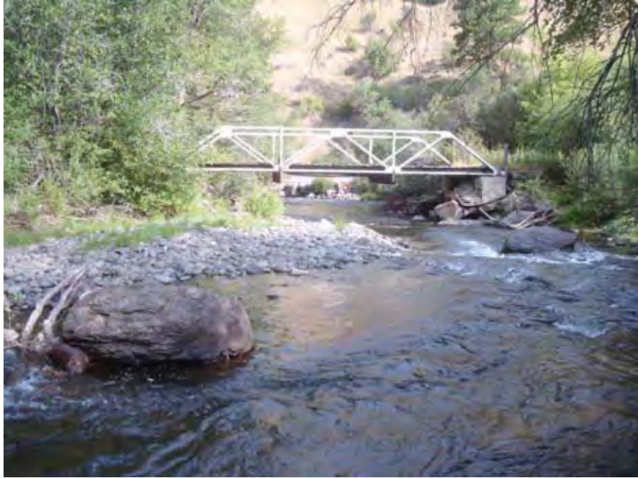
Photograph 43. View looking downstream at residential access bridge across Catherine Creek near river mile 47.15. Reach 5 – Catherine Creek, Grande Ronde Subbasin, Oregon – Bureau of Reclamation Photograph by D. Stelma, August 18, 2010.
