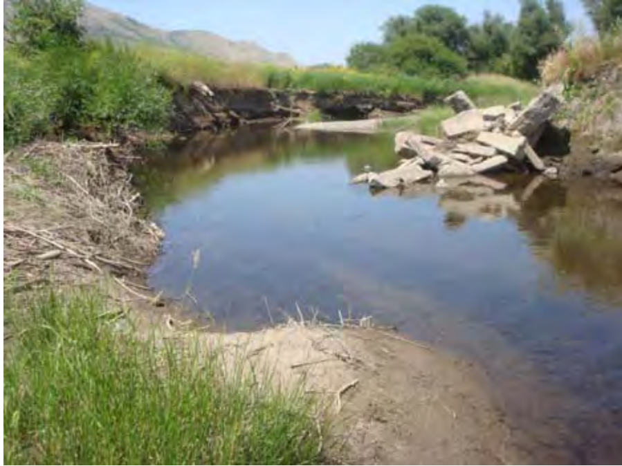
Photograph 72. View looking downstream at concrete blocks and wood debris on the banks of Catherine Creek near river mile 37.20. Reach 2 – Catherine Creek, Grande Ronde Subbasin, Oregon – Bureau of Reclamation Photograph by D. Stelma, August 3, 2010.
