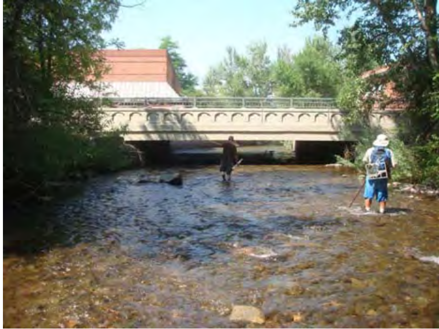
Photograph 21. View looking downstream at the North Main Street Bridge over Catherine Creek in Union, OR near river mile 40.01. Reach 3 – Catherine Creek, Grande Ronde Subbasin, Oregon – Bureau of Reclamation Photograph by D. Stelma, August 2, 2010.
