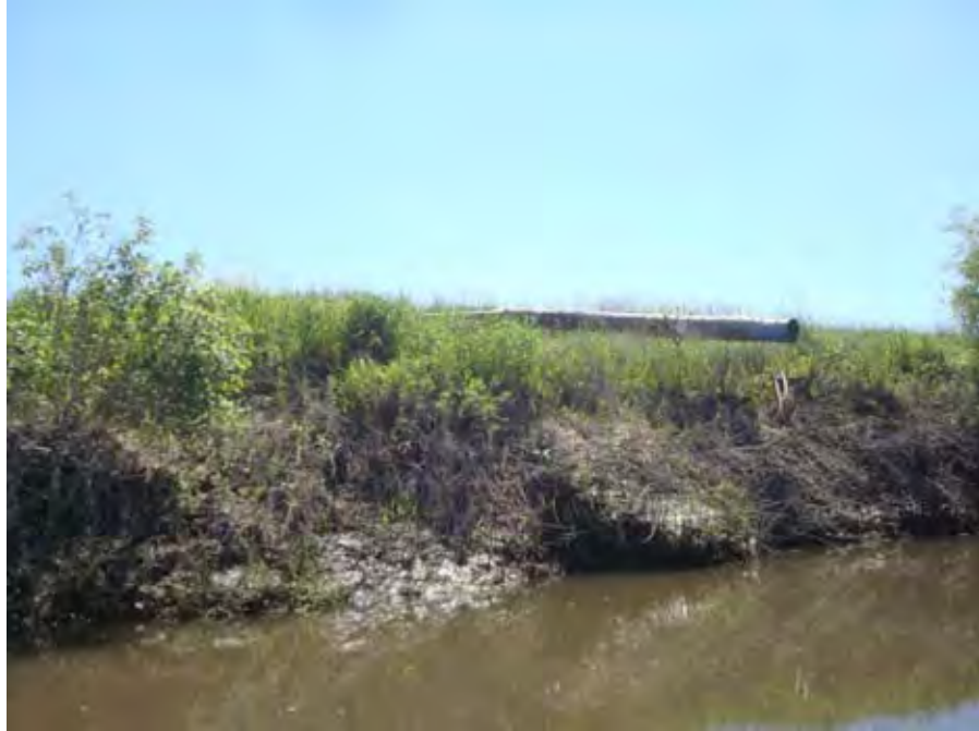
Photograph 104. View looking upstream at field/levee drain discharge pipe on right (east) bank of Catherine Creek (foreground) near river mile 0.47. Reach 1 – Catherine Creek, Grand Ronde Subbasin, Oregon – Bureau of Reclamation Photograph by D. Stelma, July 8, 2010.
