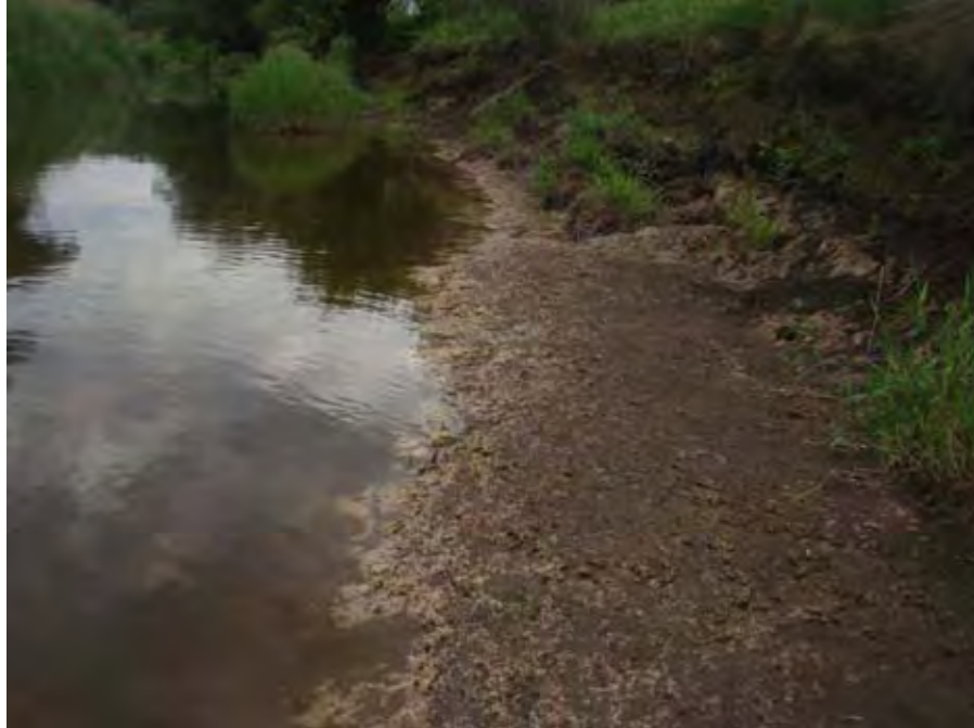
Photograph 158. A view from the right bank looking downstream at an exposure of the hard, firm fine grained material that is erosion resistant at the toe of the right bank on the outside of a meander bend at river mile 31.00, and bank slumping just downstream. Reach 2 – Catherine Creek, Grande Ronde Subbasin, Oregon – Bureau of Reclamation Photograph by R. McAfee, July 28, 2010.
