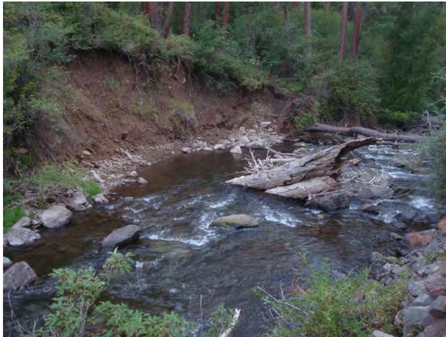
Figure 20. View looking downstream along a section where the left bank of Catherine Creek is comprised of landslide debris (Qls) near river mile 46.21. Catherine Creek Tributary Assessment-Grande Ronde River Basin-Tributary Habitat Program, Oregon – Bureau of Reclamation - August 18, 2010.
