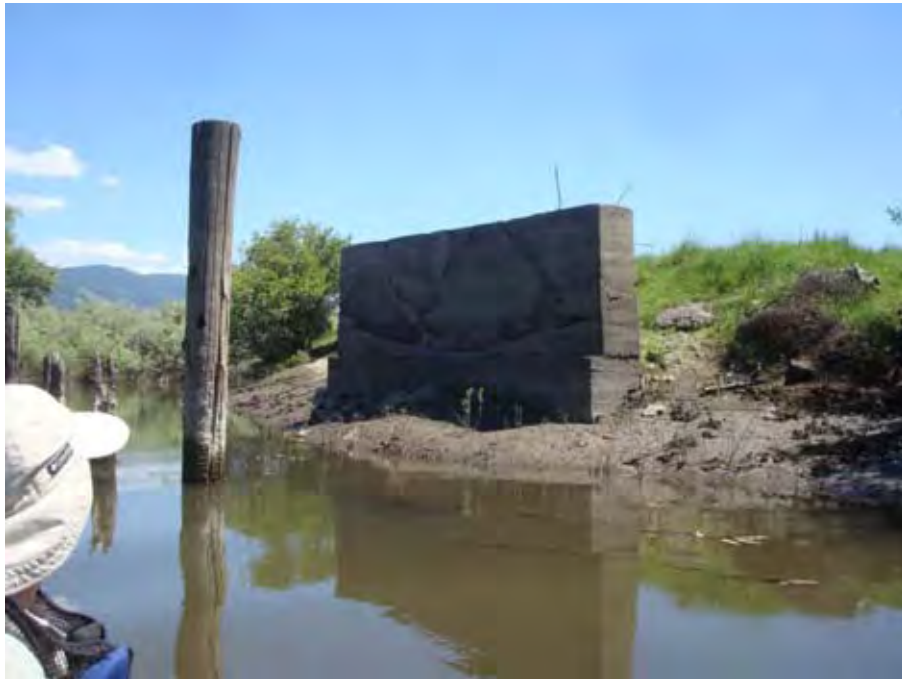
Photograph 80. View looking upstream at abandoned concrete bridge abutment near river mile 7.60. Reach 1 – Catherine Creek, Grande Ronde Subbasin, Oregon – Bureau of Reclamation Photograph by D. Stelma, July 7, 2010.
