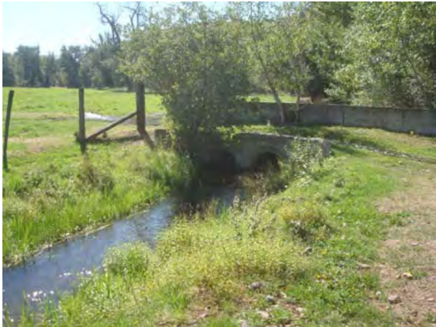
Photograph 62. View looking upstream at intake structure, farm access road and culverts near river mile 41.19. Reach 4 – Catherine Creek, Grande Ronde Subbasin, Oregon – Bureau of Reclamation Photograph by D. Stelma, August 16, 2010.
