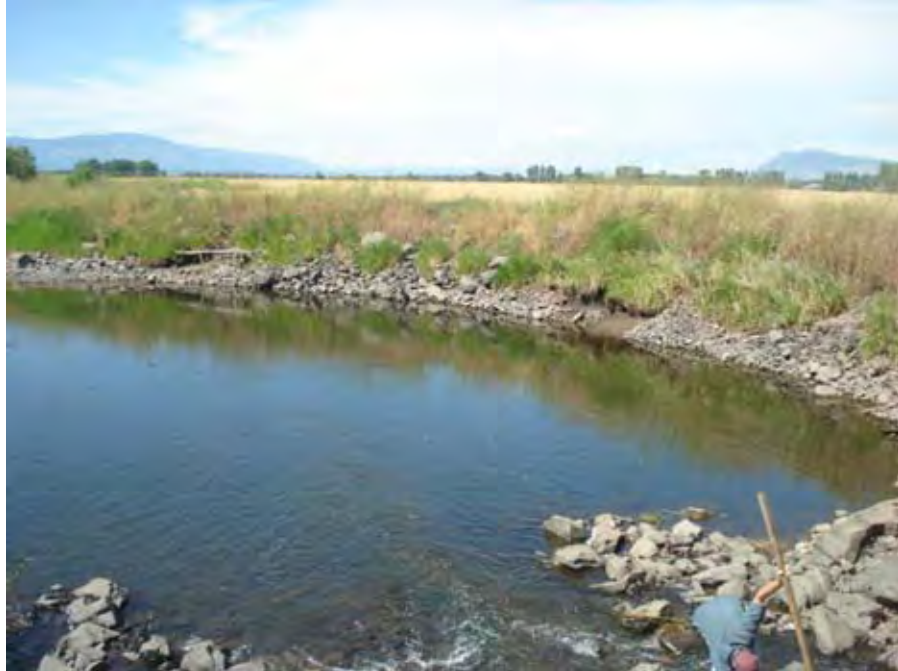
Photograph 33. View looking downstream from Upper Davis Dam at the riprap across the bottom of the channel and along the right bank near river mile 34.98. Reach 2 – Catherine Creek, Grande Ronde Subbasin, Oregon – Bureau of Reclamation Photograph by R. McAfee, July 27, 2010.
