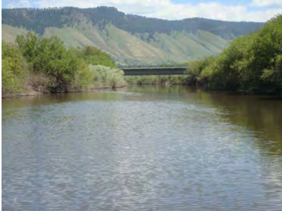
Photograph 85. View looking upstream at Market Lane Bridge near river mile 6.50. Reach 1 – Catherine Creek, Grande Ronde Subbasin, Oregon – Bureau of Reclamation Photograph by D. Stelma, July 7, 2010.
