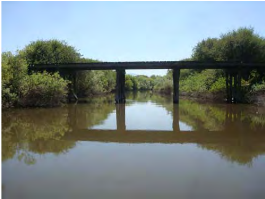
Photograph 64. View looking upstream at farm access road bridge crossing Catherine Creek near river mile 11.30. Reach 1 – Catherine Creek, Grande Ronde Subbasin, Oregon – Bureau of Reclamation Photograph by D. Stelma, July 9, 2010.
