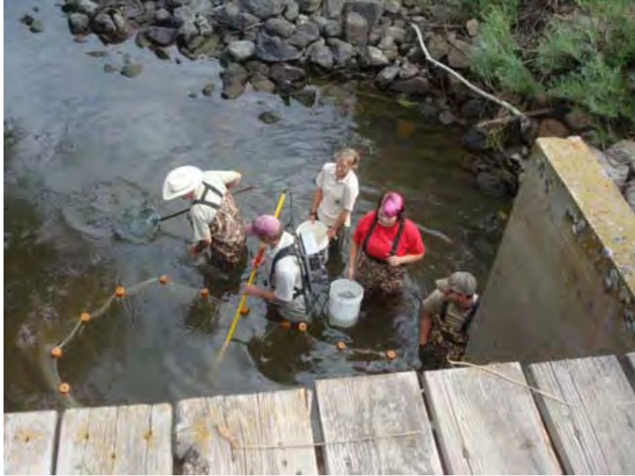
Photograph 37. View looking downstream from the crest of Davis Dam at ODFW biologist electro-shocking and capturing fish in tailrace during brief water shut-off for dam repair work near river mile 34.40. Reach 2 – Catherine Creek, Grande Ronde Subbasin, Oregon – Bureau of Reclamation Photograph by D. Stelma, July 27, 2010.
