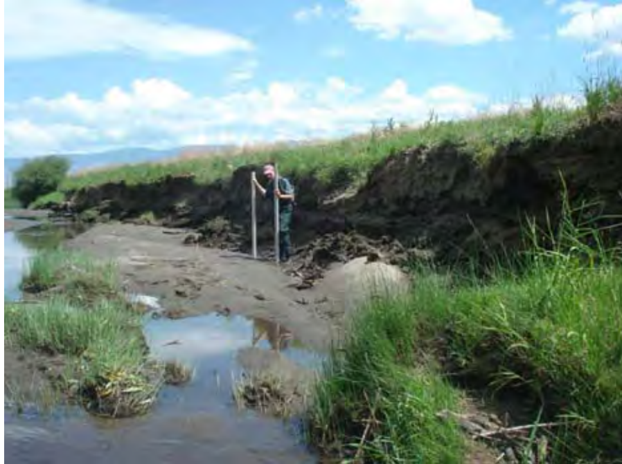
Photograph 71. View looking downstream along an eroding section of the right bank. The bank has about 6 feet of vertical face that is contributing sand, silt and clay sized material near river mile 33.65. Reach 2 – Catherine Creek, Grande Ronde Subbasin, Oregon – Bureau of Reclamation Photograph by R. McAfee, July 27, 2010.
