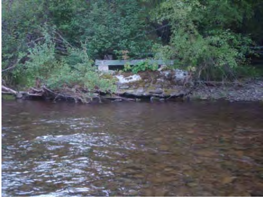
Photograph 56. Remnant of bridge abutment on the left bank of Catherine Creek near river mile 46.57. Reach 5 – Catherine Creek, Grande Ronde Subbasin, Oregon – Bureau of Reclamation Photograph by D. Stelma, August 18, 2010.
