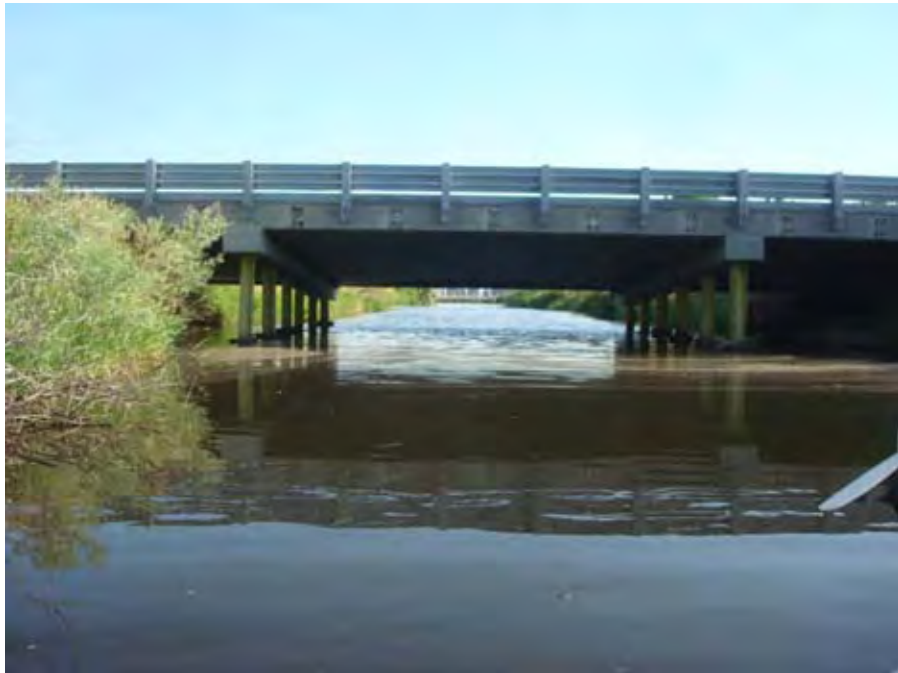
Photograph 22. View looking downstream at the Oregon State Highway 203 Bridge near river mile 35.30. Reach 2 – Catherine Creek, Grande Ronde Subbasin, Oregon – Bureau of Reclamation Photograph by D. Stelma, July 31, 2010.
