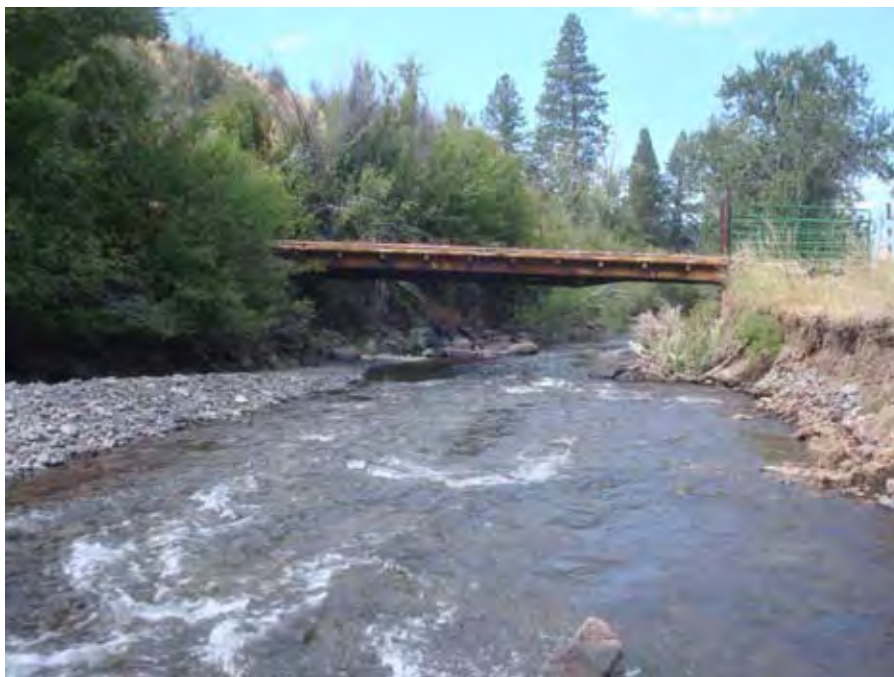
Photograph 1. View looking downstream at access bridge (rail road car frame) across Catherine Creek near river mile 45.65. Reach 4 – Catherine Creek, Grande Ronde Subbasin, Oregon – Bureau of Reclamation Photograph by D. Stelma, August 18, 2010.
