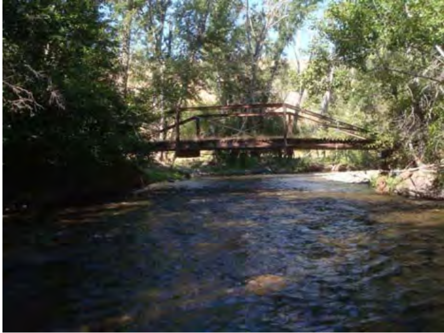
Photograph 40. View looking downstream at farm access bridge across Catherine Creek near river mile 42.25. Reach 4 – Catherine Creek, Grande Ronde Subbasin, Oregon – Bureau of Reclamation Photograph by D. Stelma, August 16, 2010.
