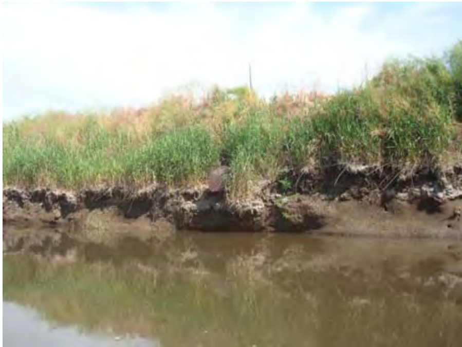
Photograph 46. View of CMP drain pipe with one-way flapper-valve on the right bank of Catherine Creek near river mile 14.06. Reach 1 – Catherine Creek, Grande Ronde Subbasin, Oregon – Bureau of Reclamation Photograph by D. Stelma, July 10, 2010.
