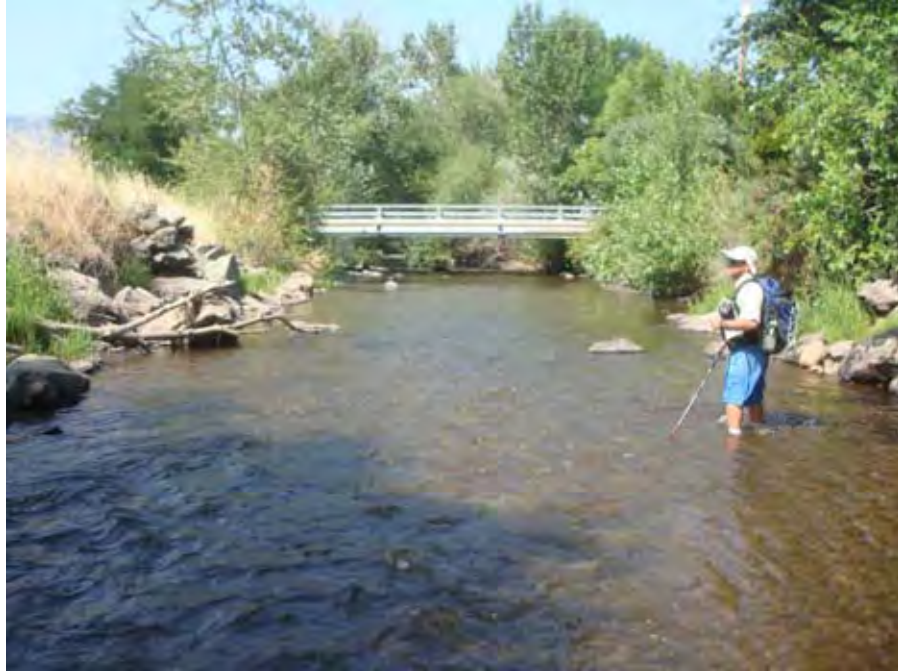
Photograph 19. View looking downstream at the North Bellwood Street Bridge over Catherine Creek in Union, OR near river mile 40.11. Reach 3 – Catherine Creek, Grande Ronde Subbasin, Oregon – Bureau of Reclamation Photograph by D. Stelma, August 2, 2010.
