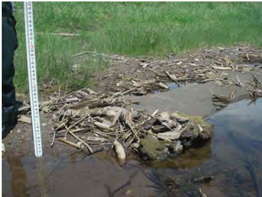
Photograph 68. View of an example of how small roughness elements can promote local deposition near river mile 33.78. Reach 2 – Catherine Creek, Grande Ronde Subbasin, Oregon – Bureau of Reclamation Photograph by R. McAfee, July 27, 2010.
