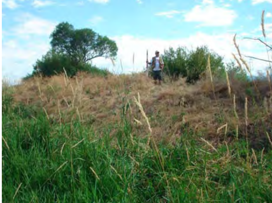
Photograph 47. A view to the northeast showing the backside of a levee placed along the left bank of Catherine Creek near river mile 34.26. Reach 2 – Catherine Creek, Grande Ronde Subbasin, Oregon – Bureau of Reclamation Photograph by R. McAfee, July 27, 2010.
