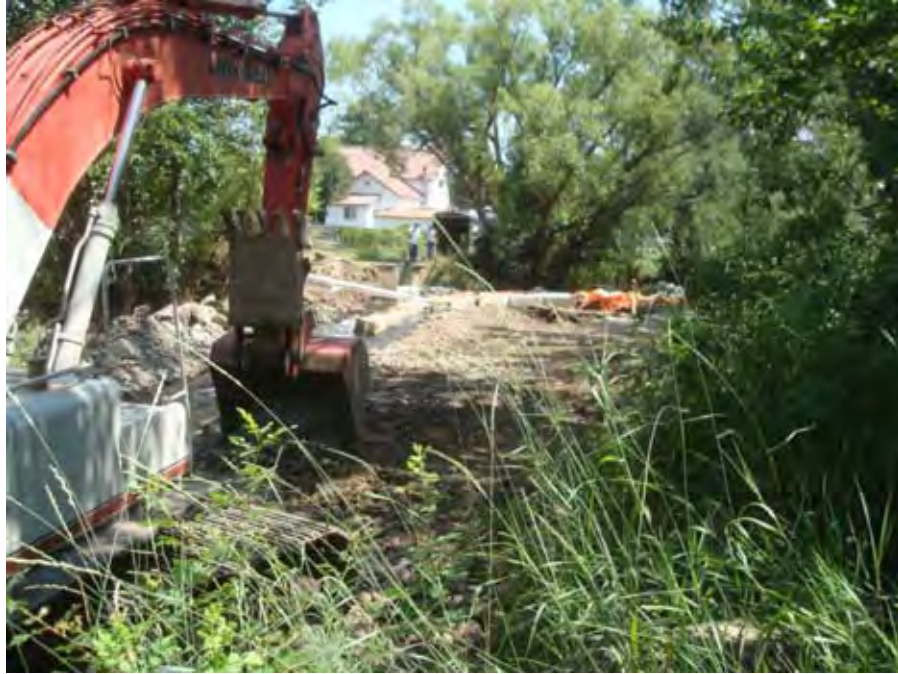
Photograph 27. View looking upstream at diversion dam work on Catherine Creek in Union, OR near river mile 39.84. Reach 3 – Catherine Creek, Grande Ronde Subbasin, Oregon – Bureau of Reclamation Photograph by D. Stelma, August 2, 2010.
