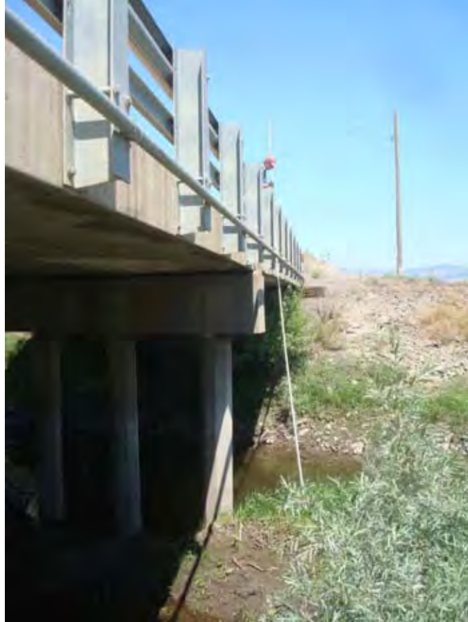
Photograph 231. View looking south at the downstream side of the Godley Lane Bridge near river mile 26.70. Reach 2 – Catherine Creek, Grande Ronde Subbasin, Oregon – Bureau of Reclamation Photograph by D. Stelma, July 29, 2010.
