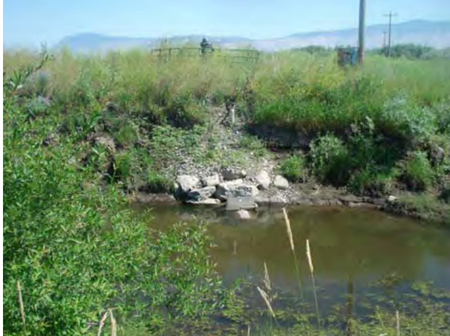
Photograph 224. View from the right bank to the left or a pump on top of the left bank with the 30-inch intake just below the water level at the toe of the left bank and riprap protection along the bank toe near river mile 27.30. Reach 2 – Catherine Creek, Grande Ronde Subbasin, Oregon – Bureau of Reclamation Photograph by R. McAfee, July 29, 2010.
