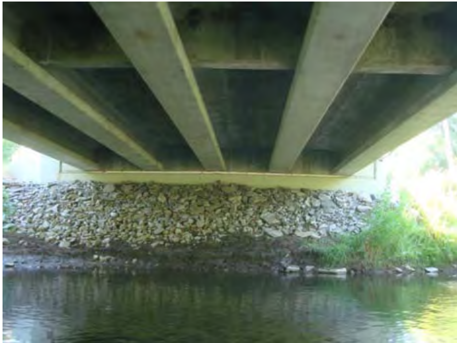
Photograph 12. Left abutment of Miller Lane Bridge near river mile 36.48. Reach 2 – Catherine Creek, Grande Ronde Subbasin, Oregon – Bureau of Reclamation Photograph by D. Stelma, July 31, 2010.
