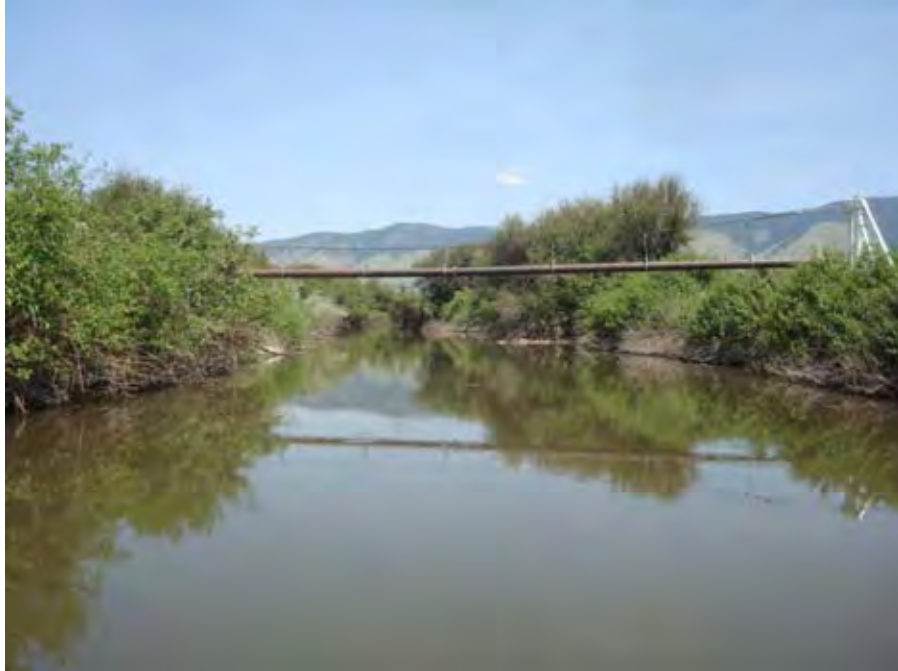
Photograph 12. View looking downstream at irrigation pipe crossing Catherine Creek near river mile 20.81. Reach 1 – Catherine Creek, Grande Ronde Subbasin, Oregon – Bureau of Reclamation Photograph by D. Stelma, July 11, 2010.
