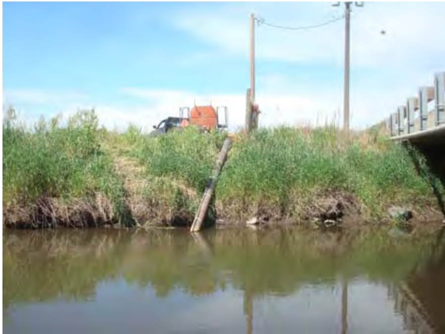
Photograph 39. Pumping plant on left (west) bank of Catherine Creek upstream of Booth Road bridge near river mile 15.30. Reach 1 – Catherine Creek, Grande Ronde Subbasin, Oregon – Bureau of Reclamation Photograph by D. Stelma, July 10, 2010.
