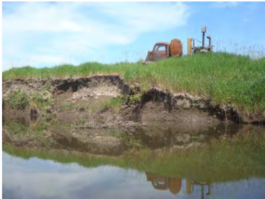
Photograph 25. View looking at erosion and truck-mounted pump (abandoned?) on left (west) bank of Catherine Creek near river mile 17.10. Reach 1 – Catherine Creek, Grande Ronde Subbasin, Oregon – Bureau of Reclamation Photograph by D. Stelma, July 10, 2010.
