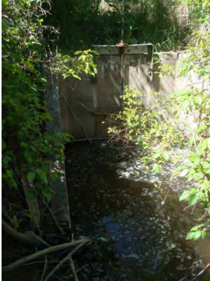
Photograph 65. View of diversion structure and slide-gate on the left bank of Catherine Creek at the rock push-up dam near river mile 40.80. Reach 4 – Catherine Creek, Grande Ronde Subbasin, Oregon – Bureau of Reclamation Photograph by D. Stelma, August 16, 2010.
