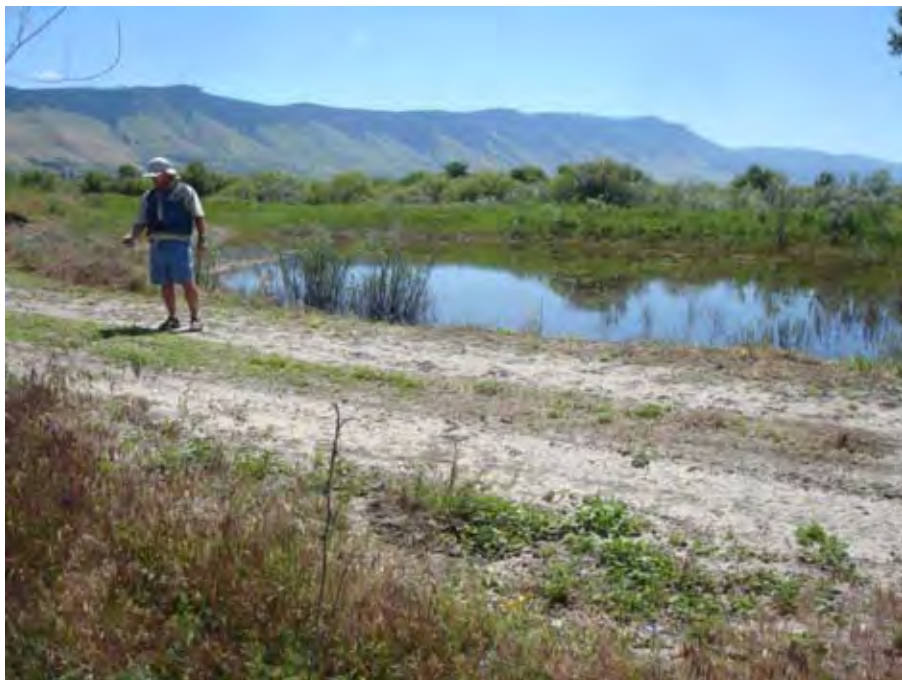
Photograph 97. View looking southeast the crest of a levee and standing water behind levee along the left bank of Catherine Creek near river mile 2.25. Reach 1 – Catherine Creek, Grande Ronde Subbasin, Oregon – Bureau of Reclamation Photograph by D. Stelma, July 7, 2010.
