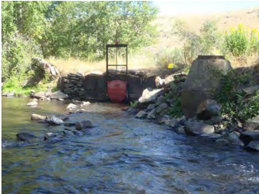
Photograph 29. View looking downstream at the fish trap holding pond intake structure and slide gate on the right bank of Catherine near river mile 42.54. Reach 4 – Catherine Creek, Grande Ronde Subbasin, Oregon – Bureau of Reclamation Photograph by D. Stelma, August 19, 2010.
