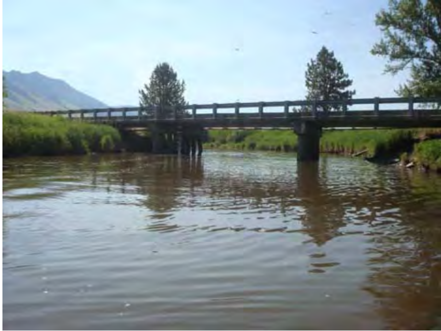
Photograph 38. View looking upstream at Booth Road Bridge near river mile 15.30. Reach 1 – Catherine Creek, Grande Ronde Subbasin, Oregon – Bureau of Reclamation Photograph by D. Stelma, July 10, 2010.
