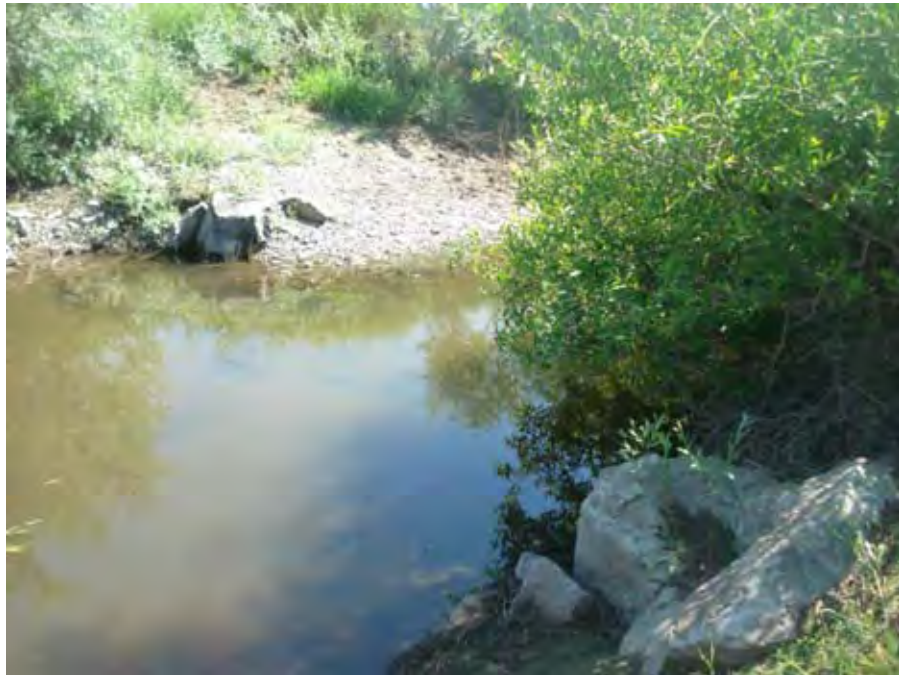
Photograph 221. View from the right bank of riprap hardened points along both banks at river mile 27.72. Reach 2 – Catherine Creek, Grande Ronde Subbasin, Oregon – Bureau of Reclamation Photograph by R. McAfee, July 29, 2010.
