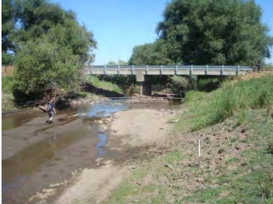
Photograph 119. View looking downstream at the Wilkinson Lane Bridge near river mile 32.00. Reach 2 – Catherine Creek, Grande Ronde Subbasin, Oregon – Bureau of Reclamation Photograph by D. Stelma, August 1, 2010.
