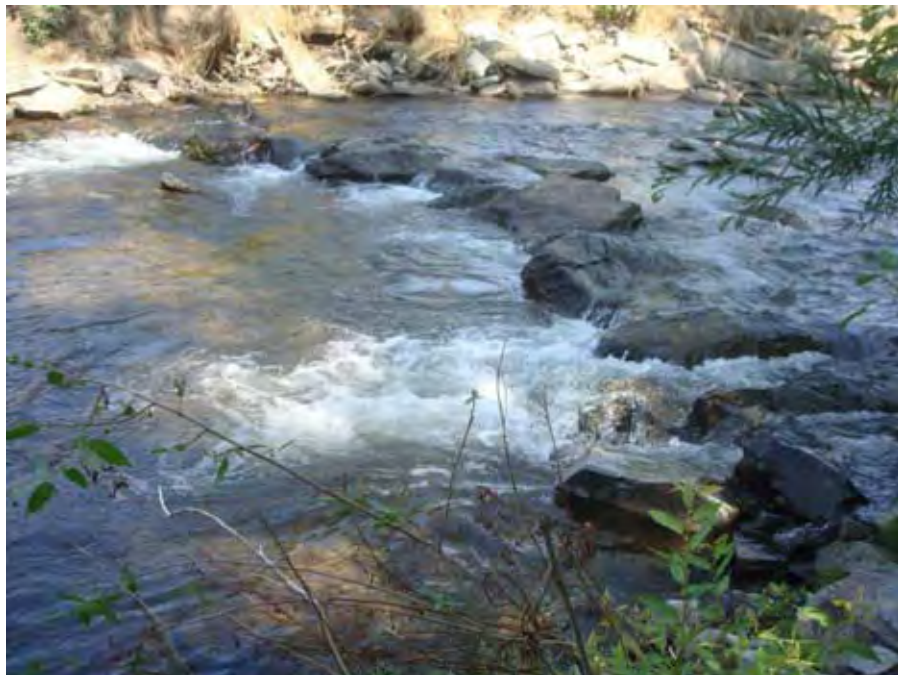
Photograph 16. View looking from left to right across the Catherine Creek in Union, OR at a rock weir (energy dissipater) structure near river mile 40.27. Reach 3 – Catherine Creek, Grande Ronde Subbasin, Oregon – Bureau of Reclamation Photograph by D. Stelma, August 2, 2010.
