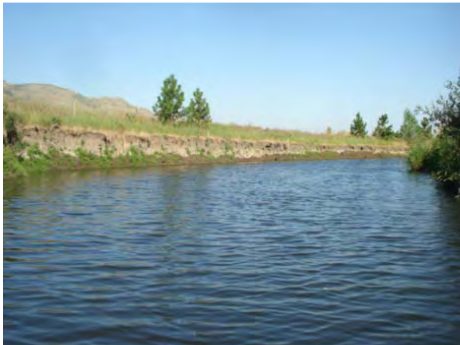
Photograph 14. View looking downstream at a section of the left bank that is nearly vertical near river mile 36.25. Note the predominantly grass vegetation. Reach 2 – Catherine Creek, Grande Ronde Subbasin, Oregon – Bureau of Reclamation Photograph by R. McAfee, July 31, 2010.
