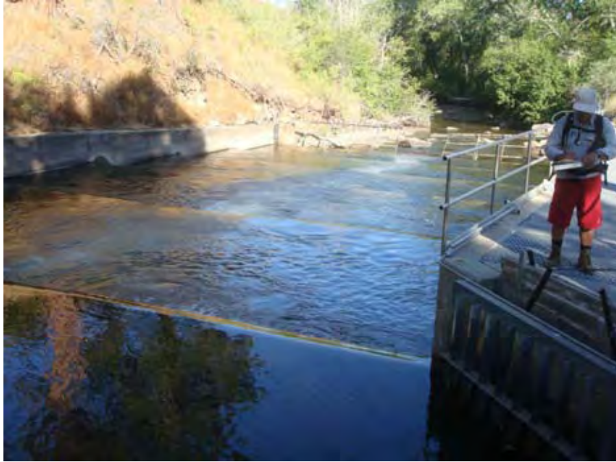
Photograph 30. View looking downstream at the fish trap structure and Catherine Creek channel near river mile 42.50. Reach 4 – Catherine Creek, Grande Ronde Subbasin, Oregon – Bureau of Reclamation Photograph by D. Stelma, August 16, 2010.
