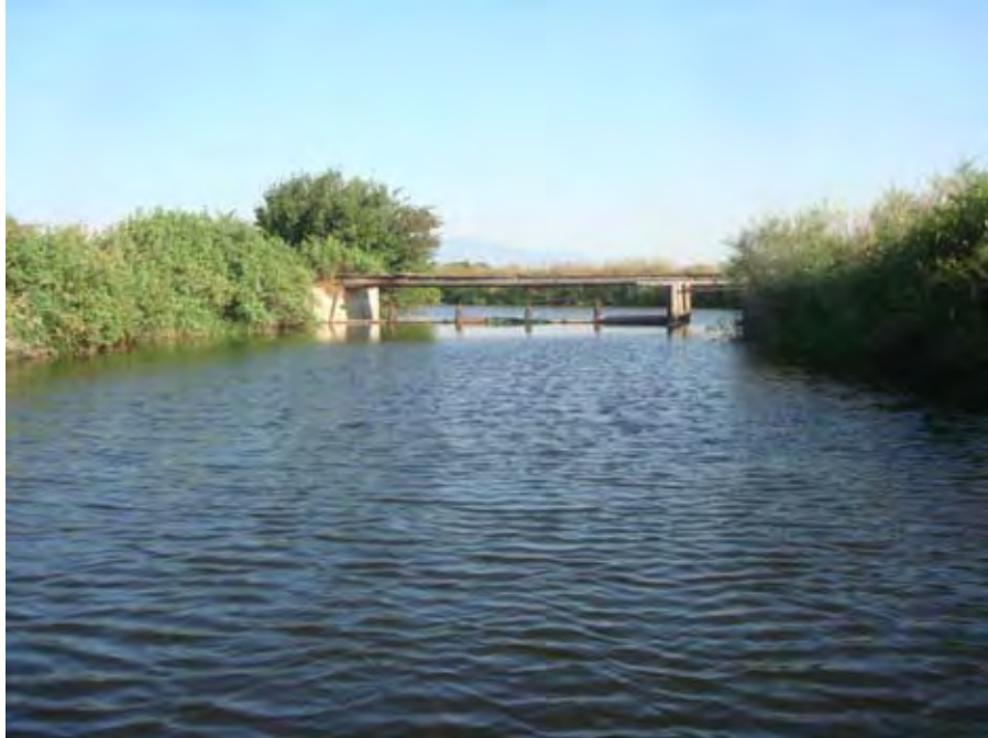
Photograph 25. View looking downstream at the upstream side of Upper Davis Dam, note (lower) Davis Dam tail water in background near river mile 34.99. Reach 2 – Catherine Creek, Grande Ronde Subbasin, Oregon – Bureau of Reclamation Photograph by D. Stelma, July 31, 2010.
