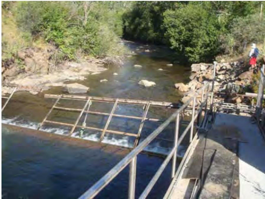
Photograph 31. View looking downstream at the fish trap structure and Catherine Creek channel near river mile 42.50. Reach 4 – Catherine Creek, Grande Ronde Subbasin, Oregon – Bureau of Reclamation Photograph by D. Stelma, August 16, 2010.
