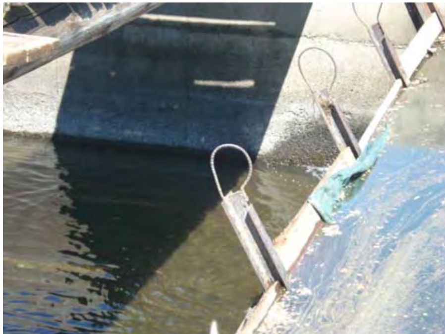
Photograph 28. View from the left bank of the checked-up water level upstream of Upper Davis Dam near river mile 34.98. Reach 2 – Catherine Creek, Grande Ronde Subbasin, Oregon – Bureau of Reclamation Photograph by R. McAfee, July 27, 2010.
