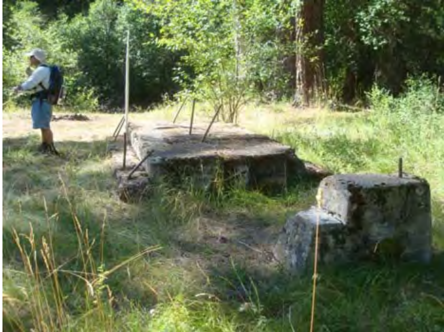
Photograph 8. Concrete footings and foundations on upper right bank of Catherine Creek, upstream from Catherine Creek State Park near river mile 49.50. Reach 5 – Catherine Creek, Grande Ronde Subbasin, Oregon – Bureau of Reclamation Photograph by D. Stelma, August 17, 2010.
