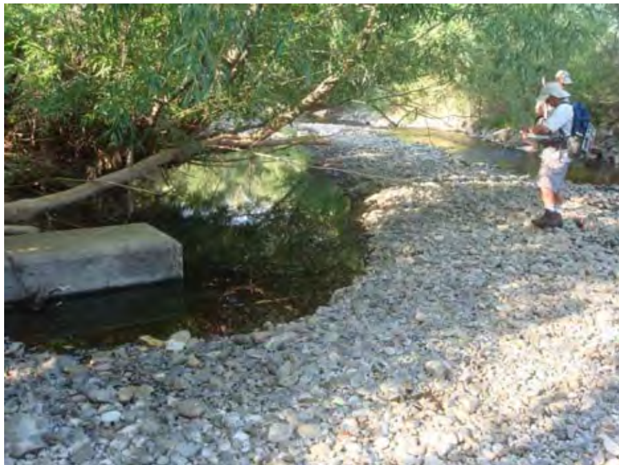
Photograph 42. View looking downstream at the Catherine Creek channel near the waste water treatment plant near river mile 39.00, note concrete encased discharge pipe entering the channel from the left. Reach 3 – Catherine Creek, Grande Ronde Subbasin, Oregon – Bureau of Reclamation Photograph by D. Stelma, August 3, 2010.
