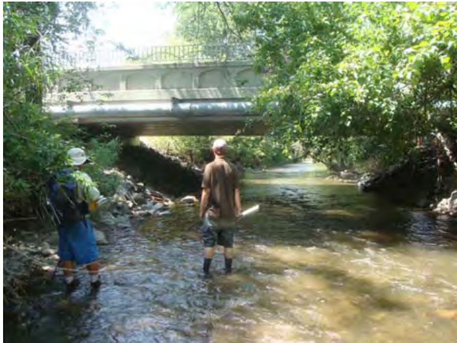
Photograph 28. View looking downstream at the North 5 th Street Bridge over Catherine Creek in Union, OR near river mile 39.72. Reach 3 – Catherine Creek, Grande Ronde Subbasin, Oregon – Bureau of Reclamation Photograph by D. Stelma, August 2, 2010.
