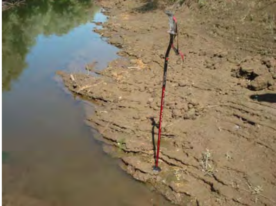
Photograph 222. View from the right bank looking downstream at another exposure of thinly bedded clayey-silty sand material near river mile 27.59. The vertical and/or undercut ledge just beneath the water surface is up to 2 feet tall. Reach 2 – Catherine Creek, Grande Ronde Subbasin, Oregon – Bureau of Reclamation Photograph by R. McAfee, July 29, 2010.
