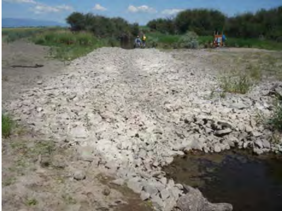
Photograph 4. View looking downstream at the dam and spillway channel, the (former) Grande Ronde River is in the lower right corner of photo, Catherine Creek is at top center of photo near river mile 22.50. Reach 1 – Catherine Creek, Grande Ronde Subbasin, Oregon – Bureau of Reclamation Photograph by D. Stelma, July 11, 2010.
