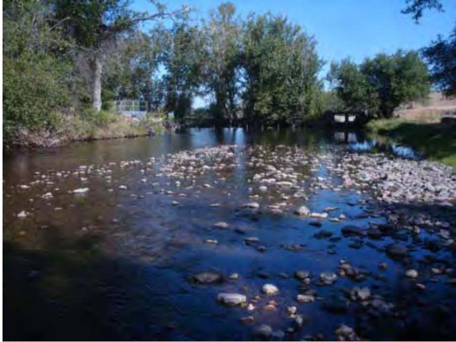
Photograph 57. View looking downstream at concrete diversion dam on Catherine Creek near river mile 41.19, structure diverts water north to Little Creek. Reach 4 – Catherine Creek, Grande Ronde Subbasin, Oregon – Bureau of Reclamation Photograph by D. Stelma, August 16, 2010.
