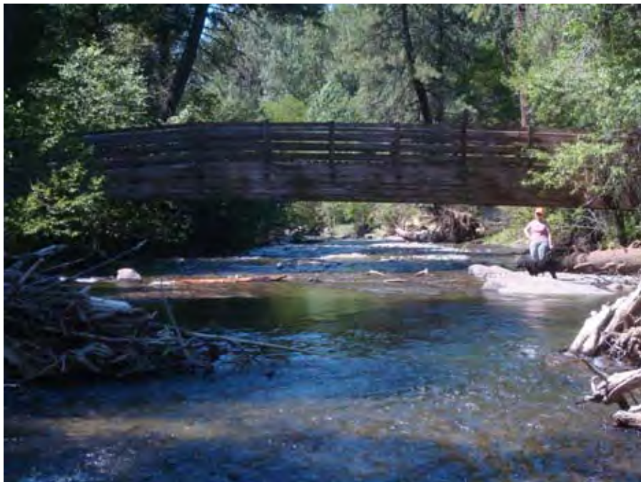
Photograph 21. View looking downstream at Catherine Creek within Catherine Creek State Park near river mile 48.63. Reach 5 – Catherine Creek, Grande Ronde Subbasin, Oregon – Bureau of Reclamation Photograph by D. Stelma, August 17, 2010.
