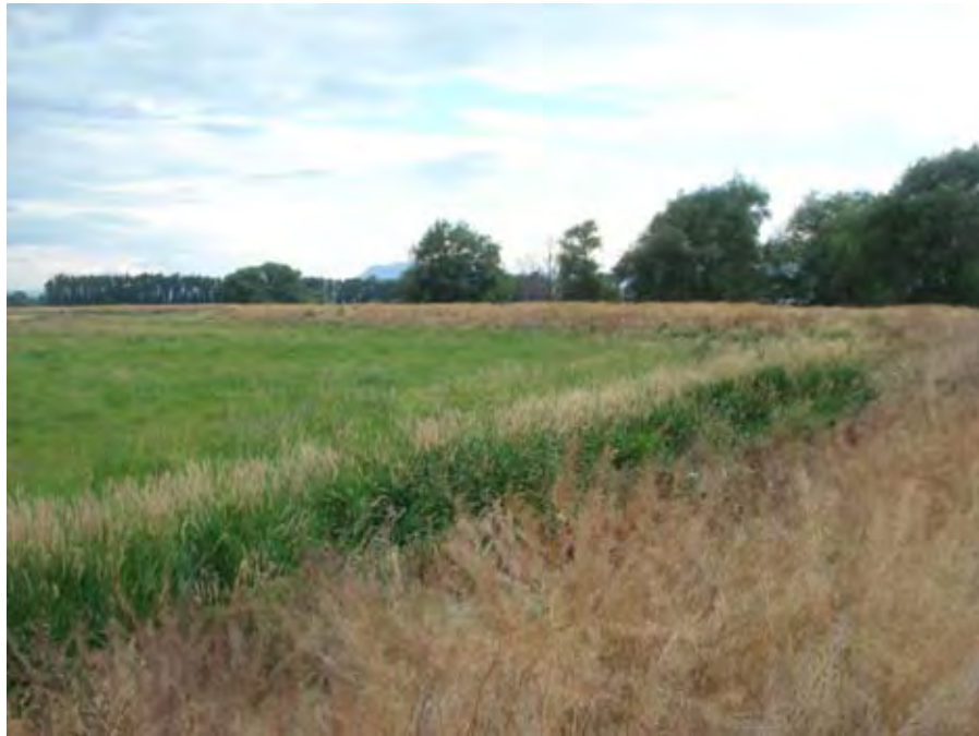
Photograph 76. A view looking to the north of the back side of a levee that runs along the left bank near river mile 33.59. Reach 2 – Catherine Creek, Grande Ronde Subbasin, Oregon – Bureau of Reclamation Photograph by R. McAfee, July 27, 2010.
