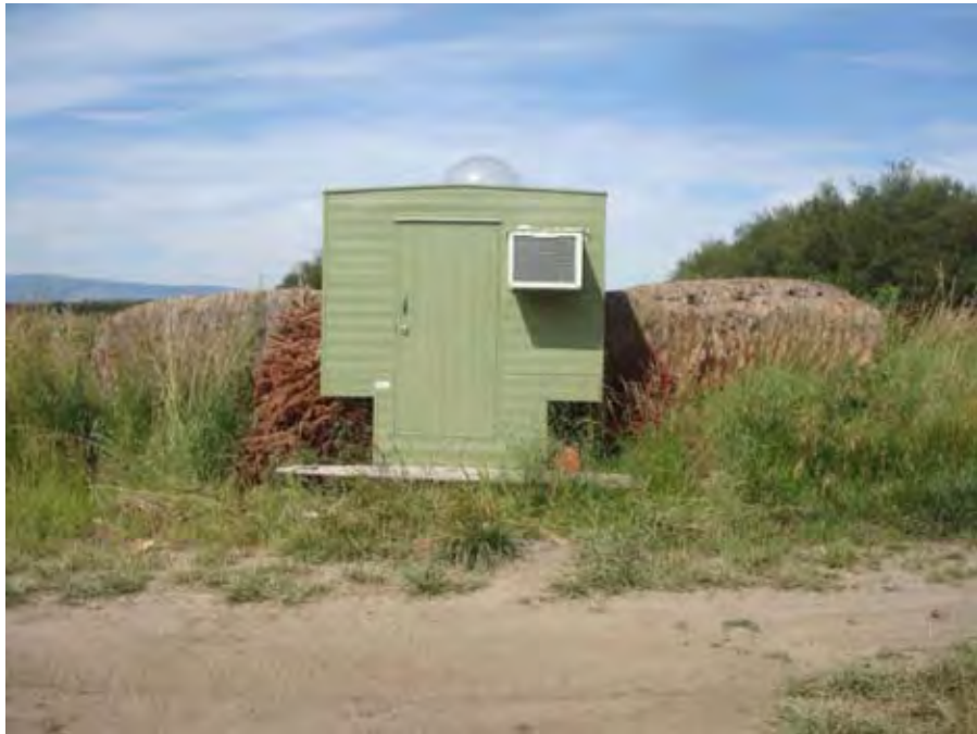
Photograph 52. Pump house on west side of Catherine Creek near river mile 13.62. Reach 1 – Catherine Creek, Grande Ronde Subbasin, Oregon – Bureau of Reclamation Photograph by D. Stelma, July 10, 2010.
