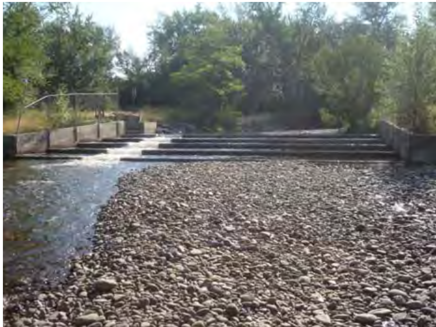
Photograph 4. View looking upstream at Schwackhammer diversion dam near river mile 40.60. Reach 3 – Catherine Creek, Grande Ronde Subbasin, Oregon – Bureau of Reclamation Photograph by D. Stelma, August 2, 2010.
