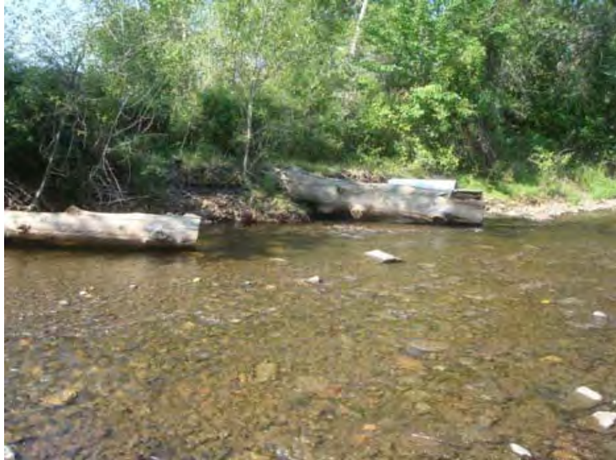
Photograph 9. View looking at log flow deflectors on the left bank of Catherine Creek in Union, OR near river mile 40.50. Reach 3 – Catherine Creek, Grande Ronde Subbasin, Oregon – Bureau of Reclamation Photograph by D. Stelma, August 2, 2010.
