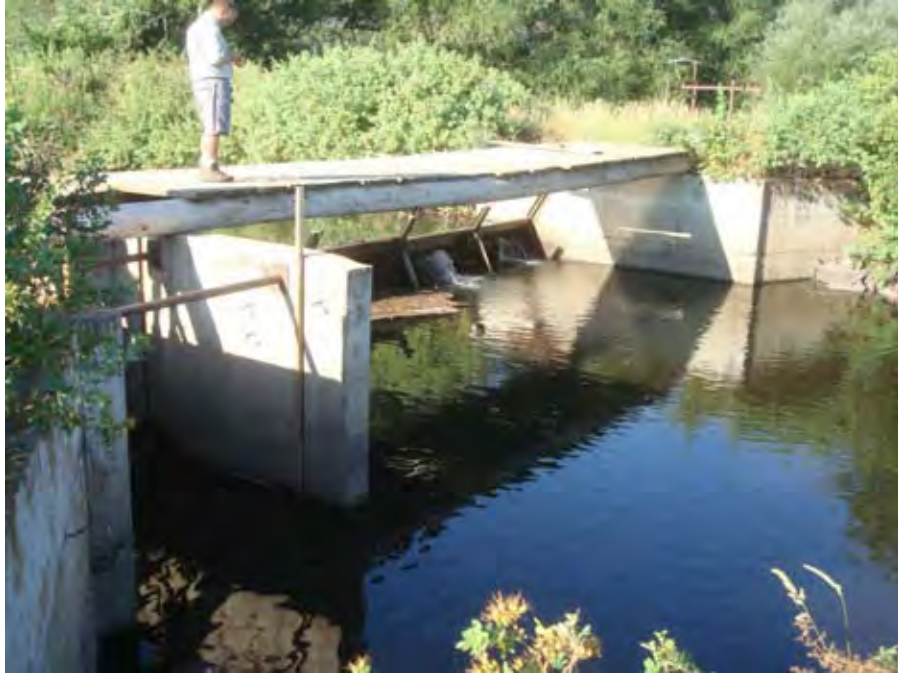
Photograph 29. View looking from right to left at the downstream side of Upper Davis Dam, note (lower) Davis Dam tail water level approximately 2- to 3-feet below gates near river mile 34.98. Reach 2 – Catherine Creek, Grande Ronde Subbasin, Oregon – Bureau of Reclamation Photograph by D. Stelma, August 1, 2010.
