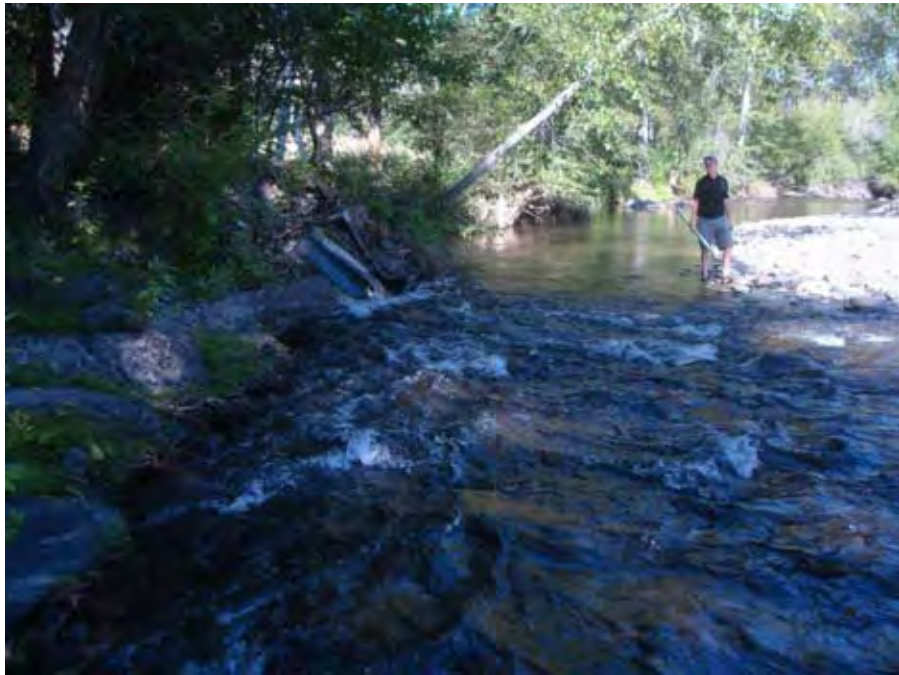
Photograph 41. View looking downstream at Catherine Creek channel near river mile 42.24, note concrete blocks and automobile for erosion protection on left side creek. Reach 4 – Catherine Creek, Grande Ronde Subbasin, Oregon – Bureau of Reclamation Photograph by D. Stelma, August 16, 2010.
