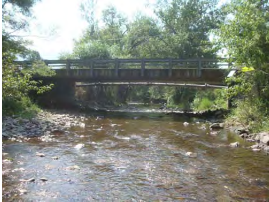
Photograph 35. View looking downstream at the North 10 th Street Bridge over Catherine Creek in Union, OR near river mile 39.46, note river flow gage station (with solar panel) near the right abutment of the bridge. Reach 3 – Catherine Creek, Grande Ronde Subbasin, Oregon – Bureau of Reclamation Photograph by D. Stelma, August 2, 2010.
