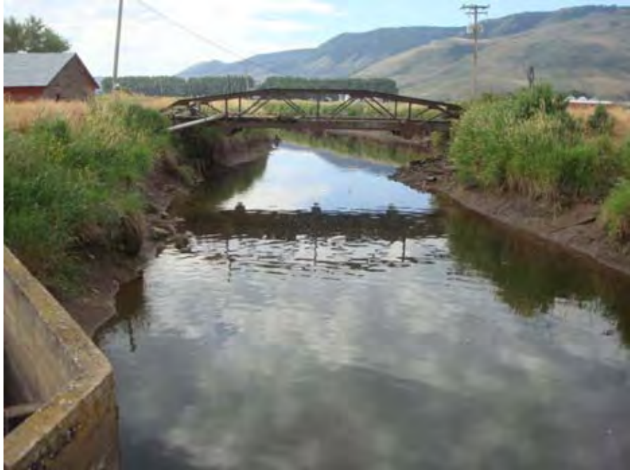
Photograph 39. View looking upstream from the crest of Davis Dam near river mile 34.40. Reach 2 – Catherine Creek, Grande Ronde Subbasin, Oregon– Bureau of Reclamation Photograph by D. Stelma, July 27, 2010.
