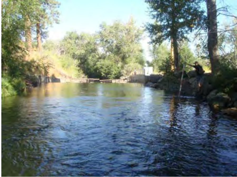
Photograph 32. View looking downstream at fish trap structure and Catherine Creek channel near river mile 42.50. Reach 4 – Catherine Creek, Grande Ronde Subbasin, Oregon – Bureau of Reclamation Photograph by D. Stelma, August 16, 2010.
