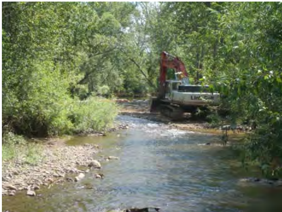
Photograph 26. View looking upstream at excavator being used to repair or modify small diversion dam on Catherine Creek in Union, OR near river mile 39.84. Reach 3 – Catherine Creek, Grande Ronde Subbasin, Oregon – Bureau of Reclamation Photograph by D. Stelma, August 2, 2010.
