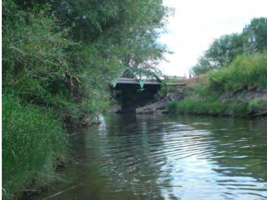
Photograph 61. View from left bank looking downstream at the Woodruff Lane Bridge near river mile 33.85. Reach 2 – Catherine Creek, Grande Ronde Subbasin, Oregon – Bureau of Reclamation Photograph by R. McAfee, July 27, 2010.
