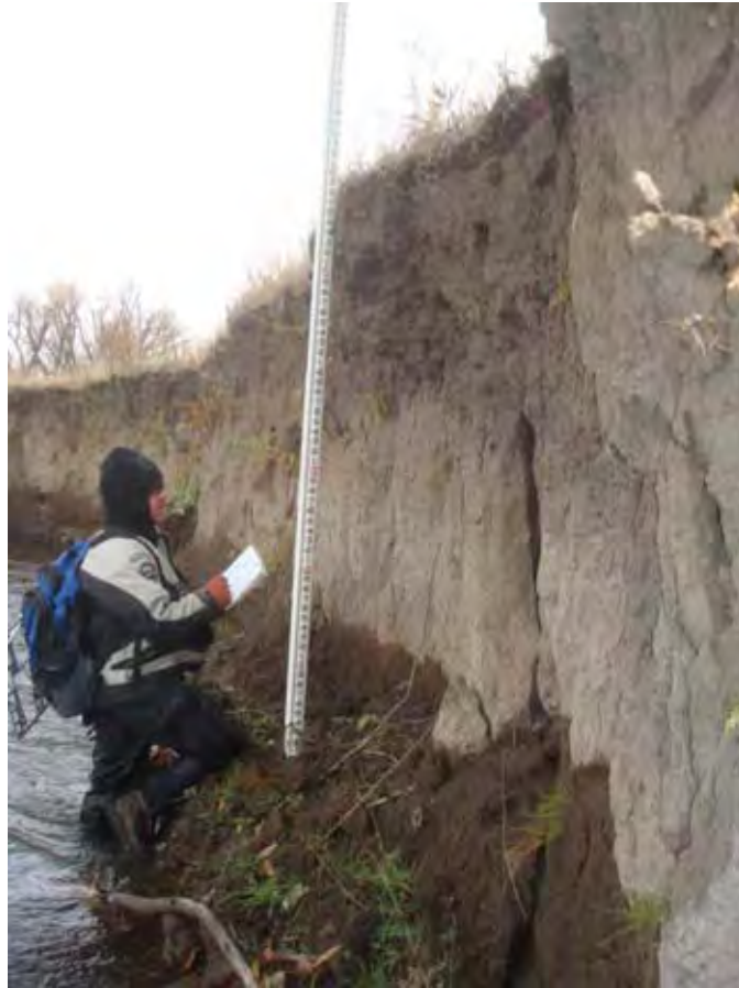
Photograph 1. View looking downstream over-steepened right bank of Catherine Creek, note vertical cracks in silt deposits near river mile 37.20. Reach 2 – Catherine Creek, Grande Ronde Subbasin, Oregon – Bureau of Reclamation Photograph by D. Stelma, November 10, 2010.
