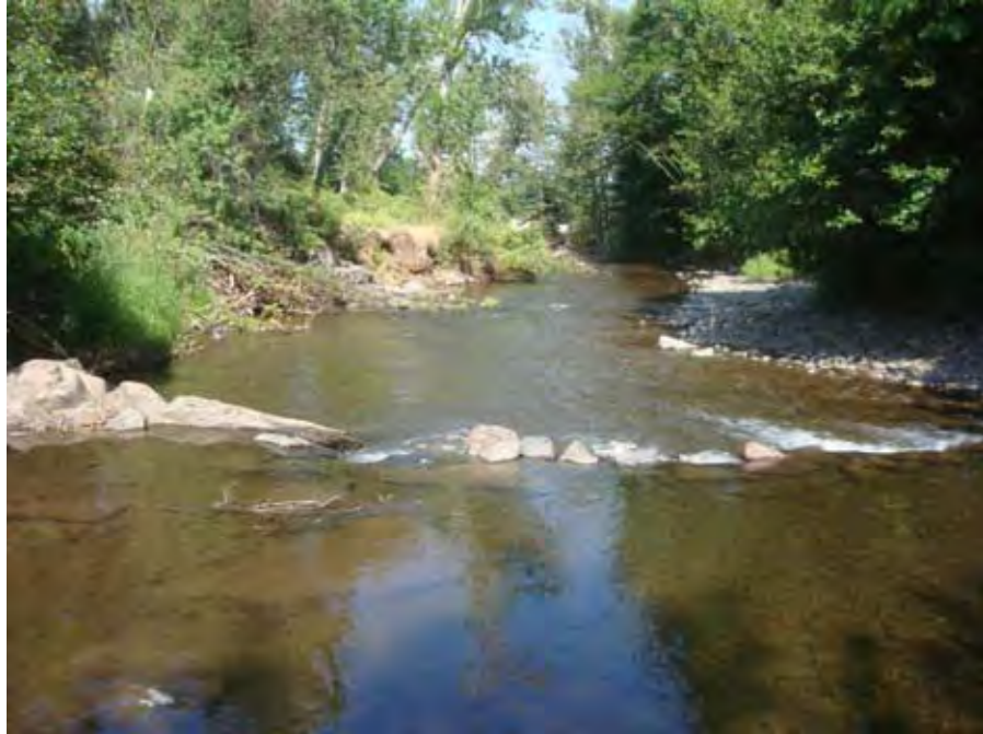
Photograph 12. View looking downstream at rock weir (energy dissipater) structure on Catherine Creek in Union, OR near river mile 40.33. Reach 3 – Catherine Creek, Grande Ronde Subbasin, Oregon – Bureau of Reclamation Photograph by D. Stelma, August 2, 2010.
