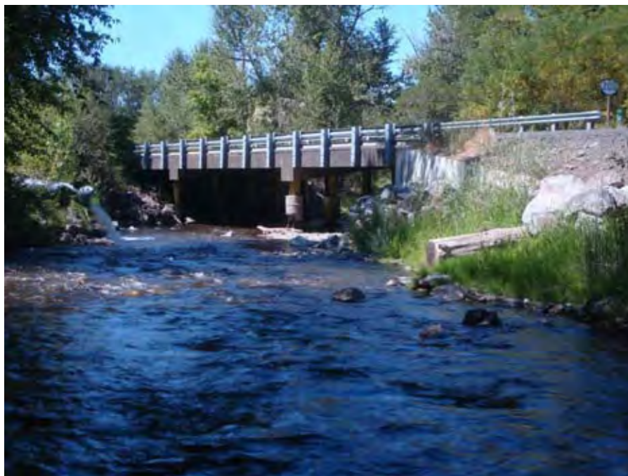
Photograph 1. View looking downstream at the Oregon State (Medical Springs) Highway 203 Bridge over Catherine Creek at Union, OR near river mile 40.65, note return flow from CMP on left side of channel. Reach 3 – Catherine Creek, Grande Ronde Subbasin, Oregon – Bureau of Reclamation Photograph by D. Stelma, August 16, 2010.
