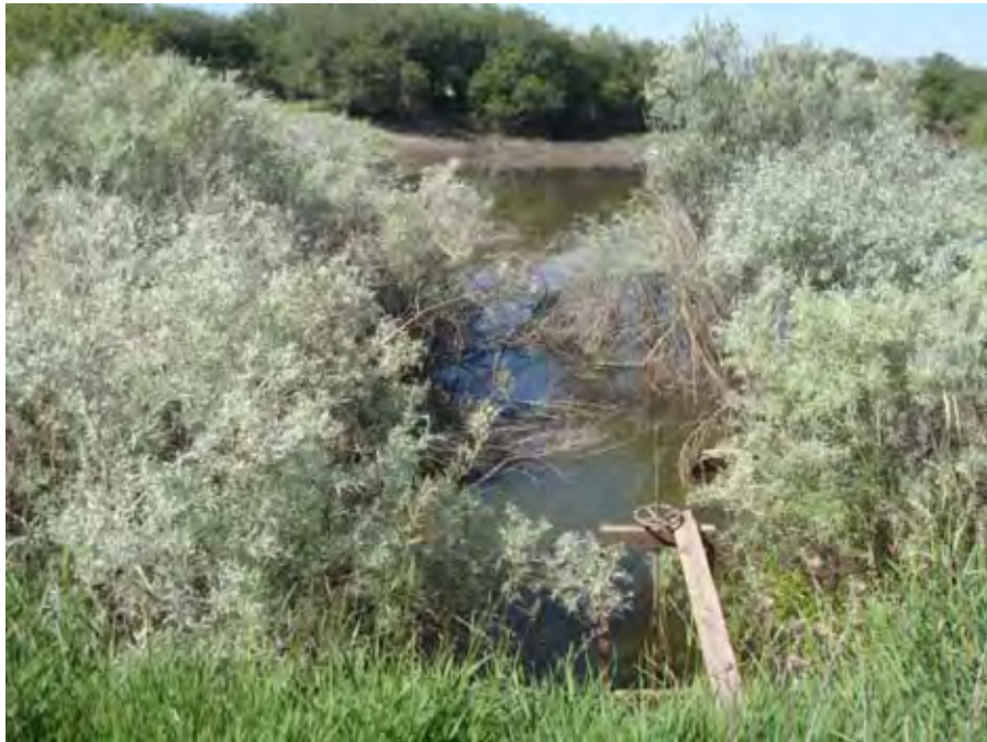
Photograph 77. View looking west at oxbow lake discharge headgate and Catherine Creek in background near river mile 7.80. Reach 1 – Catherine Creek, Grande Ronde Subbasin, Oregon – Bureau of Reclamation Photograph by D. Stelma, July 9, 2010.
