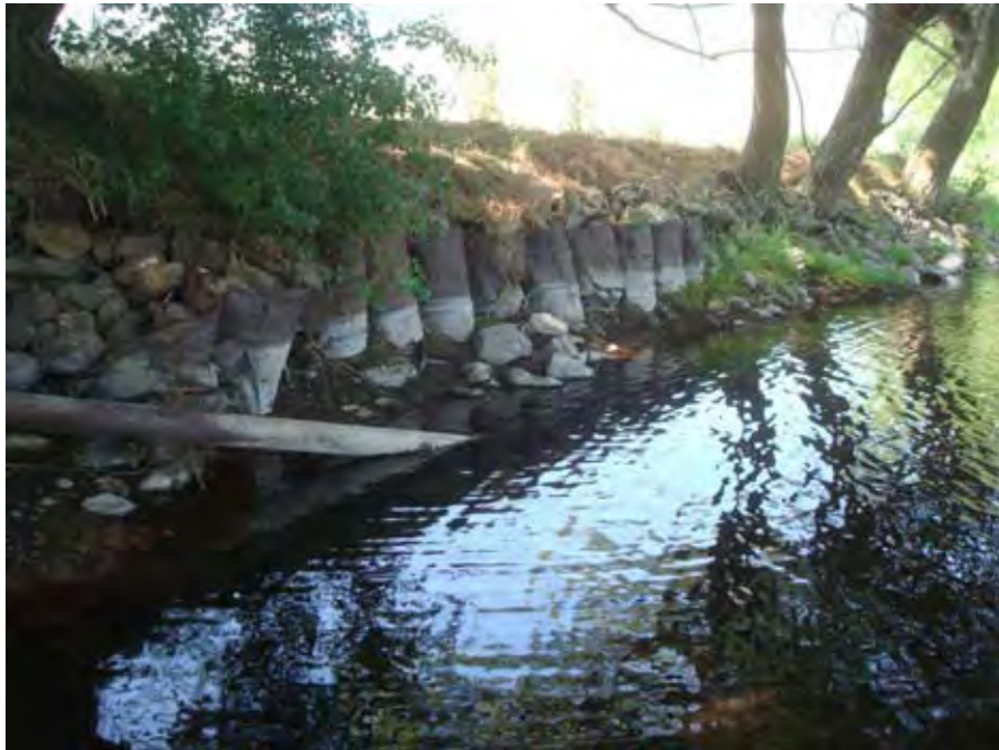
Photograph 61. Rock-filled drums used for erosion protection on the left bank of Catherine Creek near river mile 37.63. Reach 3 – Catherine Creek, Grande Ronde Subbasin, Oregon – Bureau of Reclamation Photograph by D. Stelma, August 3, 2010.
