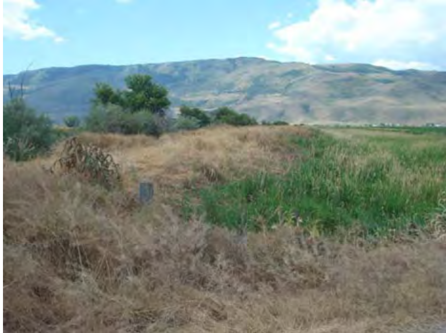
Photograph 63. View from Woodruff Lane looking down a levee along the right bank near river mile 33.84. Reach 2 – Catherine Creek, Grande Ronde Subbasin, Oregon – Bureau of Reclamation Photograph by R. McAfee, July 27, 2010.
