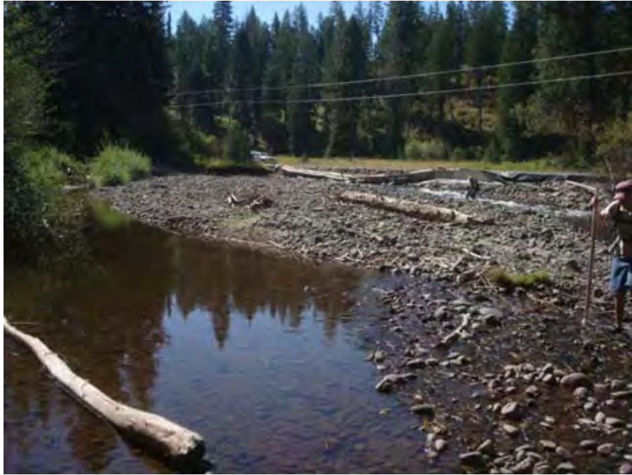
Photograph 1. View looking upstream at Catherine Creek channel near river mile 52.00, note failed concrete blocks along U.S.F.S. Road 7785 in background. Reach 6 – Catherine Creek, Grande Ronde Subbasin, Oregon – Bureau of Reclamation Photograph by D. Stelma, August 19, 2010.
