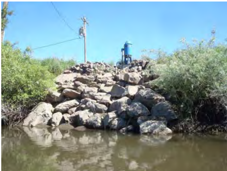
Photograph 107. View looking at pumping station on the right bank of Catherine Creek near river mile 0.40. Reach 1 – Catherine Creek, Grande Ronde Subbasin, Oregon – Bureau of Reclamation Photograph by D. Stelma, July 7, 2010.
