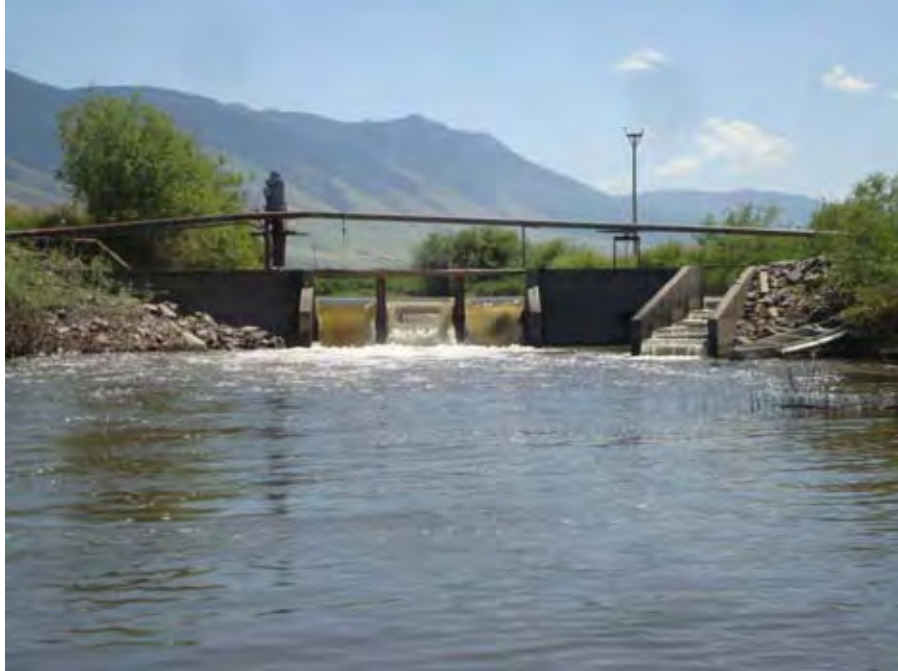
Photograph 55. View looking upstream at Elmer Dam near river mile 13.13. Reach 1 – Catherine Creek, Grande Ronde Subbasin, Oregon – Bureau of Reclamation Photograph by D. Stelma, July 9, 2010.
