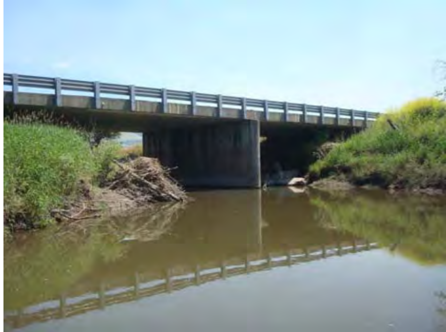
Photograph 10. View looking downstream at the Oregon State Highway 237 (Cove Highway) Bridge near river mile 21.29. Reach 1 – Catherine Creek, Grande Ronde Subbasin, Oregon – Bureau of Reclamation Photograph by D. Stelma, July 11, 2010.
