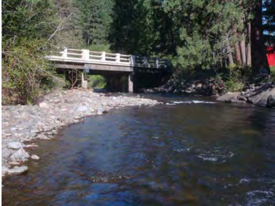
Photograph 3. View looking downstream at Catherine Creek channel and the Oregon State Highway (Medical Spring) 203 Bridge near river mile 49.90. Reach 5 – Catherine Creek, Grande Ronde Subbasin, Oregon – Bureau of Reclamation Photograph by D. Stelma, August 17, 2010.
