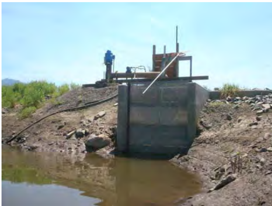
Photograph 2. View looking upstream at the dam and screened outlet/inlet at the mouth of the (former) Grande Ronde River, Catherine Creek in foreground near river mile 22.50. Reach 1 – Catherine Creek, Grande Ronde Subbasin, Oregon – Bureau of Reclamation Photograph by D. Stelma, July 11, 2010.
