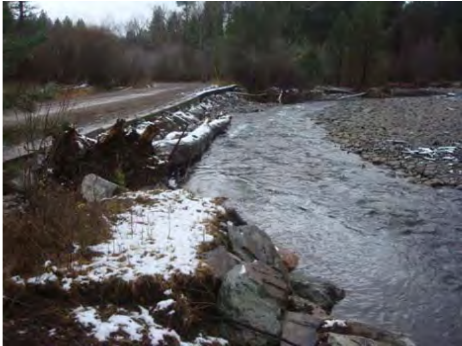
Photograph 3. View looking downstream at Catherine Creek channel near river mile 52.00, note repaired erosion protection (concrete blocks, rip rap and log) along U.S.F.S. Road 7785 in background. Reach 6 – Catherine Creek, Grande Ronde Subbasin, Oregon – Bureau of Reclamation Photograph by D. Stelma, November 10, 2010.
