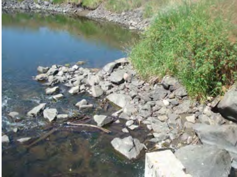
Photograph 31. View looking downstream from Upper Davis Dam at the riprap across the bottom of the channel and along the right bank near river mile 34.98. Reach 2 – Catherine Creek, Grande Ronde Subbasin, Oregon – Bureau of Reclamation Photograph by R. McAfee, July 27, 2010.
