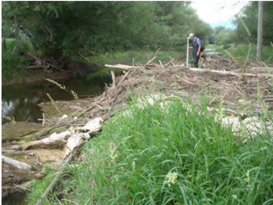
Photograph 175. View looking downstream at wood debris on upper right bank of Catherine Creek near river mile 30.40. Reach 2 – Catherine Creek, Grande Ronde Subbasin, Oregon – Bureau of Reclamation Photograph by D. Stelma, July 28, 2010.
