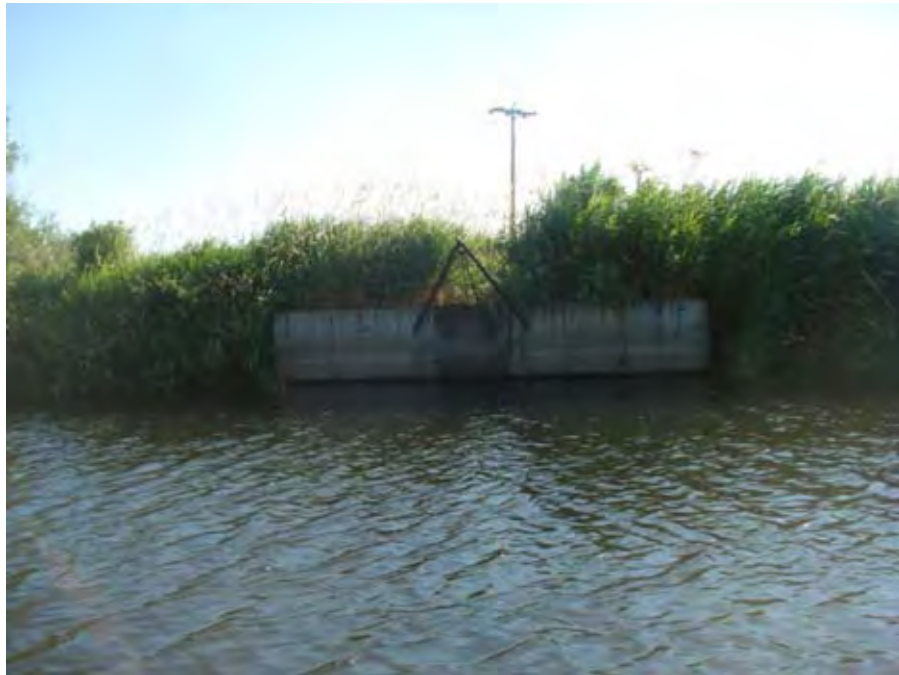
Photograph 24. View of a diversion headgate along the right bank of Catherine Creek near river mile 35.02, upstream of Upper Davis Dam. Reach 2 – Catherine Creek, Grande Ronde Subbasin, Oregon – Bureau of Reclamation Photograph by R. McAfee, July 31, 2010.
