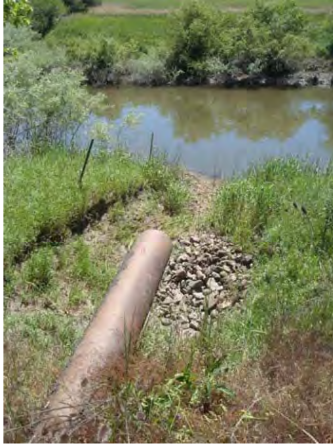
Photograph 87. View of meander pond discharge pipe and rock erosion protection with Catherine Creek in background near river mile 5.70. Reach 1 – Catherine Creek, Grande Ronde Subbasin, Oregon – Bureau of Reclamation Photograph by D. Stelma, July 7, 2010.
