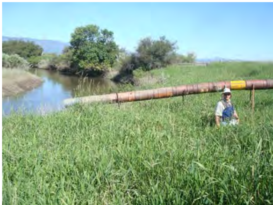
Photograph 105. View looking downstream at fabricated-barrel discharge pipe used to drain water from behind a levee along the right bank of Catherine Creek near river mile 0.47. Reach 1 – Catherine Creek, Grande Ronde Subbasin, Oregon – Bureau of Reclamation Photograph by D. Stelma, July 7, 2010.
