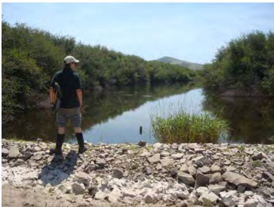
Photograph 3. View from the crest of the embankment dam looking upstream at the (former) Grande Ronde River near river mile 22.50. Reach 1 – Catherine Creek, Grande Ronde Subbasin, Oregon – Bureau of Reclamation Photograph by D. Stelma, July 11, 2010.
