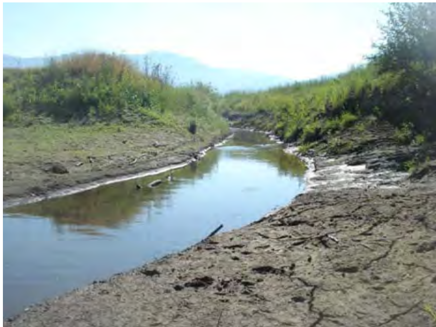
Photograph 250. View right bank looking up into Mill Creek near river mile 24.11. Note the amount of apparent incision on Mill Creek. Catherine Creek reflects the same amount of incision. Reach 2 – Catherine Creek, Grande Ronde Subbasin, Oregon – Bureau of Reclamation Photograph by R. McAfee, July 30, 2010.
