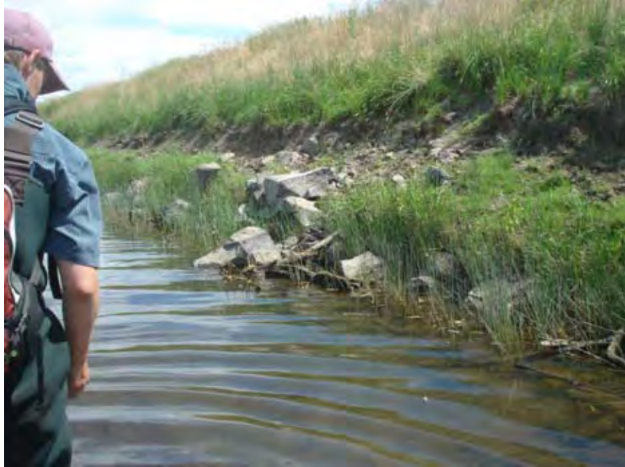
Photograph 67. View looking downstream at a small section of riprap along the right bank near river mile 33.78. Reach 2 – Catherine Creek, Grande Ronde Subbasin, Oregon – Bureau of Reclamation Photograph by R. McAfee, July 27, 2010.
