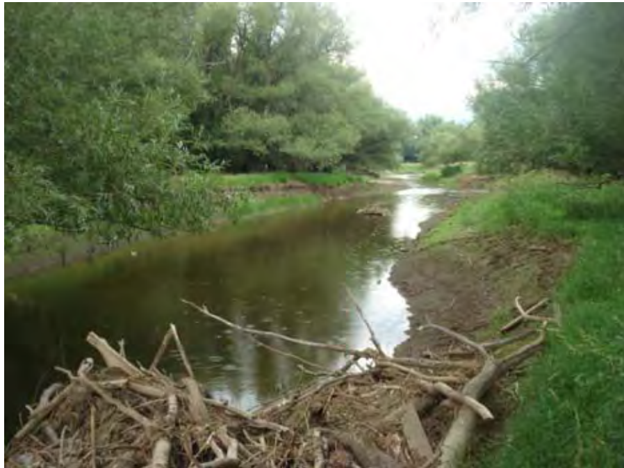
Photograph 171. View from the right bank looking downstream at mostly denuded banks and a debris accumulation along the right bank near river mile 30.43. Reach 2 – Catherine Creek, Grande Ronde Subbasin, Oregon – Bureau of Reclamation Photograph by R. McAfee, July 28, 2010.
