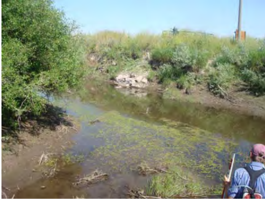
Photograph 220. Views looking north at side drainage channel discharge, and pumps on north side of Catherine Creek near river mile 27.72. Reach 2 – Catherine Creek, Grande Ronde Subbasin, Oregon – Bureau of Reclamation Photograph by D. Stelma, July 29, 2010.
