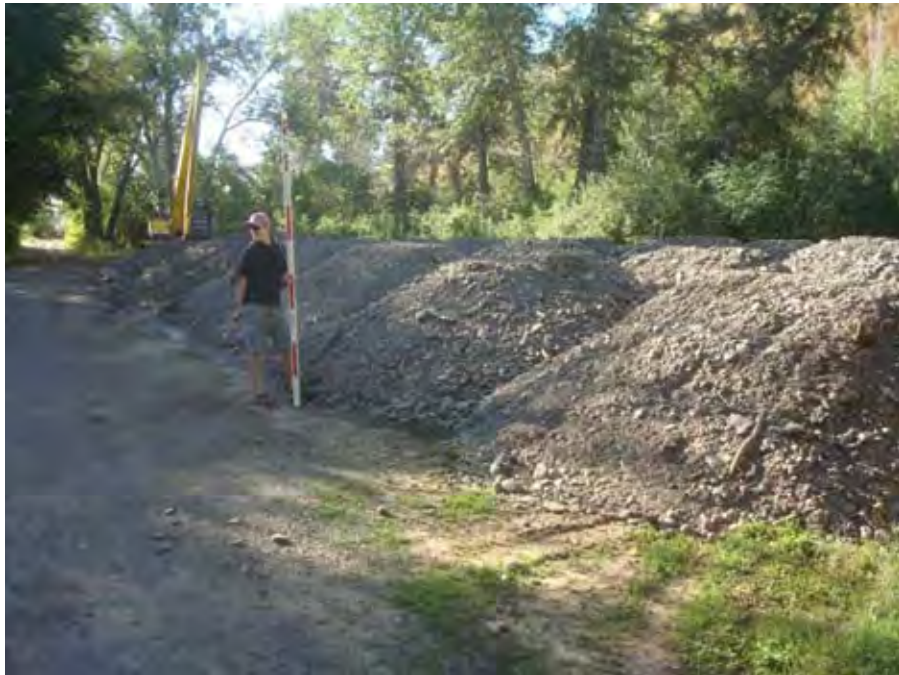
Photograph 33. Sediment excavated from the bed of Catherine Creek upstream and within the concrete fish trap structure, stockpiled on right bank downstream of the fish trap near river mile 42.49. Reach 4 – Catherine Creek, Grande Ronde Subbasin, Oregon – Bureau of Reclamation Photograph by D. Stelma, August 16, 2010.
