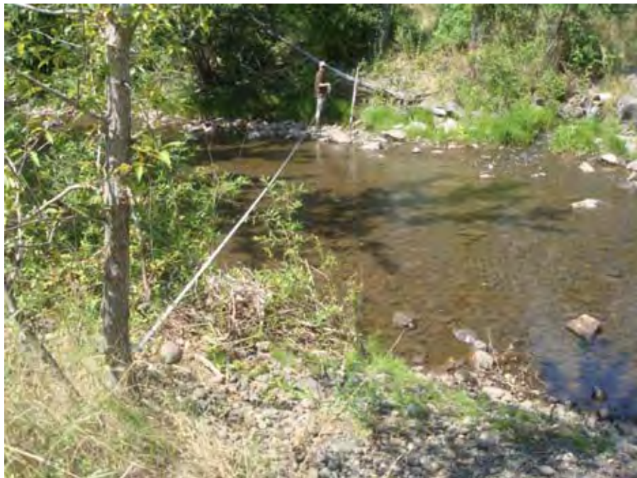
Photograph 34. View looking from left to right across Catherine Creek at profile location immediately downstream from concrete diversion dam near river mile 39.60. Reach 3 – Catherine Creek, Grande Ronde Subbasin, Oregon – Bureau of Reclamation Photograph by D. Stelma, August 2, 2010.
