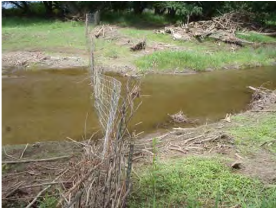
Photograph 191. View looking from right to left at fence across Catherine Creek near river mile 30.00. Reach 2 – Catherine Creek, Grande Ronde Subbasin, Oregon – Bureau of Reclamation Photograph by D. Stelma, July 28, 2010.
