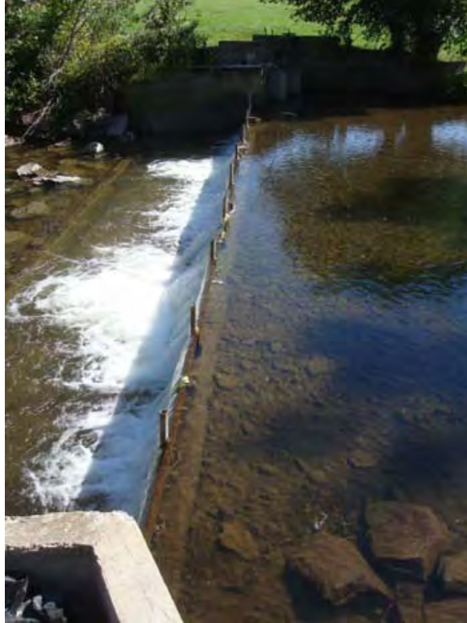
Photograph 60. View looking from the right abutment toward the left abutment at concrete diversion dam on Catherine Creek, irrigation diversion intake structure in background (left side) near river mile 41.19. Reach 4 – Catherine Creek, Grande Ronde Subbasin, Oregon – Bureau of Reclamation Photograph by D. Stelma, August 16, 2010.
