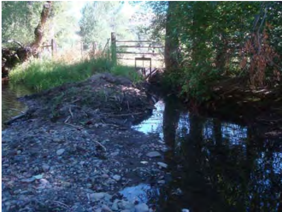
Photograph 23. View looking toward left bank (north) at small push-up diversion dam and head gate structure near river mile 42.80. Reach 4 – Catherine Creek, Grande Ronde Subbasin, Oregon – Bureau of Reclamation Photograph by D. Stelma, August 19, 2010.
