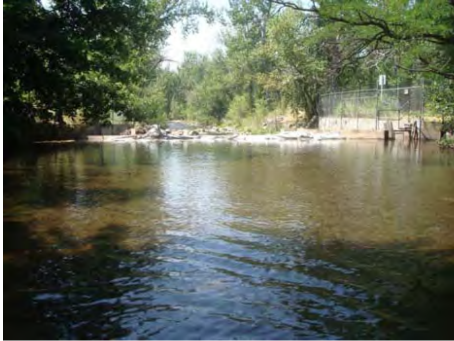
Photograph 31. View looking downstream at the Catherine Creek channel and concrete diversion dam within the city of Union, OR near river mile 39.63, note ditch/canal intake on the upstream right side of the structure. Reach 3 – Catherine Creek, Grande Ronde Subbasin, Oregon – Bureau of Reclamation Photograph by D. Stelma, August 2, 2010.
