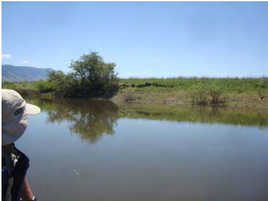
Photograph 95. View of slumping fine-grained alluvial soil (Qal2) on the outer side a meander on the left bank of Catherine Creek near river mile 3.15. Reach 1 – Catherine Creek, Grande Ronde Subbasin, Oregon – Bureau of Reclamation Photograph by D. Stelma, July 7, 2010.
