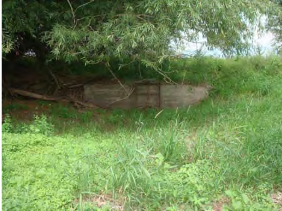
Photograph 152. View looking at drain slide-gate on the left bank of Catherine Creek near river mile 31.18. Reach 2 – Catherine Creek, Grande Ronde Subbasin, Oregon – Bureau of Reclamation Photograph by D. Stelma, July 28, 2010.
