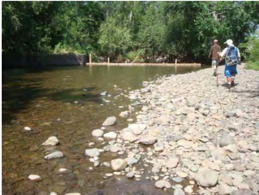
Photograph 22. View looking downstream at diversion dam on Catherine Creek in Union, OR near river mile 39.98. Reach 3 – Catherine Creek, Grande Ronde Subbasin, Oregon – Bureau of Reclamation Photograph by D. Stelma, August 2, 2010.
