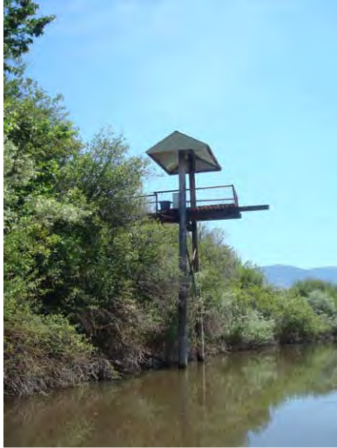
Photograph 56. View looking upstream at observation deck on east bank of Catherine Creek downstream of Elmer Dam near river mile 13.13. Reach 1 – Catherine Creek, Grande Ronde Subbasin, Oregon – Bureau of Reclamation Photograph by D. Stelma, July 9, 2010.
