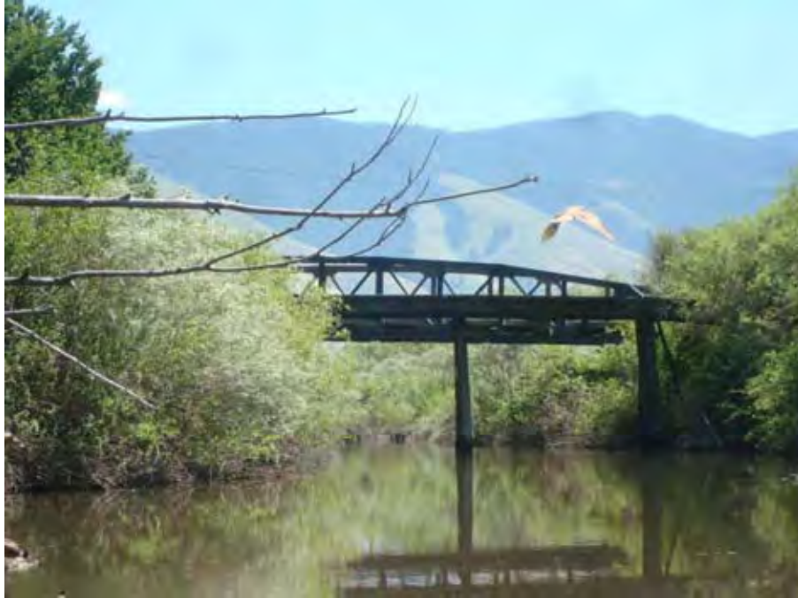
Photograph 57. View looking upstream at farm access road bridge across Catherin Creek downstream of Elmer Dam near river mile 12.95. Reach 1 – Catherine Creek, Grande Ronde Subbasin, Oregon – Bureau of Reclamation Photograph by D. Stelma, July 9, 2010.
