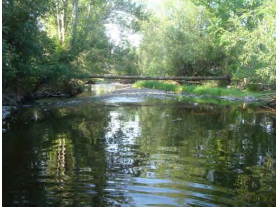
Photograph 45. View looking downstream at Catherine Creek channel near river mile 38.77, note pipeline crossing from the waste water treatment plant in background. Reach 3 – Catherine Creek, Grande Ronde Subbasin, Oregon – Bureau of Reclamation Photograph by D. Stelma, August 3, 2010.
