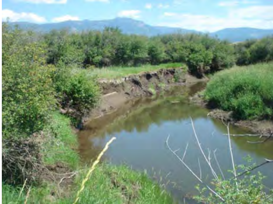
Photograph 247. View from the left bank looking downstream at bank slumps and denudation of the bank indicates, which can indicate local fine sediment input at this site at river mile 24.54. Reach 2 – Catherine Creek, Grande Ronde Subbasin, Oregon – Bureau of Reclamation Photograph by R. McAfee, July 29, 2010.
