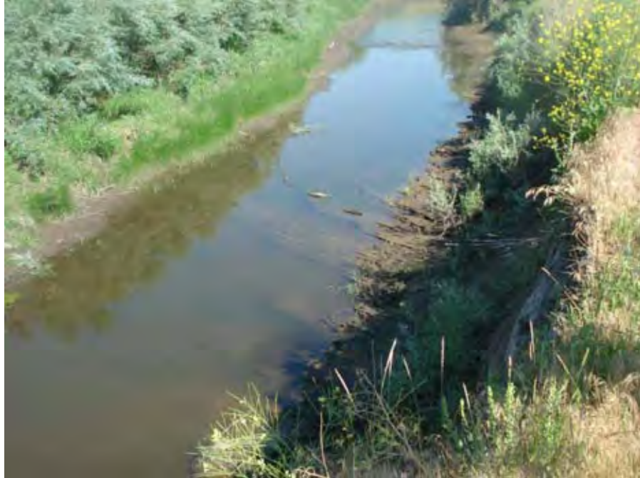
Photograph 213. View from the right bank looking downstream at a grass/willow vegetated banks, and a thinly bedded clayey-silty sand material along the toe of the right bank and in the wetted channel at river mile 27.94. Reach 2 – Catherine Creek, Grande Ronde Subbasin, Oregon – Bureau of Reclamation Photograph by R. McAfee, July 29, 2010.
