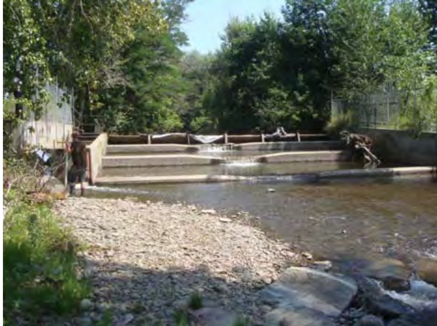
Photograph 29. View looking upstream at the Catherine Creek channel and concrete diversion dam within the city of Union, OR near river mile 39.63. Reach 3 – Catherine Creek, Grande Ronde Subbasin, Oregon – Bureau of Reclamation Photograph by D. Stelma, August 2, 2010.
