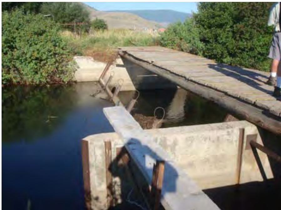
Photograph 26. View looking from right to left at the upstream side of Upper Davis Dam near river mile 34.98. Reach 2 – Catherine Creek, Grande Ronde Subbasin, Oregon – Bureau of Reclamation Photograph by D. Stelma, August 1, 2010.
