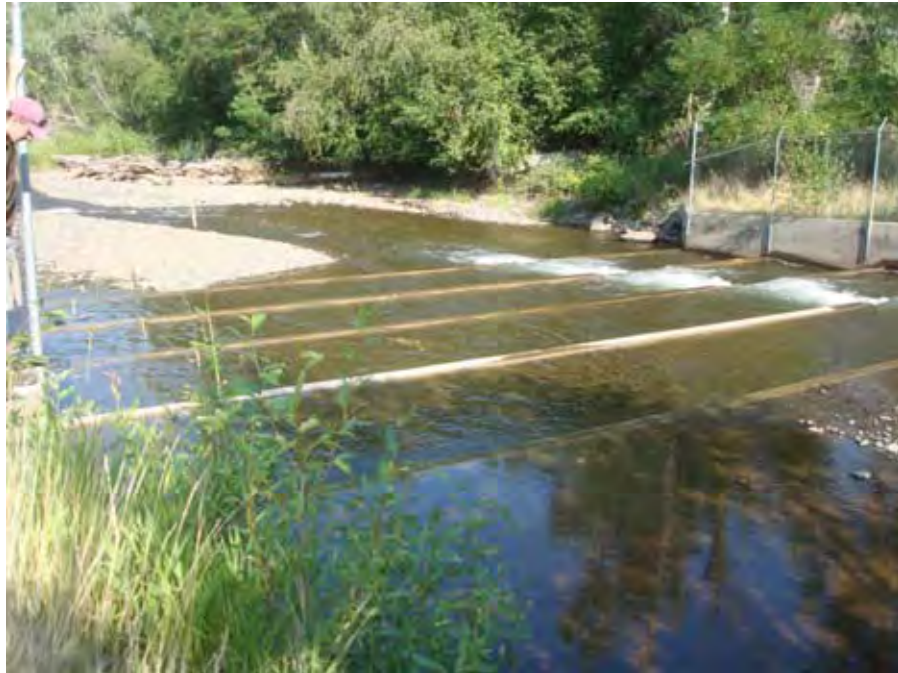
Photograph 3. View looking downstream at Schwackhammer diversion dam near river mile 40.60. Reach 3 – Catherine Creek, Grande Ronde Subbasin, Oregon – Bureau of Reclamation Photograph by D. Stelma, August 2, 2010.
