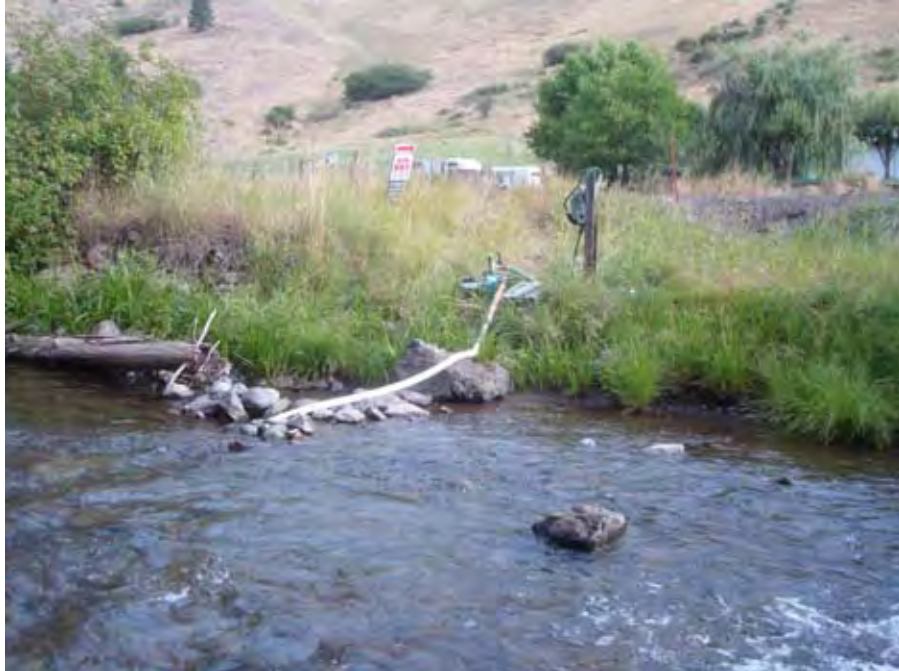
Photograph 39. View looking at 2-inch pump intake on the right bank of Catherine Creek near river mile 47.31. Reach 5 – Catherine Creek, Grande Ronde Subbasin, Oregon – Bureau of Reclamation Photograph by D. Stelma, August 18, 2010.
