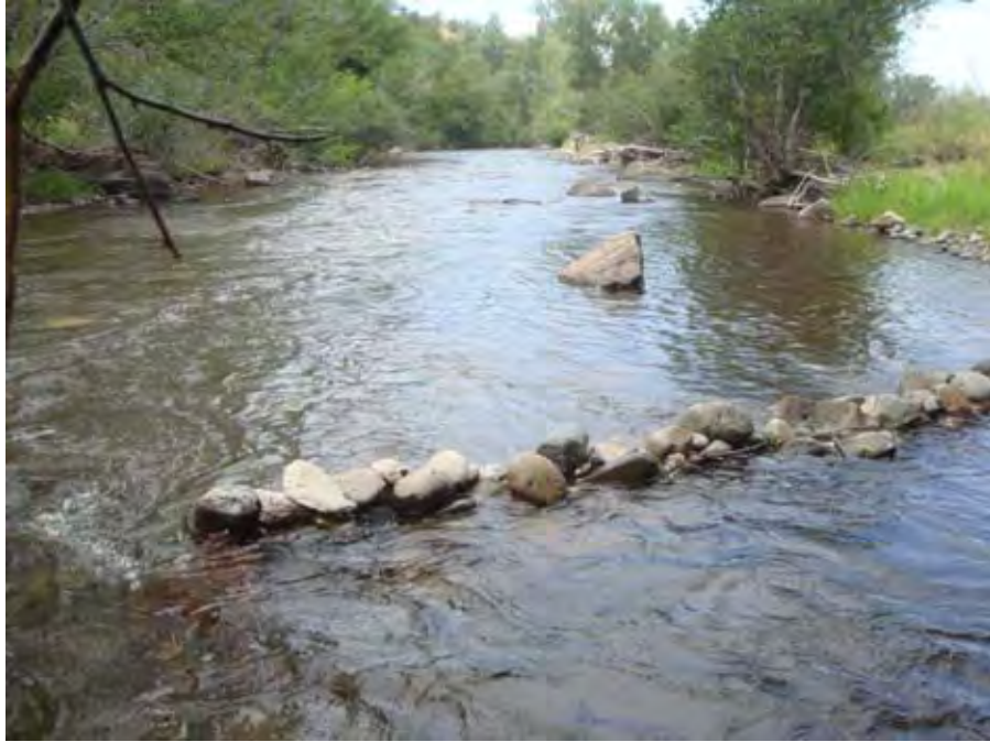
Photograph 73. View looking downstream at small rock (partial) diversion dam on the left bank of Catherine Creek near river mile 45.85. Reach 5 – Catherine Creek, Grande Ronde Subbasin, Oregon – Bureau of Reclamation Photograph by D. Stelma, August 18, 2010.
