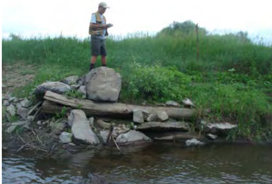
Photograph 179. A close-up view of a buried log and riprap structure along the left bank at river mile 30.30. Reach 2 – Catherine Creek, Grande Ronde Subbasin, Oregon – Bureau of Reclamation Photograph by R. McAfee, July 28, 2010.
