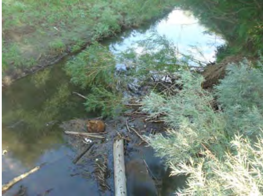
Photograph 123. A view looking downstream from Wilkinson Bridge at debris collecting in front of the sapling-pole vegetation along the right bank near river mile 31.95. Reach 2 – Catherine Creek, Grande Ronde Subbasin, Oregon – Bureau of Reclamation Photograph by R. McAfee, July 28, 2010.
