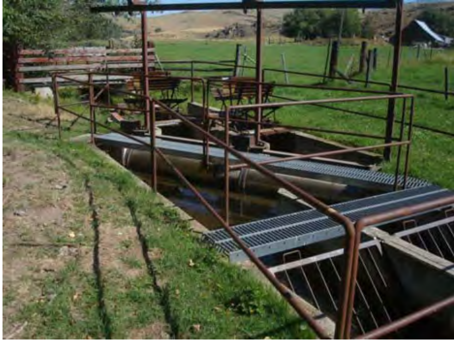
Photograph 61. Irrigation canal intake with fish screens near river mile 41.19. Reach 4 – Catherine Creek, Grande Ronde Subbasin, Oregon – Bureau of Reclamation Photograph by D. Stelma, August 16, 2010.
