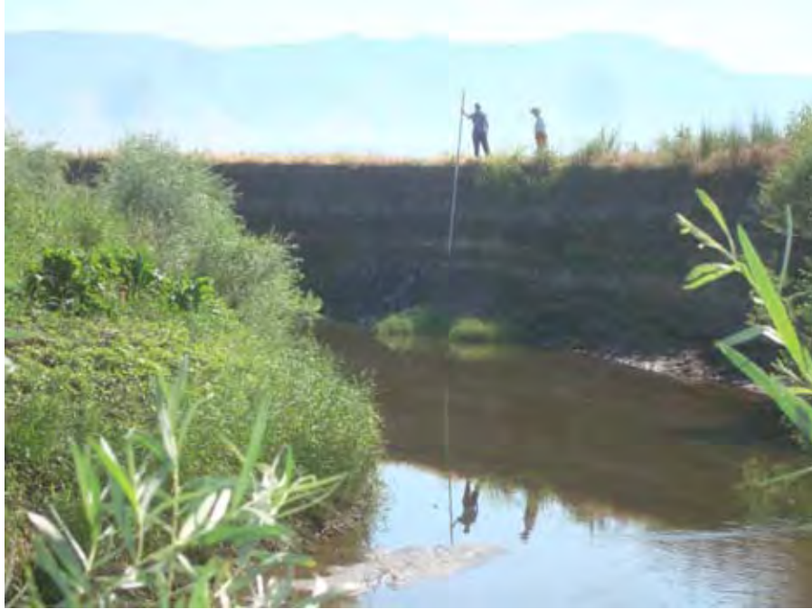
Photograph 210. View looking downstream at fine-grained alluvial sediments exposed along the right (south) bank of Catherine Creek near river mile 27.98. Reach 2 – Catherine Creek, Grande Ronde Subbasin, Oregon – Bureau of Reclamation Photograph by D. Stelma, July 29, 2010.
