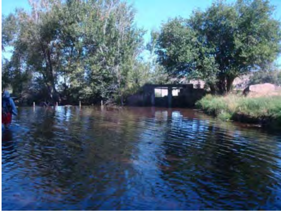
Photograph 59. View looking downstream at irrigation intake structure on the left side of the channel near river mile 41.19. Reach 4 – Catherine Creek, Grande Ronde Subbasin, Oregon – Bureau of Reclamation Photograph by D. Stelma, August 16, 2010.
