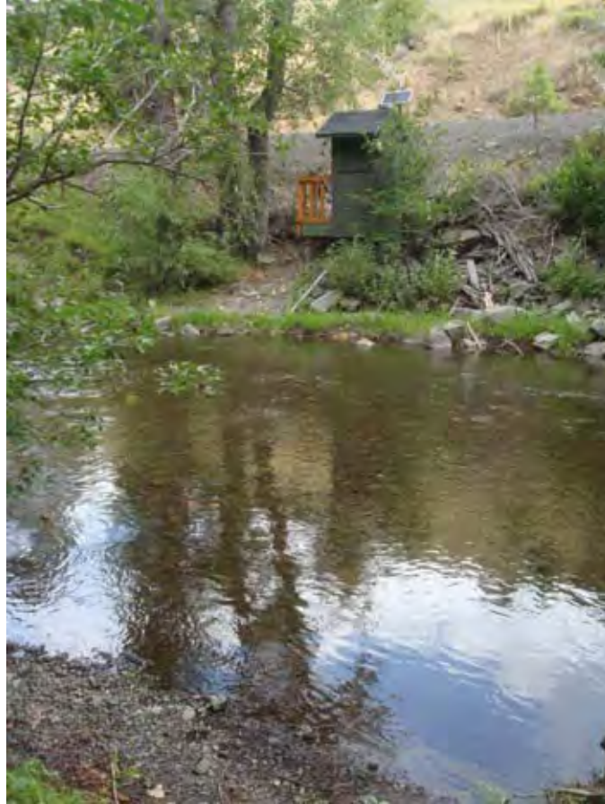
Photograph 53. View looking toward right bank at river gage station on Catherine Creek, note Oregon State (Medical Springs) Highway 203 behind building near river mile 46.70. Reach 5 – Catherine Creek, Grande Ronde Subbasin, Oregon – Bureau of Reclamation Photograph by D. Stelma, August 18, 2010.
