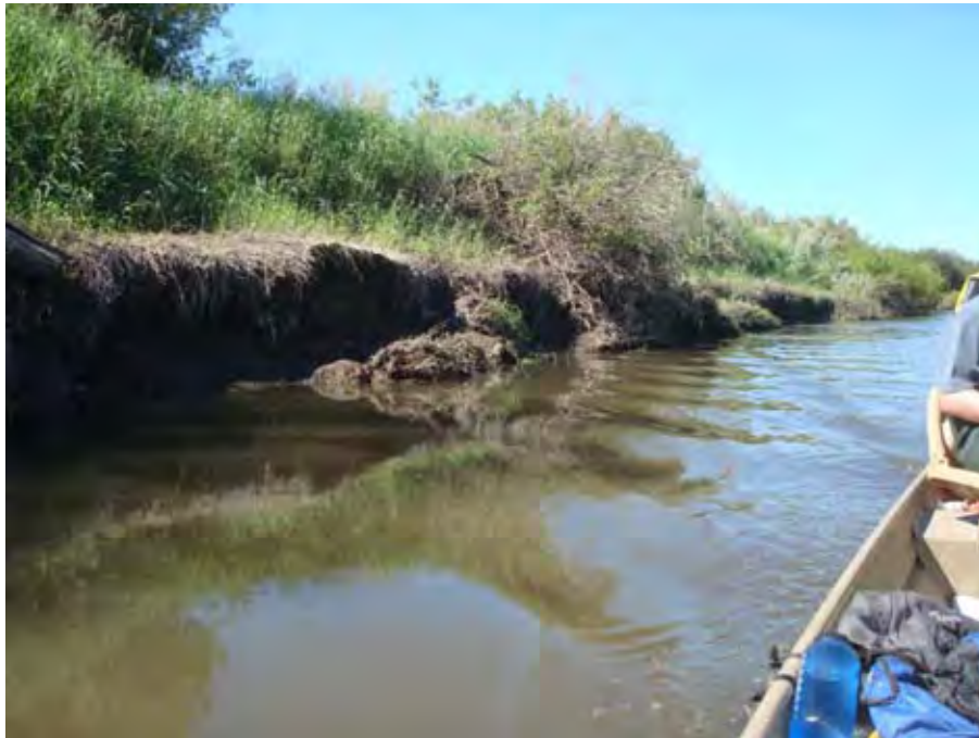
Photograph 109. View looking downstream at grass covered levee, and slumping fine-grained alluvial soil (Qal2) along the left bank of Catherine Creek near river mile 0.03. Reach 1 – Catherine Creek, Grande Ronde Subbasin, Oregon – Bureau of Reclamation Photograph by D. Stelma, July 7, 2010.
