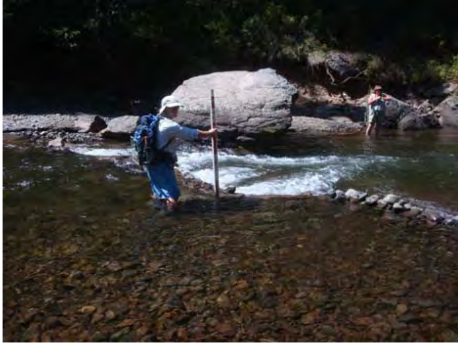
Photograph 14. View looking downstream at rock weir and pool, Catherine Creek State Park near river mile 48.99. Reach 5 – Catherine Creek, Grande Ronde Subbasin, Oregon – Bureau of Reclamation Photograph by D. Stelma, August 17, 2010.
