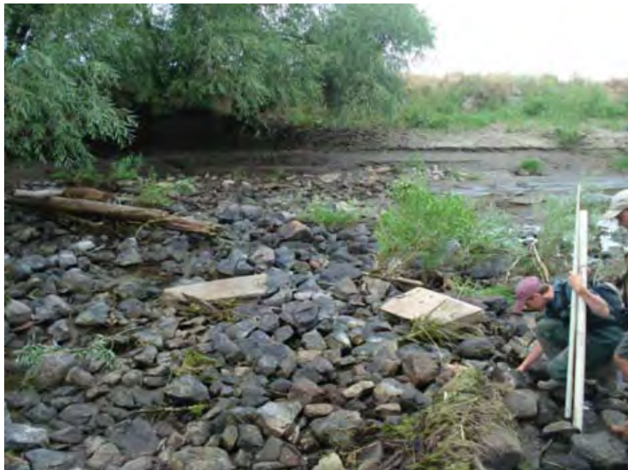
Photograph 40. View from the right bank looking downstream at 8-to-12 inch placed riprap directly downstream of Lower Davis Dam at river mile 34.40. Reach 2 – Catherine Creek, Grande Ronde Subbasin, Oregon – Bureau of Reclamation Photograph by R. McAfee, July 27, 2010.
