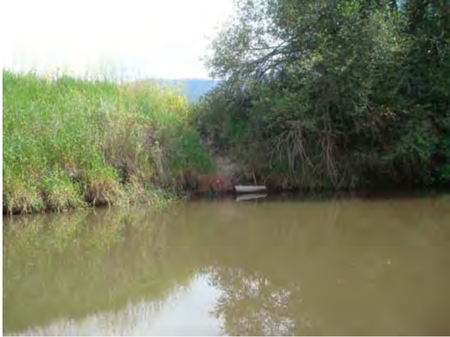
Photograph 26. View looking downstream at discharge pipe with one-way flapper valve on right bank of Catherine Creek near river mile 16.93. Reach 1 – Catherine Creek, Grand Ronde Subbasin, Oregon – Bureau of Reclamation Photograph by D. Stelma, July 10, 2010.
