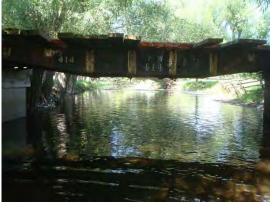
Photograph 60. View looking downstream at farm access bridge across Catherine Creek on the Yeargain property near river mile 37.64. Reach 3 – Catherine Creek, Grande Ronde Subbasin, Oregon – Bureau of Reclamation Photograph by D. Stelma, August 3, 2010.
