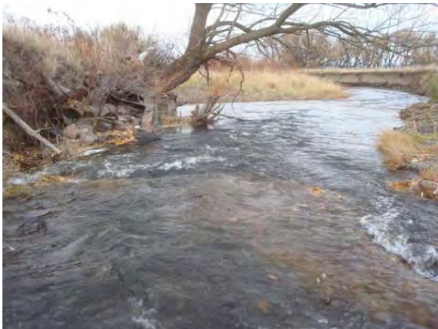
Photograph 69. View looking downstream Catherine Creek channel and head-cut area, not rock-filled automobile for erosion protection on the left bank near river mile 37.26. Reach 3 – Catherine Creek, Grande Ronde Subbasin, Oregon – Bureau of Reclamation Photograph by D. Stelma, November 9, 2010.
