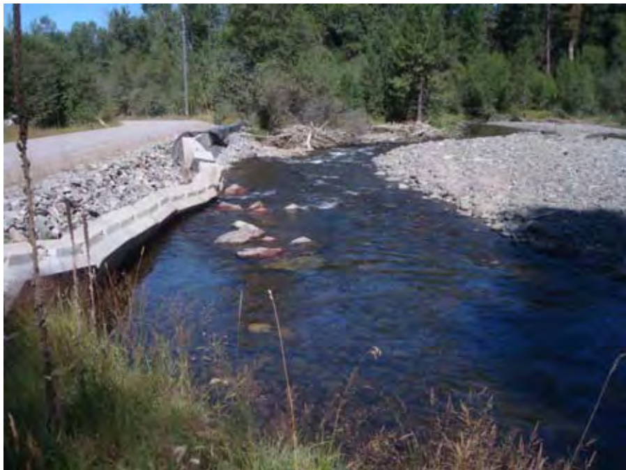
Photograph 2. View looking downstream at Catherine Creek channel near river mile 52.00, note failed concrete blocks along U.S.F.S. Road 7785 in on left side of creek. Reach 6 –
