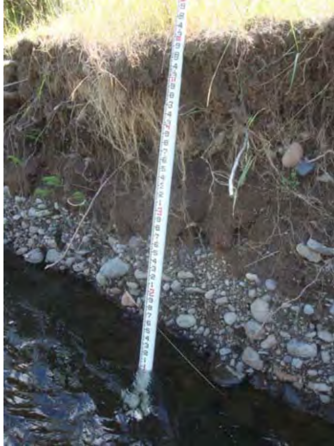
Photograph 32. View looking at top soil overlying alluvium along the left bank of Catherine Creek near river mile 47.93. Reach 5 – Catherine Creek, Grande Ronde Subbasin, Oregon – Bureau of Reclamation Photograph by D. Stelma, August 17, 2010.
