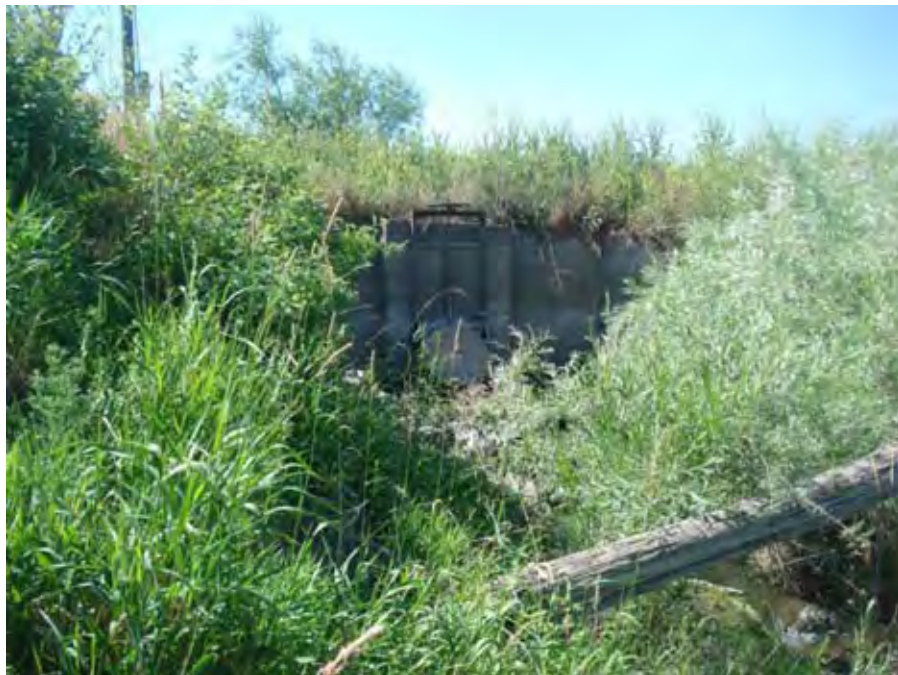
Photograph 225. View of an irrigation return constructed of concrete with a metal drum gate along the right bank near river mile 27.30. Reach 2 – Catherine Creek, Grande Ronde Subbasin, Oregon – Bureau of Reclamation Photograph by R. McAfee, July 29, 2010.
