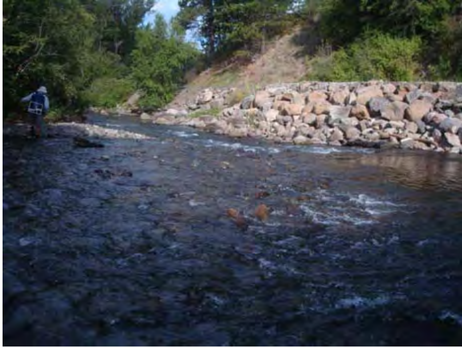
Photograph 37. View looking downstream at Catherine Creek channel, Oregon State (Medical Springs) Highway 203 in background near river mile 47.51, note rip rap erosion protection along road embankment. Reach 5 – Catherine Creek, Grande Ronde Subbasin, Oregon – Bureau of Reclamation Photograph by D. Stelma, August 18, 2010.
