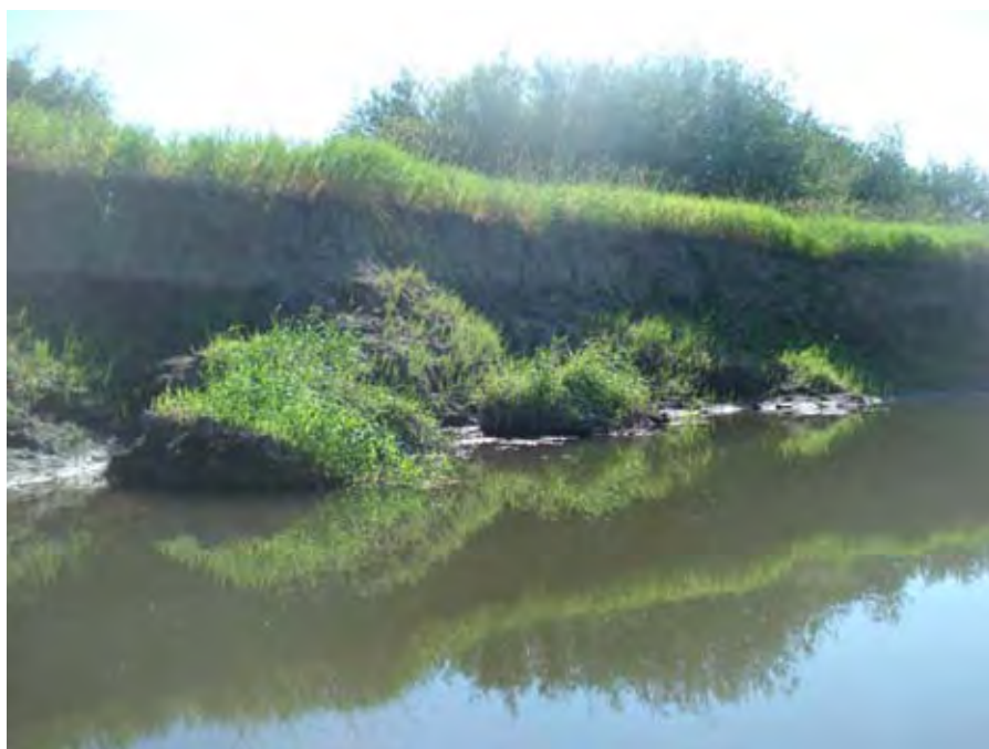
Photograph 252. View looking at block-sized bank slumps along the right bank near river 23.92. Reach 2 – Catherine Creek, Grande Ronde Subbasin, Oregon – Bureau of Reclamation Photograph by R. McAfee, July 30, 2010.
