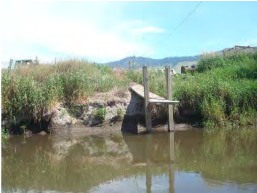
Photograph 37. Dock on right (east) bank of Catherine Creek upstream of Booth Road bridge near river mile 15.45. Reach 1 – Catherine Creek, Grande Ronde Subbasin, Oregon – Bureau of Reclamation Photograph by D. Stelma, July 10, 2010.
