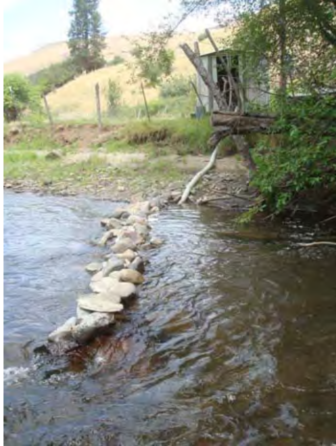
Photograph 72. View looking downstream at small rock (partial) diversion dam on the left bank of Catherine Creek near river mile 45.85, note pump intake in creek and pump house on upper left bank. Reach 5 – Catherine Creek, Grande Ronde Subbasin, Oregon – Bureau of Reclamation Photograph by D. Stelma, August 18, 2010.
