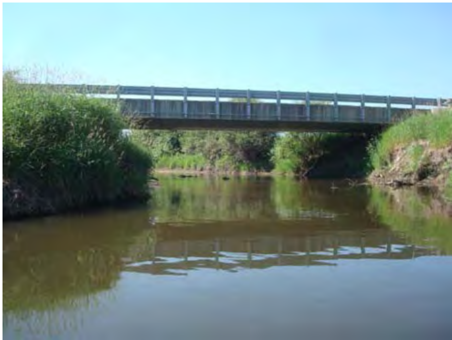
Photograph 254. View looking upstream at the Gekler Lane Bridge near river mile 23.68. Reach 2 – Catherine Creek, Grande Ronde Subbasin, Oregon – Bureau of Reclamation Photograph by D. Stelma, July 30, 2010.
