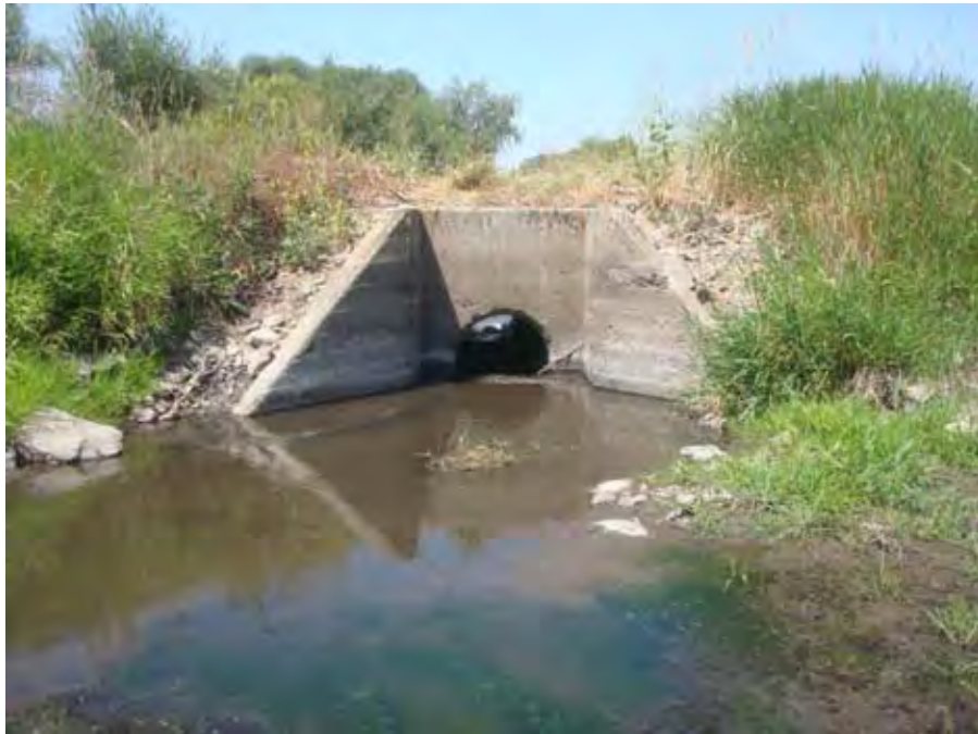
Photograph 9. View looking downstream at culvert and farm road crossing Pyles Creek near the confluence with Catherine Creek near river mile 36.89. Reach 2 – Catherine Creek, Grande Ronde Subbasin, Oregon – Bureau of Reclamation Photograph by D. Stelma, August 3, 2010.
