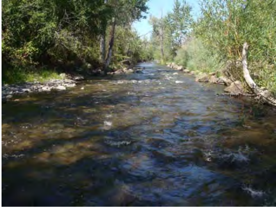
Photograph 63. View looking downstream at the Catherine Creek channel adjacent to Oregon State (Medical Springs) Highway 203, located to the right, near river mile 41.05, note rip rap erosion protection on right bank. Reach 4 – Catherine Creek, Grande Ronde Subbasin, Oregon – Bureau of Reclamation Photograph by D. Stelma, August 16, 2010.
