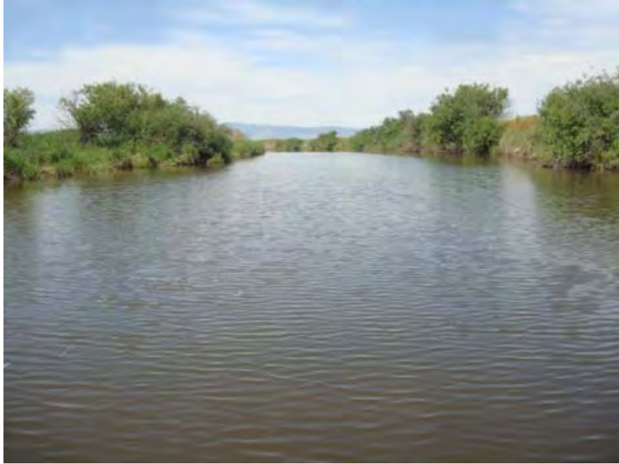
Photograph 43. View looking upstream at Catherine Creek channel upstream of Elmer Dam near river mile 14.40. Reach 1 – Catherine Creek, Grande Ronde Subbasin, Oregon – Bureau of Reclamation Photograph by D. Stelma, July 10, 2010.
