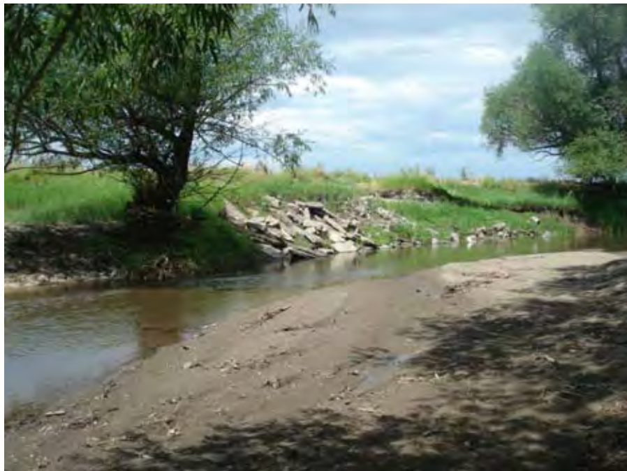
Photograph 189. View from the right bank looking downstream at a section of concrete slab armoring along the left bank and a point bar comprised of sand-sized material along the right bank river mile 30.11. Reach 2 – Catherine Creek, Grande Ronde Subbasin, Oregon – Bureau of Reclamation Photograph by R. McAfee, July 28, 2010.
