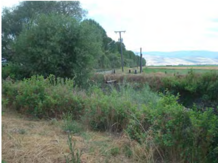
Photograph 62. View from the top of the left bank looking downstream at a floodwater pump and return upstream the Woodruff Lane Bridge near river mile 33.85. Reach 2 – Catherine Creek, Grande Ronde Subbasin, Oregon – Bureau of Reclamation Photograph by R. McAfee, July 27, 2010.
