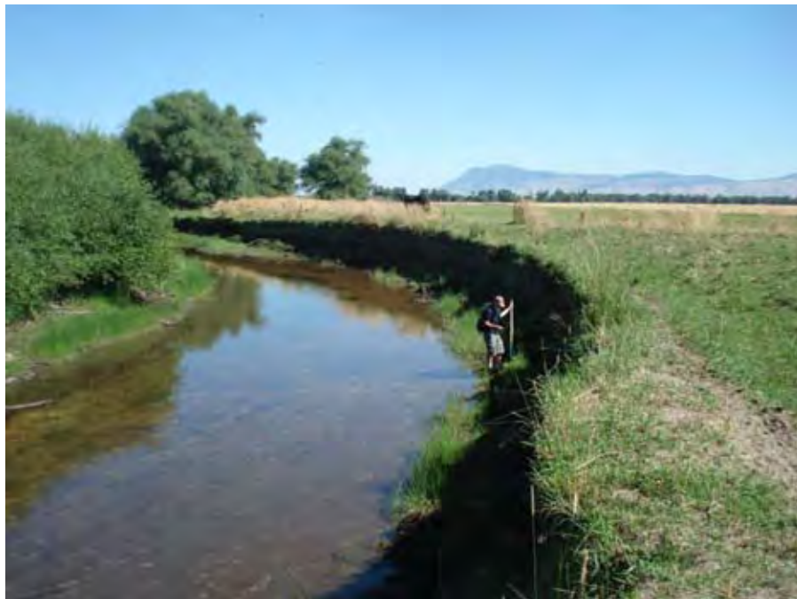
Photograph 94. View of a section of the right bank that is near vertical, with banks slumps at the toe near river mile 32.90. Note the firm, silty material that is erosion resistant in the channel. Reach 2 – Catherine Creek, Grande Ronde Subbasin, Oregon – Bureau of Reclamation Photograph by R. McAfee, August 1, 2010.
