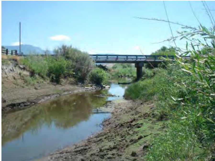
Photograph 229. View from the right bank looking downstream at Godley Lane Bridge at river mile 26.70. Note the small section of riprap on the left bank underneath the bush at the water's edge. Reach 2 – Catherine Creek, Grande Ronde Subbasin, Oregon – Bureau of Reclamation Photograph by R. McAfee, July 29, 2010.
