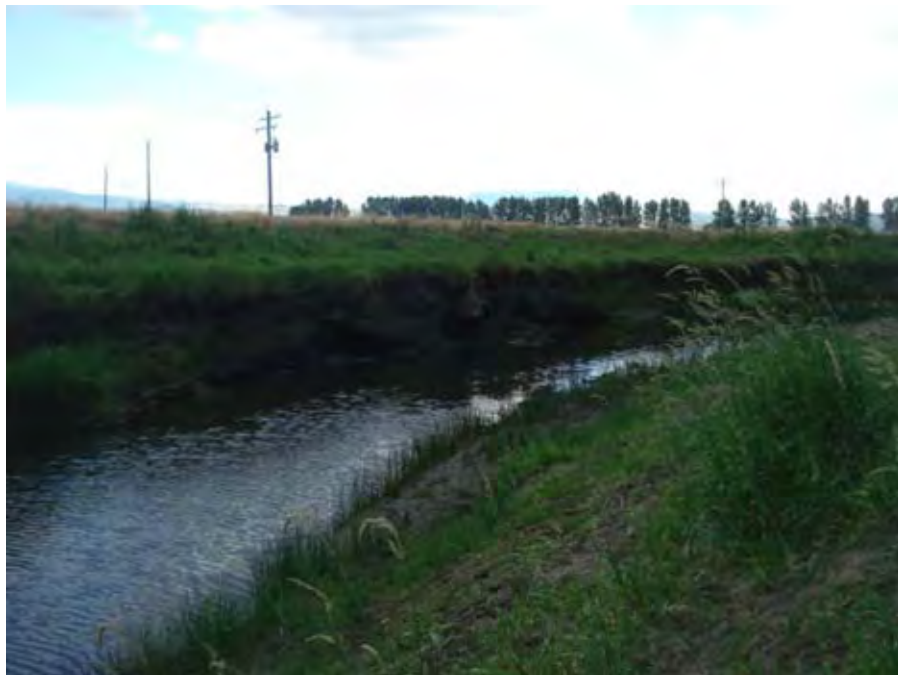
Photograph 78. View to the south, looking upstream at an eroding grass-covered right bank on the outside of a meander bend near river mile 33.50. Reach 2 – Catherine Creek, Grande Ronde Subbasin, Oregon – Bureau of Reclamation Photograph by R. McAfee, July 27, 2010.
