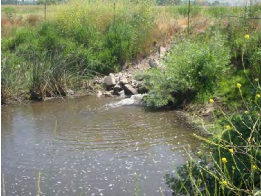
Photograph 8. Pyles Creek discharge from culvert near the confluence with Catherine Creek near river mile 36.89. Reach 2 – Catherine Creek, Grande Ronde Subbasin, Oregon – Bureau of Reclamation Photograph by D. Stelma, August 3, 2010.
