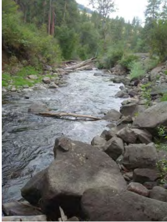
Photograph 62. View looking downstream at Catherine Creek channel in the canyon section, Oregon State (Medical Springs) Highway 203 is to the right near river mile 46.22, note abundance of boulders derived from landslide debris (left bank) and road construction (right bank). Reach 5 – Catherine Creek, Grande Ronde Subbasin, Oregon – Bureau of Reclamation Photograph by D. Stelma, August 18, 2010.
