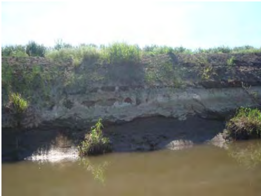
Photograph 13. View of fine-grained alluvium exposed on the right (east) bank of Catherine Creek near river mile 20.65. Reach 1 – Catherine Creek, Grande Ronde Subbasin, Oregon – Bureau of Reclamation Photograph by D. Stelma, July 11, 2010.
