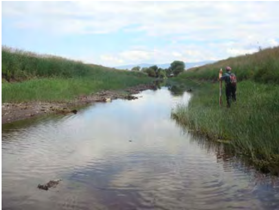
Photograph 66. View looking downstream at Catherine Creek through the long straight artificial channel section, note silty sand and sand silt bed deposits near river mile 33.80. Reach 2 – Catherine Creek, Grande Ronde Subbasin, Oregon – Bureau of Reclamation Photograph by D. Stelma, July 27, 2010.
