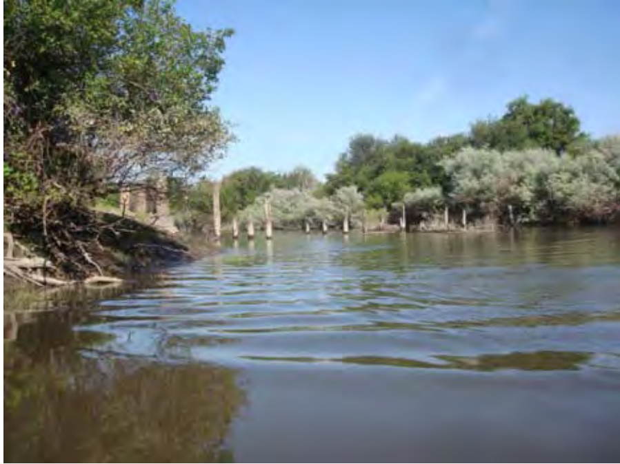
Photograph 79. View looking downstream at abandoned bridge piers near river mile 7.60. Reach 1 – Catherine Creek, Grande Ronde Subbasin, Oregon – Bureau of Reclamation Photograph by D. Stelma, July 9, 2010.
