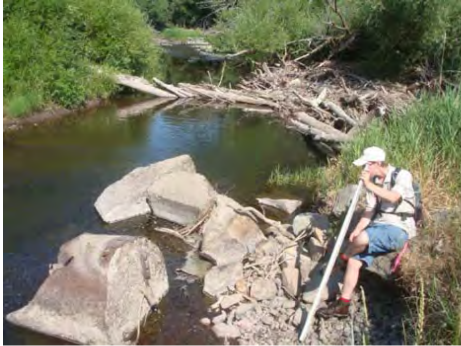
Photograph 53. View looking downstream at log jam and rip rap within the Catherine Creek channel near river mile 38.19. Reach 3 – Catherine Creek, Grande Ronde Subbasin, Oregon – Bureau of Reclamation Photograph by D. Stelma, August 3, 2010.
