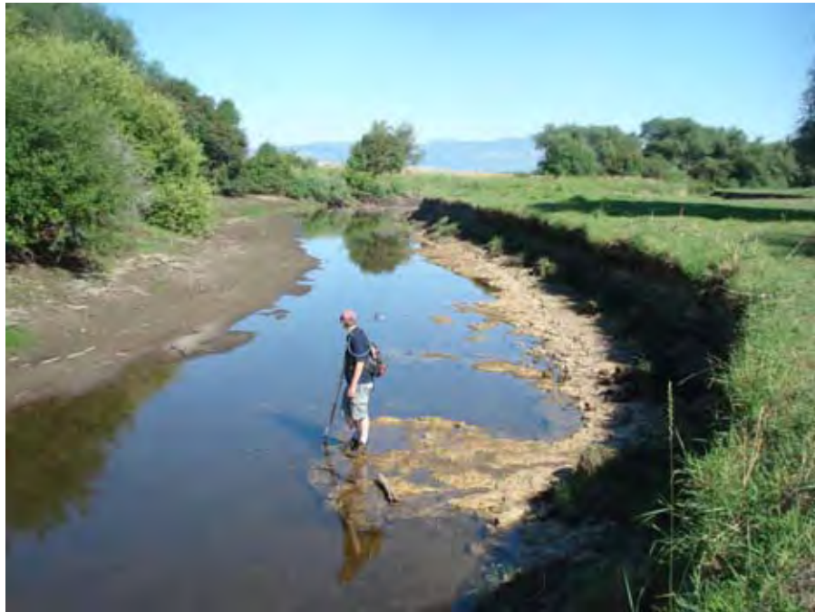
Photograph 153. View looking downstream from the top of the right bank near river mile 31.14. The channel bottom is comprised of a dense, firm silty material that is erosion resistant, and visible along the toe of the right bank. Reach 2 – Catherine Creek, Grande Ronde Subbasin, Oregon – Bureau of Reclamation Photograph by R. McAfee, August 1, 2010.
