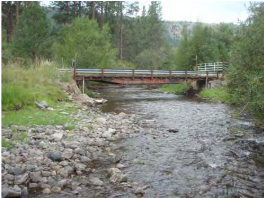
Photograph 57. View looking downstream at residential access bridge across Catherine Creek near river mile 46.53. Reach 5 – Catherine Creek, Grande Ronde Subbasin, Oregon – Bureau of Reclamation Photograph by D. Stelma, August 18, 2010.
