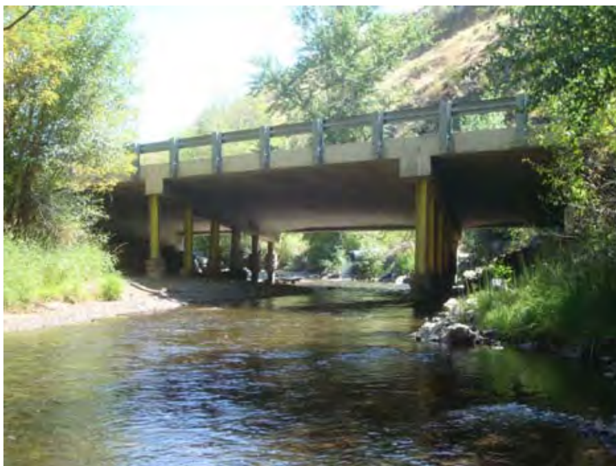
Photograph 2. View looking upstream at the Oregon State (Medical Springs) Highway 203 Bridge over Catherine Creek at Union, OR near river mile 40.65. Reach 3 – Catherine Creek, Grande Ronde Subbasin, Oregon – Bureau of Reclamation Photograph by D. Stelma, August 16, 2010.
