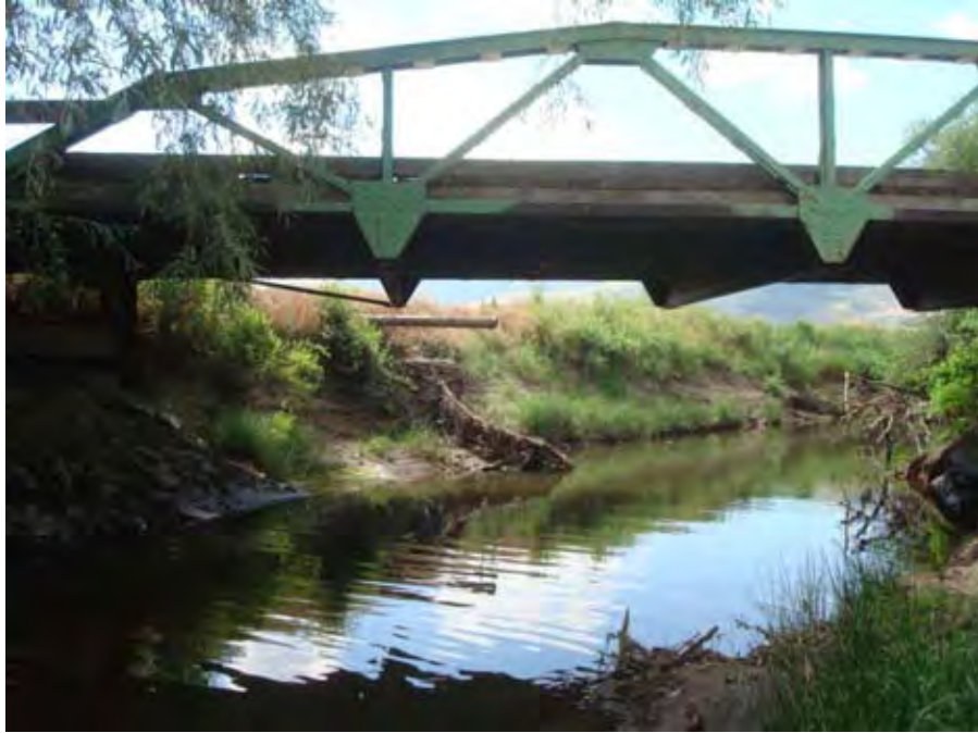
Photograph 65. View looking downstream at the Woodruff Lane Bridge near river mile 33.84. Reach 2 – Catherine Creek, Grande Ronde Subbasin, Oregon – Bureau of Reclamation Photograph by D. Stelma, July 27, 2010.
