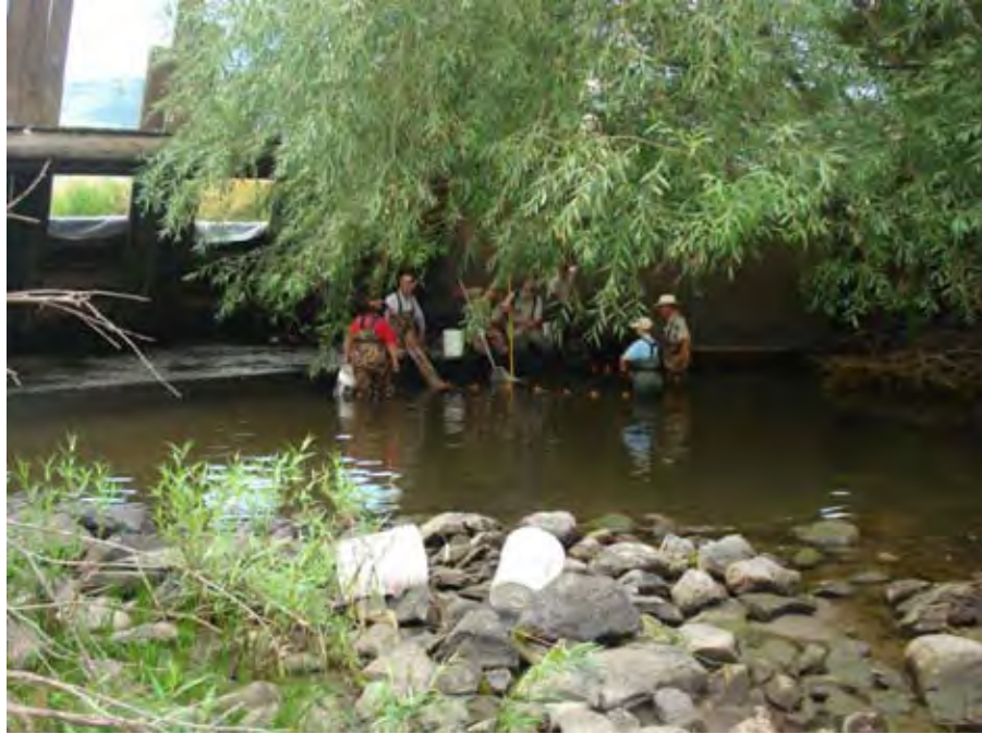
Photograph 41. View from the right bank looking upstream at a plunge pool located on the downstream side of Lower Davis Dam near river mile 34.40. Reach 2 – Catherine Creek, Grande Ronde Subbasin, Oregon – Bureau of Reclamation Photograph by R. McAfee, July 27 2010.
