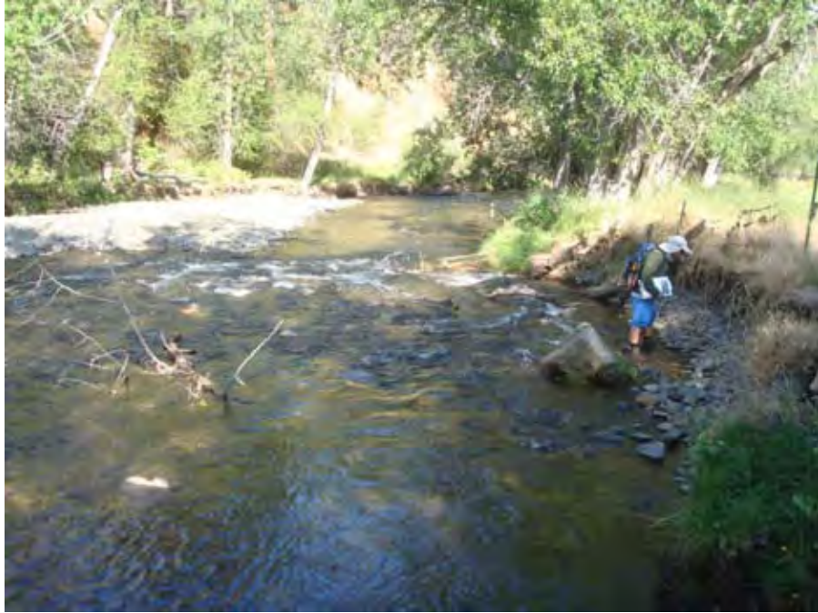
Photograph 20. View looking downstream at Catherine Creek channel near river mile 42.96, note left bank erosion. Reach 4 – Catherine Creek, Grande Ronde Subbasin, Oregon – Bureau of Reclamation Photograph by D. Stelma, August 19, 2010.
