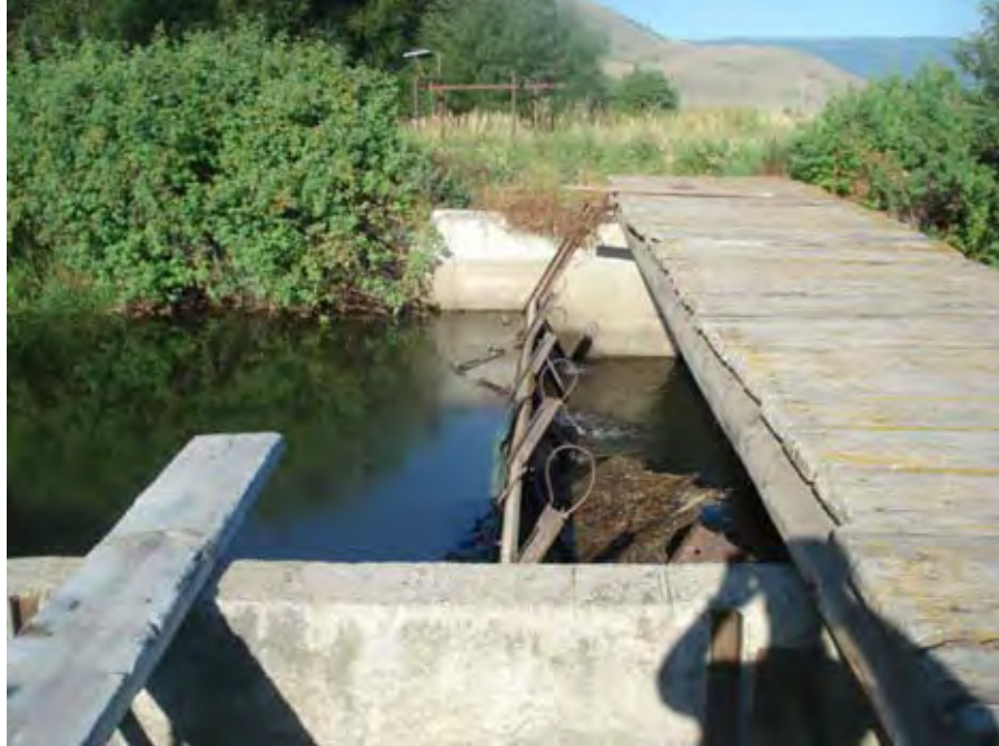
Photograph 27. View of water backed up at Upper Davis Dam at river mile 34.98. Reach 2 – Catherine Creek, Grande Ronde Subbasin, Oregon – Bureau of Reclamation Photograph by R. McAfee, August 1, 2010.
