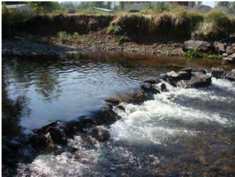
Photograph 13. View looking from right to left across the Catherine Creek in Union, OR at a rock weir (energy dissipater) structure near river mile 40.33. Reach 3 – Catherine Creek, Grande Ronde Subbasin, Oregon – Bureau of Reclamation Photograph by D. Stelma, August 2, 2010.
