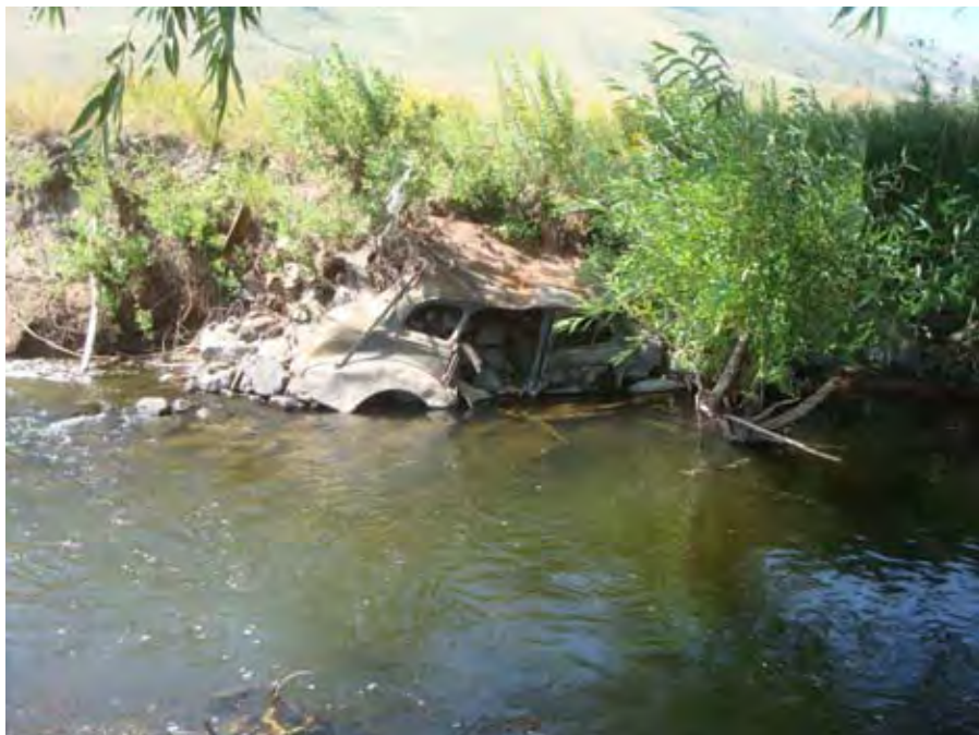
Photograph 71. Rock-filled automobile used for erosion protection on the left bank of Catherine Creek near river mile 37.26. Reach – Catherine Creek, Grande Ronde Subbasin, Oregon – Bureau of Reclamation Photograph by D. Stelma, August 3, 2010.
