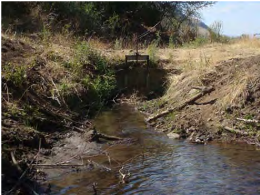
Photograph 8. Close-up of diversion and head gate on right bank of Catherine Creek near river mile 44.98. Reach 4 – Catherine Creek, Grande Ronde Subbasin, Oregon – Bureau of Reclamation Photograph by D. Stelma, August 18, 2010.
