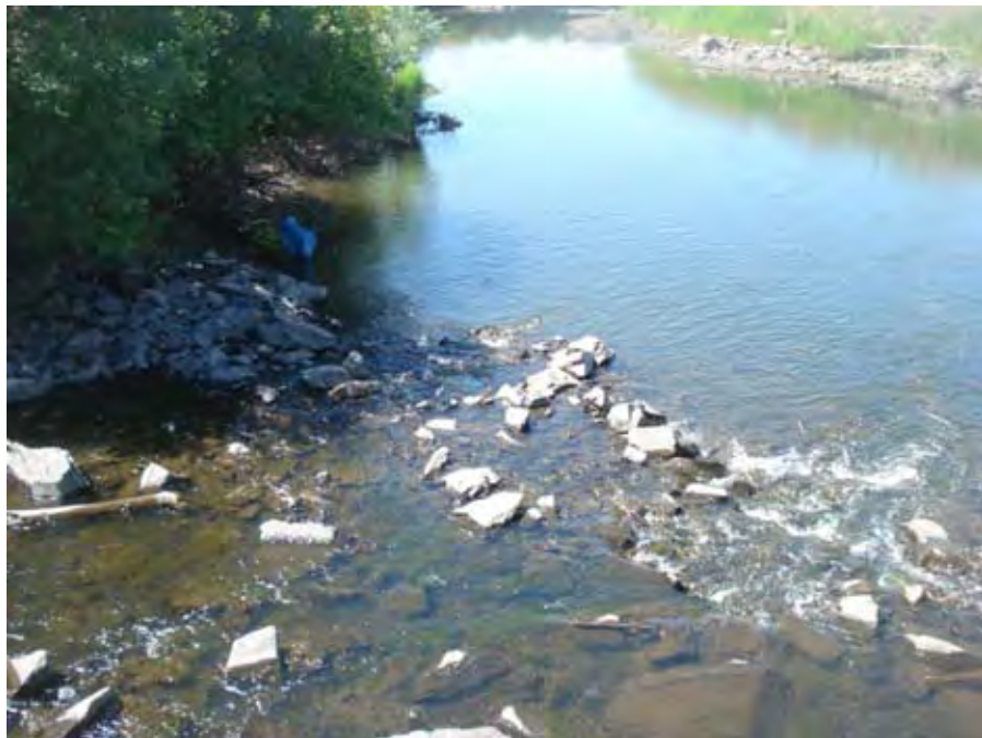
Photograph 32. View looking downstream from Upper Davis Dam at the riprap across the bottom of the channel and along the left bank near river mile 34.98. Reach 2 – Catherine Creek, Grande Ronde Subbasin, Oregon – Bureau of Reclamation Photograph by R. McAfee, July 27, 2010.
