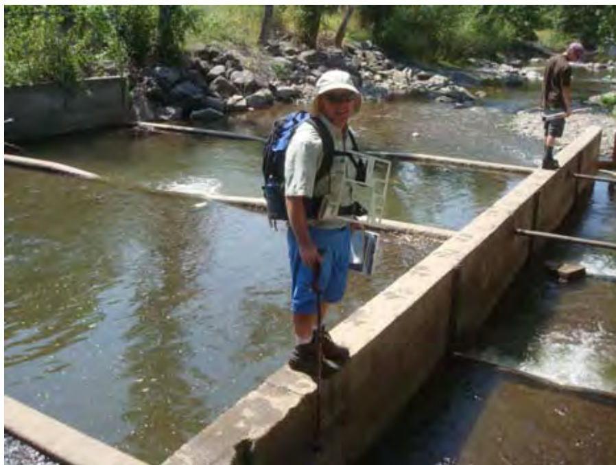
Photograph 30. View looking downstream at the Catherine Creek channel and concrete diversion dam within the city of Union, OR near river mile 39.63. Reach 3 – Catherine Creek, Grande Ronde Subbasin, Oregon – Bureau of Reclamation Photograph by D. Stelma, August 2, 2010.
