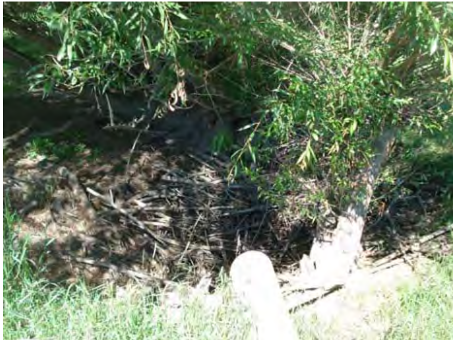
Photograph 96. View of a pump discharge on the inside of a levee set back from the right bank near river mile 32.88. Reach 2 – Catherine Creek, Grande Ronde Subbasin, Oregon – Bureau of Reclamation Photograph by R. McAfee, August 1, 2010.
