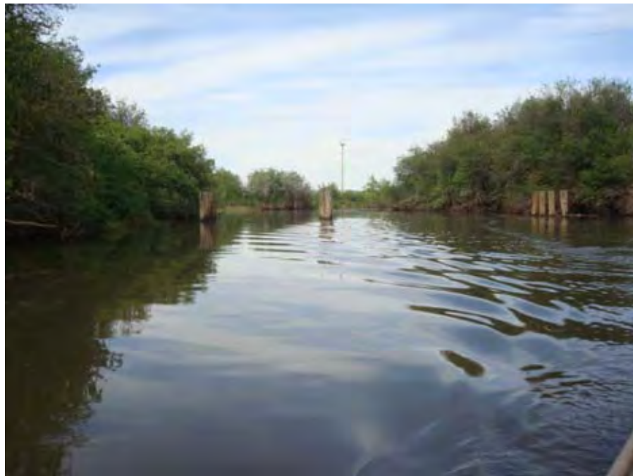
Photograph 54. View looking downstream at abandoned bridge piers exposed in the Catherine Creek channel upstream of Elmer Dam near river mile 13.24. Reach 1 – Catherine Creek, Grande Ronde Subbasin, Oregon – Bureau of Reclamation Photograph by D. Stelma, July 10, 2010.
