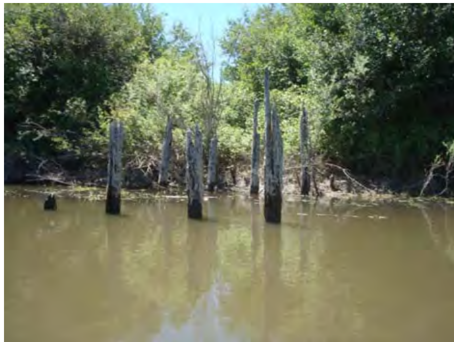
Photograph 89. Remnants of bridge supports, Catherine Creek near river mile 5.30. Reach 1 – Catherine Creek, Grande Ronde Subbasin, Oregon – Bureau of Reclamation Photograph by D. Stelma, July 7, 2010.
