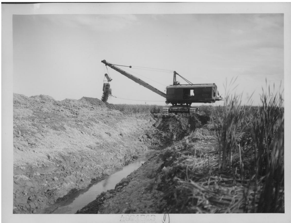
Figure 15 June 22, 1914 "Electric Dredge on Wilson Slough Drain." 101
