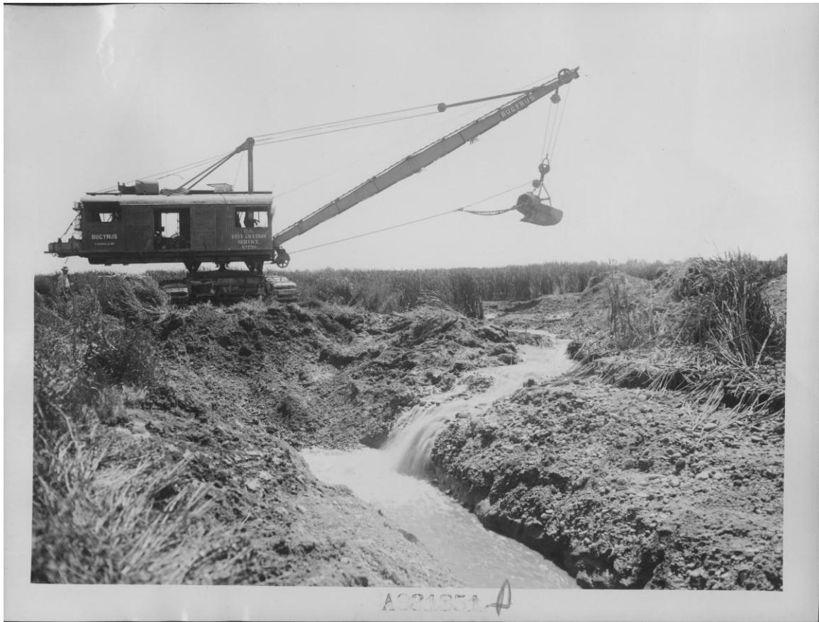
Figure 22 June 22, 1914 Electric Dredge excavating, Purdam Slough Drain on Lemp's Ranch." 108
