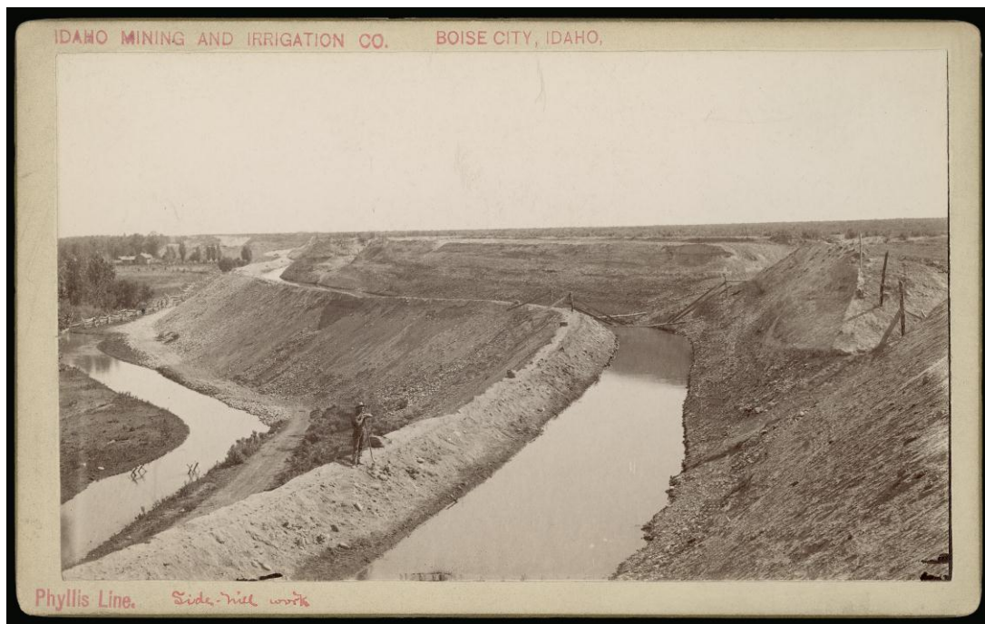
Figure 3 Phyllis Canal, Side Hill Work, c. 1890 Courtesy of Brigham Young University, Idaho Mining and Irrigation Co. Photo Collection
