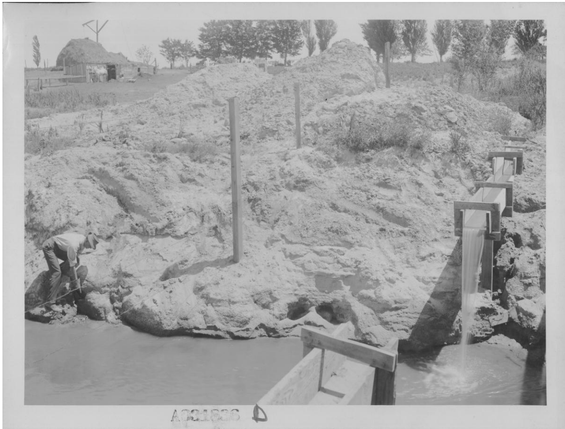
Figure 18 (no date, likely June 22, 1914) "View showing drainage from water bearing strata on Mason Creek Drain." 104
