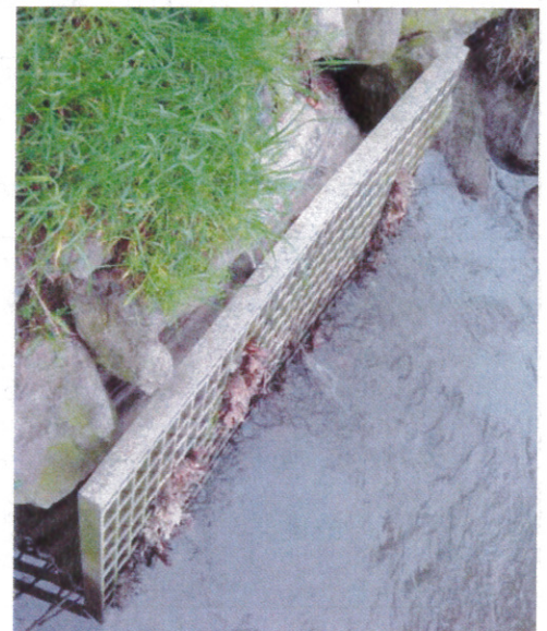
City storm water outfall located at Coyote Creek.
