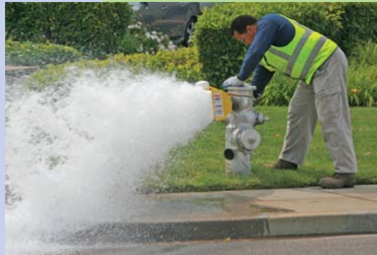
Operator flushes the distribution system
