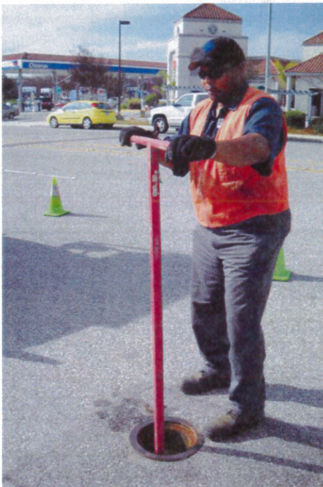
City worker, Jon Frost, exercises a water valve.
