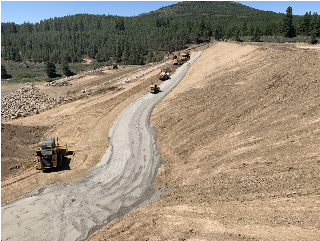
Construction of filter zones at Boca Dam; filter zones layer filter sand against existing embankment, followed by drain rock. The filter zone is then encapsulated with in-reservoir-borrow material.
