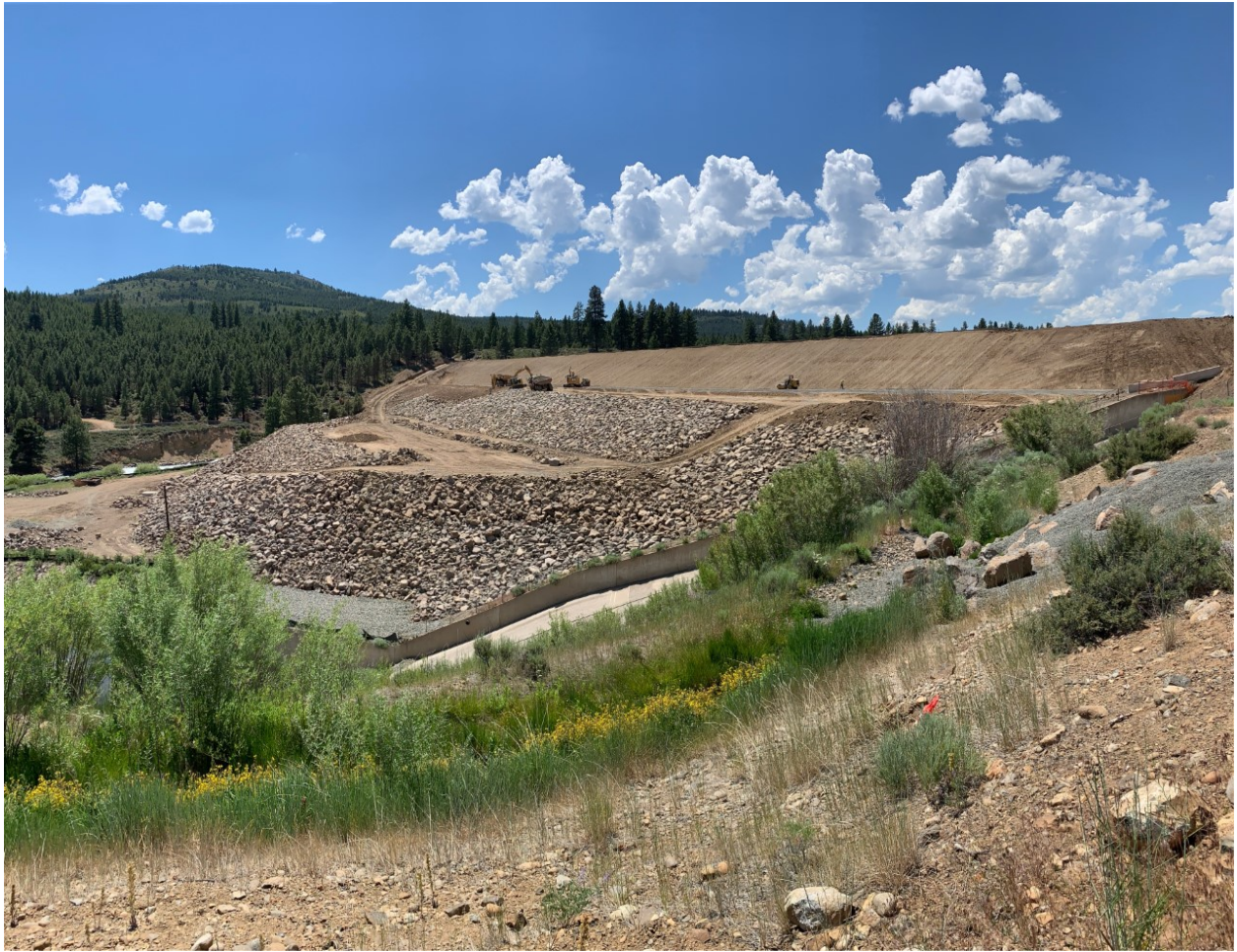
Construction of dam embankment and filter zones in progress (remove period after progress).
