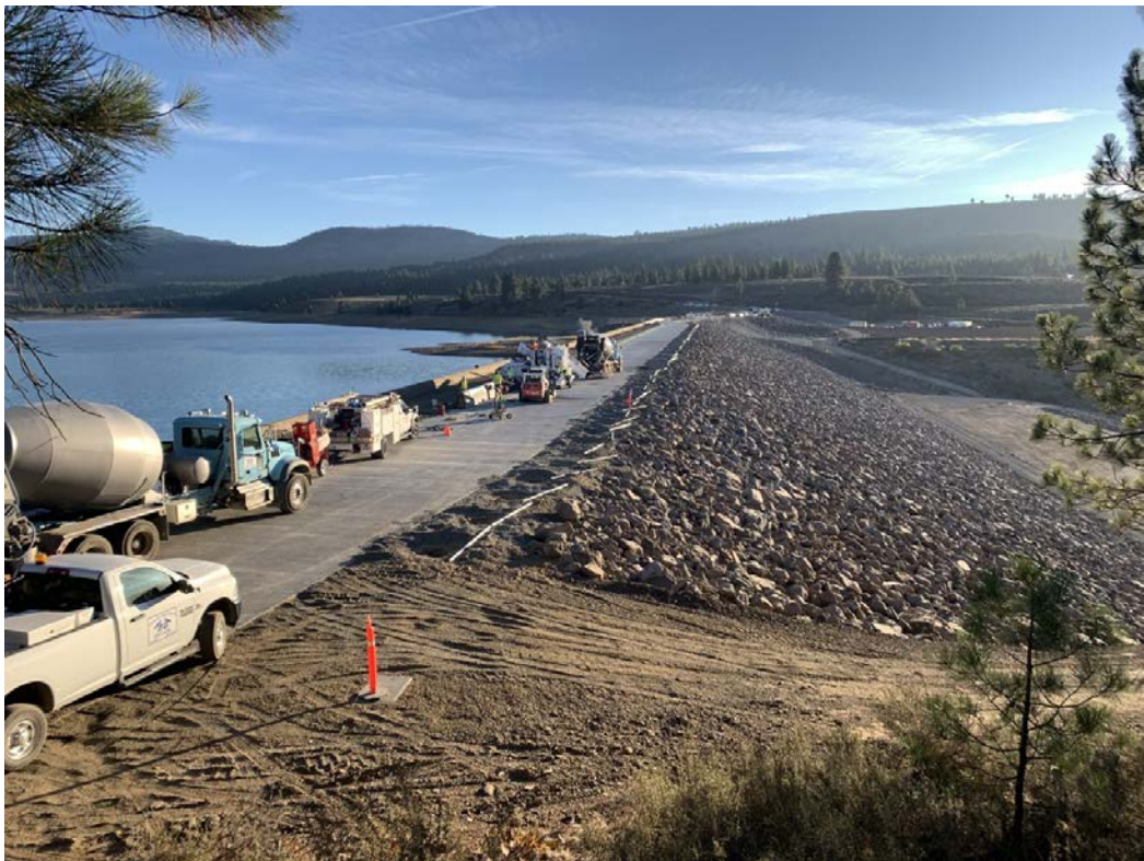
Construction of concrete barrier in progress
