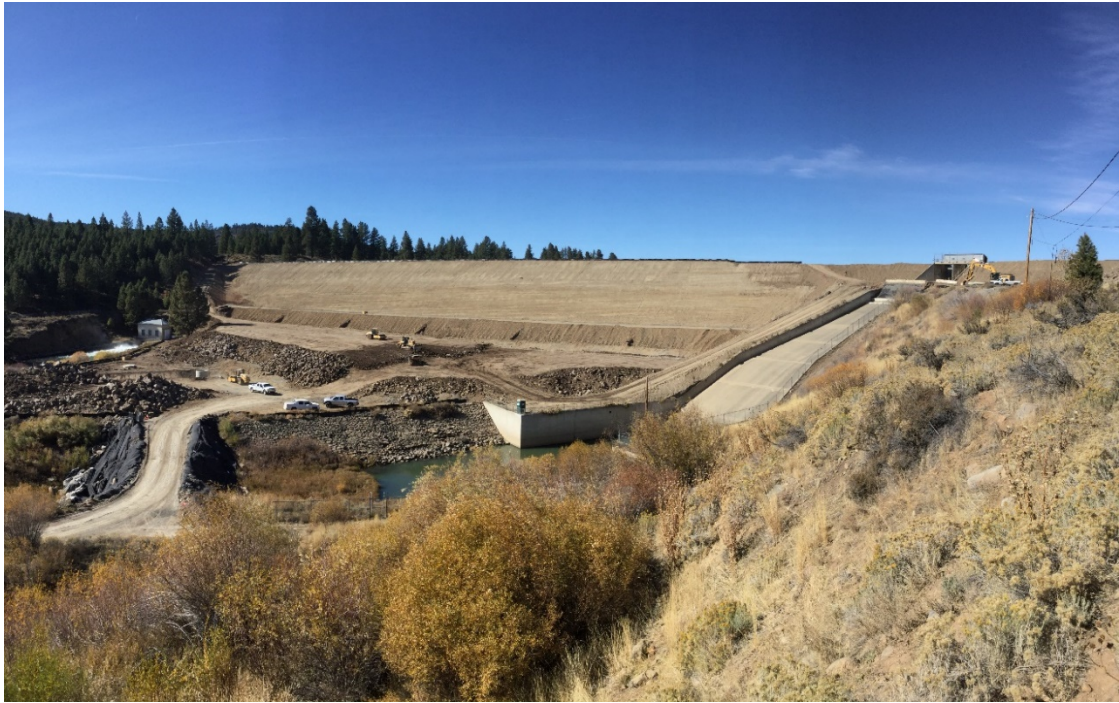
Construction of stability berm in progress
