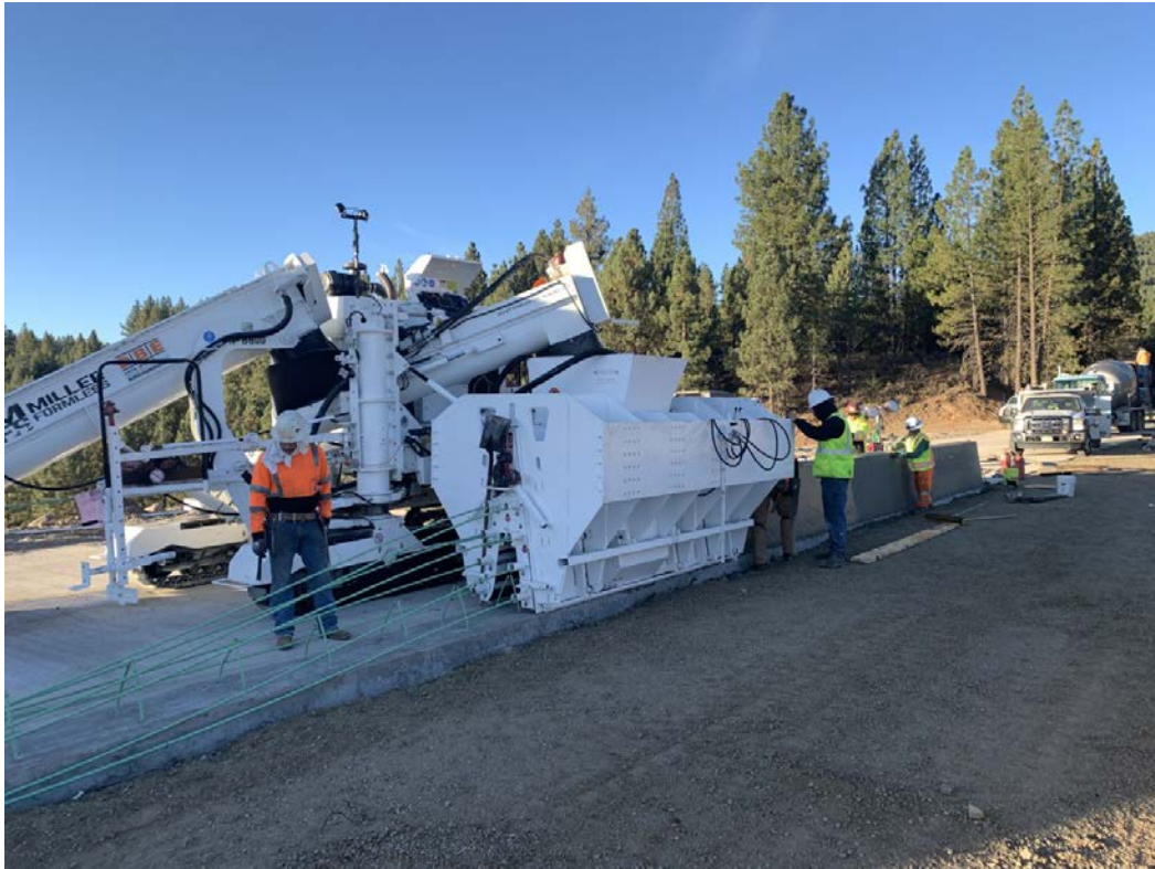
Concrete barrier placement using slip form method; this method places concrete into a continuously moving form.
