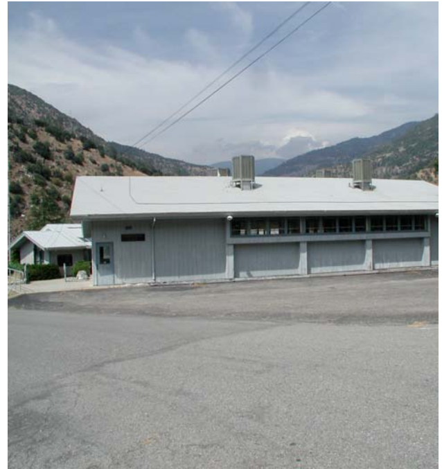
Above: Chawanakee School at SCE's former Powerhouse 3 community, view northeast—shows entire building (mid-afternoon). (P6180045.JPG)
