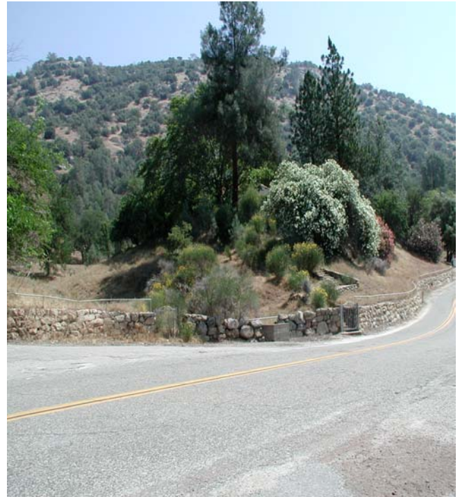
Above: Former PG&E residential area across from A.G. Wishon Powerhouse; note oleanders (late morning). (P6180022.JPG)
