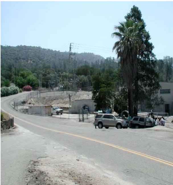
Above: General view of A.G. Wishon Powerhouse (PG&E) from across the road, view northeast (late morning). (P6180023.JPG)
