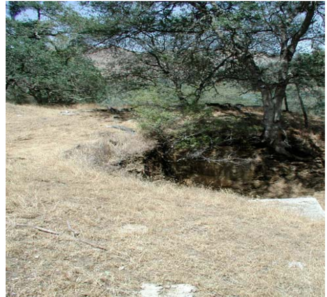
Above: Excavation for stamp mill at Patterson Mine, Millerton Lake State Recreation Area, SE ¼ Sect. 7, R22E T10S, elevation < 800'; concrete foundation of stamp mill barely shows (would be inundated by MP 279 dam, and by MP 274 dam) (early afternoon). (P190083.JPG)
