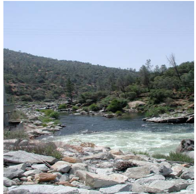
Above: View upstream, at SCE's Big Creek Powerhouse No. 4 (late morning). (P6180028.JPG)
