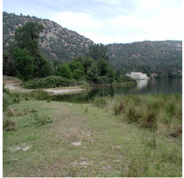
Above: View east at mouth of creek or discharge channel; A.G. Wishon Powerhouse in background (early afternoon). (P6180035.JPG)
