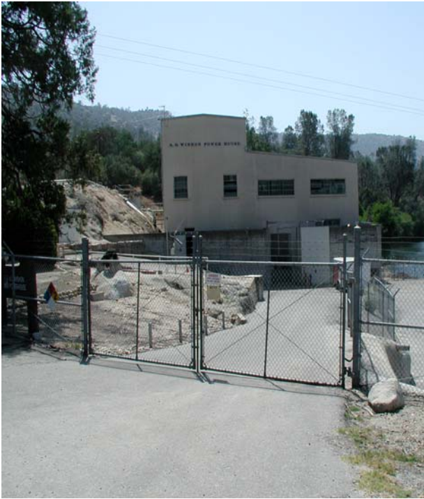
Above: A.G. Wishon Powerhouse (PG&E), view north; late morning. (P6180021.JPG)
