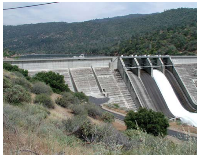
Above: Redinger Lake Dam, close-up, view east (mid-afternoon). (P6180039.JPG)
