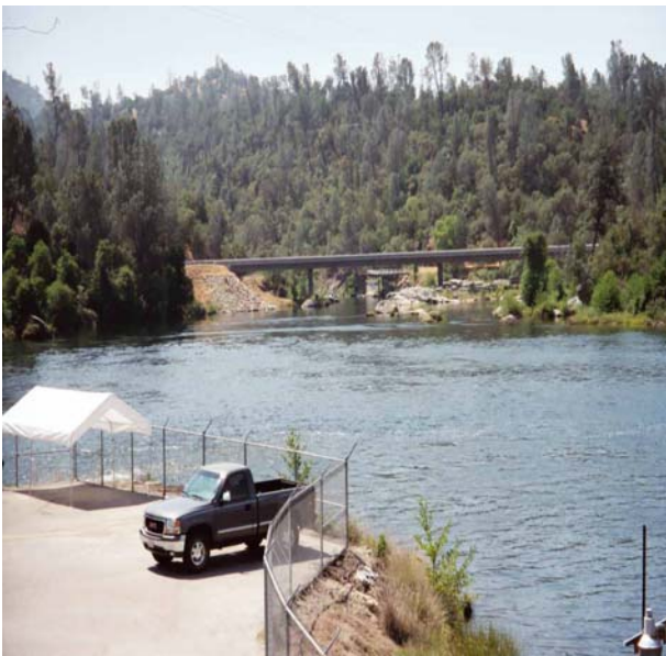
Above: Kerkhoff Reservoir near Wishon Powerhouse (view upstream, June 18 2003) (011_8.JPG)
