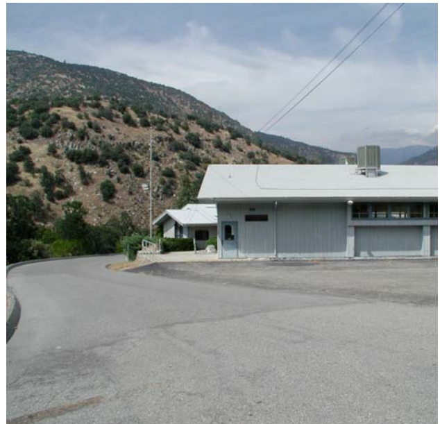
Above: Chawanakee School at SCE's former Powerhouse 3 community, view northeast but only shows one end of the building (mid-afternoon). (P6180043.JPG)
