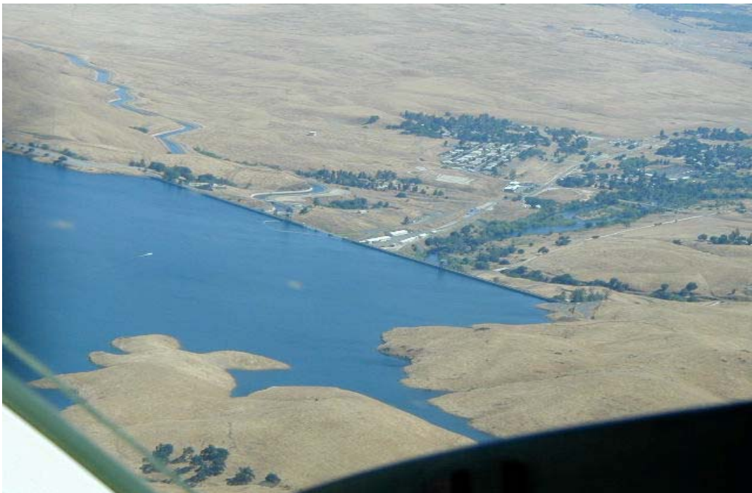
Picture: P5290030 Air photo Millerton Lake and Friant Dam looking south-west.
