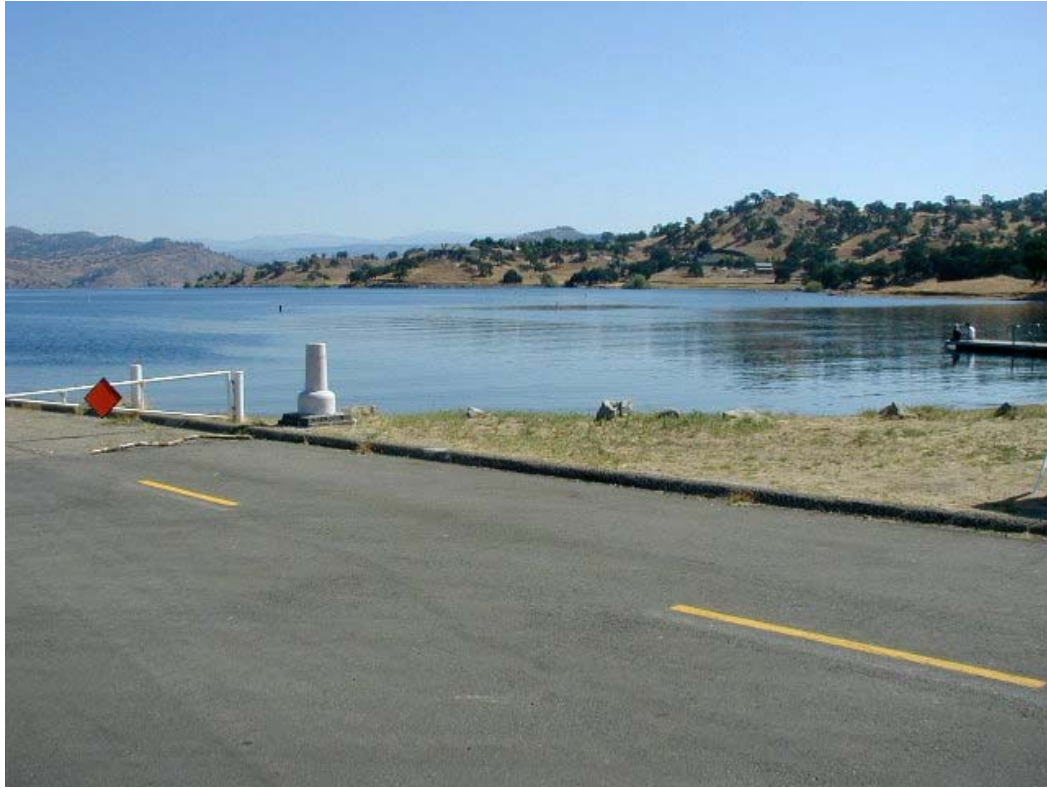
Picture: P5290092 Friant Dam dock area. South shoreline, looking north.
