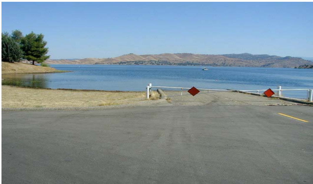
Picture: P5290093 Friant Dam dock area. South shoreline, looking north.
