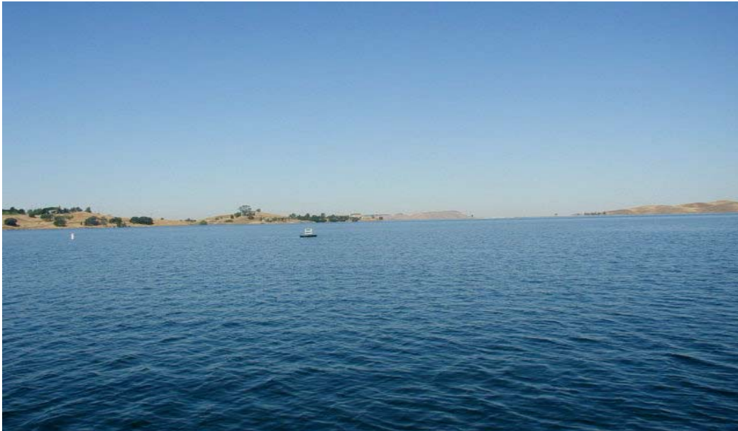
Picture: P5290095 Millerton Lake from boat near south shoreline looking north-west. Friant dam toward right of photo.
