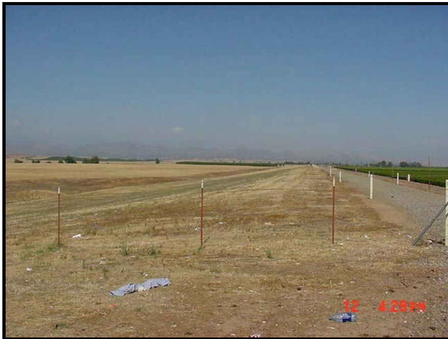
Eastward view along embankment
