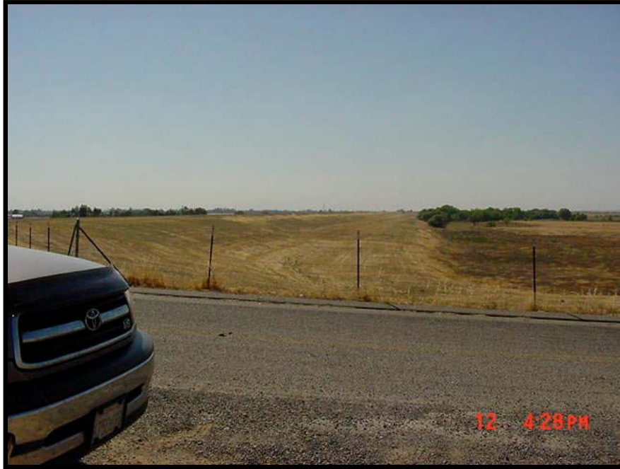
Dry Creek – Westward view along Big Dry Creek embankment
