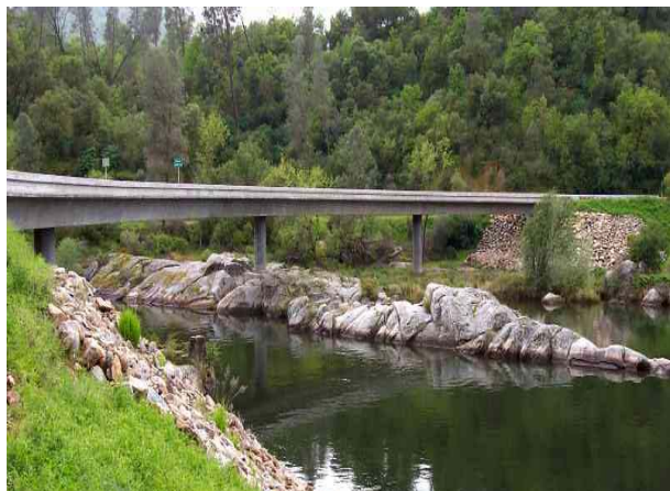
Bridge over San Joaquin River at Kerckhoff Lake
