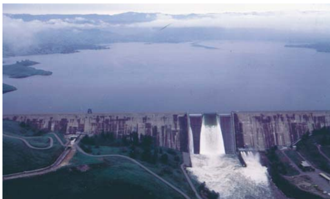
Friant Dam – January 1997 Flood Release
