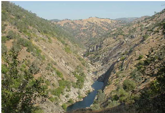
Temperance Flat RM 286 Dam Site on the San Joaquin River
