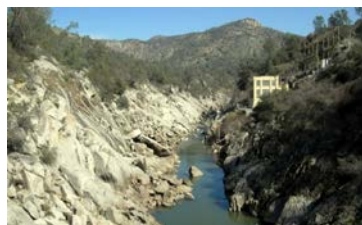
San Joaquin River near Kerckhoff Powerhouse
