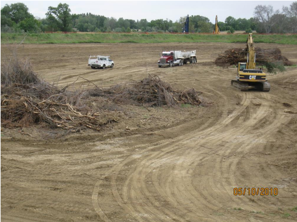
Clearing and Grubbing the sediment ponds.
