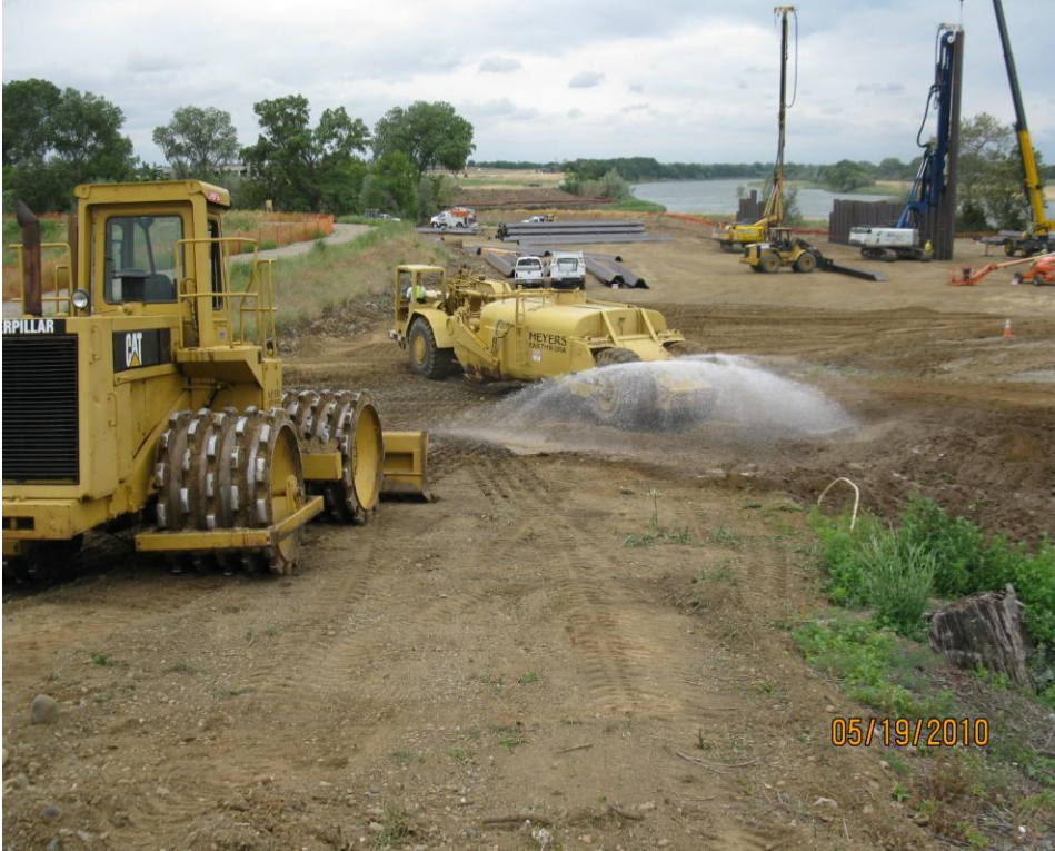
Compacting fill and controlling the dust.
