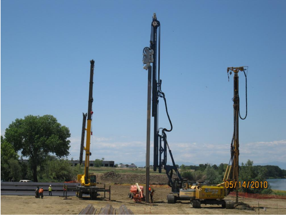
Driving Sheet Piles.
