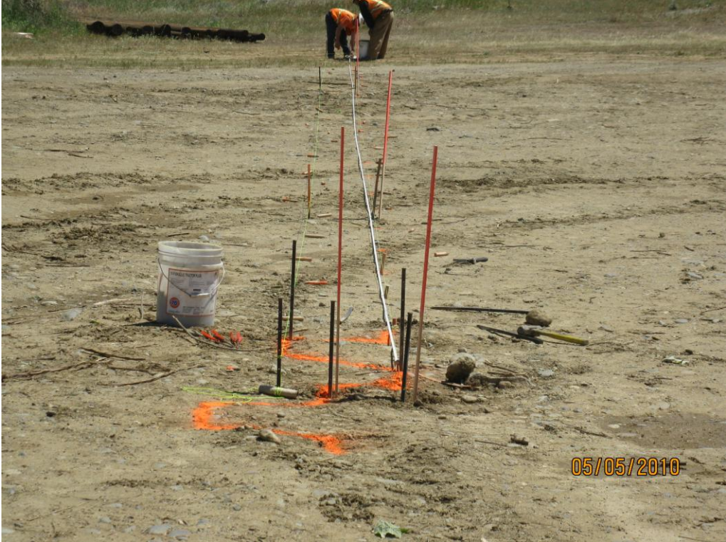
Laying out the Sheet Pile locations.
