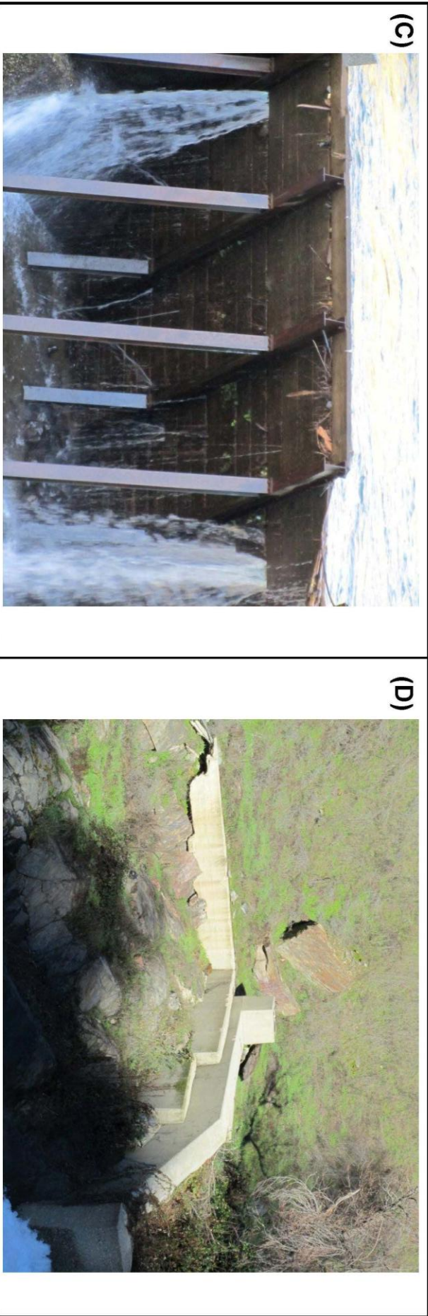
Stanislaus Afterbay Dam Removal EA Project Figure 1 Stanislaus Afterbay Dam - Existing Dam Condition Calaveras and Tuolumne Counties, California Notes: Photo (A): Timber Facing and Steel Buttresses Photo (B): Top of the Center Concrete Gravity Section and Left Buttress Photo (C): Degraded Timbers Photo (D): Right Buttress
