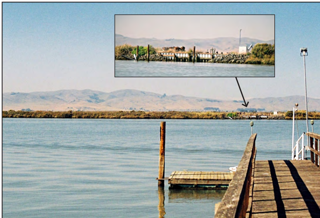
Photo 4. This photo depicts common infrastructure in the marsh including a pier and pylons, outfall structure, and riprap (inset). The building in the inset photo is the lower Joice Island Fish Screen Facility.
