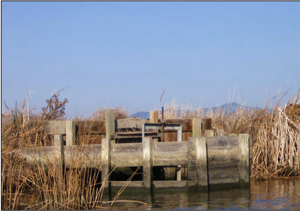
Photo 3. This photo depicts an outfall structure that is common to the project area.
