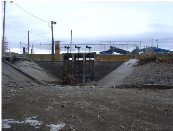
a) Photo from upstream of existing C-Canal intake structure showing three sluice gates
