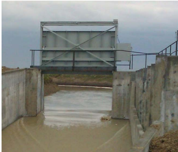
a) Typical roller gate in open position.
