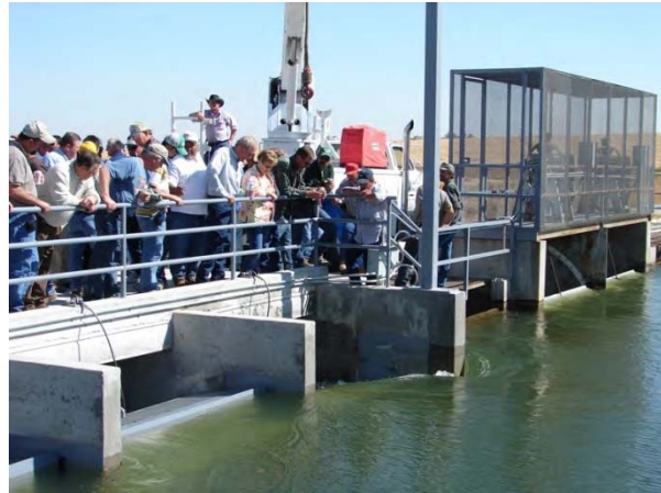
c) Typical automatic trip gates (one closed, one open).
