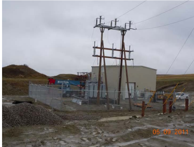
Figure 8. Example of interconnect substation.
