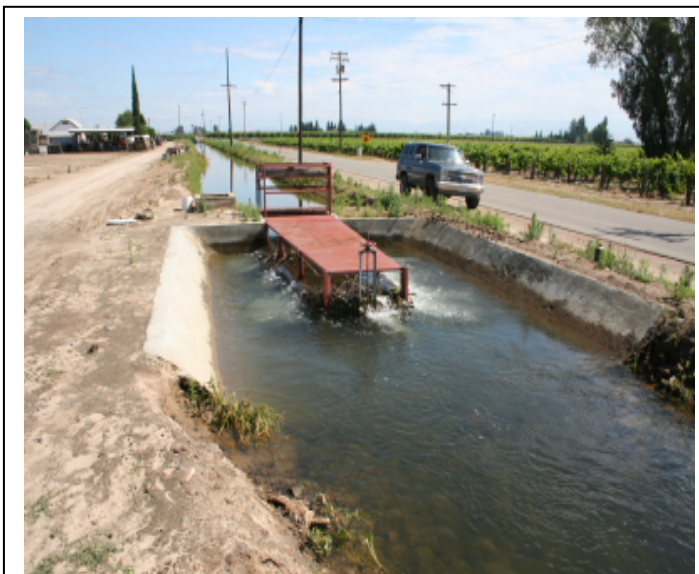
Figure 9. View north along canal at Long Crested check weir.
