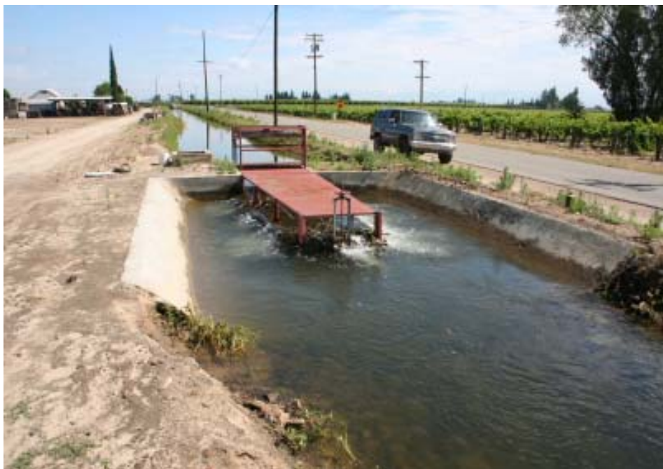
Figure 1. View north along Briggs Canal at Long Crested check weir at Fowler Avenue.
