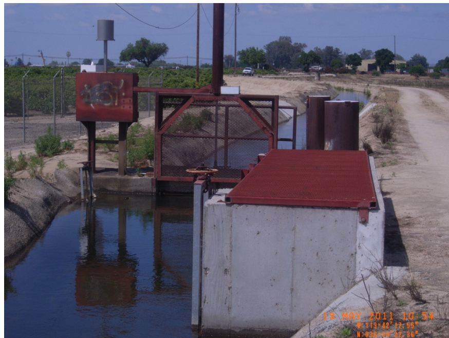
Photo 8: View west of Briggs Canal facilities with manual and automated controls at upstream end of project area.
