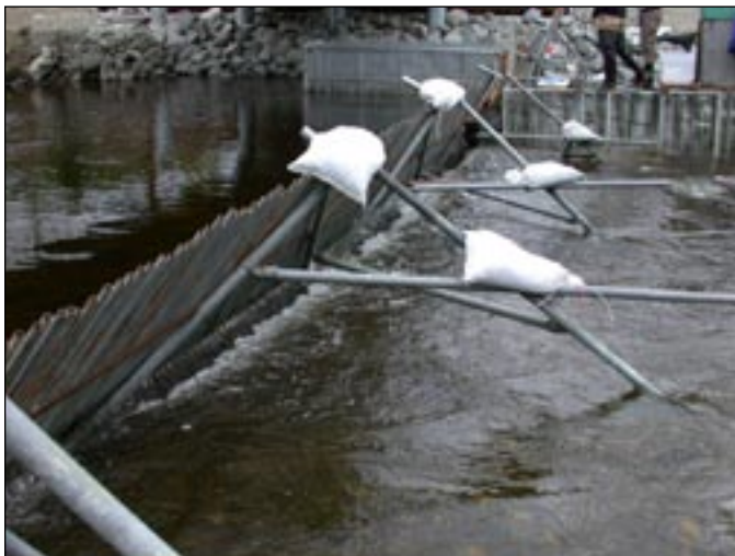
FIGURE 3. — Construction details of tripods and weir panels made of metal stringers and pickets of galvanized electrical conduit.
