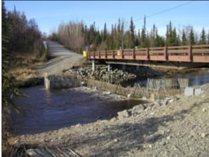
FIGURE 1. — A temporary weir constructed of metal tripods, stringers, and galvanized conduit with both an upstream and downstream trap. Ninilchik River, Alaska.
