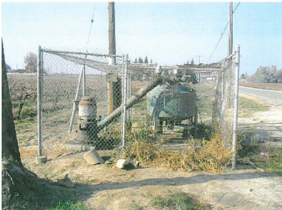
Photograph 6. Existing irrigation well and filter station that could be used as a recovery well. Well is adjacent to Lincoln Avenue near the northern line of the southern boundary.
