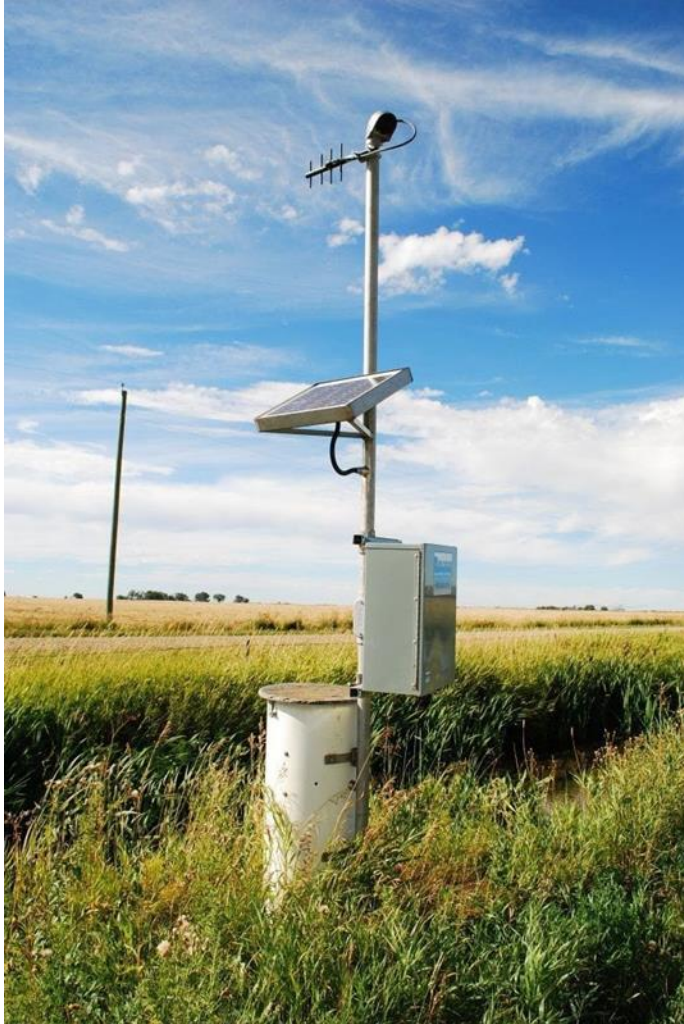
Figure 1. Wireless SCADA System Example. Source: Aqua Systems 2000 (2024)
