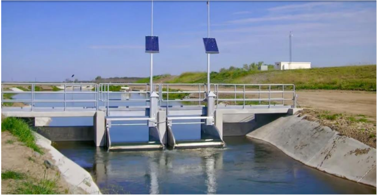
Figure 2. Automated Gate Example. Source: Rubicon (2024)
