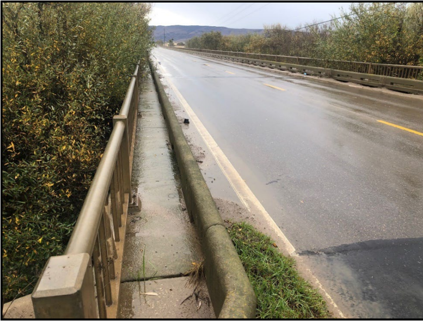
FIGURE 5: 16-inch walkways spanning the Highway 1 Bridge
