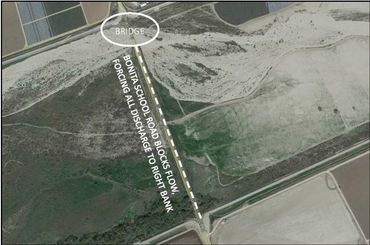
FIGURE 2: Bonita School Road Bridge (soon to be demolished)
