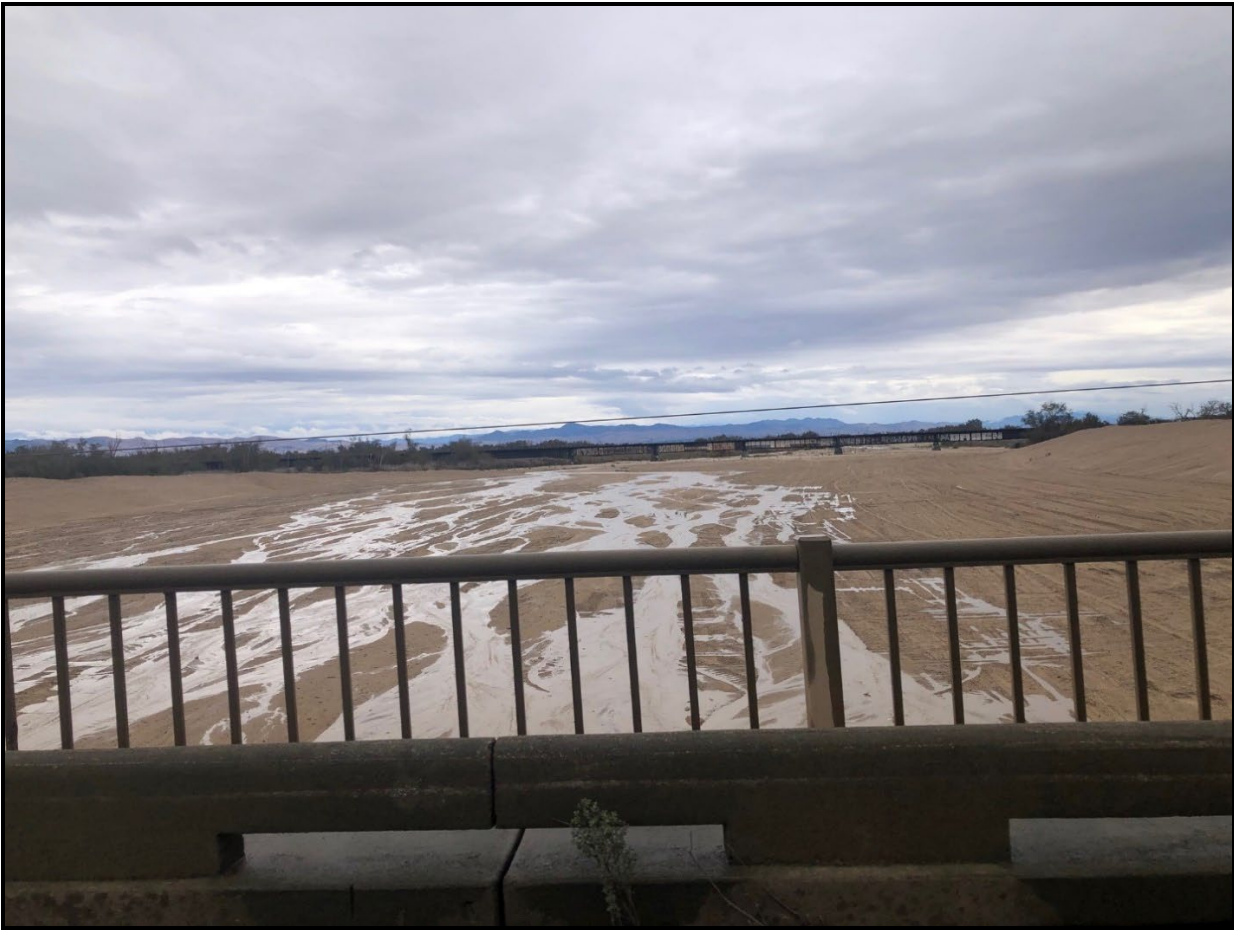
FIGURE 6: Upstream view from Highway 1 Bridge. Wide, unstable sand channel prone to severe scour and fill will meander at different flow regimes.
